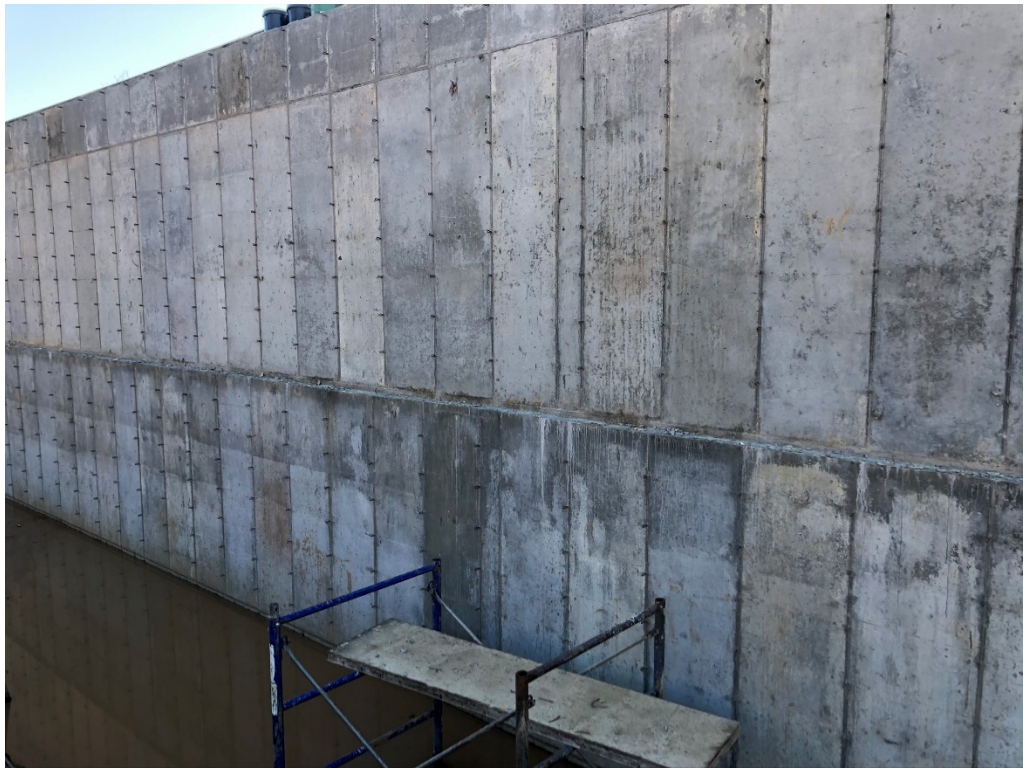
Figure 11 – Foundation Wall, Earth-side
