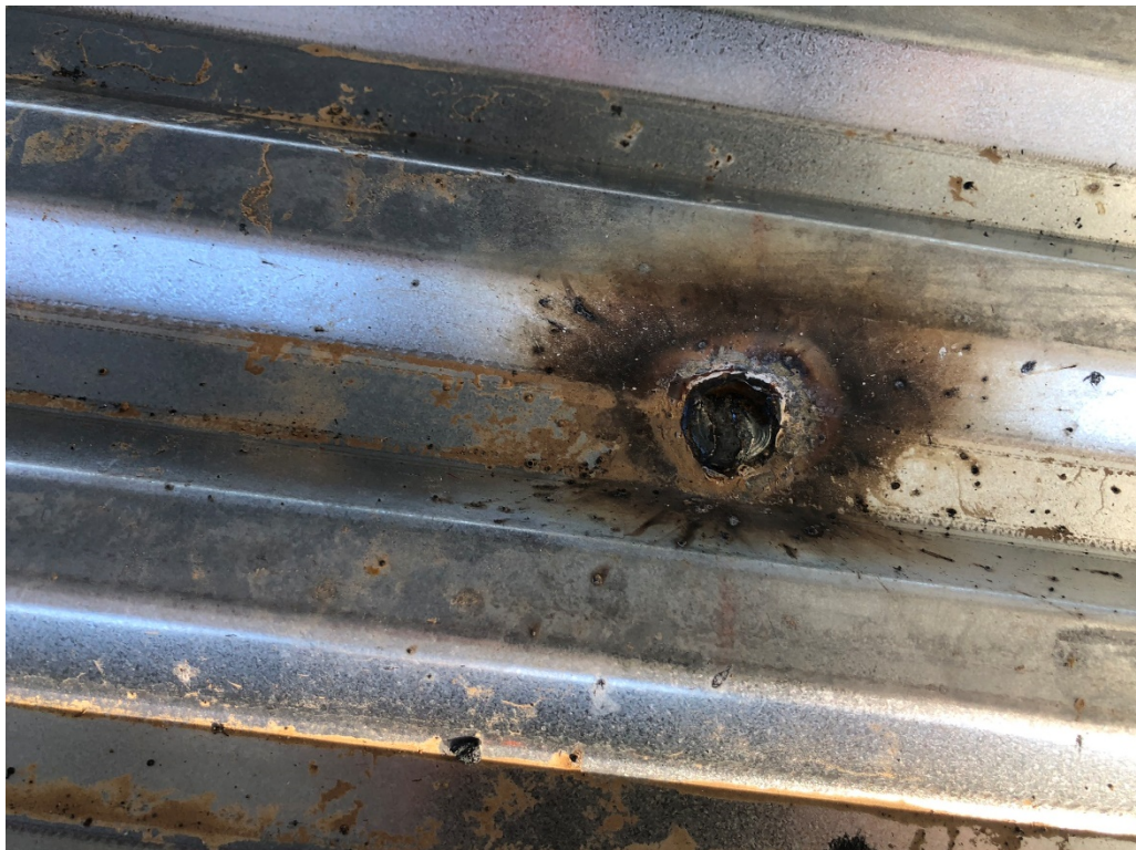
Figure 4 – Spot Welds through Decking (typical)
