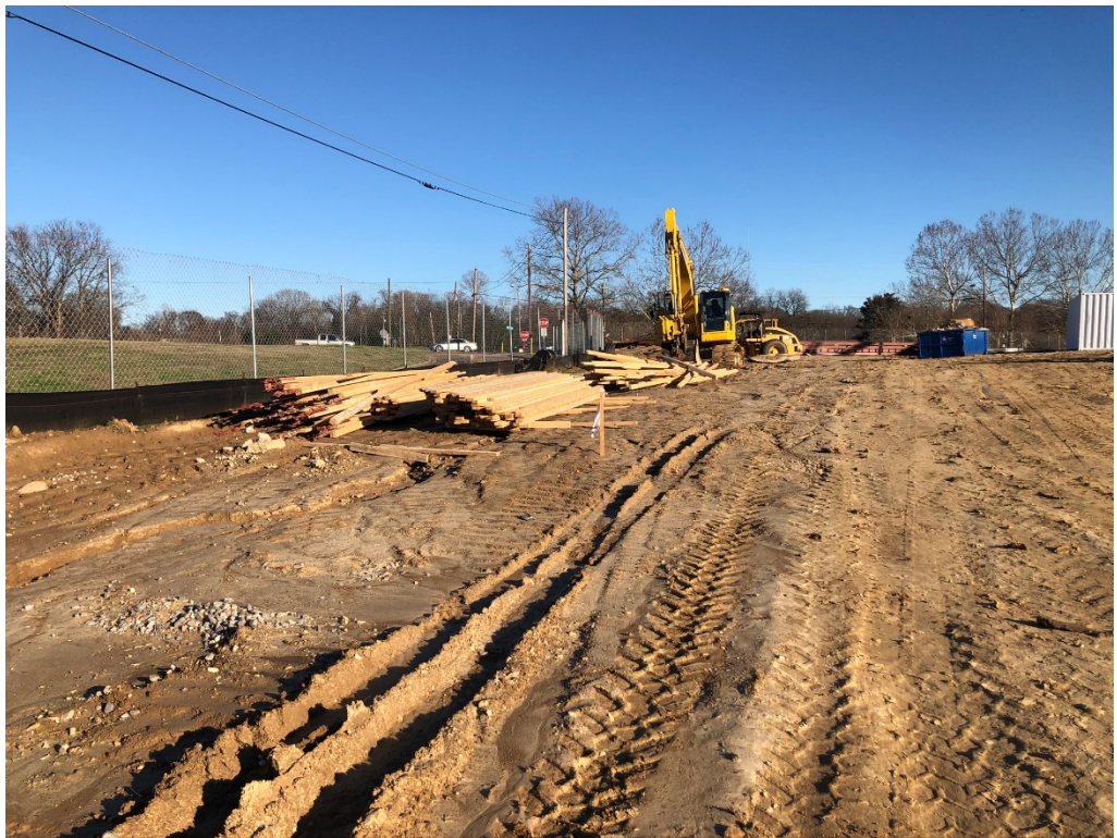
Figure 18 – Stored Lumber On-site
