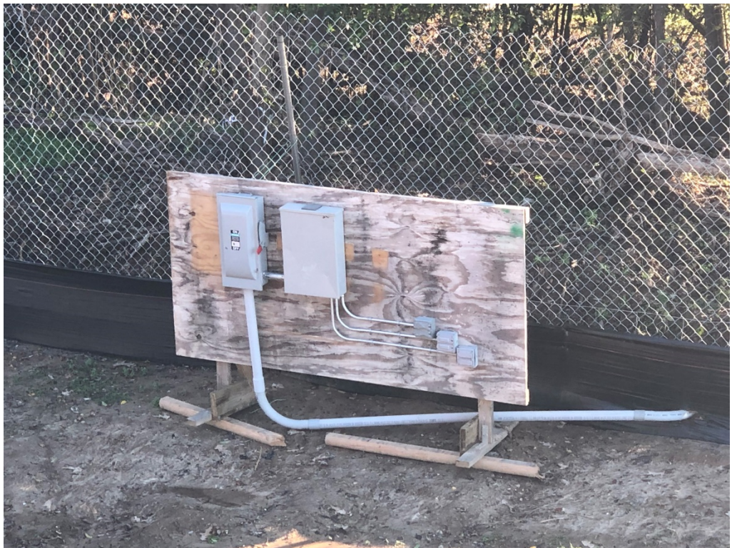
Figure 6 – Onsite Temporary Electrical Service
