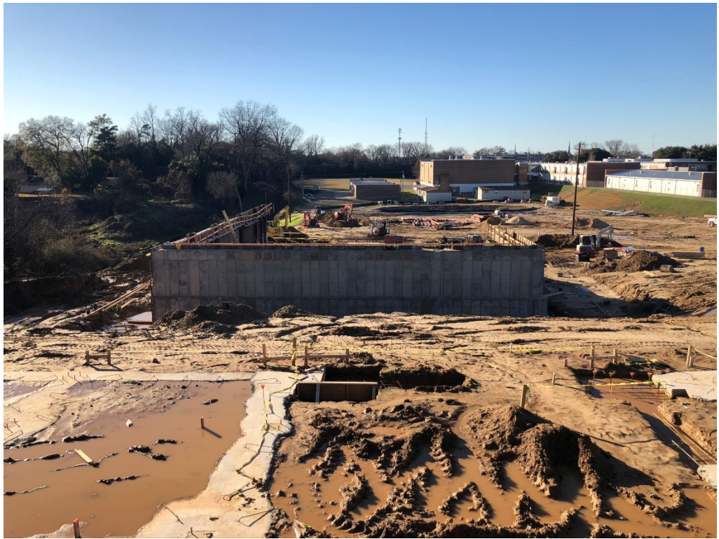
Figure 5 – Foundation Wall Progress
