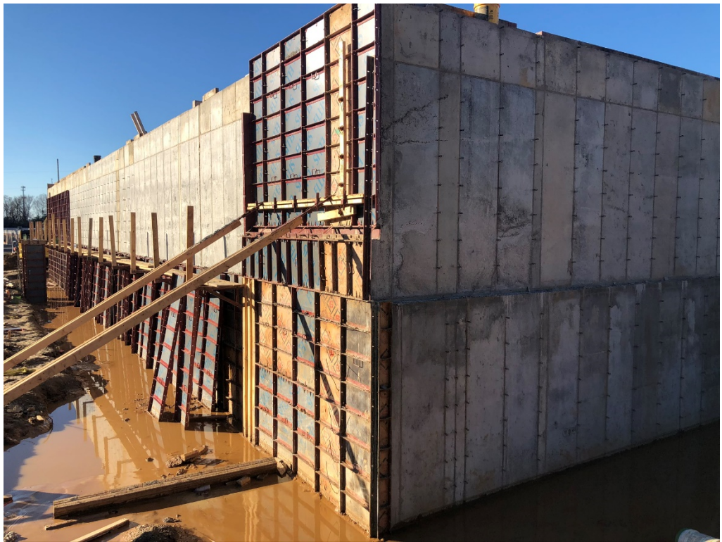
Figure 12 – Foundation Wall, Earth-side, Southeast Corner
