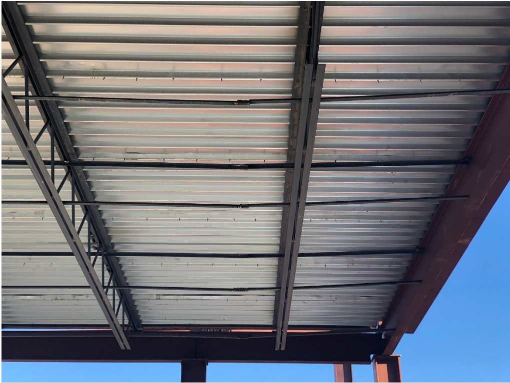
Figure 7 – 2 nd Floor Roof Decking from Below
