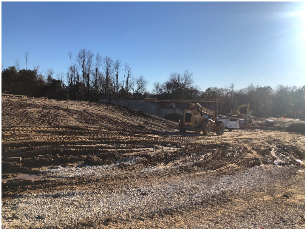
Figure 16 – North Entry Looking South
