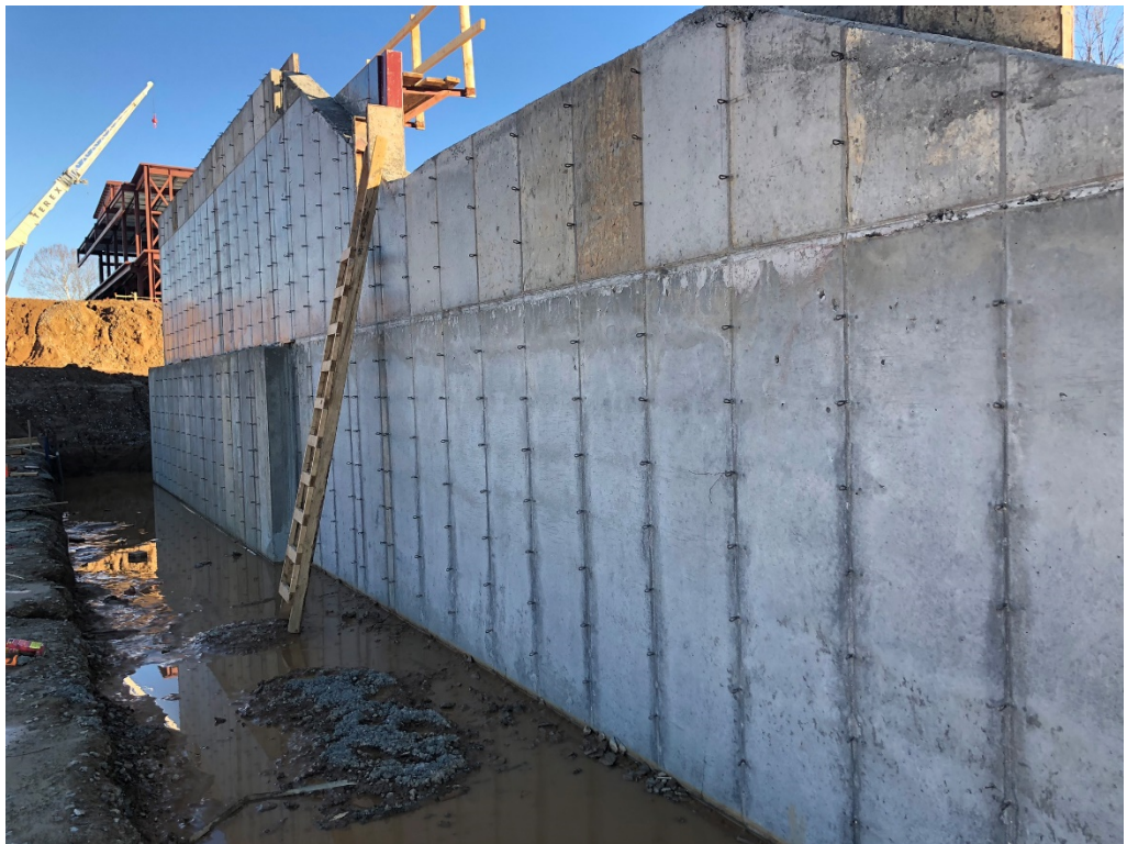
Figure 14 – North Foundation Wall, Earth-side
