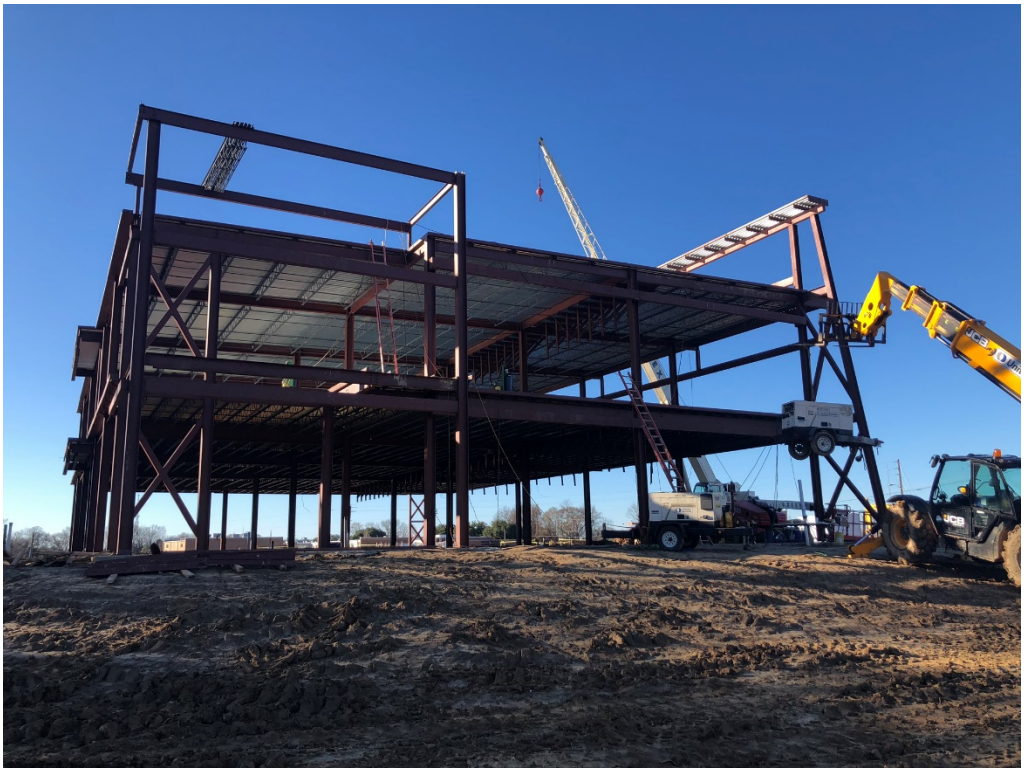
Figure 1 – Red Steel Erected
