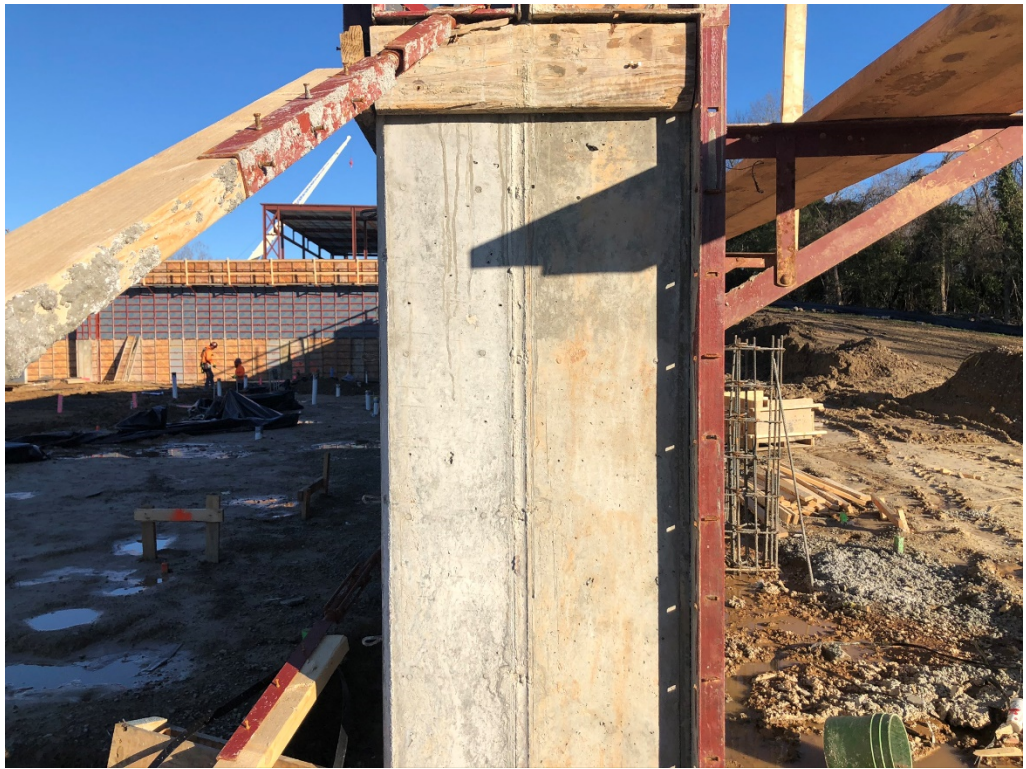
Figure 13 – West Edge of Foundation Wall
