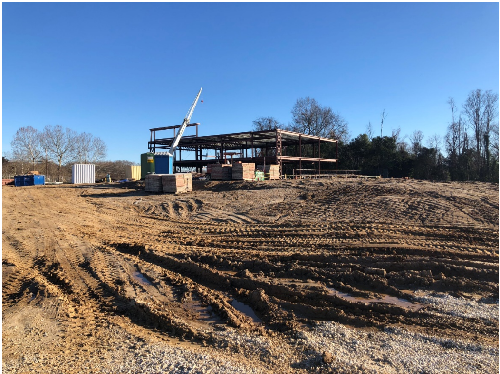
Figure 15 – North Entry Looking East SE
