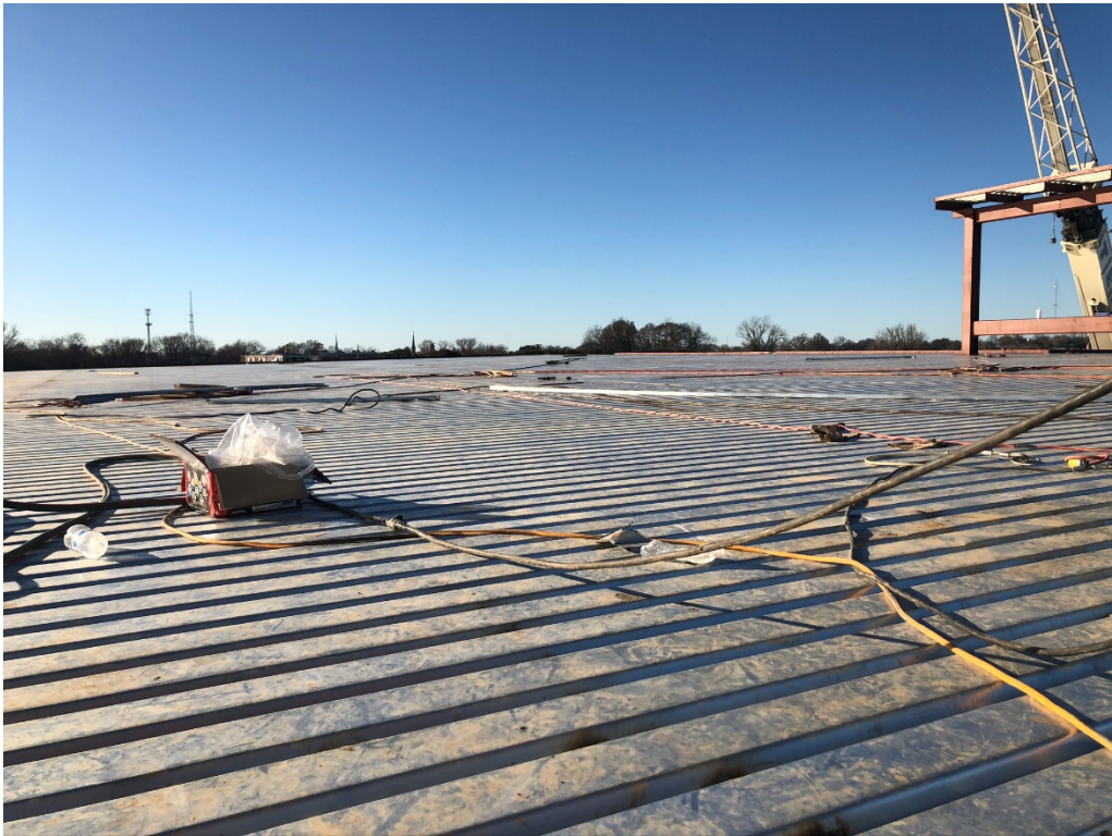
Figure 8 – Roof Deck Platform East Looking Northeast
