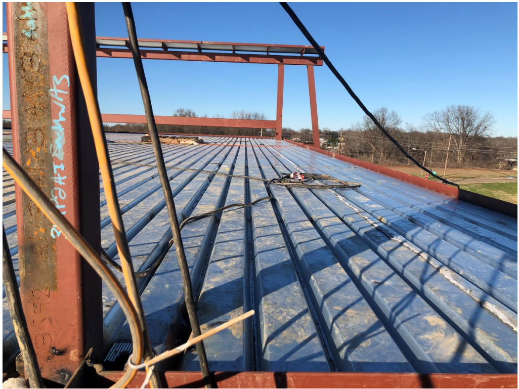
Figure 9 – Roof Deck Platform East Looking North
