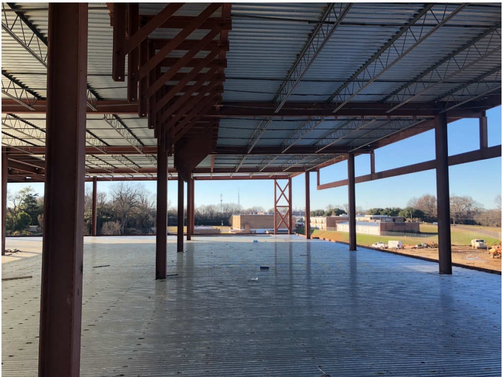
Figure 2 – 2 nd Floor Platform from East Looking West
