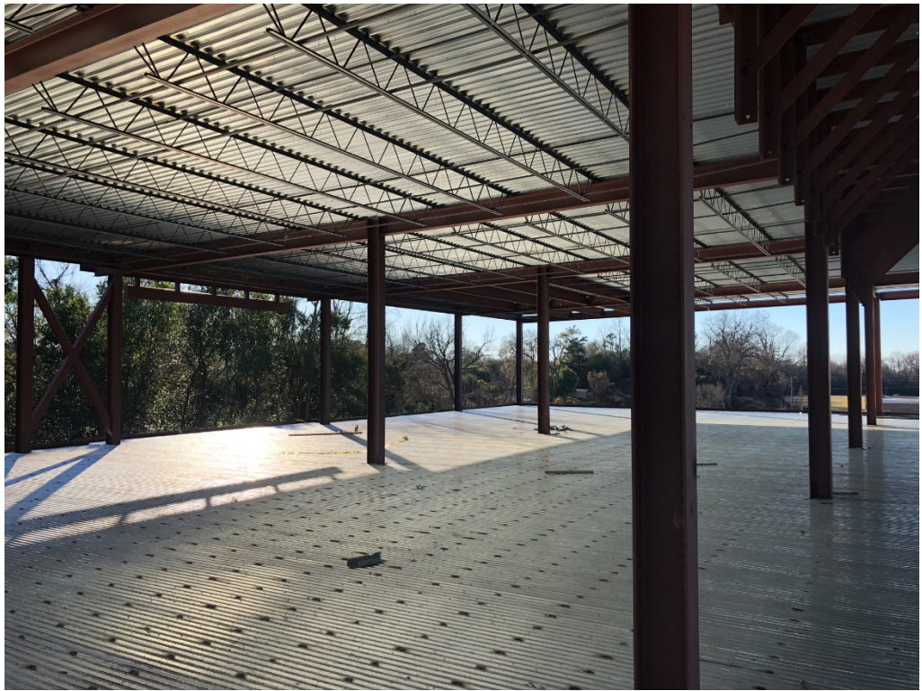
Figure 3 – 2 nd Floor Platform from East Looking Southwest
