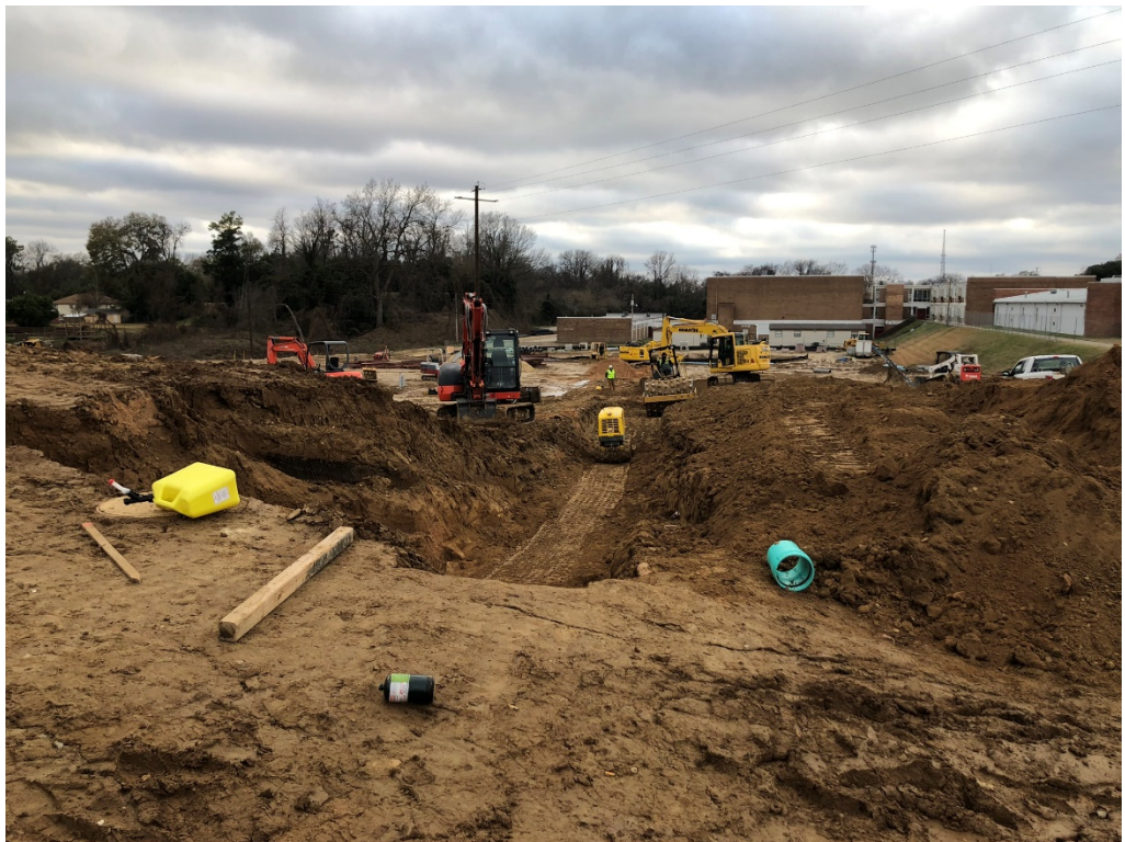
Figure 6 – Sewer Line Trenching
