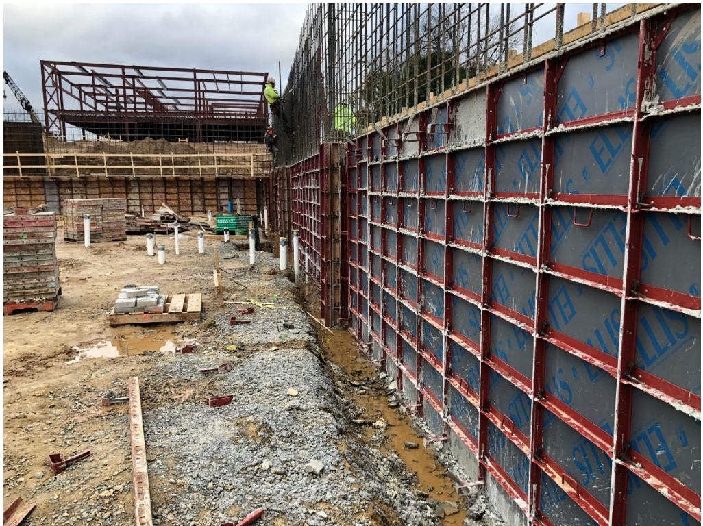
Figure 12 – Lower Level SW Corner looking E
