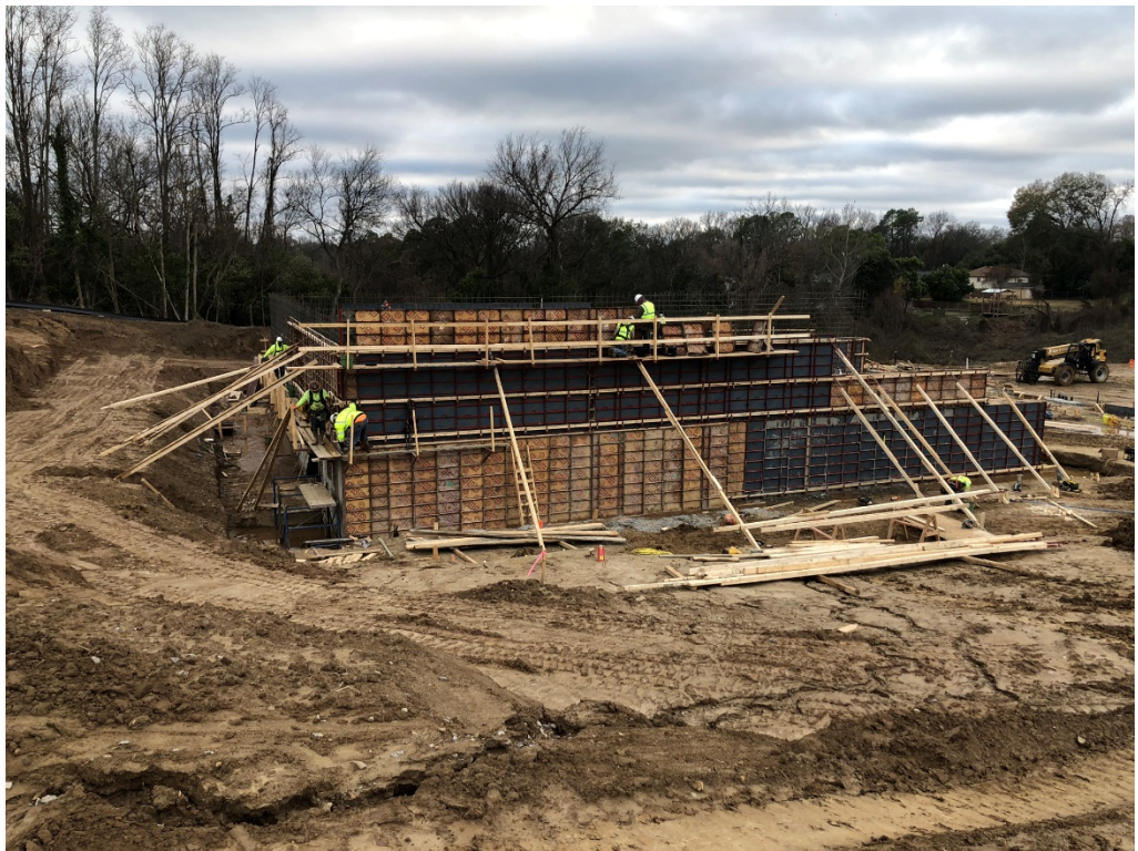
Figure 10 – Foundation Work at Lower Level
