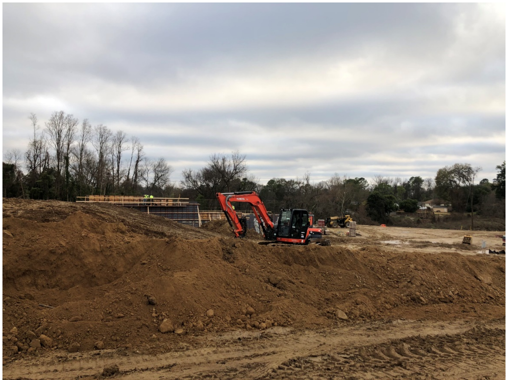
Figure 8 – North Entry Looking S
