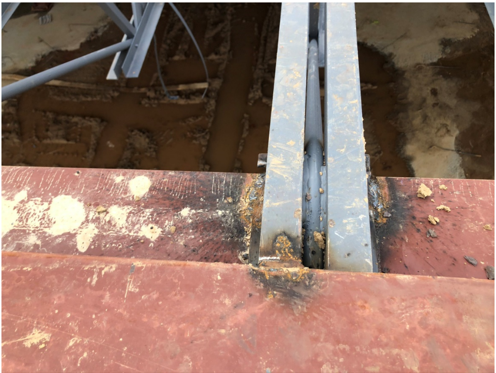
Figure 2 – Field Weld (typical)
