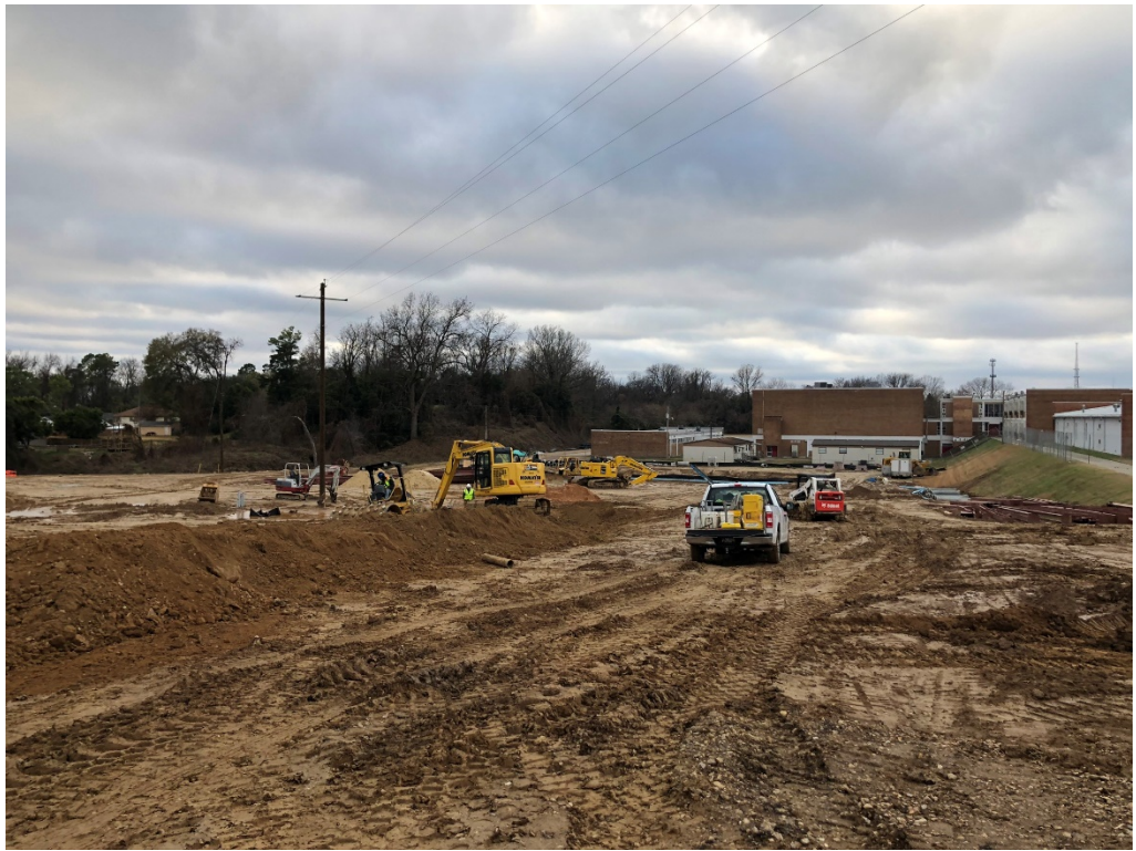
Figure 7 – North Entry Looking WSW
