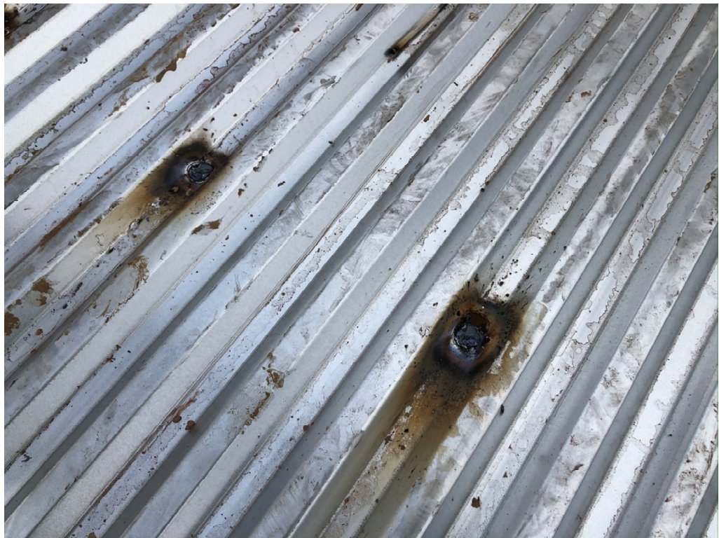
Figure 4 – Spot Welds through Decking (typical)
