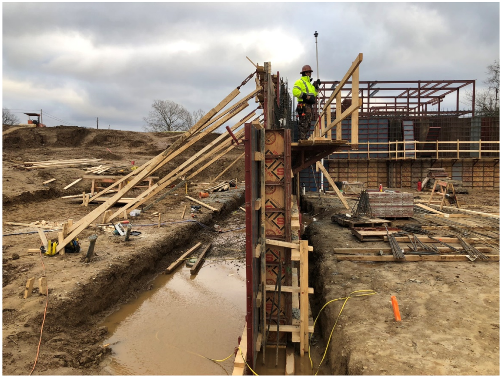
Figure 11 – Bracing and Walk Boards for Foundation Work (typical)
