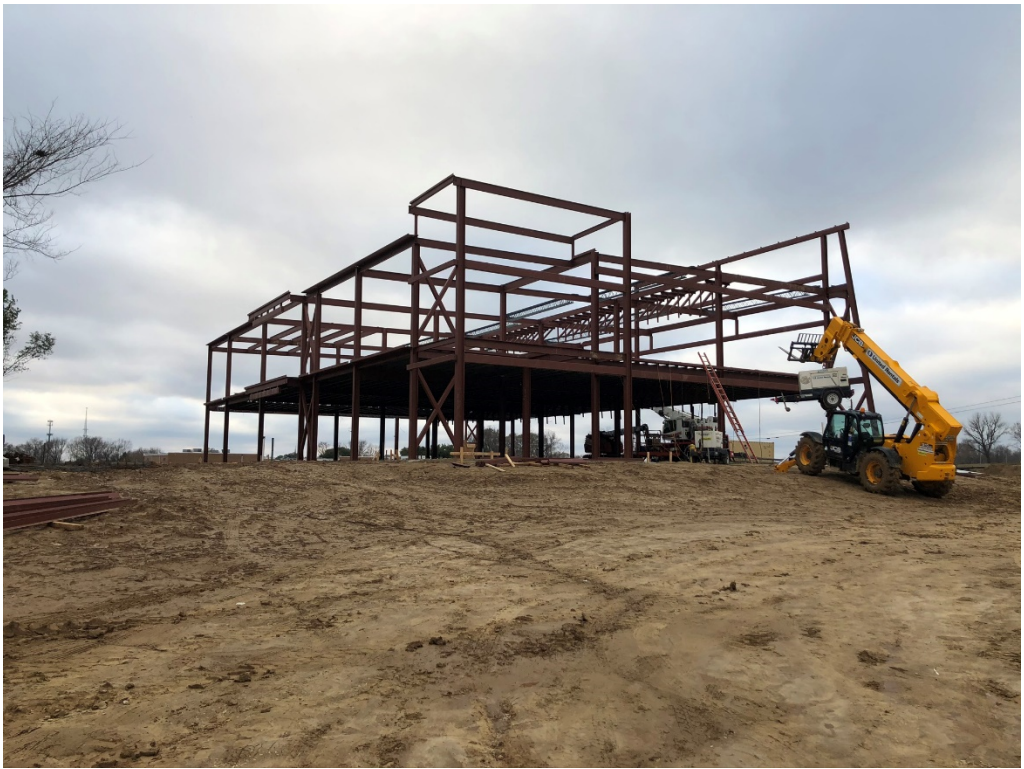
Figure 1 – Red Steel Erected
