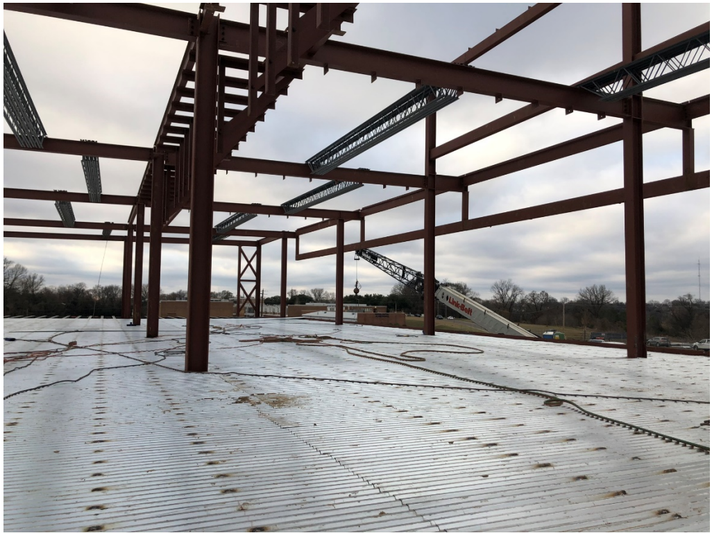
Figure 3 – Steel Deck Installed at Upper Level
