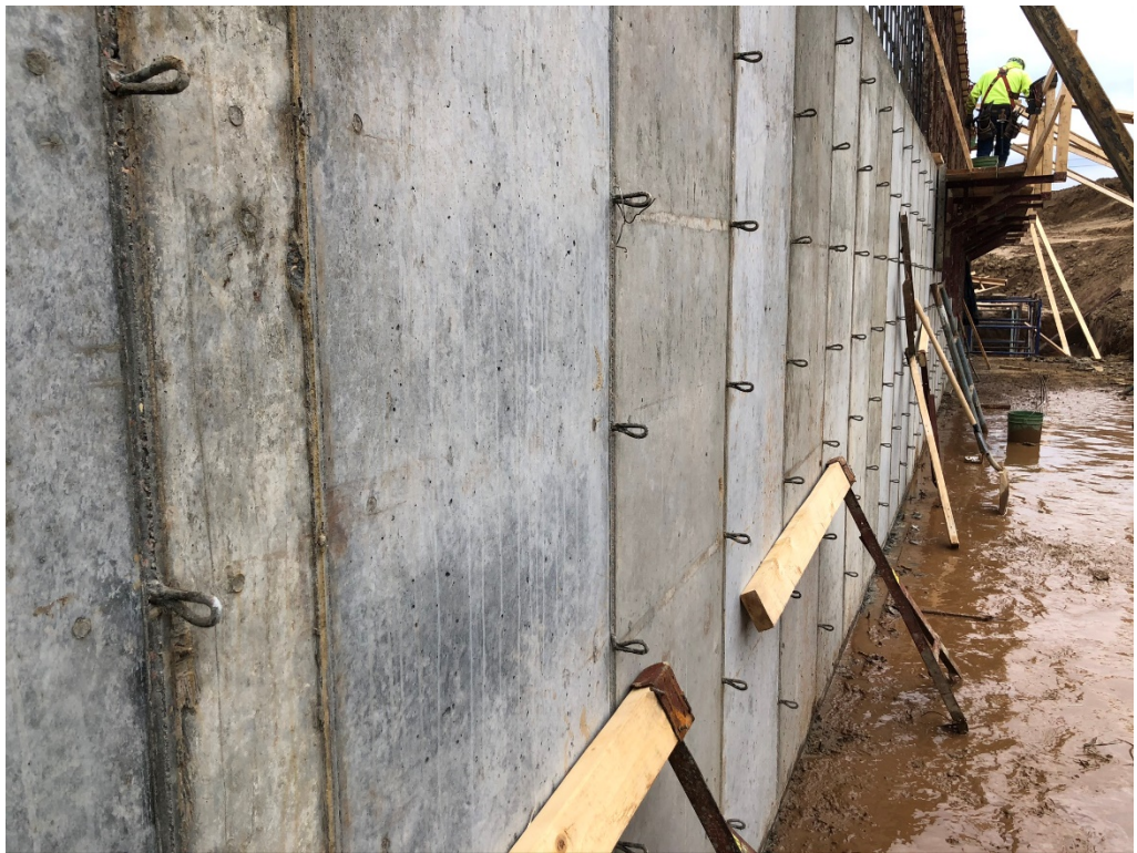
Figure 14 – Removed Forms from Retaining Wall (dirt side)
