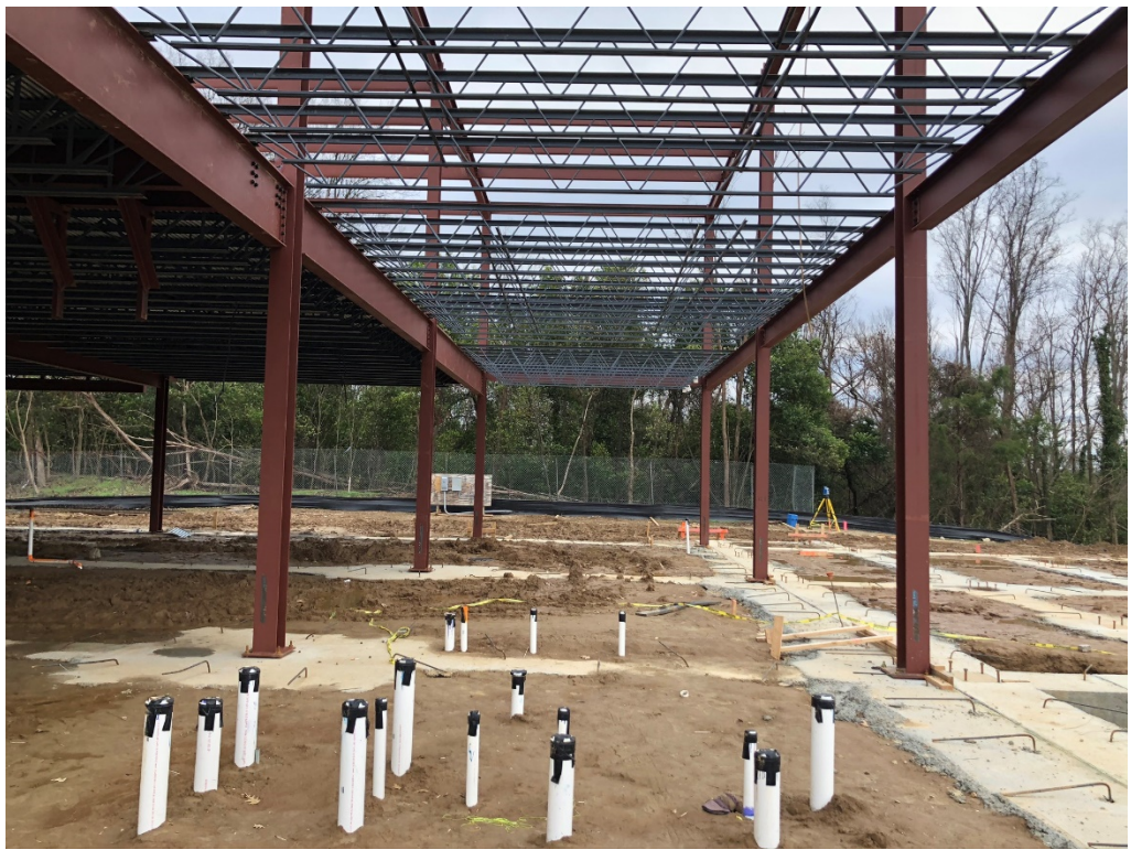
Figure 5 – Steel Joists Laid out and ready for Deck
