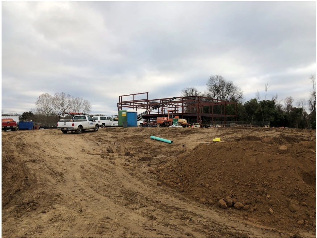
Figure 9 – North Entry Looking ESE
