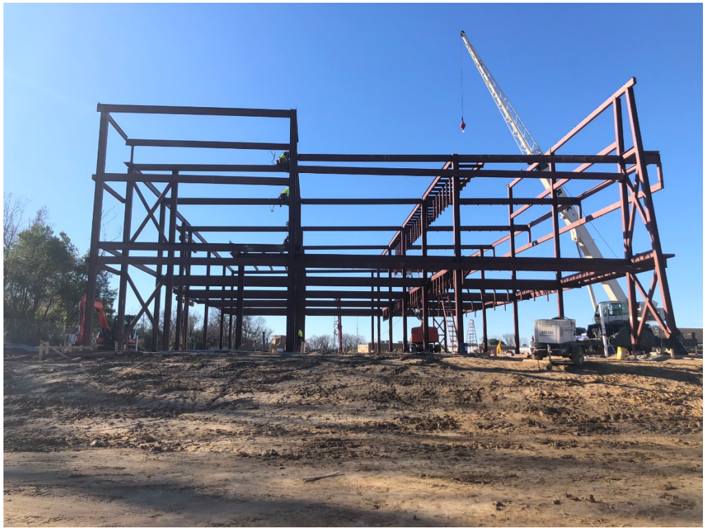
Figure 1 – Red Steel Erected
