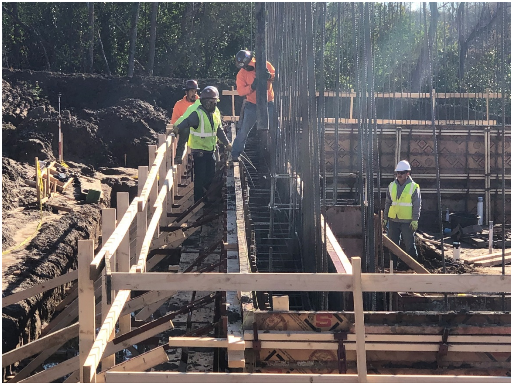
Figure 5 – Concrete work @ Foundation Wall
