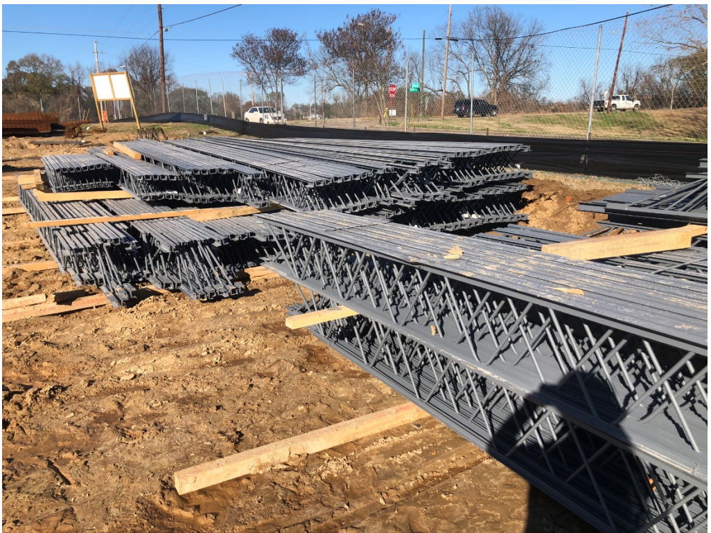
Figure 10 – Steel Trusses on Site
