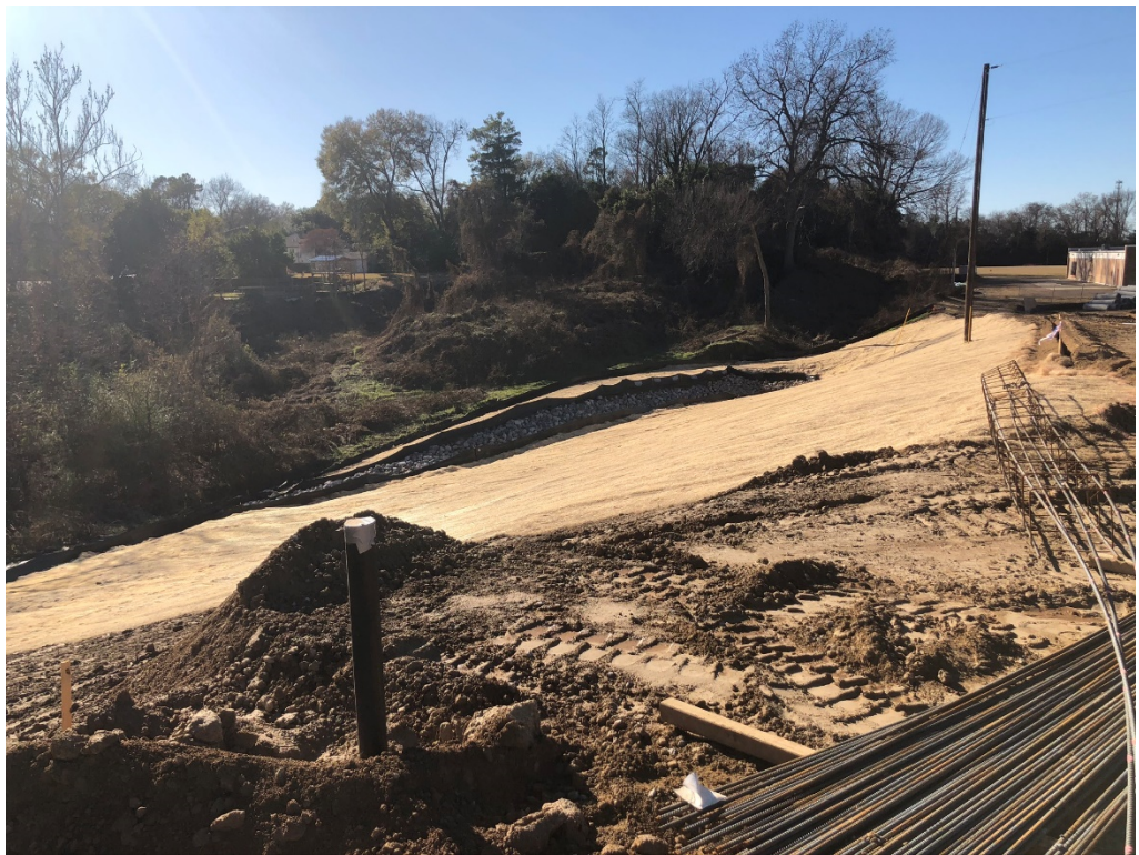
Figure 8 – Erosion Control Installed at Slope
