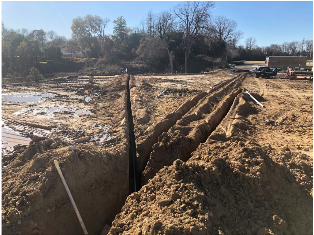
Figure 7 – Underground Conduit
