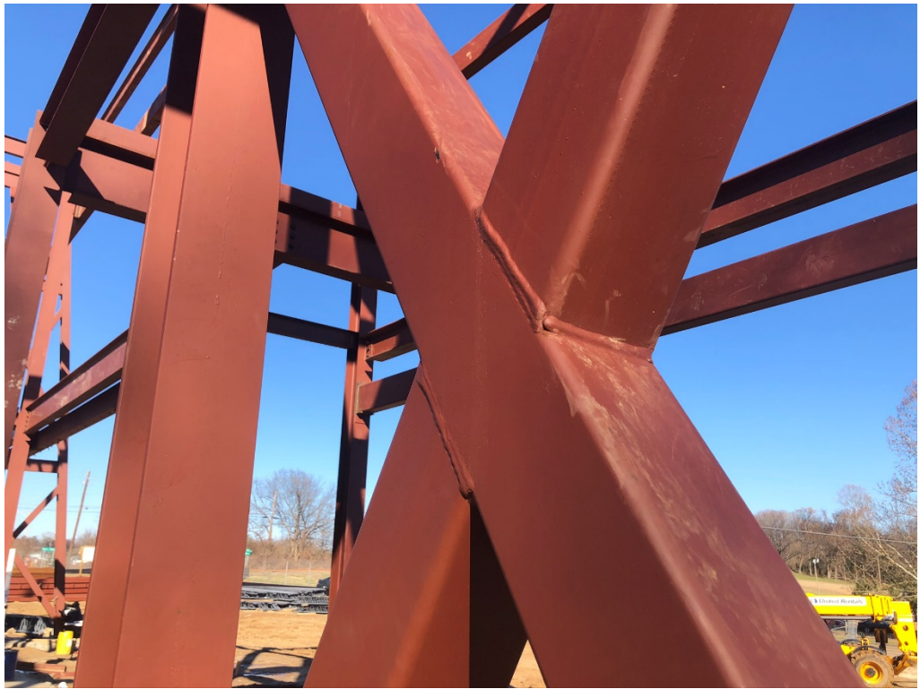
Figure 3 – Manufacturer Weld (typical)
