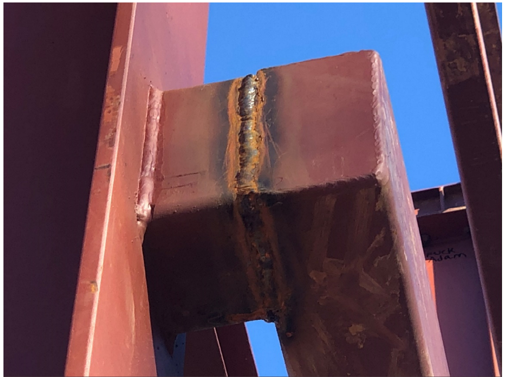
Figure 2 – Field Weld (typical)
