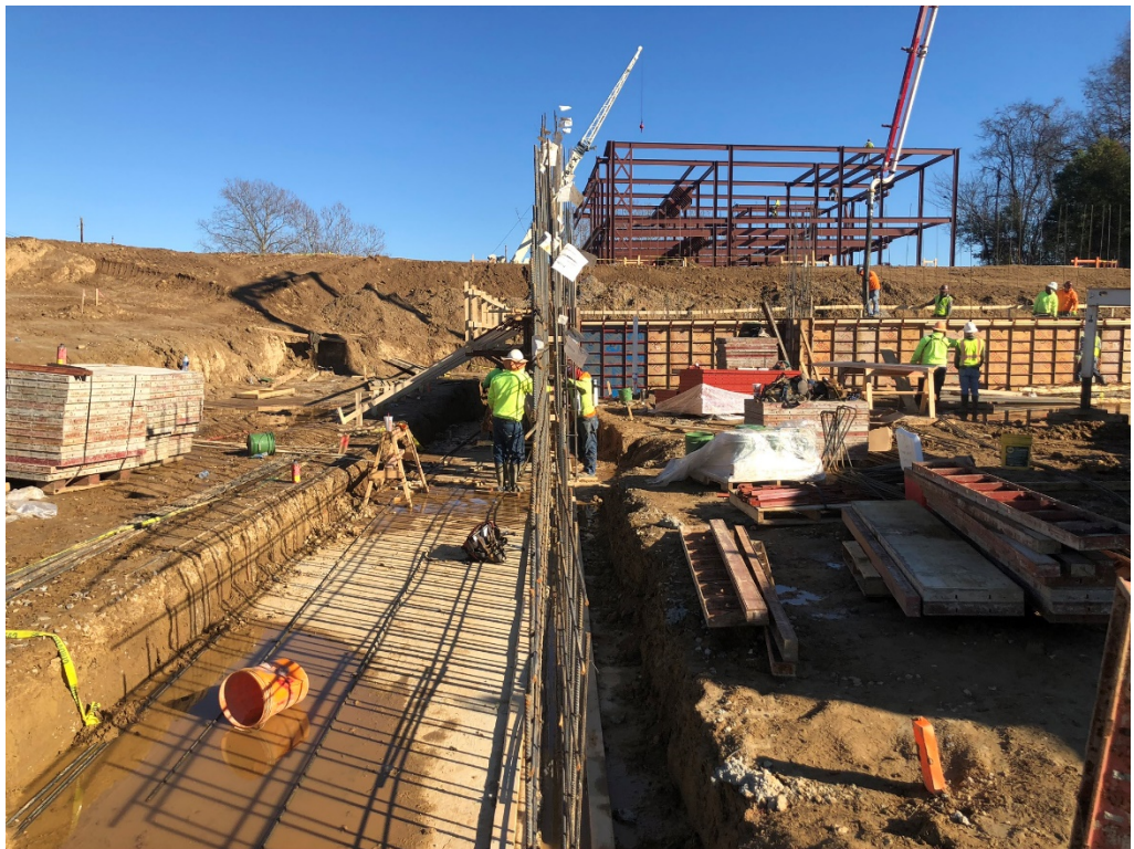
Figure 6 – Foundation Wall (rebar only)
