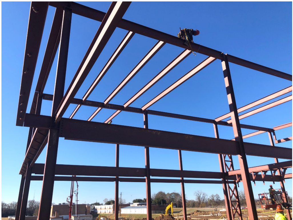
Figure 4 – Roof Girders being Set
