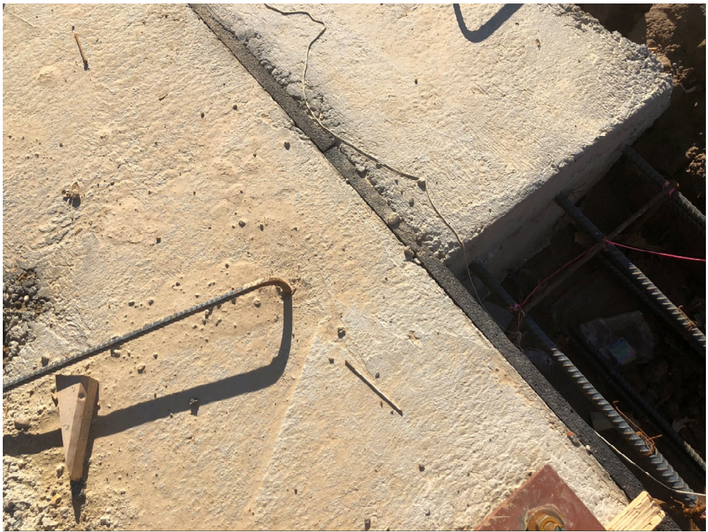
Figure 9 – Expansion joint between east and west upper building sections
