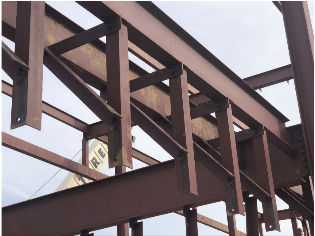
Figure 3 – Bolted Furr Down
