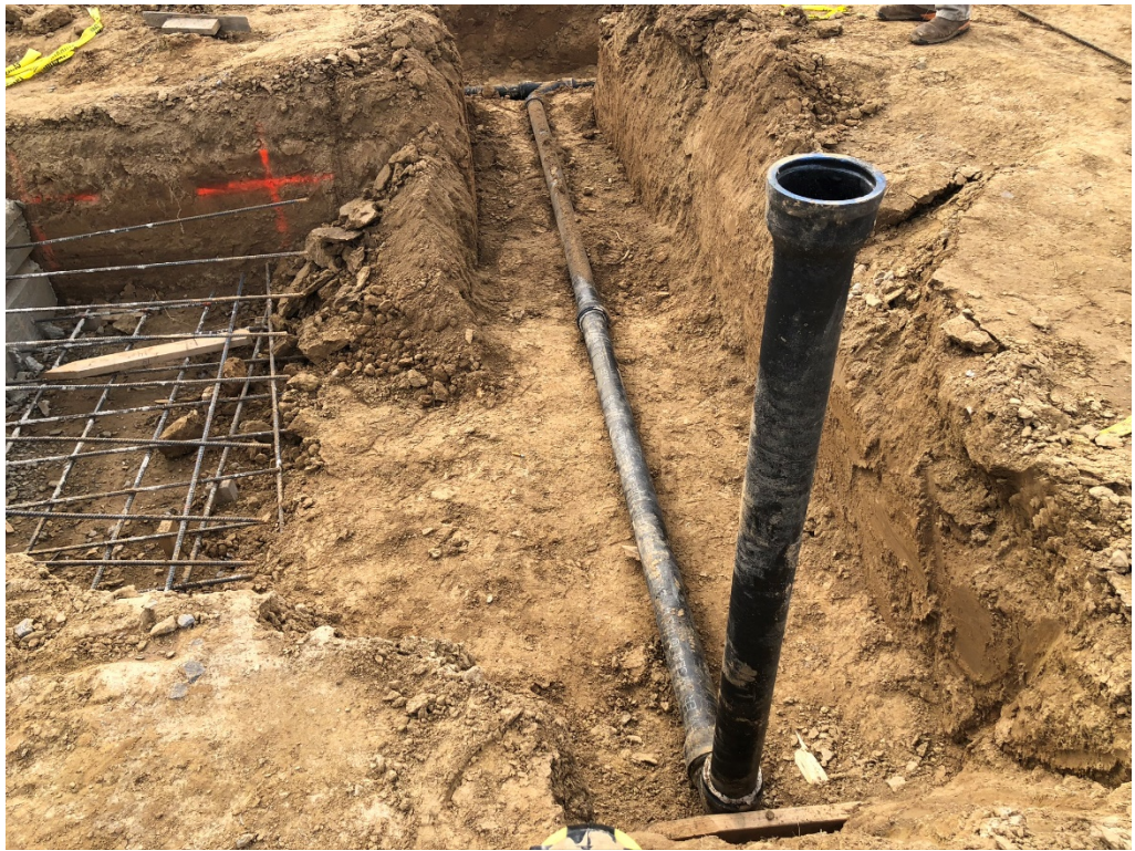
Figure 17 – Sewer Pipe for Head Test
