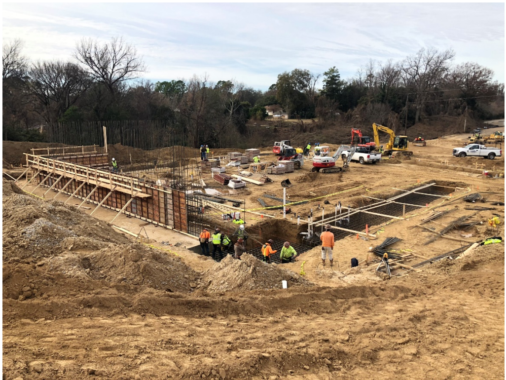
Figure 6 – Lower Level Foundation Work
