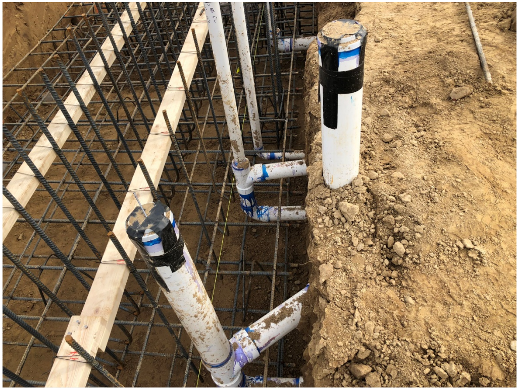
Figure 13 – Plumbing in Footing Pour
