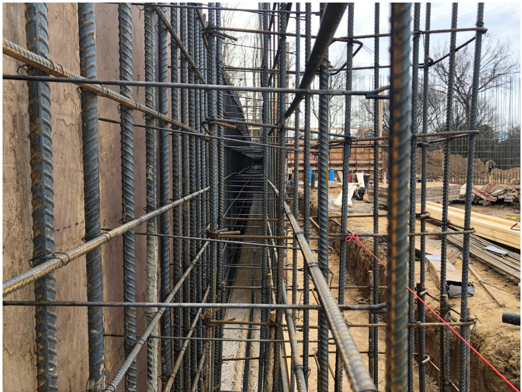
Figure 14 – Retaining Wall Rebar
