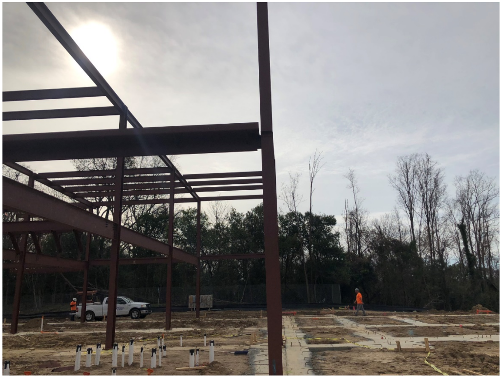
Figure 5 – Steel Plumb (typical)
