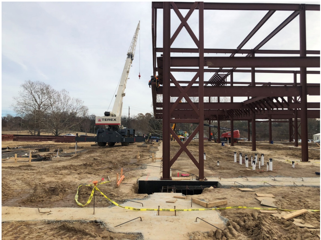
Figure 4 – Steel at Northwest Corner at Upper East Building
