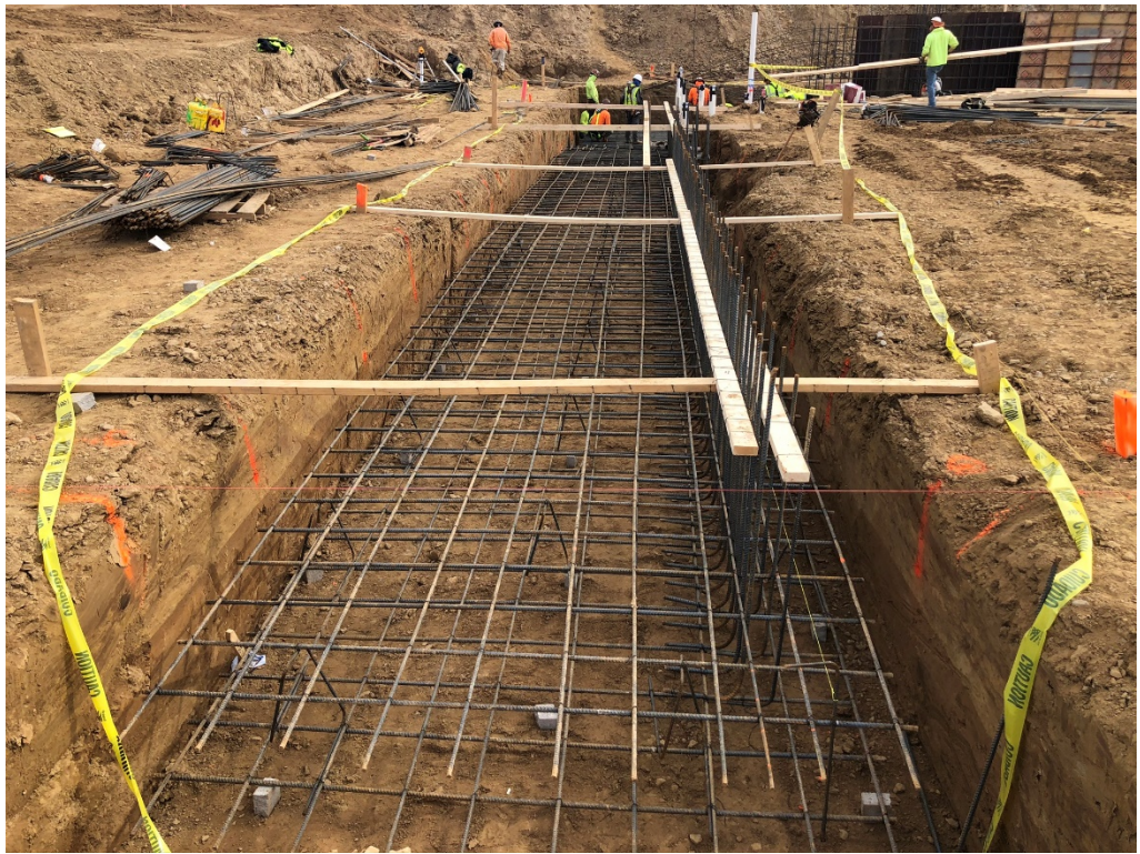
Figure 11 – North Footing on Lower Level
