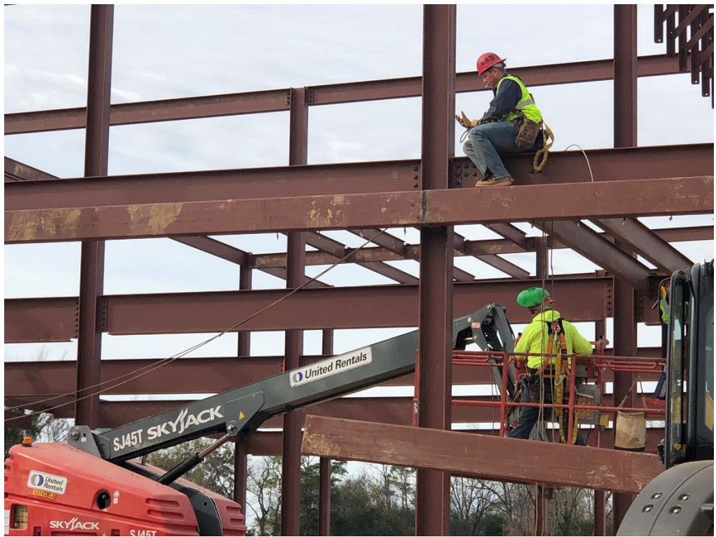
Figure 19 – East Welding Work and Erection
