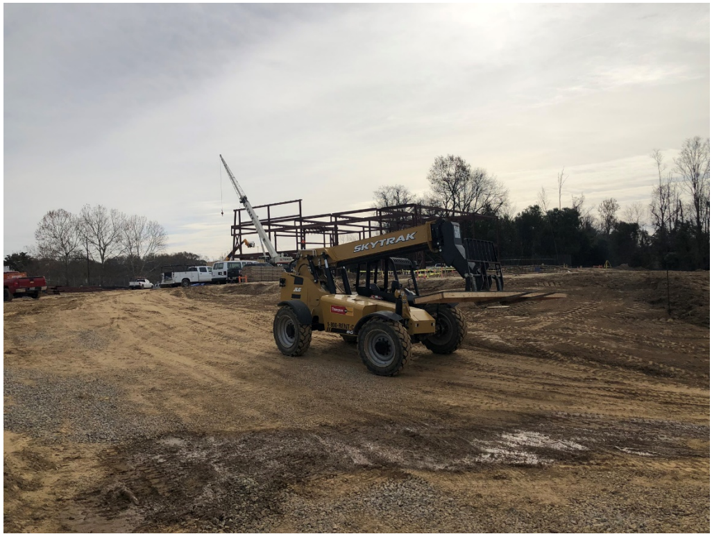
Figure 9 – North Entry Looking ESE
