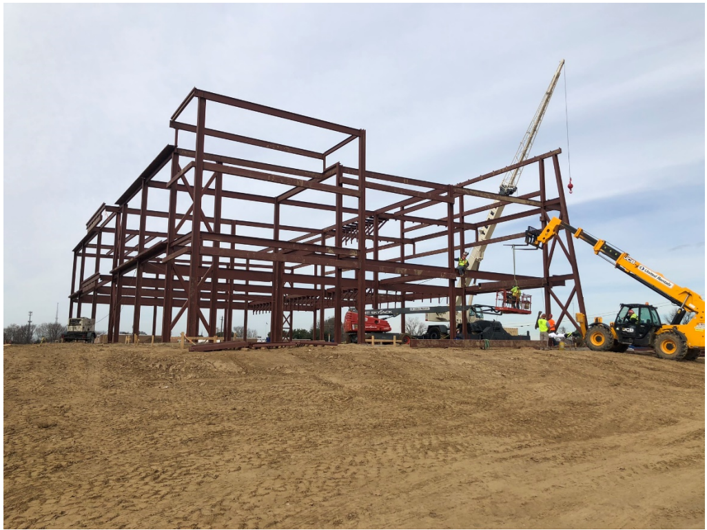
Figure 1 – Red Steel Erected
