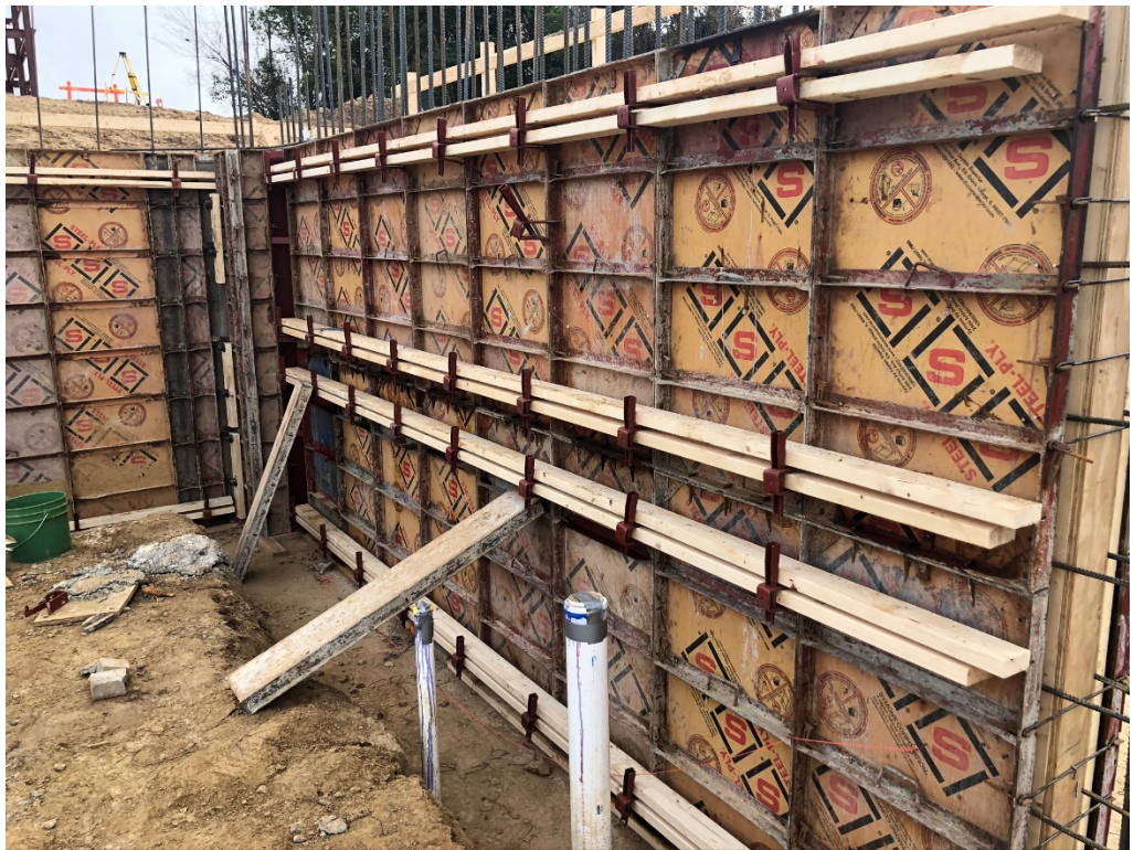
Figure 16 – Braced Retaining Wall
