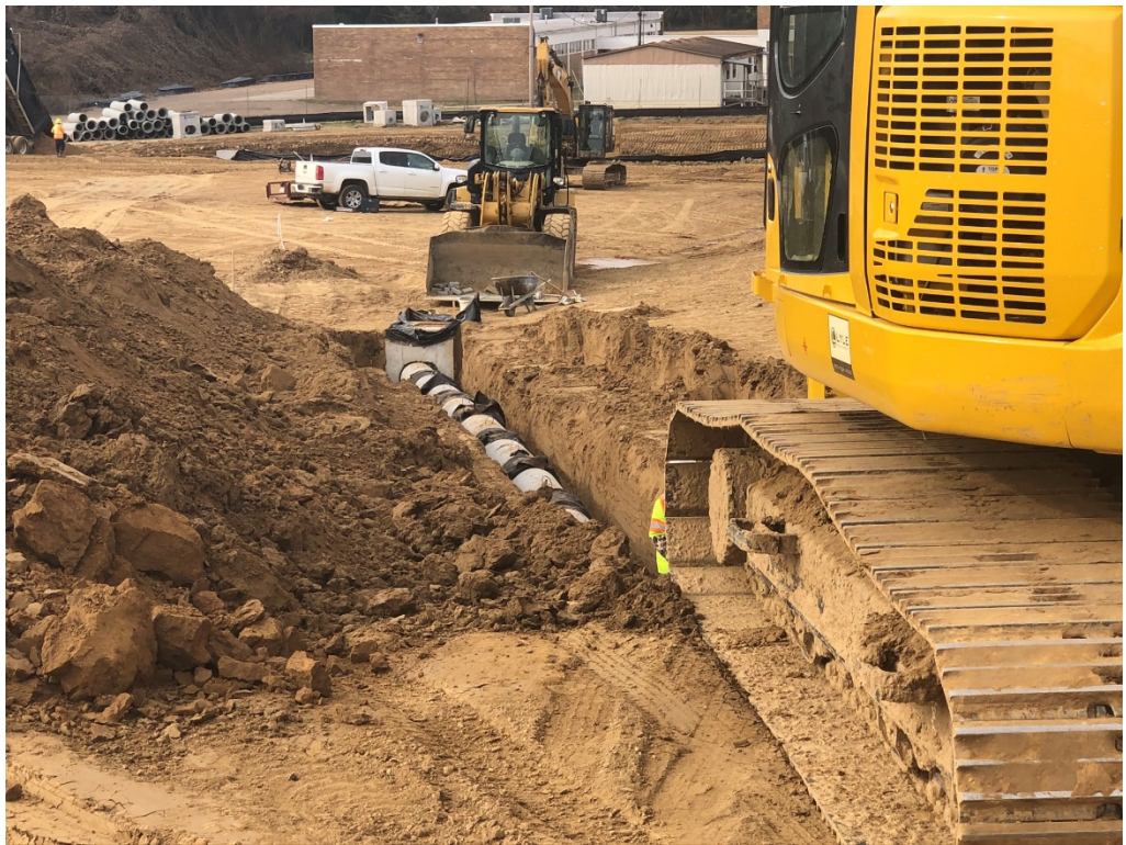
Figure 10 – Storm Sewer Work
