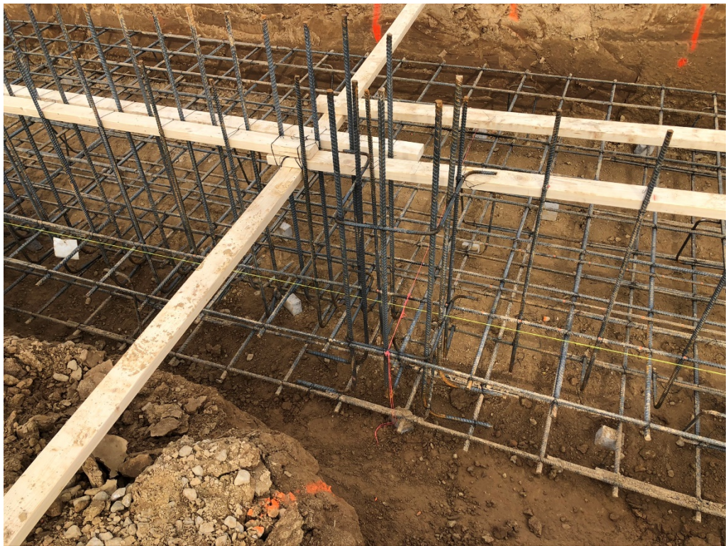
Figure 12 – Tie in Rebar at Pilaster
