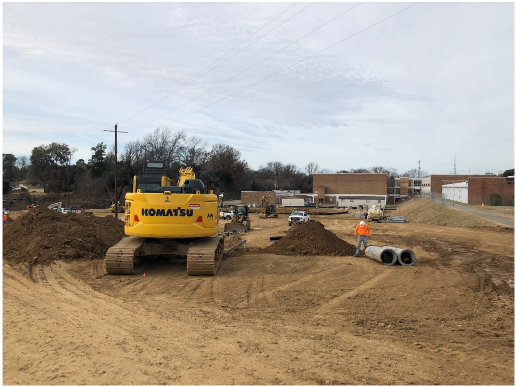
Figure 7 – North Entry Looking WSW
