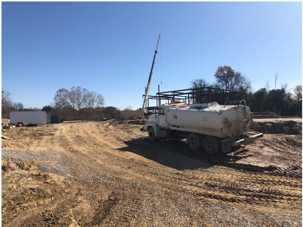
Figure 6 – North Entry Looking ESE
