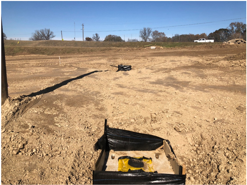
Figure 7 – Storm Sewer Connected (Inlet #8 Looking North)
