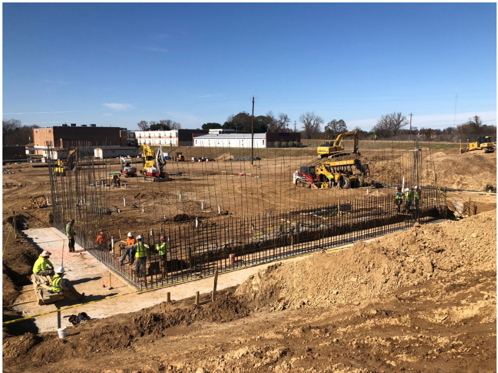
Figure 10 – Foundation Footing at Lower Level
