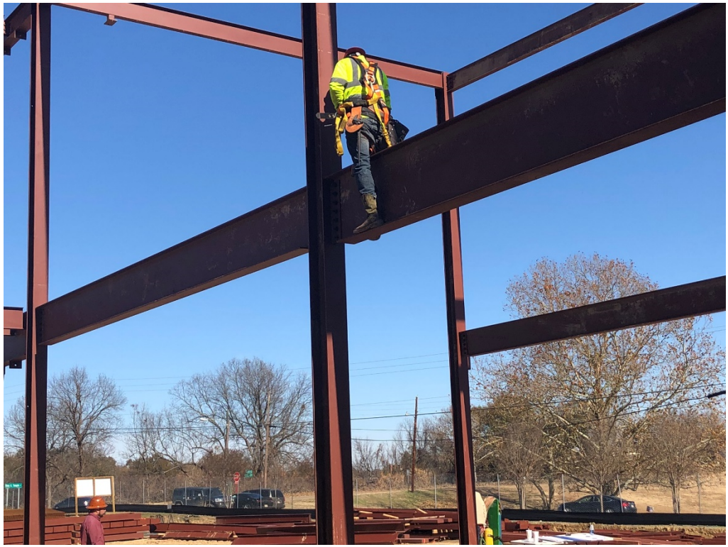
Figure 11 – Steel Erector Bolting Iron Together (Security Device Not in Use)
