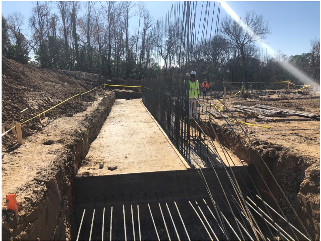
Figure 9 – Foundation Footing at Lower Level
