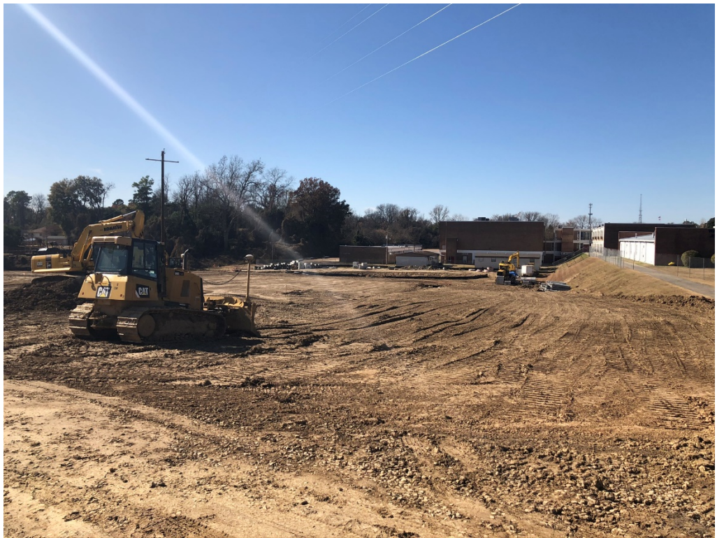
Figure 4 – North Entry Looking WSW
