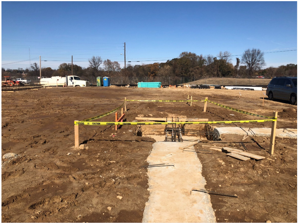
Figure 3 – Warning Tape at Excavation (Typical)
