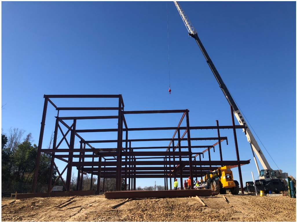
Figure 1 – Red Steel Erected
