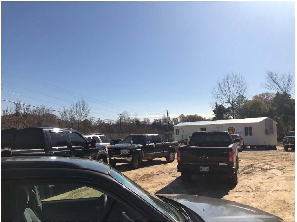
Figure 2 – Parking at Job Site Trailer
