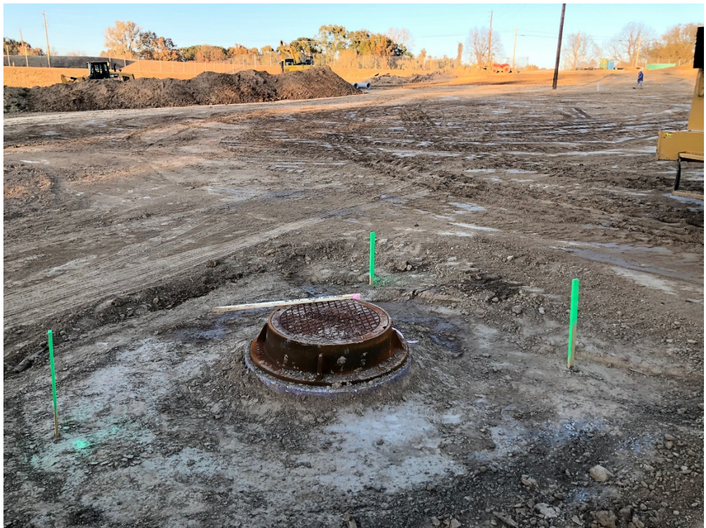
Figure 10 – Storm Sewer Installed in Parking Area
