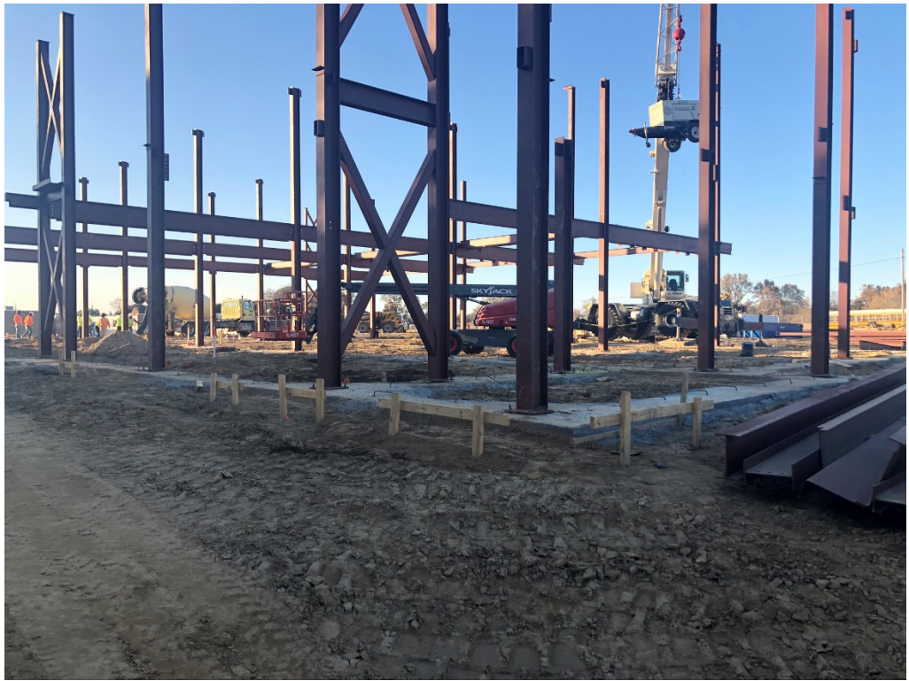
Figure 1 – Red Steel Erected
