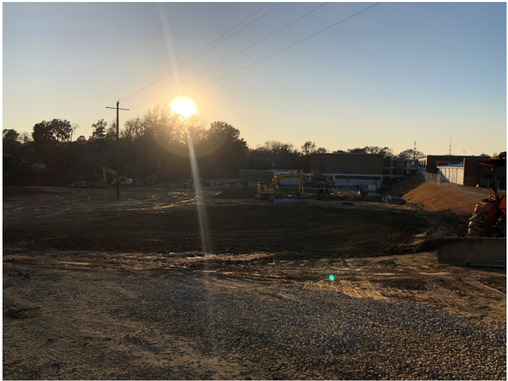
Figure 7 – North Entry Looking WSW
