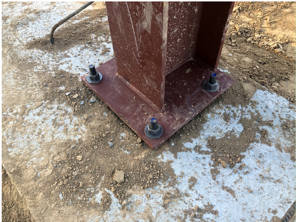
Figure 2 – Typical Connection to Footing
