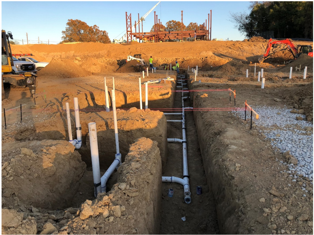
Figure 9 – Rough Plumbing at Lower Slab
