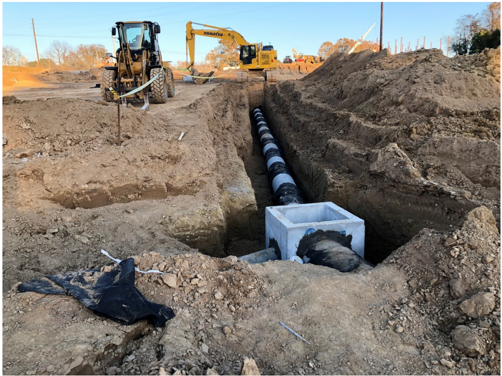
Figure 11 – Storm Sewer Work @ North Side of Parking
