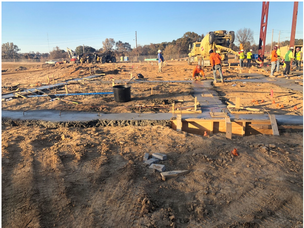
Figure 4 – Foundation Work Cont. at Upper Slab
