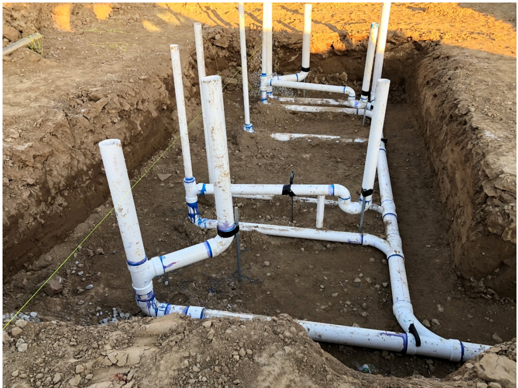
Figure 8 – Rough Plumbing at Lower Slab
