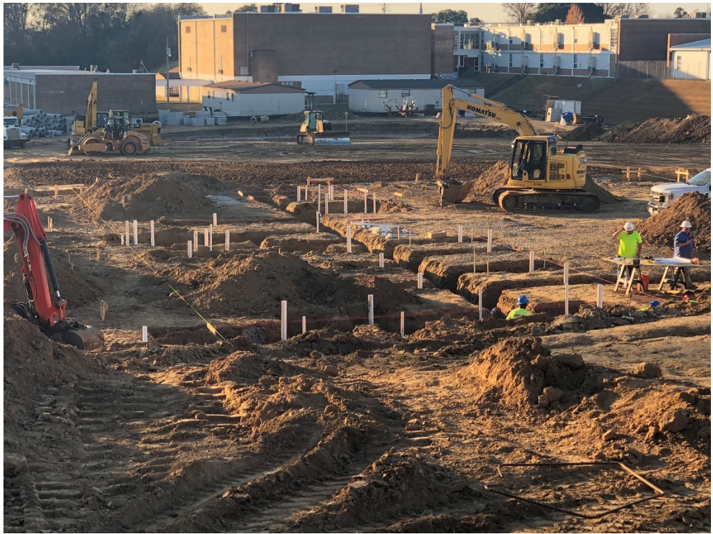
Figure 3 – Plumbing Rough-In at Lower Slab
