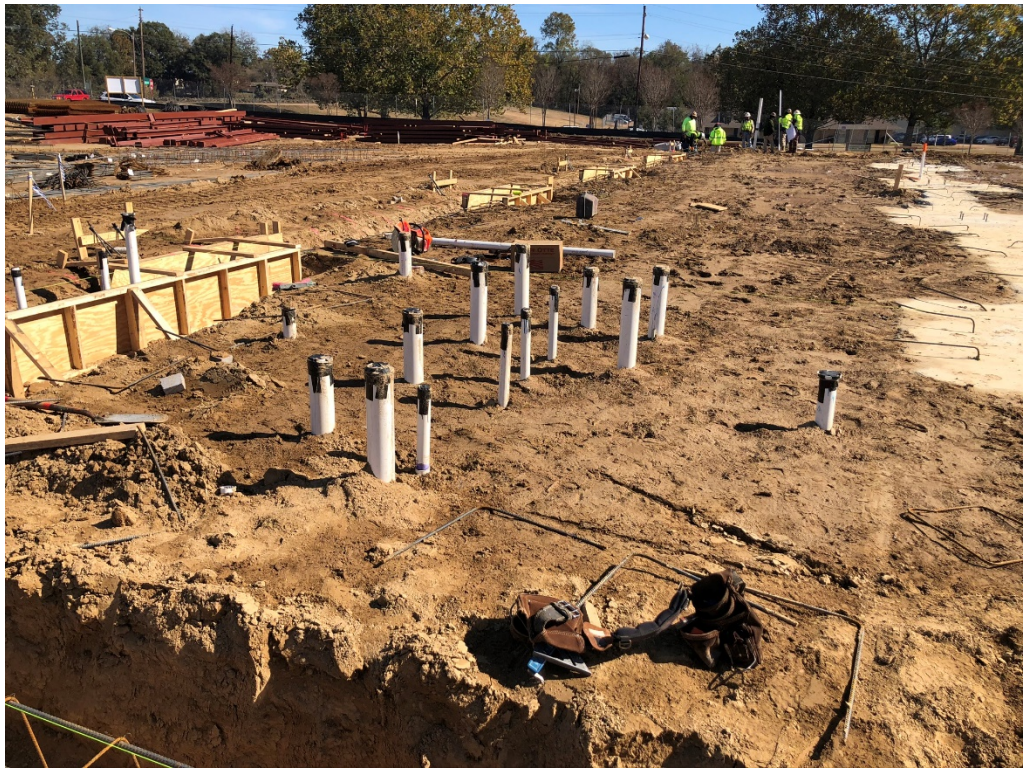
Figure 11 – Plumbing Stubbed Up
