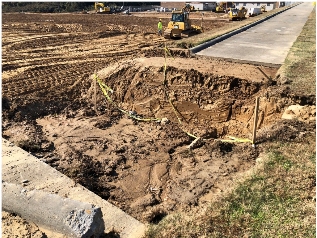
Figure 22 – Drive Removed for work on Storm Sewer Connection
