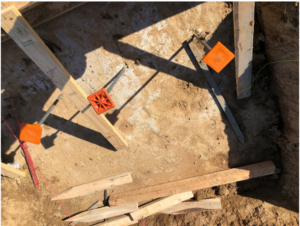
Figure 10 – Safety Caps in use @ Vertical Rebar
