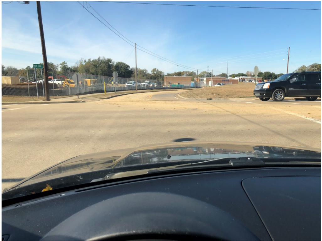
Figure 1 – Dirt Tracked out to Intersection from Work
