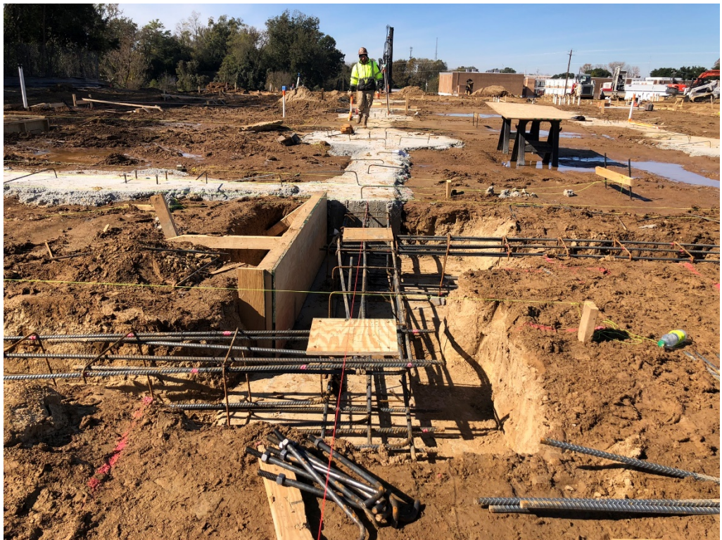
Figure 4 – Reinforcement @ Beams
