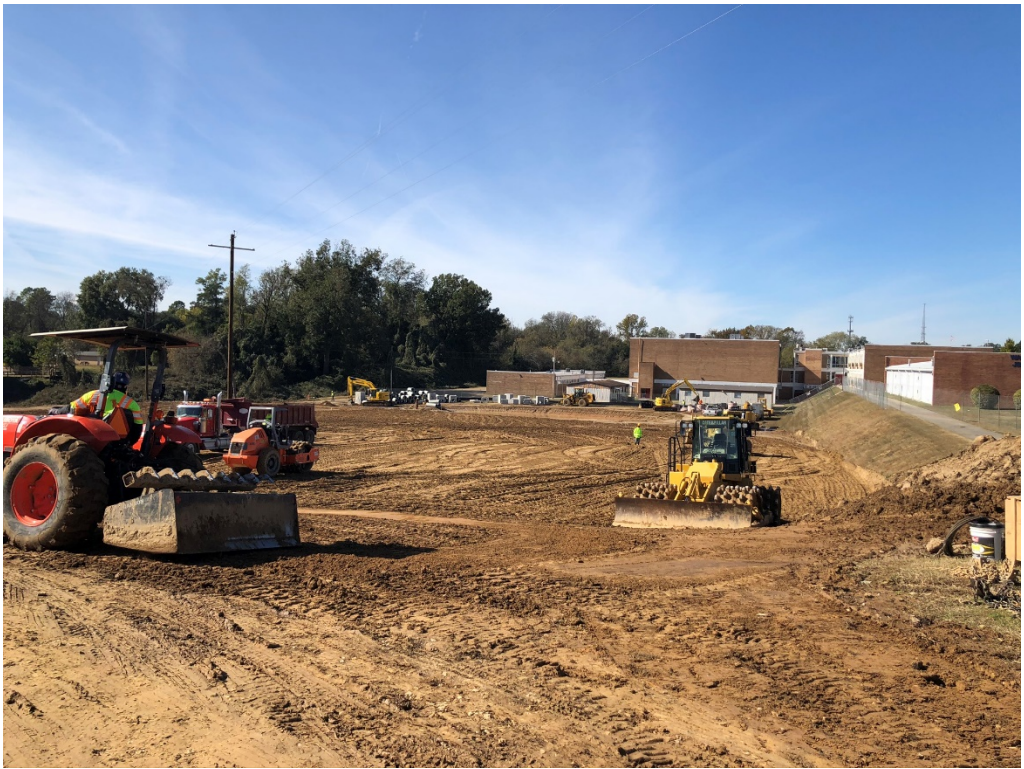
Figure 13 – North Entry Looking WSW
