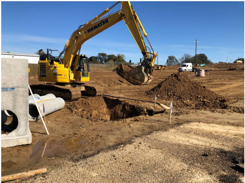
Figure 18 – Storm Sewer Excavation
