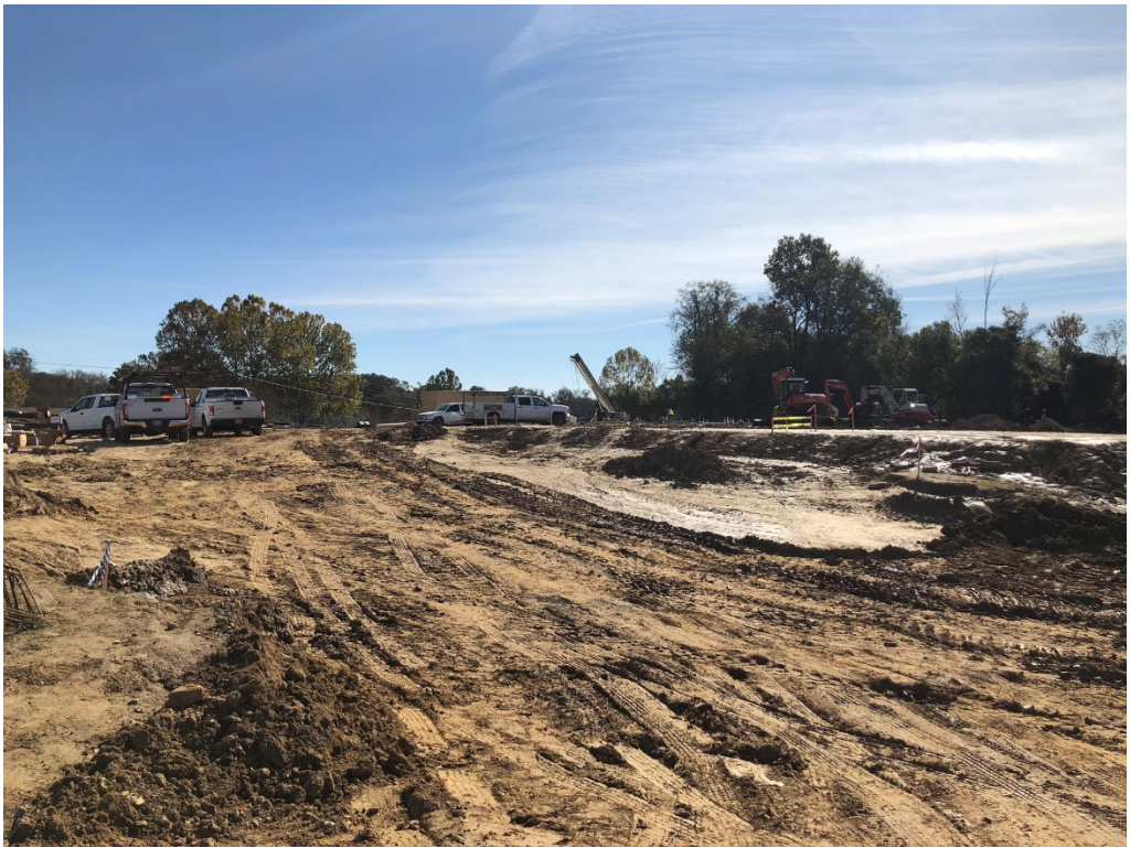
Figure 15 – North Entry Looking ESE
