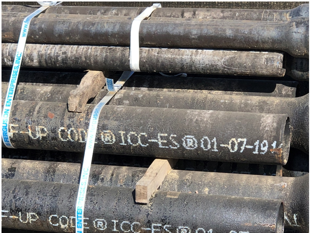
Figure 20 – Pipe Stored on Site
