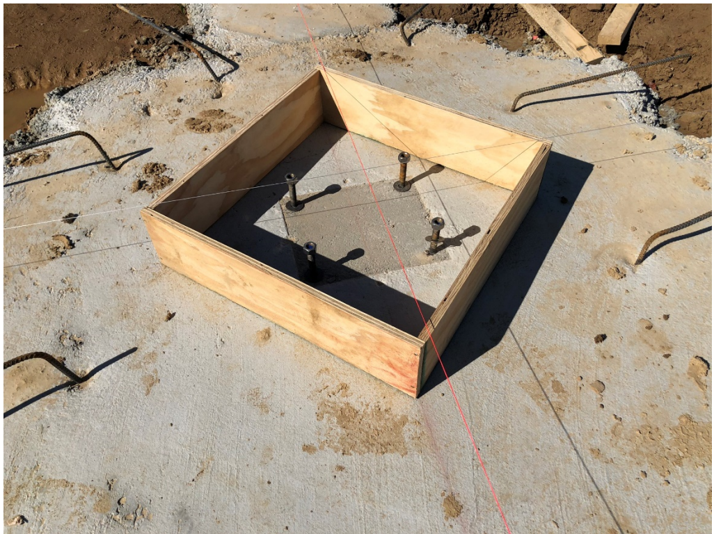
Figure 6 – Lines Laying out Beams
