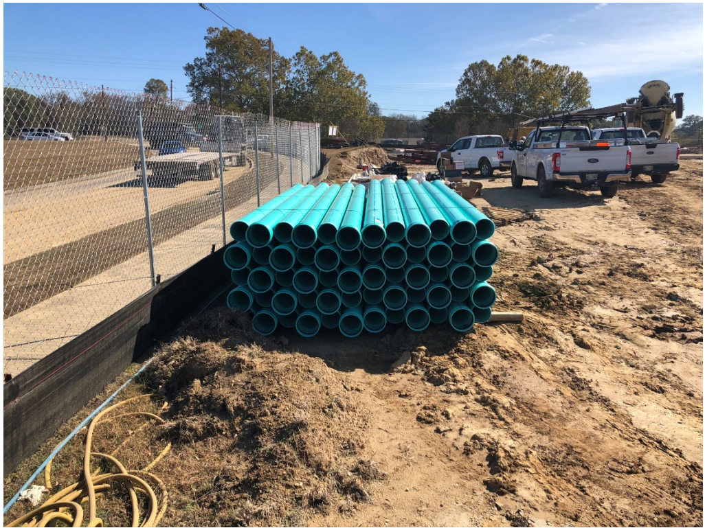
Figure 19 – Pipe Stored on Site
