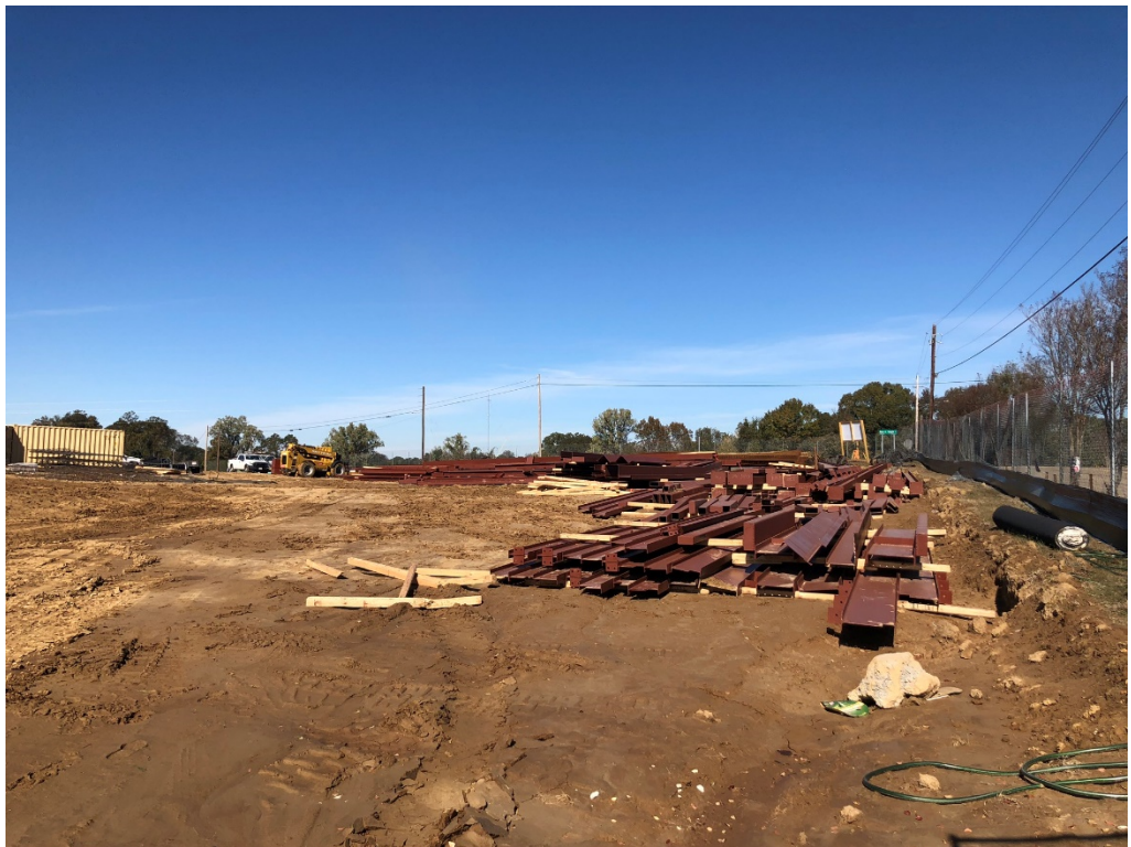
Figure 2 – Red Steel Stored on Site
