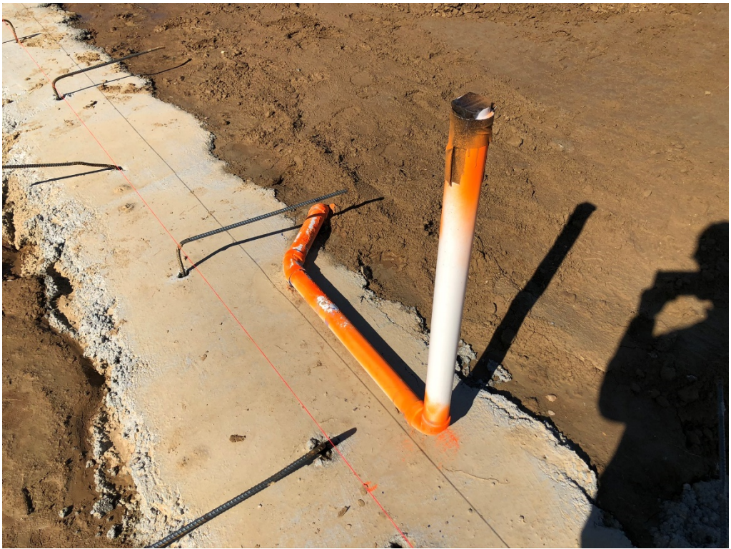
Figure 7 – Stubbed up Plumbing (Confirm to be Encased in Slab Horizontally?)
