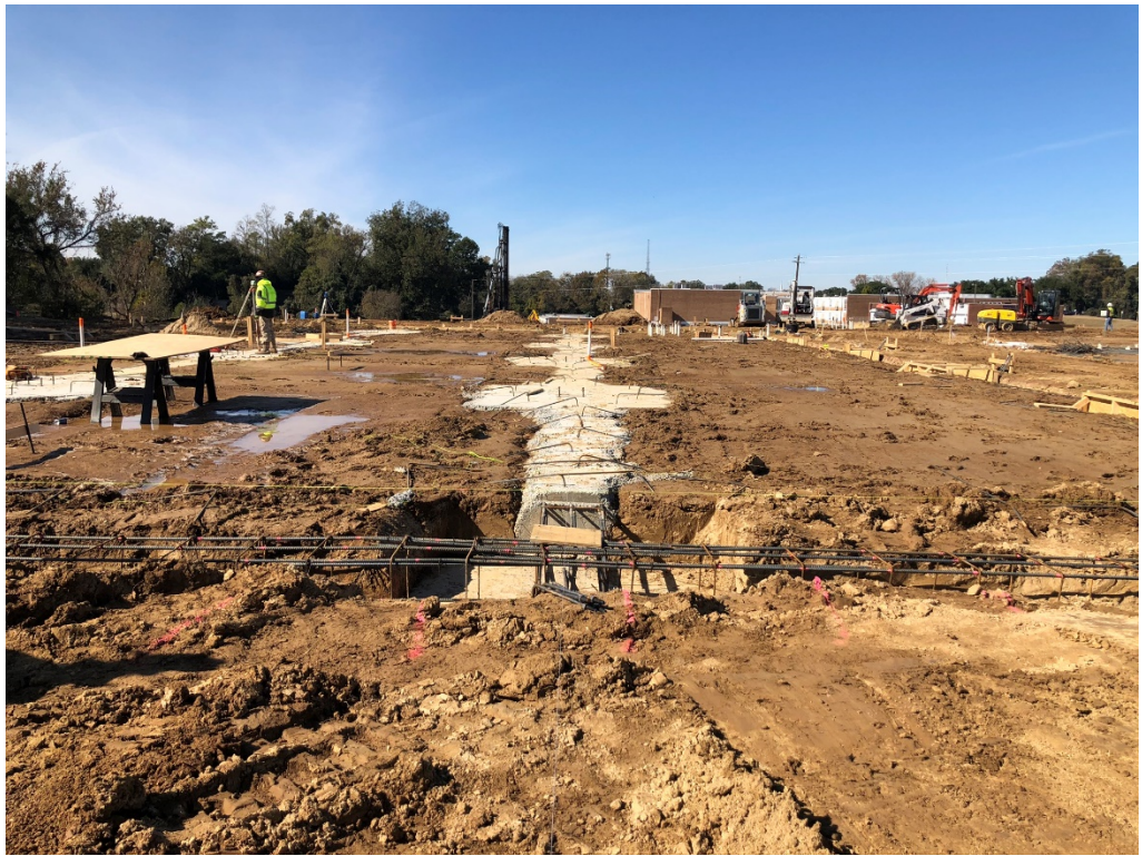
Figure 3 – Foundation Beam
