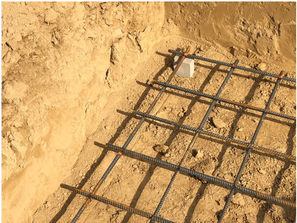
Figure 4 – Confirm Concrete Coverage between rebar and Earth
