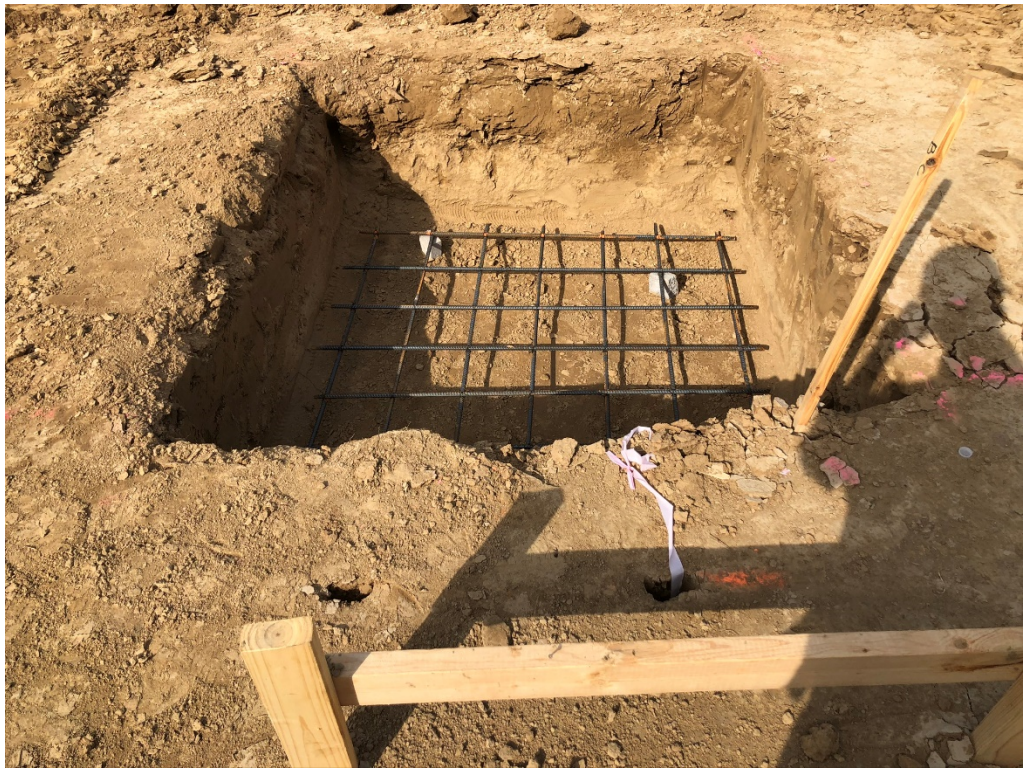
Figure 1 – Isolation Footing (typical)
