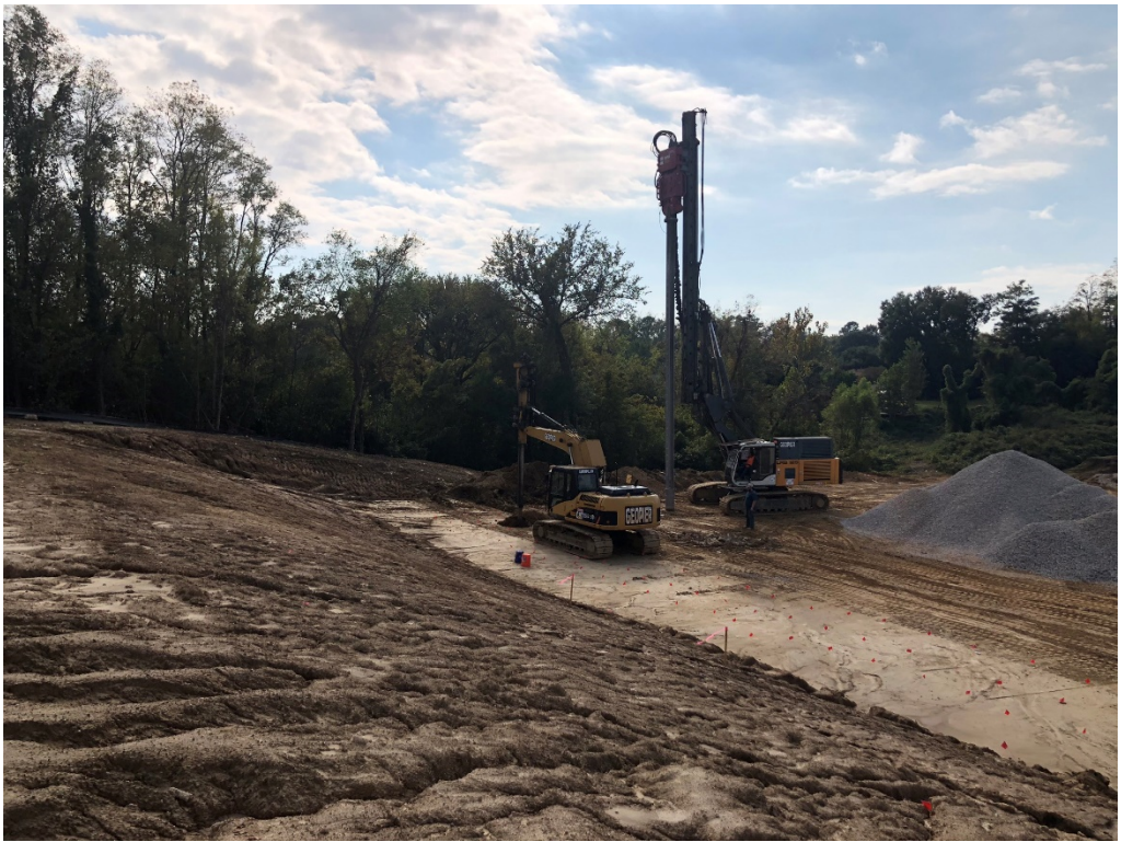
Figure 5 – Geo Pier Drill out and Install
