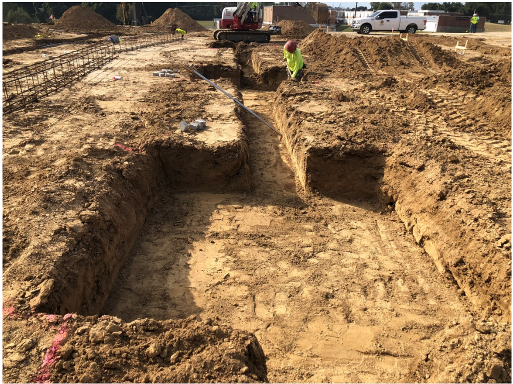
Figure 3 – Excavated Footing
