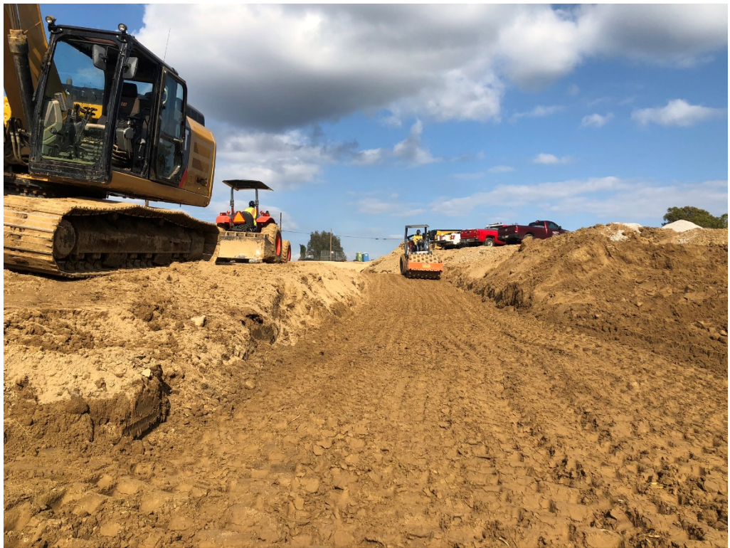
Figure 10 – Dirt Compaction on South Parking Area
