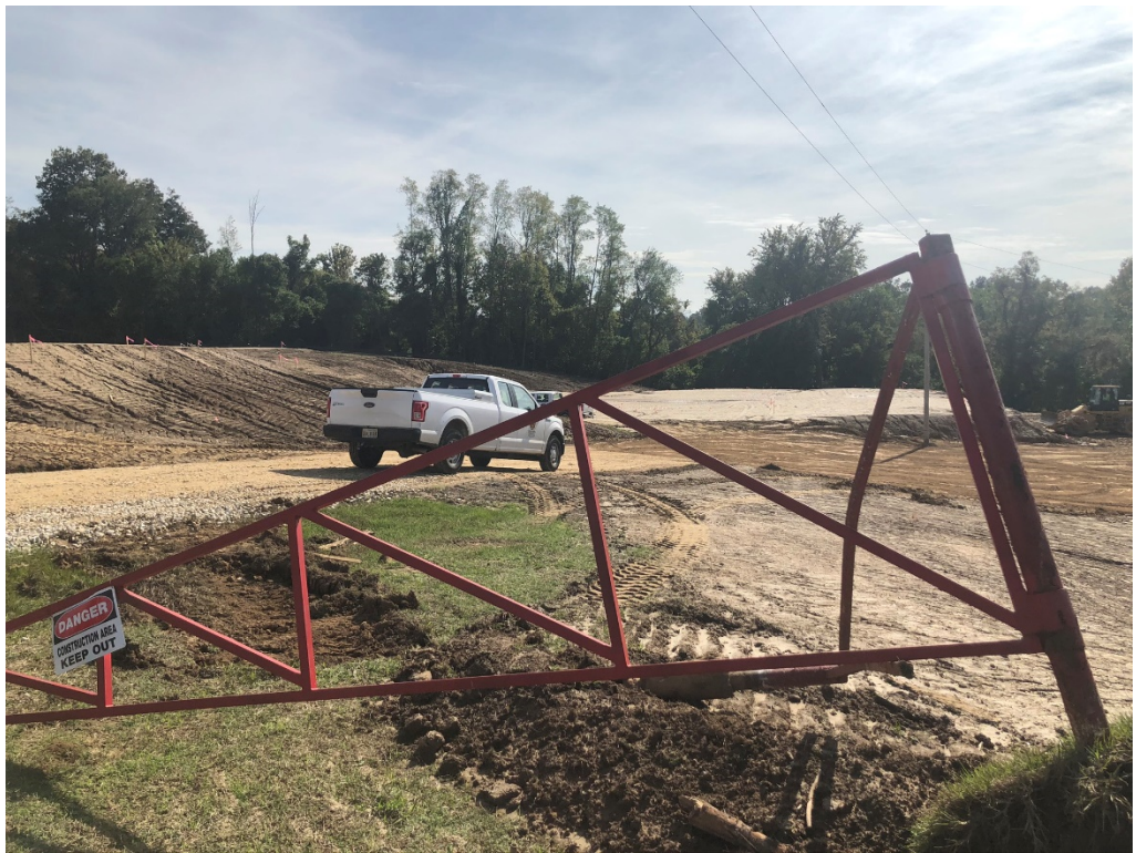
Figure 4 – Construction Barrier Removed
