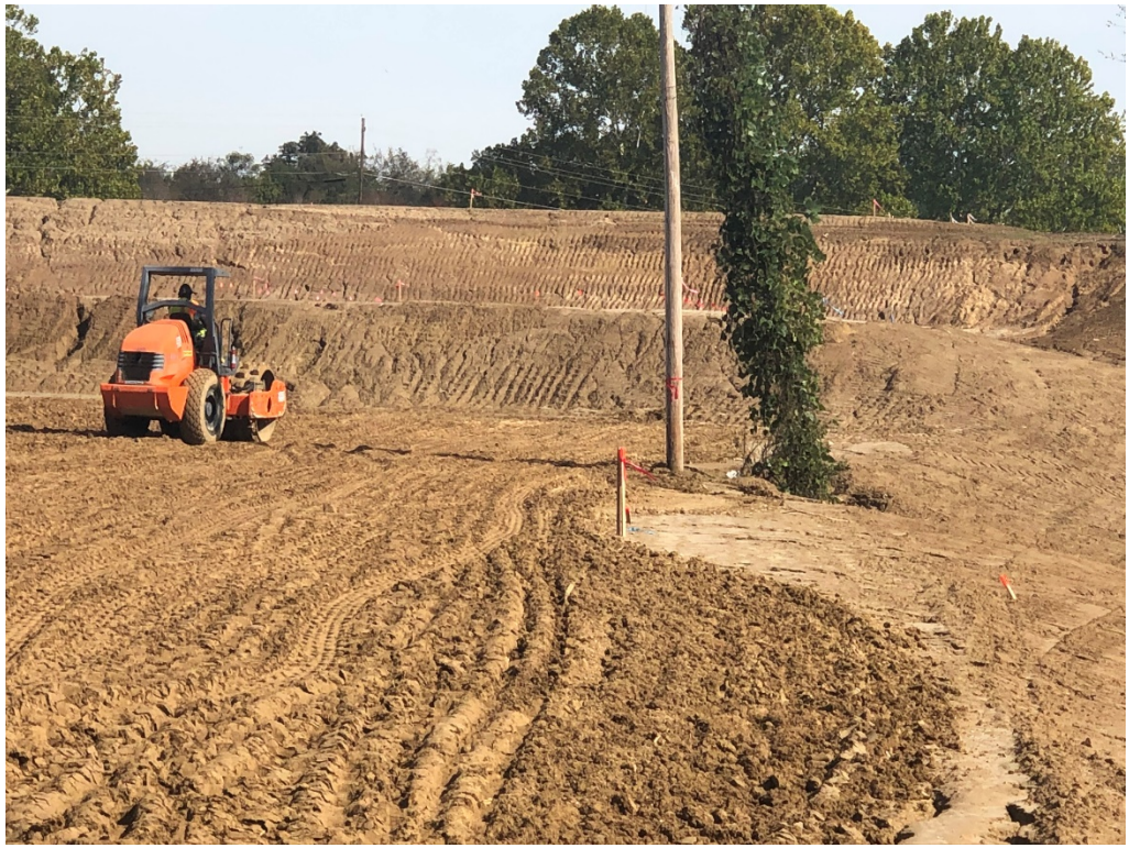
Figure 7 – Southmost Power Pole New Location
