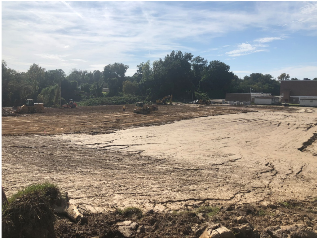
Figure 3 – Pad Work at Parking Area
