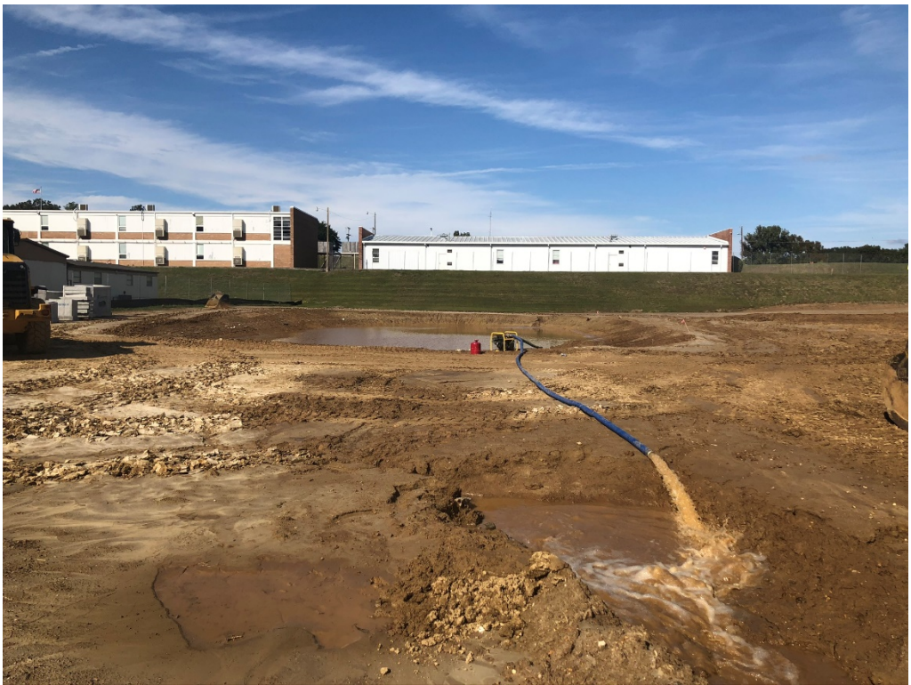
Figure 6 – Detention Pond Draining
