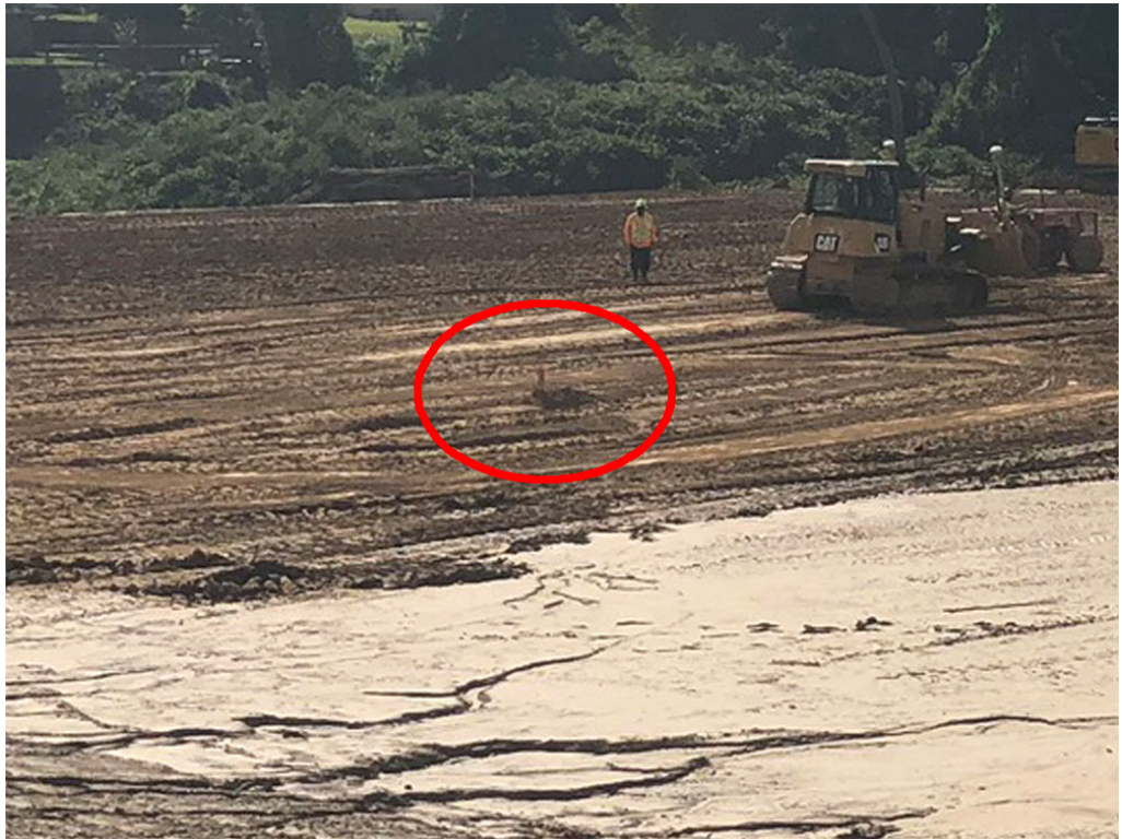
Figure 8 – Northmost Power Pole New Location
