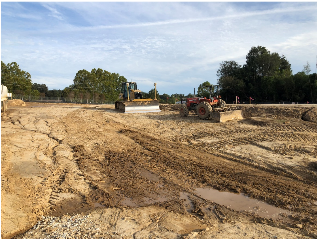
Figure 12 – North Entry Looking SE
