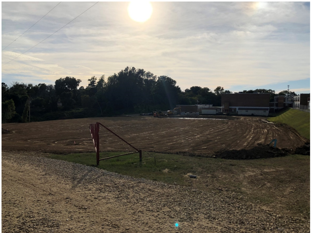
Figure 14 – North Entry Looking SW
