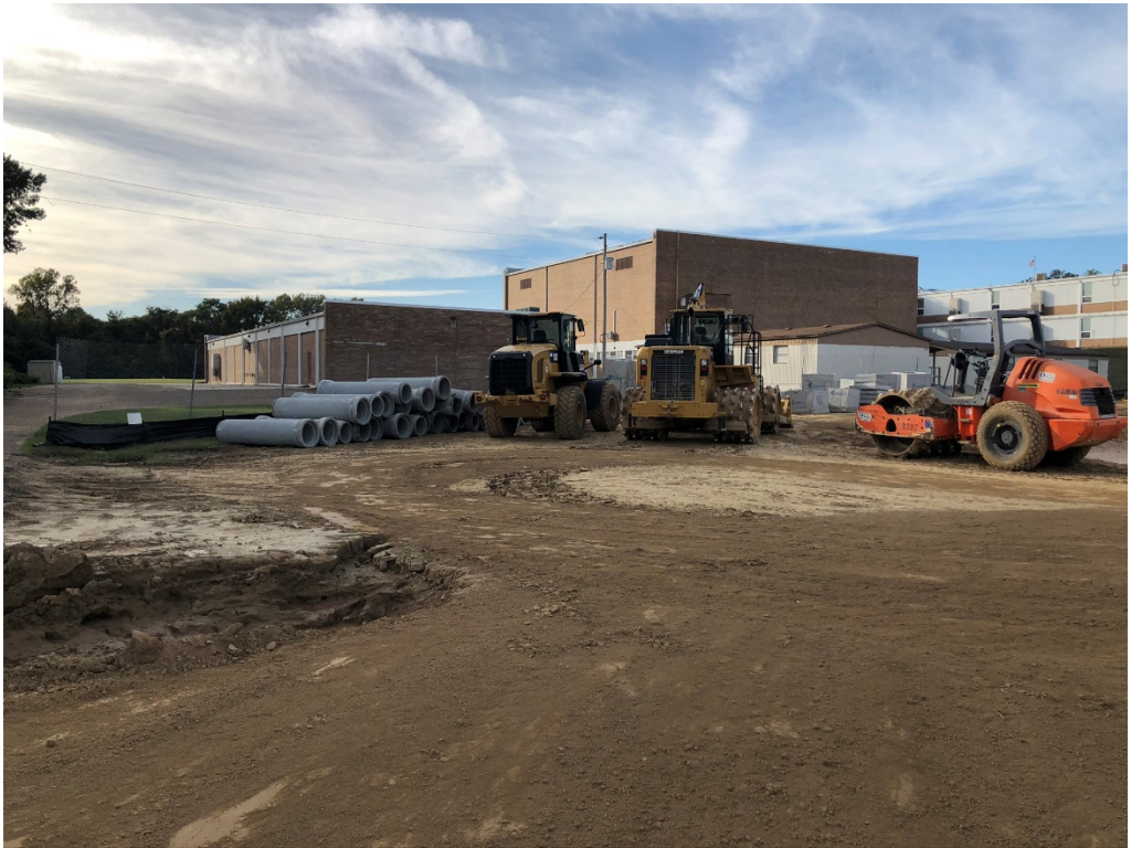
Figure 6 – Equipment and Culverts
