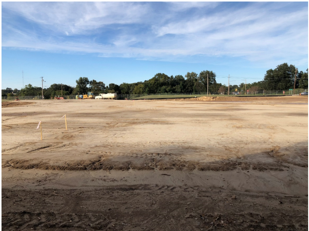
Figure 2 – South Upper Slab Looking North
