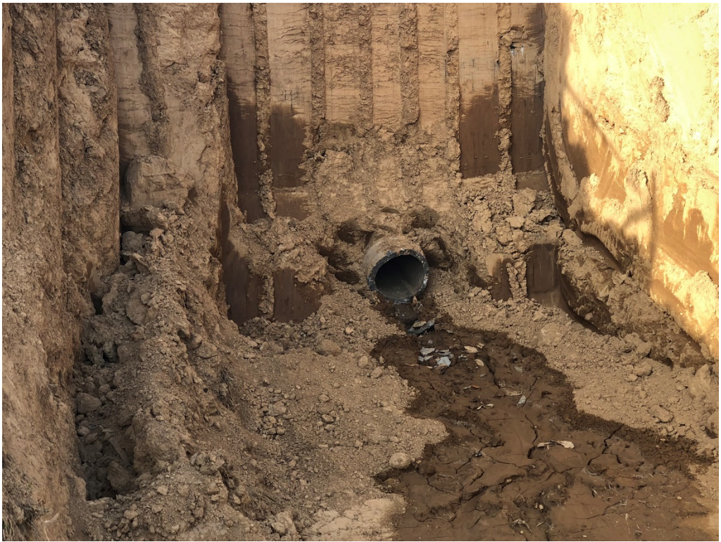
Figure 11 – Excavated Drain
