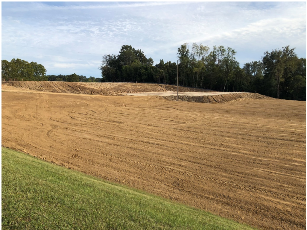
Figure 10 – Northwest Corner Looking SE
