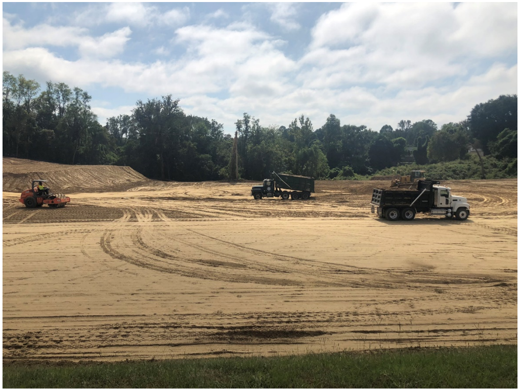
Figure 7 – North West of Center Looking South at Lower Slab/Parking
