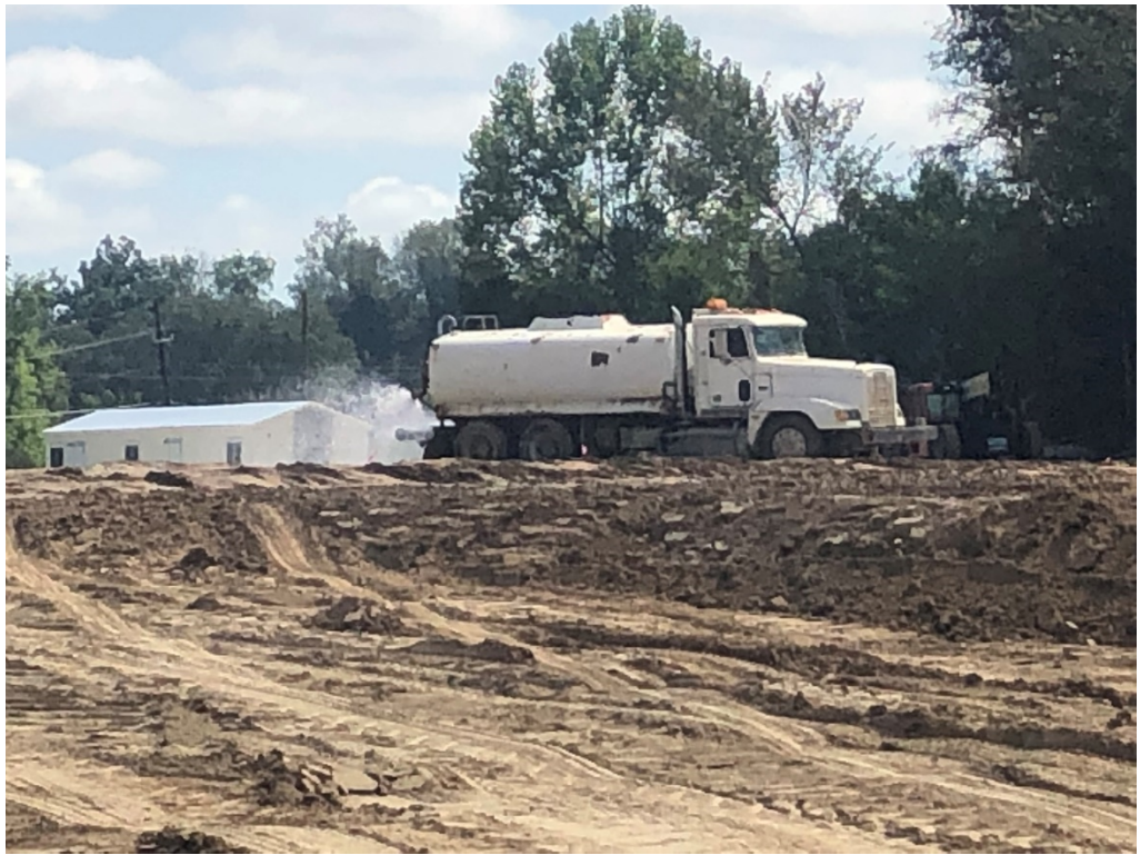
Figure 11 – Watering Truck In Use for Dirt Work
