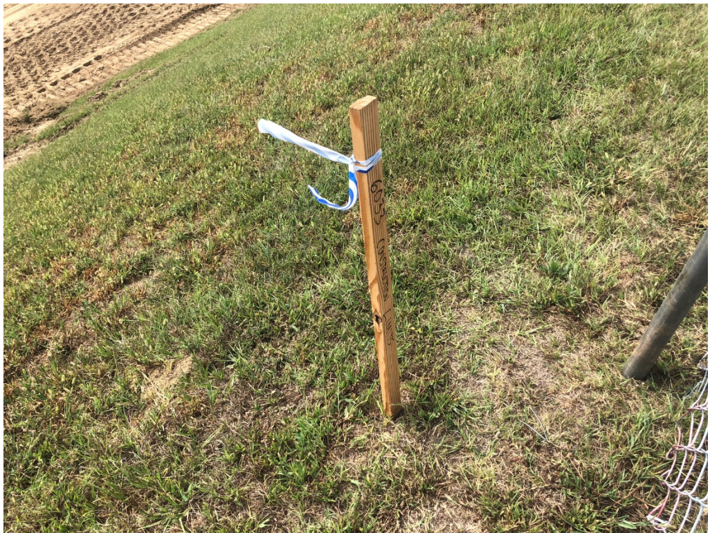
Figure 8 – Example of Site Marking Stake
