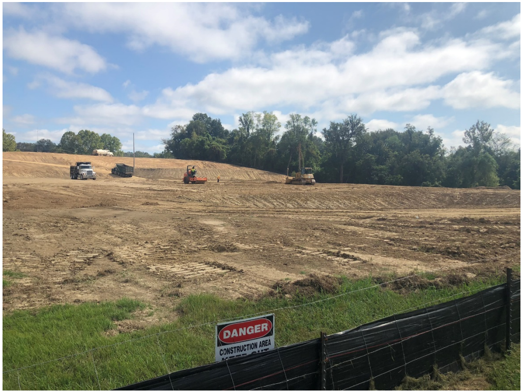
Figure 9 – North West Corner Looking SE (Parking Area)
