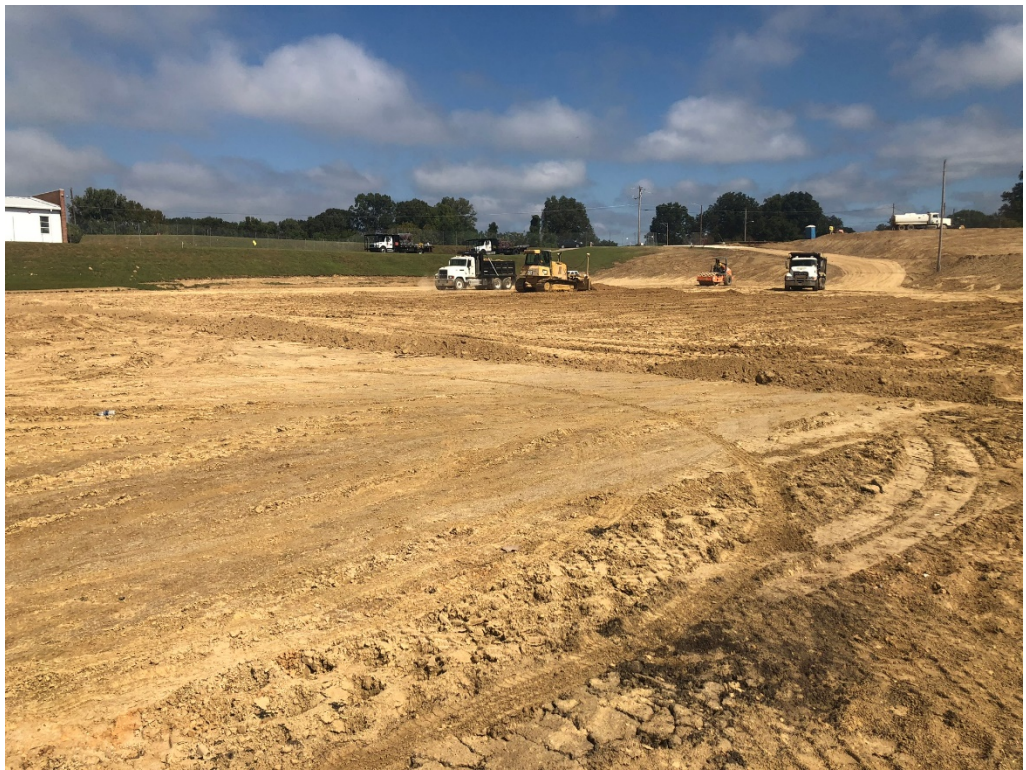
Figure 10 – South West Corner Looking NE
