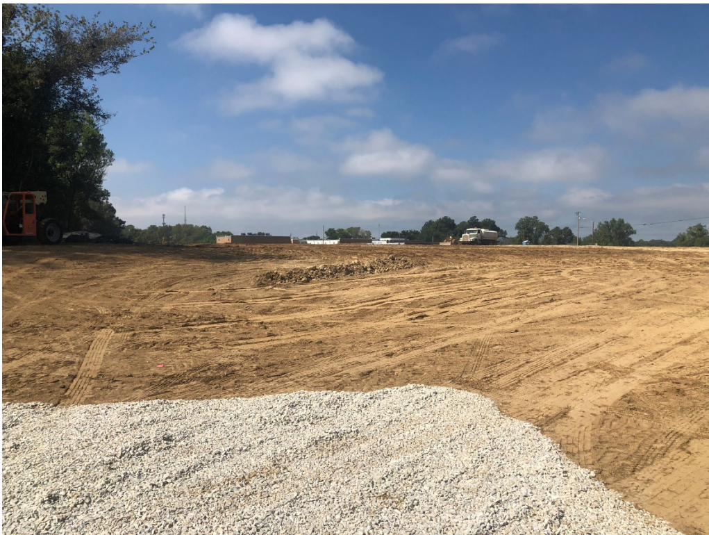
Figure 16 – South East Corner Looking WNW (Upper Slab)
