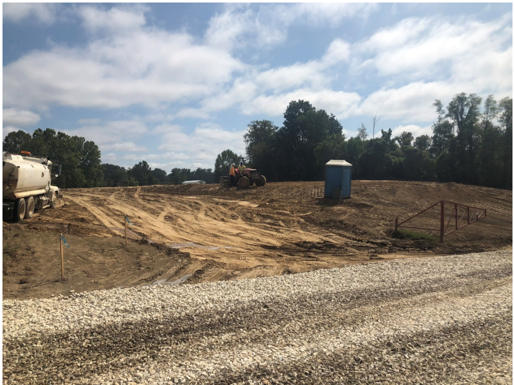
Figure 4 – Upper Pad Work (N Entrance Looking SE)
