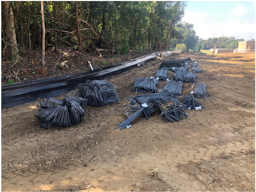
Figure 17 – Some Rebar Bends On Site Stored at South Upper Pad
