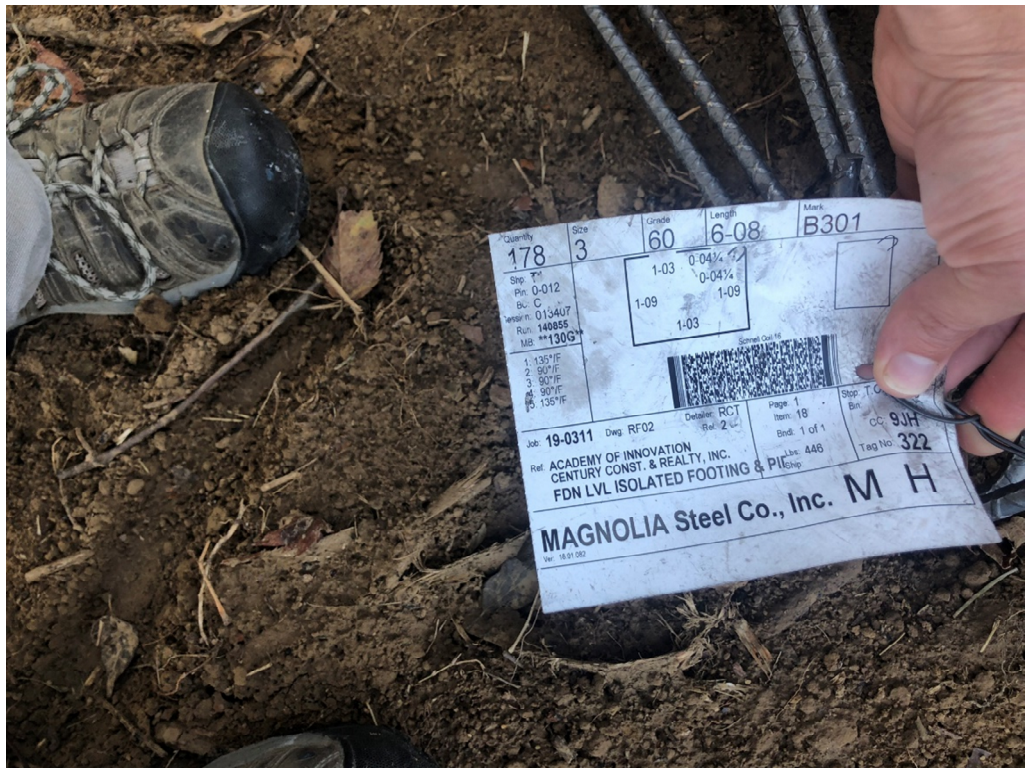
Figure 18 – Manufacturer's Tag on Rebar Bundle
