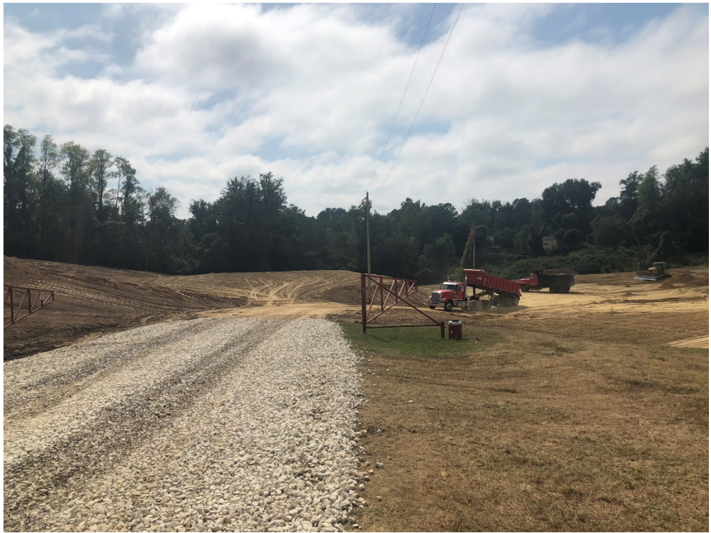
Figure 3 - Lockable Gate Entrance (N Entrance Looking S)
