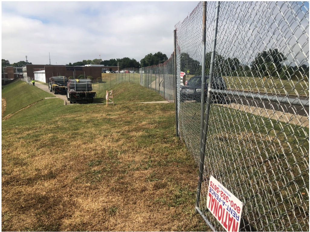
Figure 5 – Temporary Fence Being Installed
