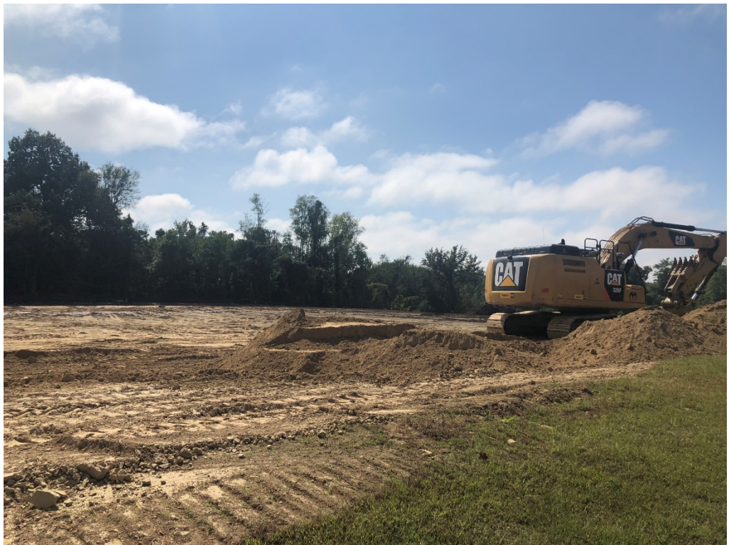
Figure 12 – North East Corner of Site Looking SW (Upper Pad)
