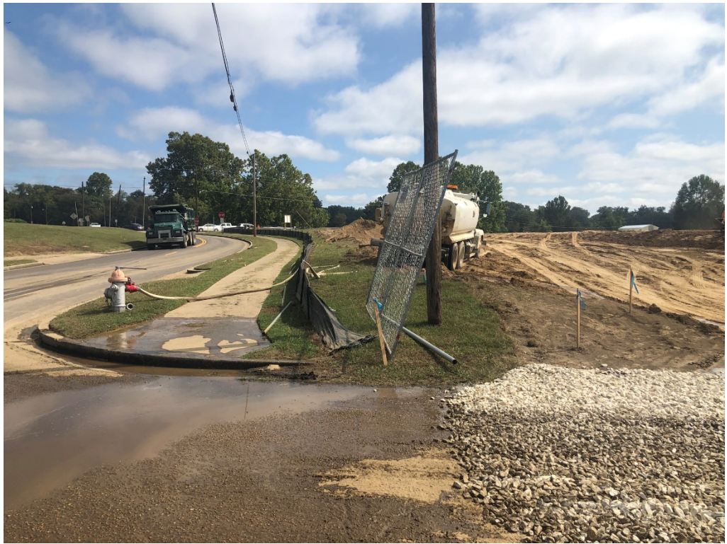
Figure 1 – Potable Water In Use for Watering Slab
