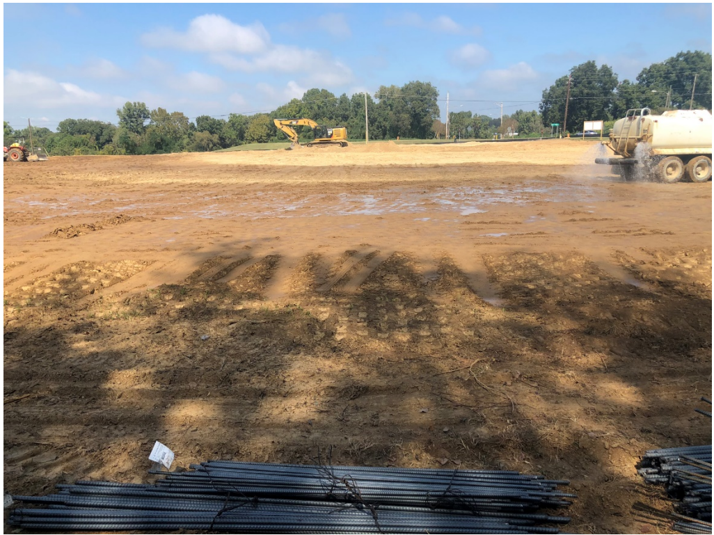
Figure 19 – South East of Center Looking North (Upper Pad)
