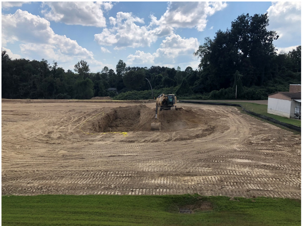
Figure 20 – Fill Dirt Excavated for Middle Slab Pad
