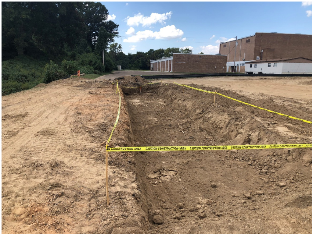
Figure 14 – Trench Dug in Parking Area
