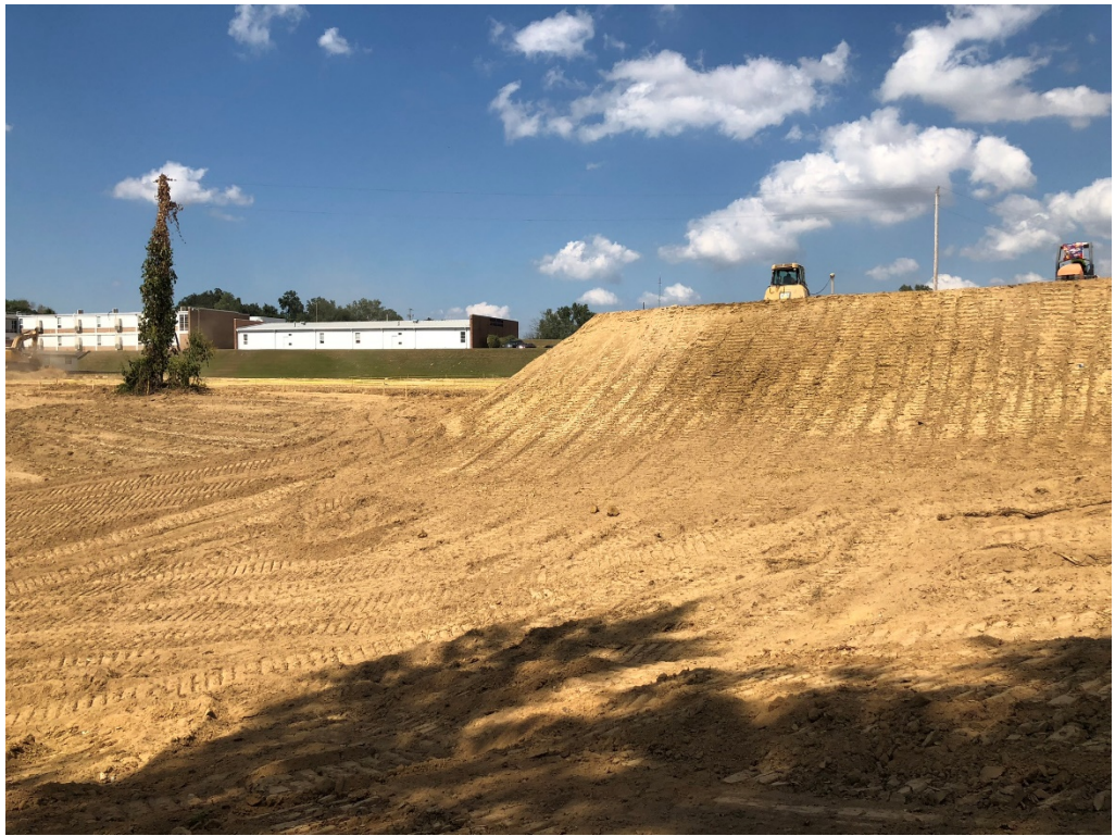
Figure 11 – South Side Center Looking NNW (Steep Grade @ Middle Pad)
