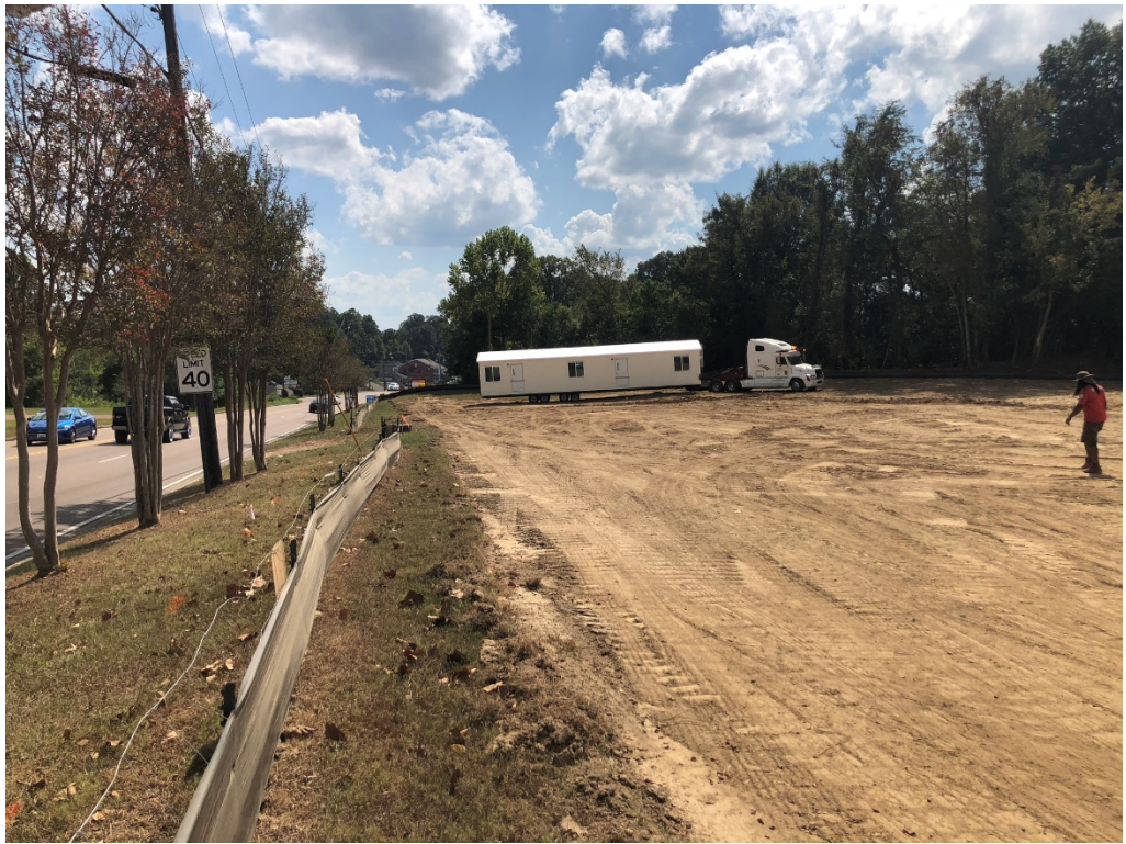
Figure 7 – Job Site Trailer Set on SE Corner of Project Site
