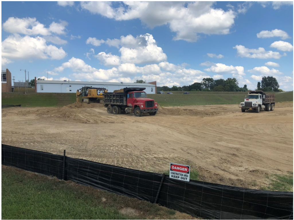
Figure 17 – Fill Dirt Transported to Middle Slab Pad
