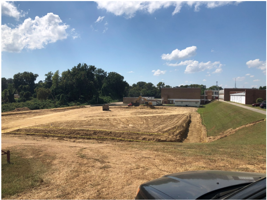
Figure 1 – Lower Pad Developing (N Entrance Looking SW)
