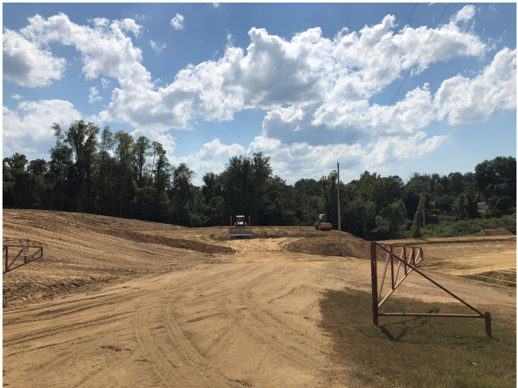
Figure 2 – Lockable Gate Entrance (N Entrance Looking S)
