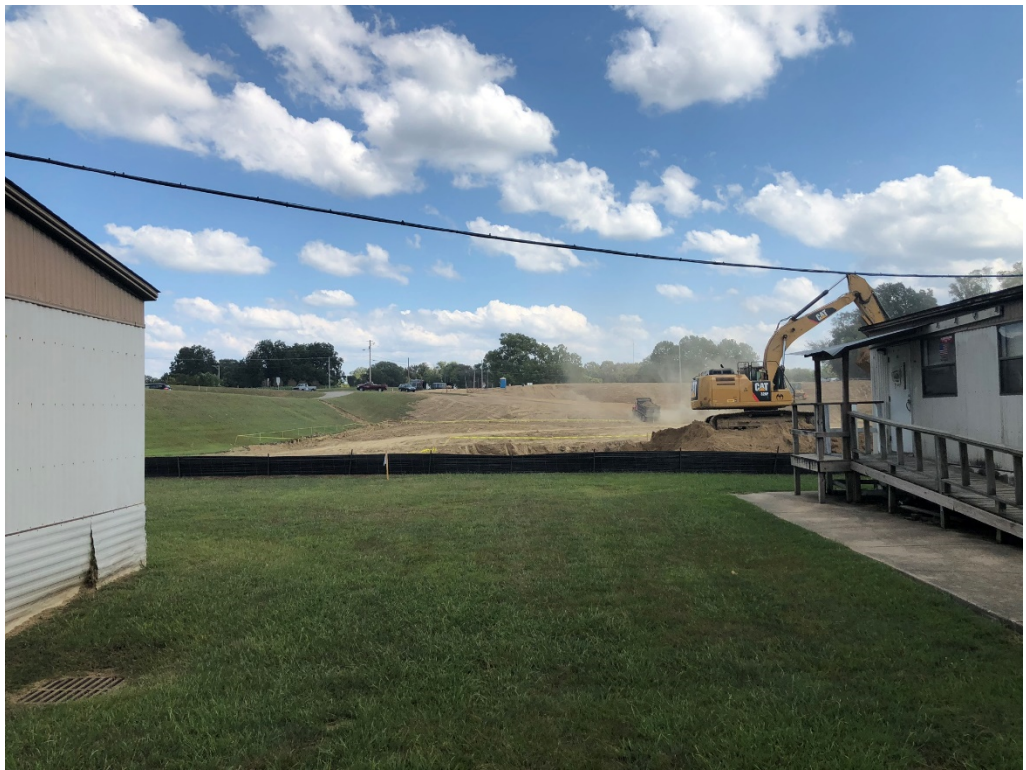
Figure 18 – West Side of Project Looking E
