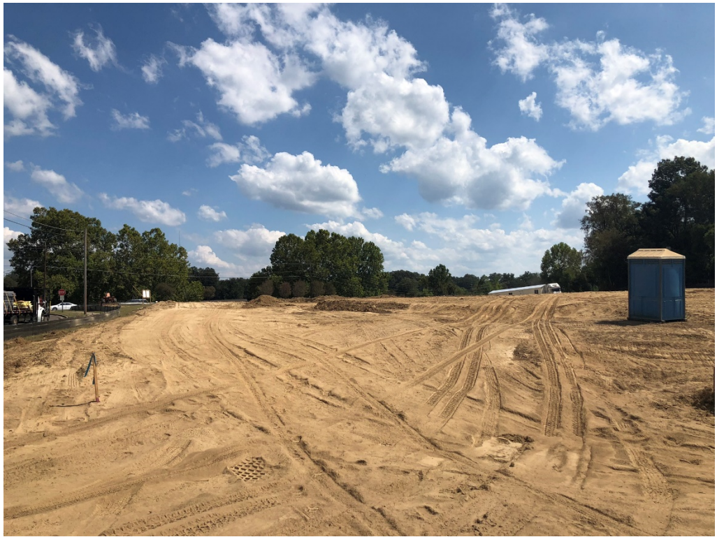
Figure 3 - Upper Pad Work (N Entrance Looking SE)
