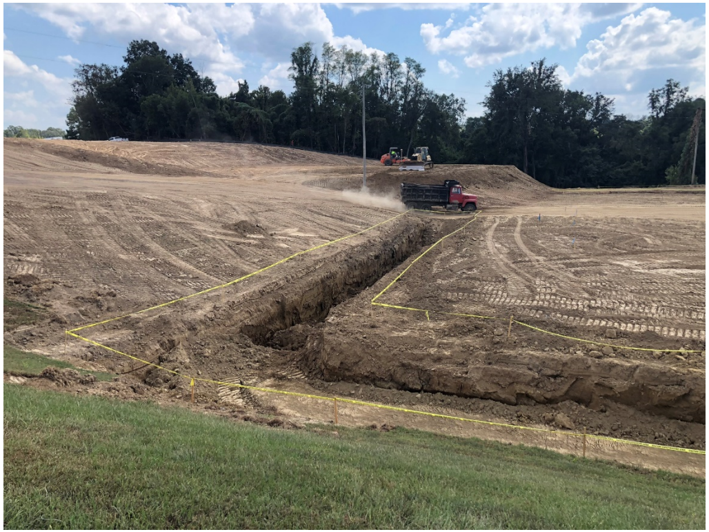
Figure 21 – Trench Dug @ North Side of Property
