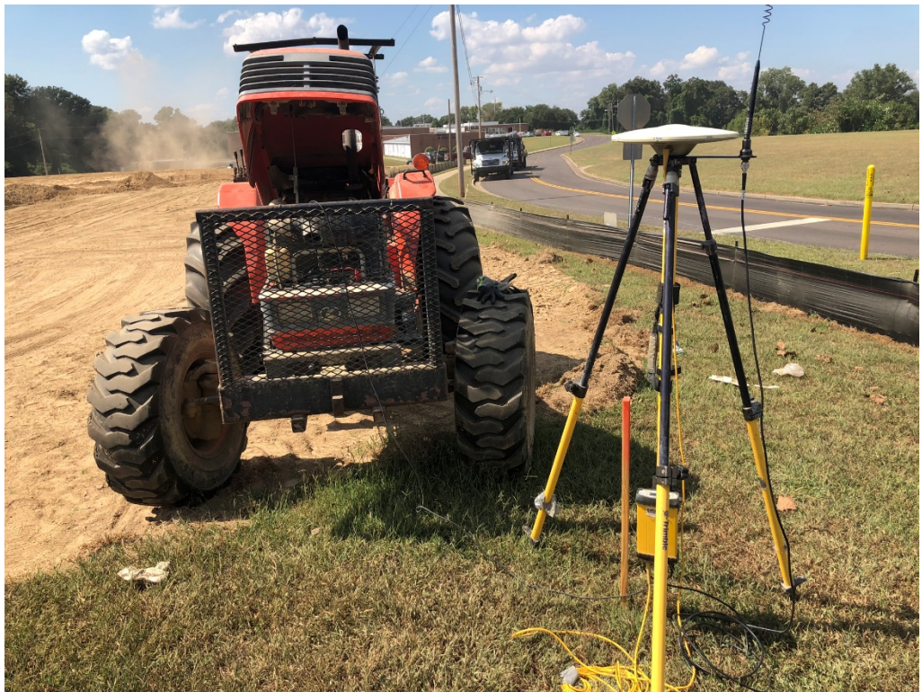
Figure 6 – GPS Locating Equipment Connected to Tractor Power
