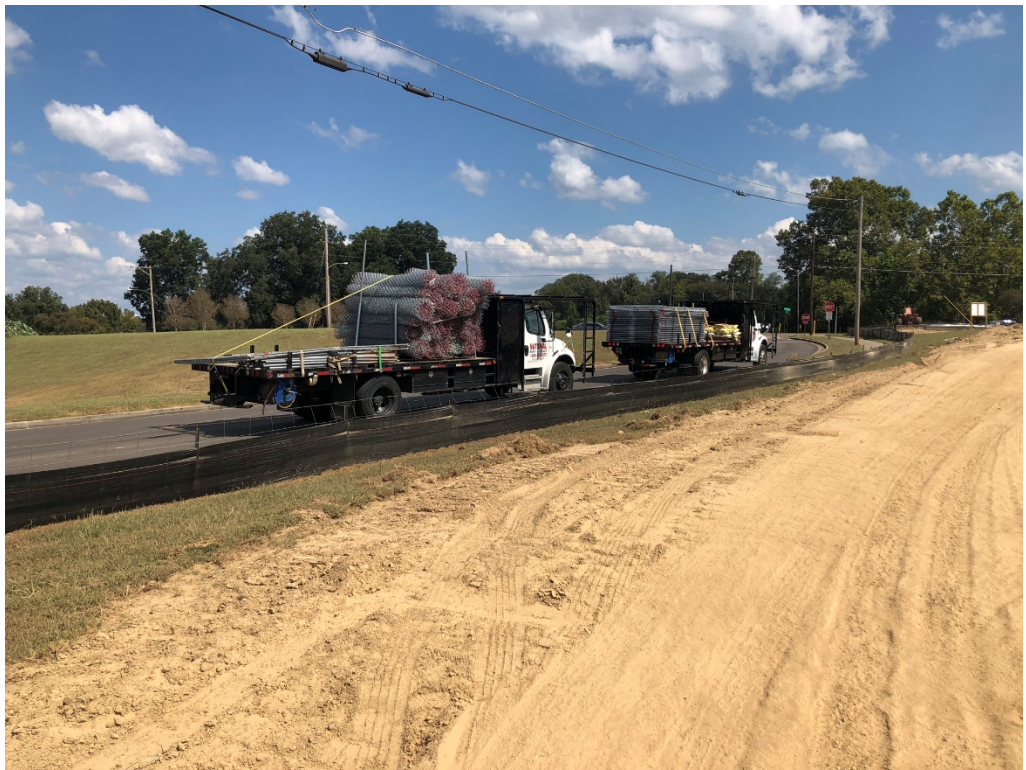
Figure 4 – Temporary Fencing being Delivered
