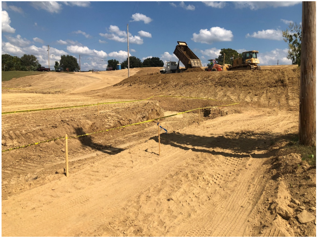
Figure 13 – South Side West of Center Looking NE
