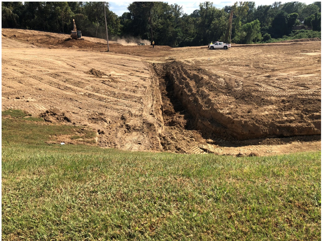
Figure 4 – Lower Slab Excavation Begun
