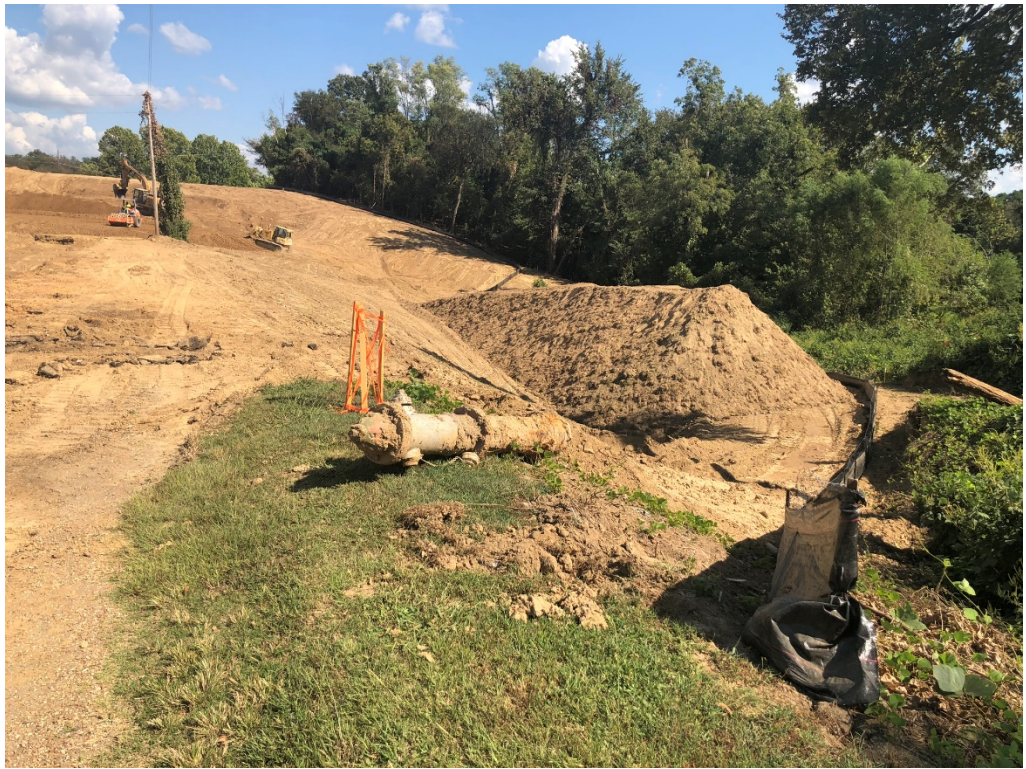
Figure 7 – Silt Fencing In Place
