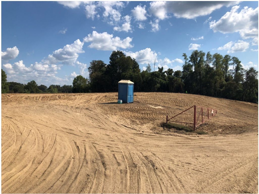
Figure 3 - Upper Pad Work (S Entrance Looking NW)
