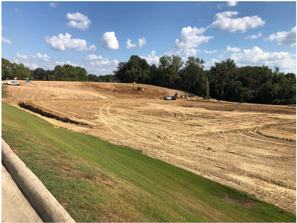
Figure 5 – North West Corner of Project Looking SE
