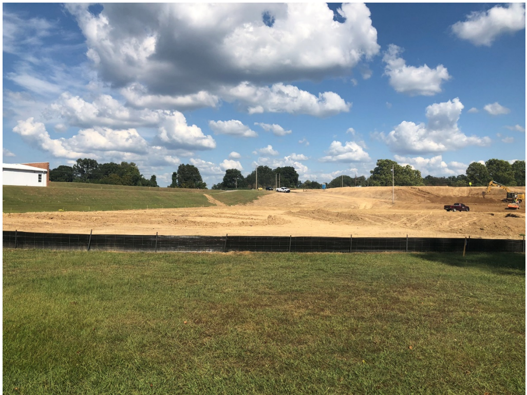
Figure 6 – Silt Fencing In Place (SW Corner of Project Looking ENE)
