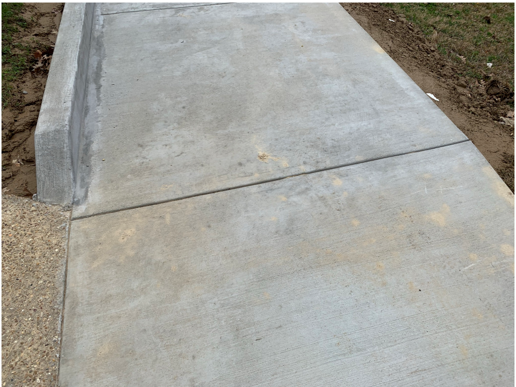
Figure 2 – ADA Ramp Clean Up
