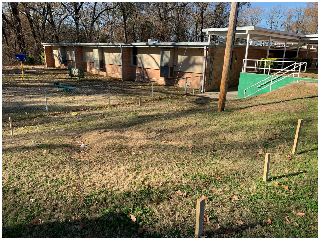
Figure 4 – ADA Ramp Layout Staked Off
