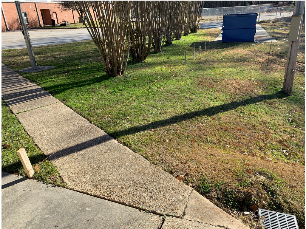
Figure 3 – ADA Ramp Layout Staked Off
