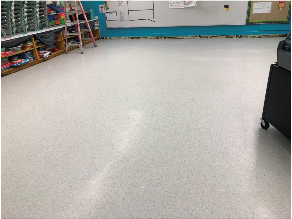
Figure 3 – West Section of Building A New Floor
