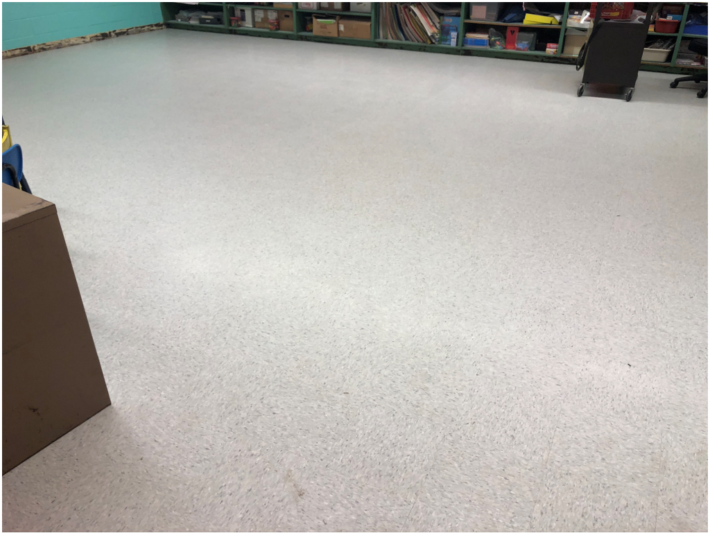
Figure 5 – West Section of Building A New Floor
