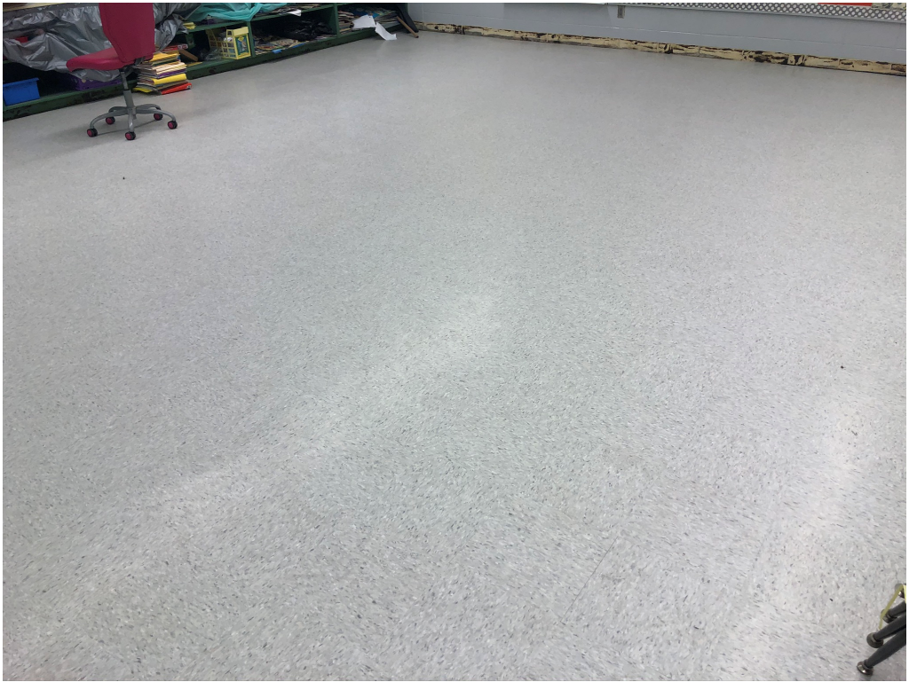
Figure 7 – West Section of Building A New Floor
