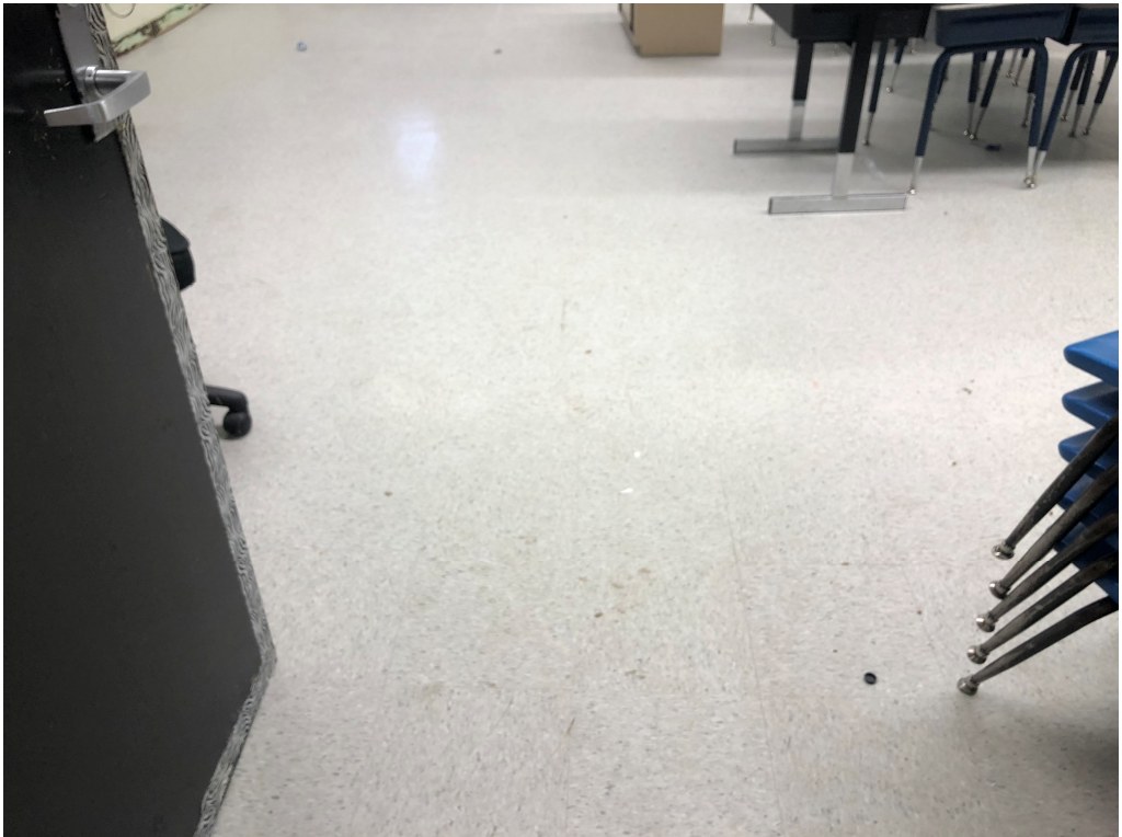
Figure 4 – West Section of Building A New Floor
