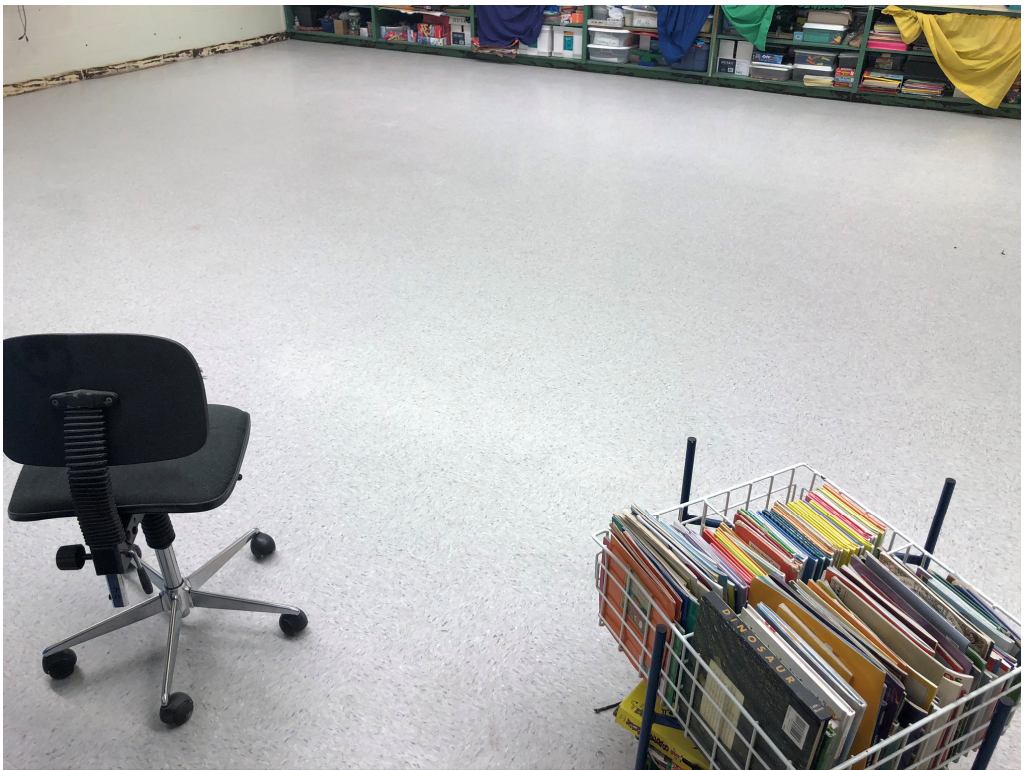
Figure 6 – West Section of Building A New Floor
