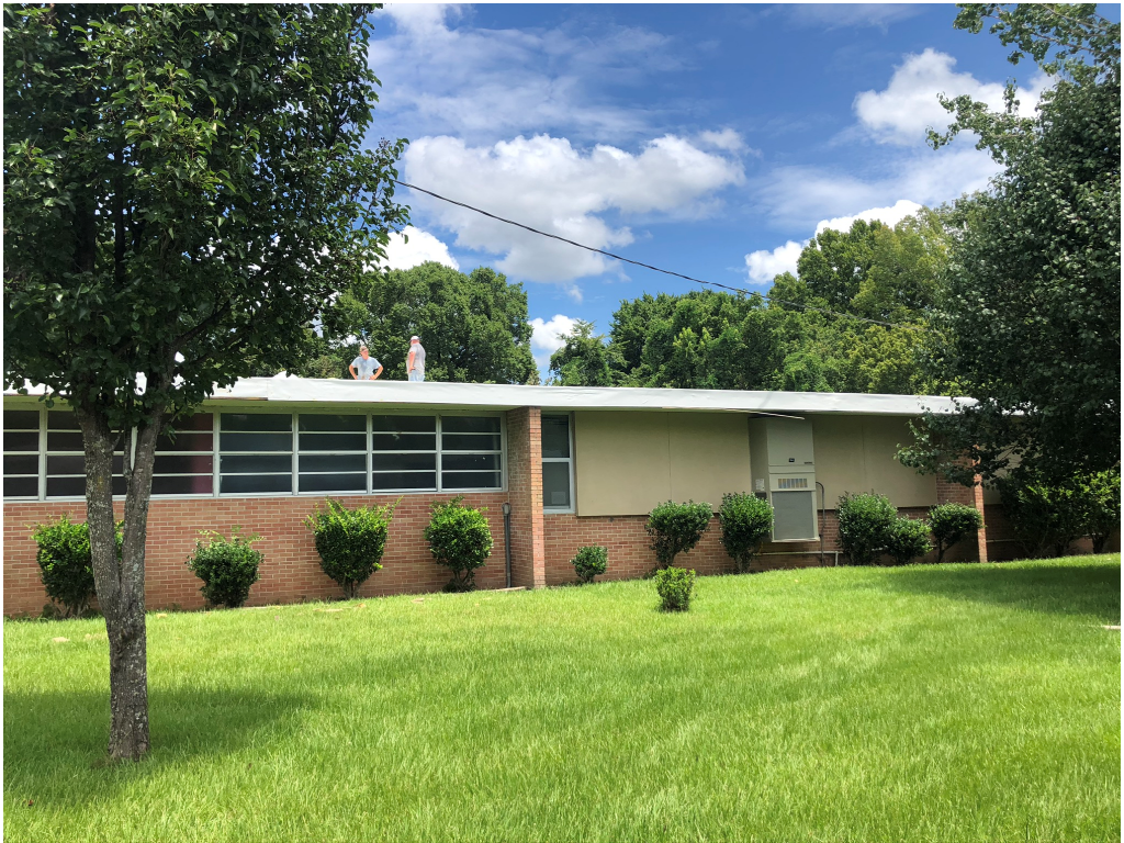
Figure 8 – Roof Work Complete; Edge Trim Still Ongoing
