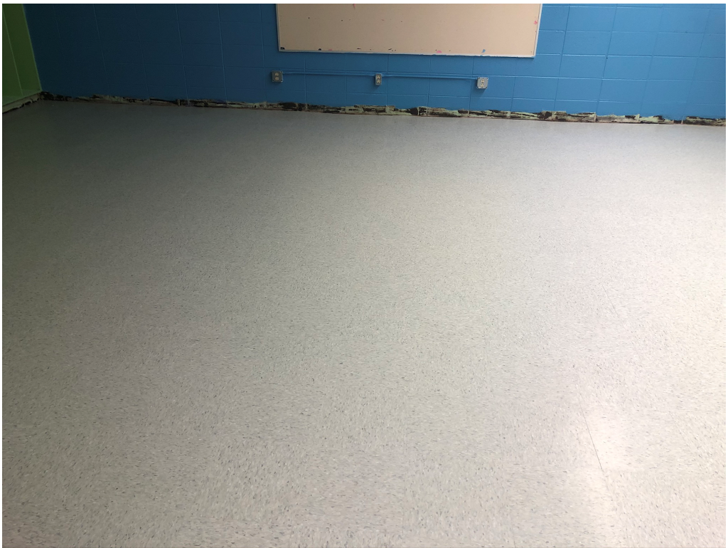
Figure 2 – West Section of Building A New Floor
