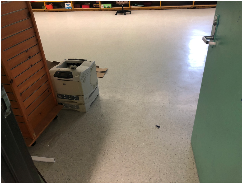
Figure 1 – West Section of Building A New Floor
