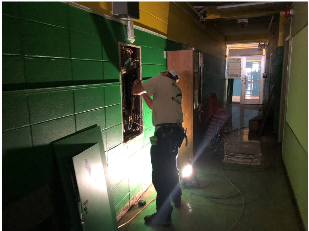
Figure 4 – Electrical Work @ Building A
