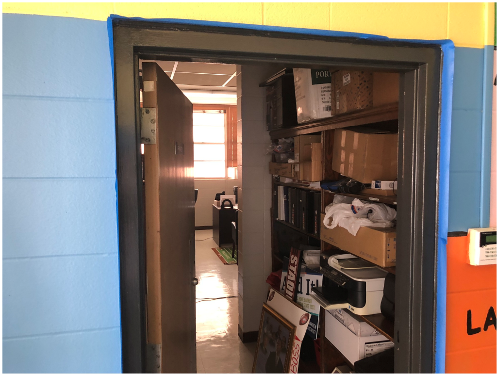
Figure 1 – Interior Paint Work @ Building A
