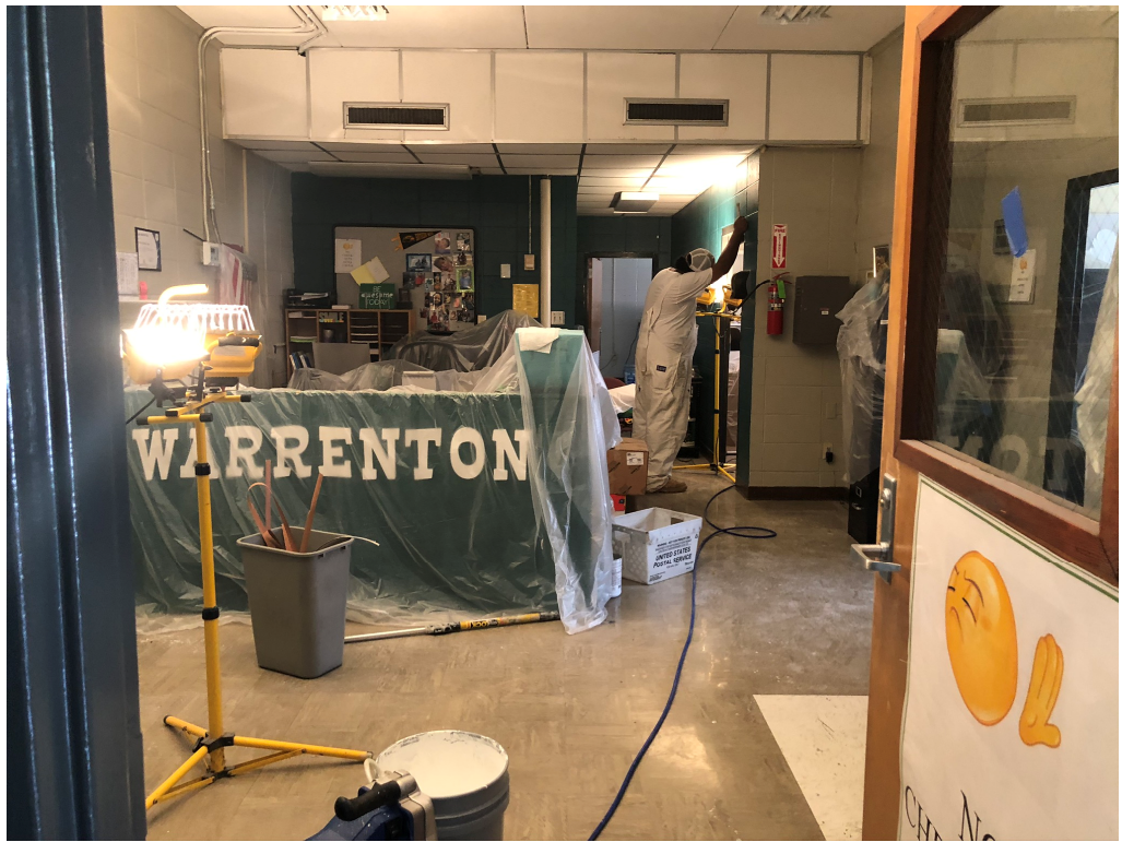
Figure 3 – Interior Paint Work @ Building A
