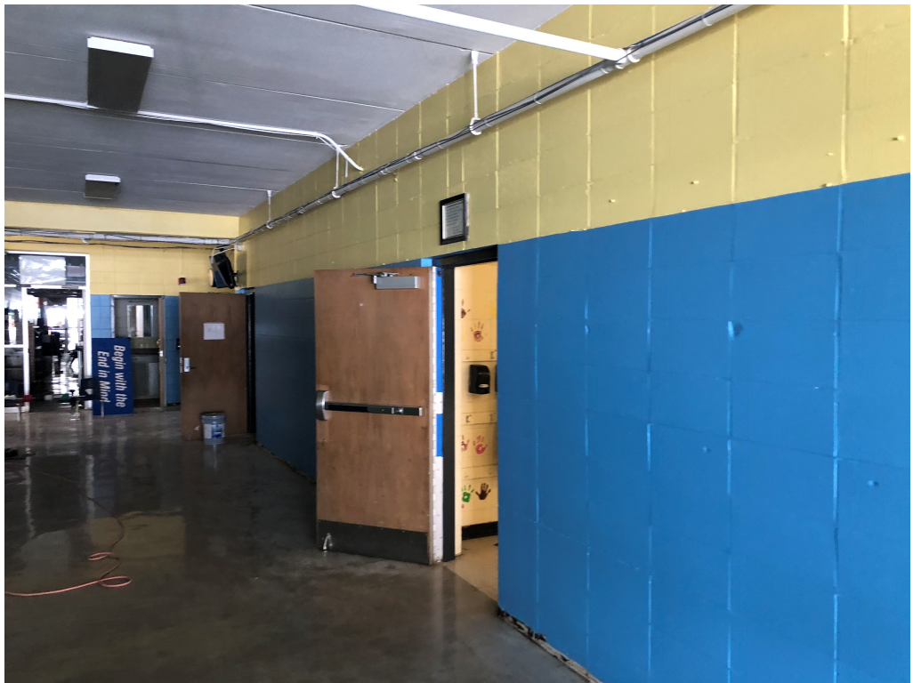
Figure 2 – Interior Paint Work @ Building A
