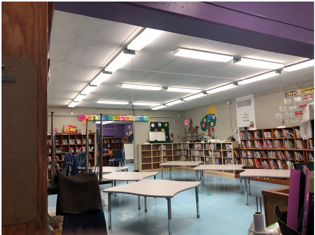
Figure 6 – Building C is in Similar Situation with Conduit Above; From Below it is impossible to know whether or no the conduit is embedded in the above roof deck or not
