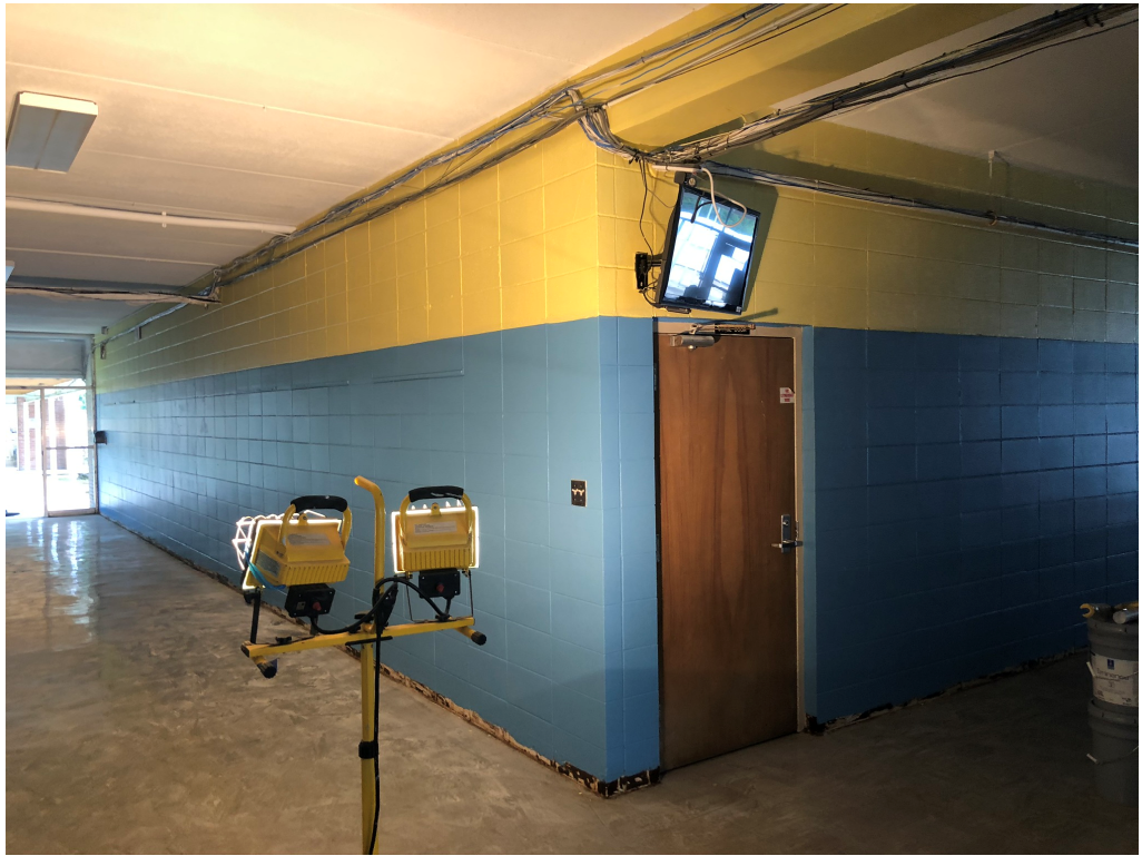
Figure 5 – Interior Paint Work @ Building A
