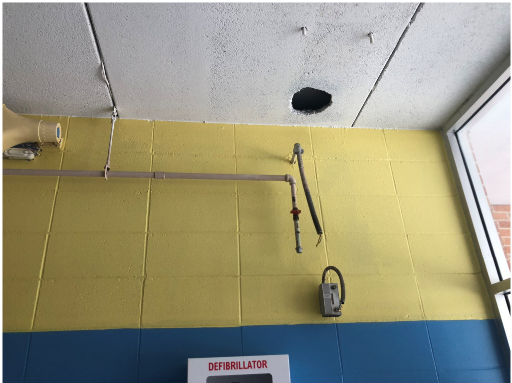
Figure 6 – Heater Removed @ Building A
