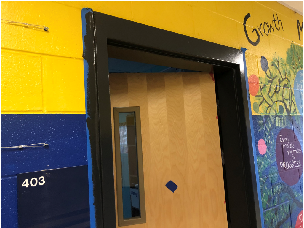
Figure 1 – Interior Paint Work @ Building D
