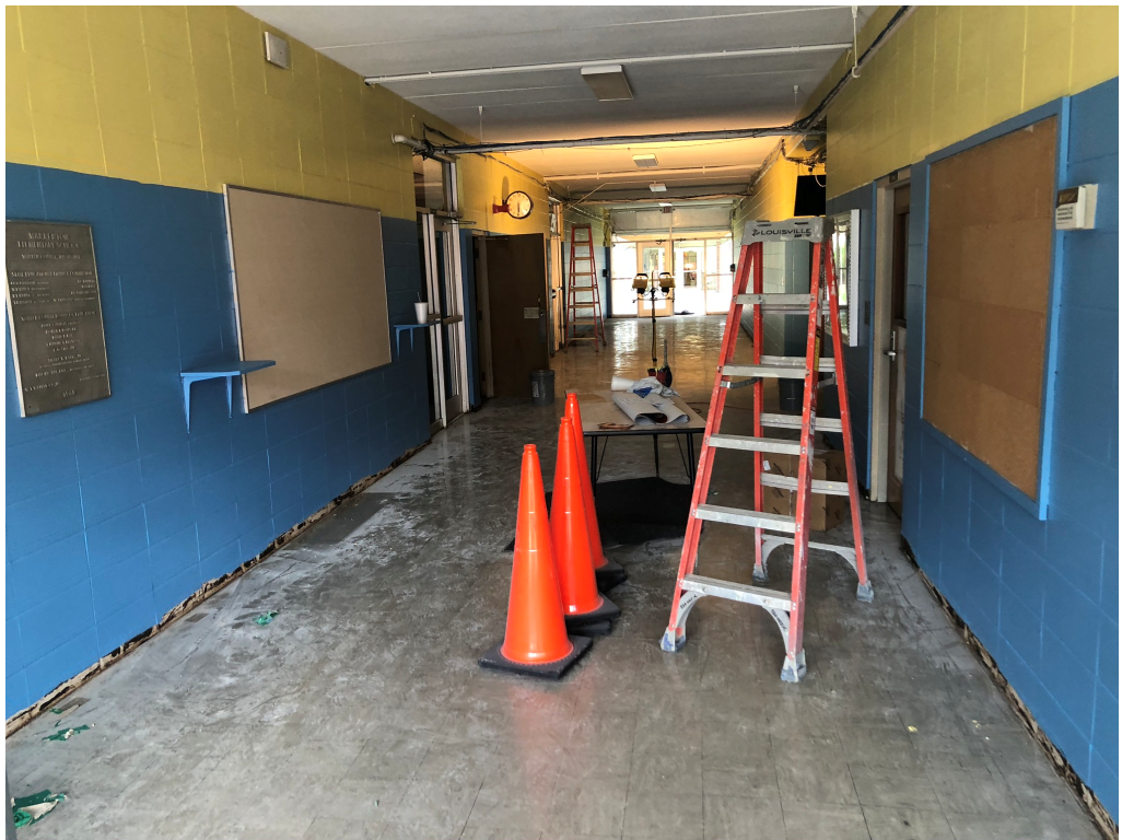
Figure 4 – Interior Paint Work @ Building A
