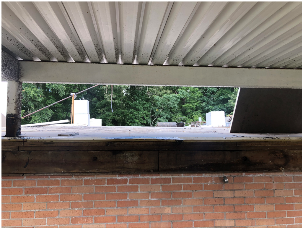
Figure 3 – Roofing Work @ Building B
