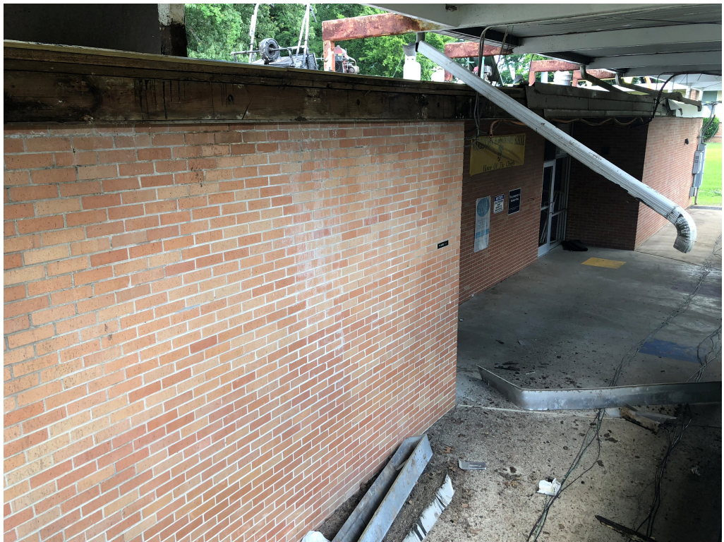
Figure 2 – Roofing Work @ Building B
