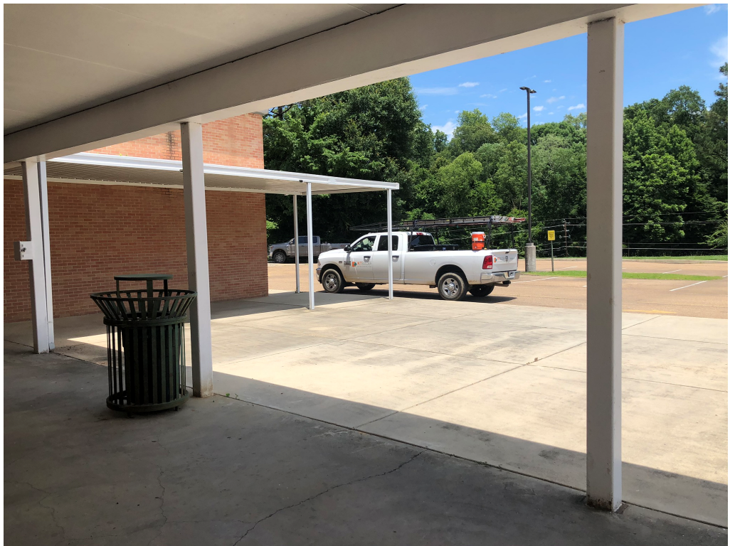
Figure 2 – Contractor On Site (First Day)
