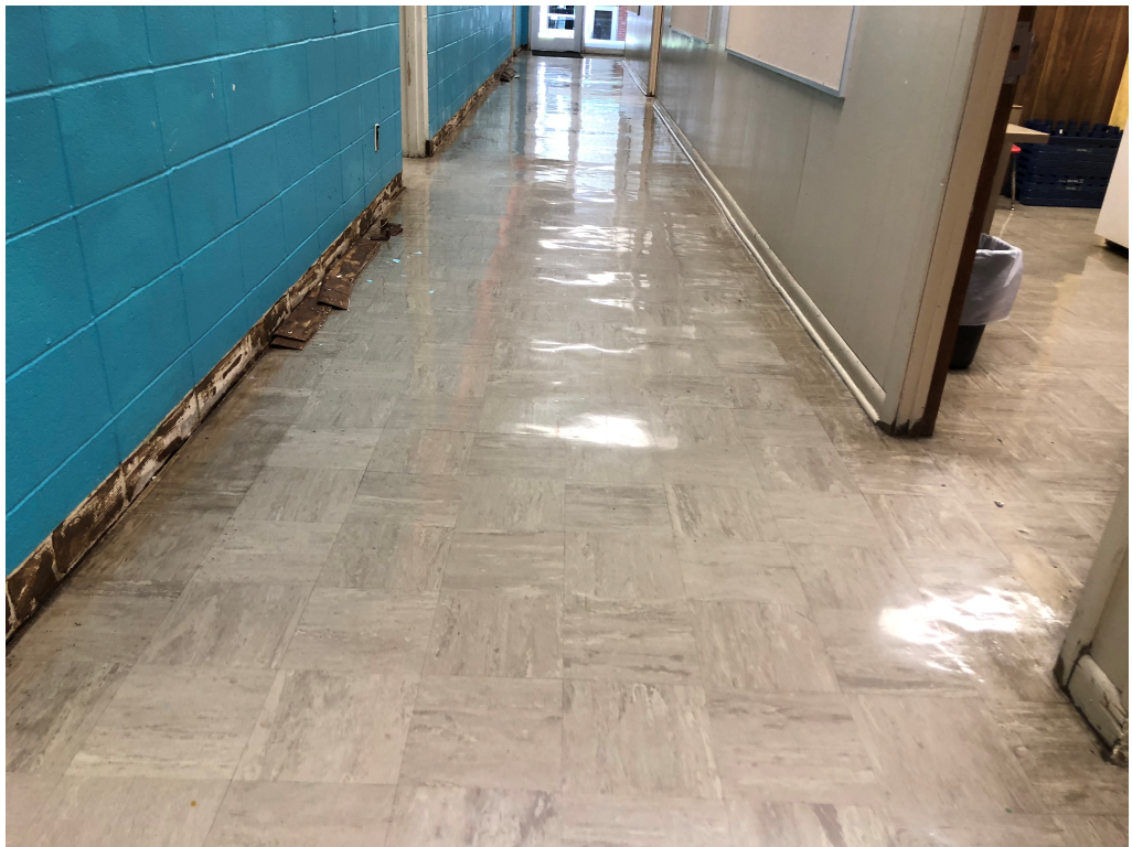
Figure 4 – Floor Base Removal Ongoing
