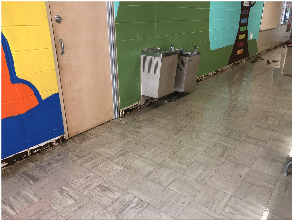
Figure 3 – Floor Base Removal Ongoing
