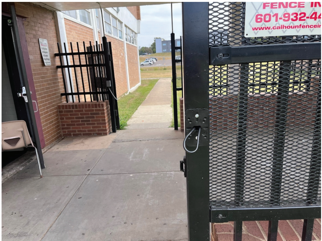
Figure 11 – School Replacing Keypads
