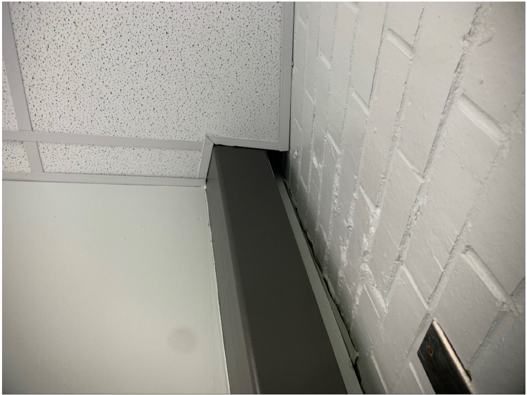
Figure 15 – Fill gap with matching trim
