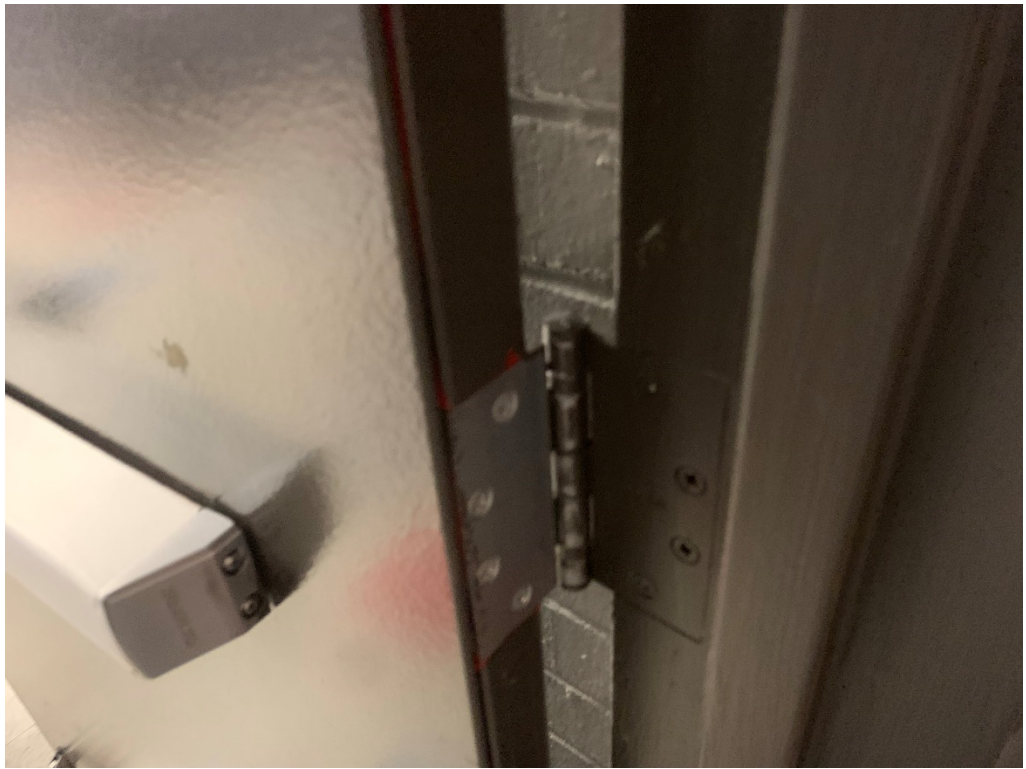
Figure 21 – Remove paint at hardware
