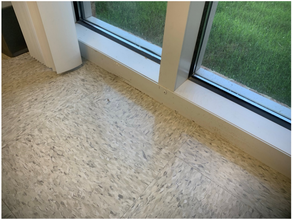
Figure 3 – New storefront to be cleaned/refinished at A-305
