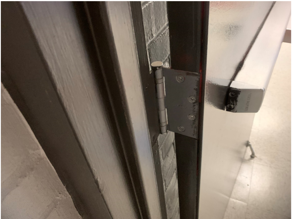
Figure 20 – Remove paint at hardware
