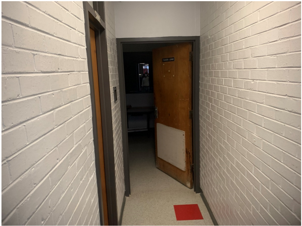
Figure 13 – Door to be removed per Construction Documents
