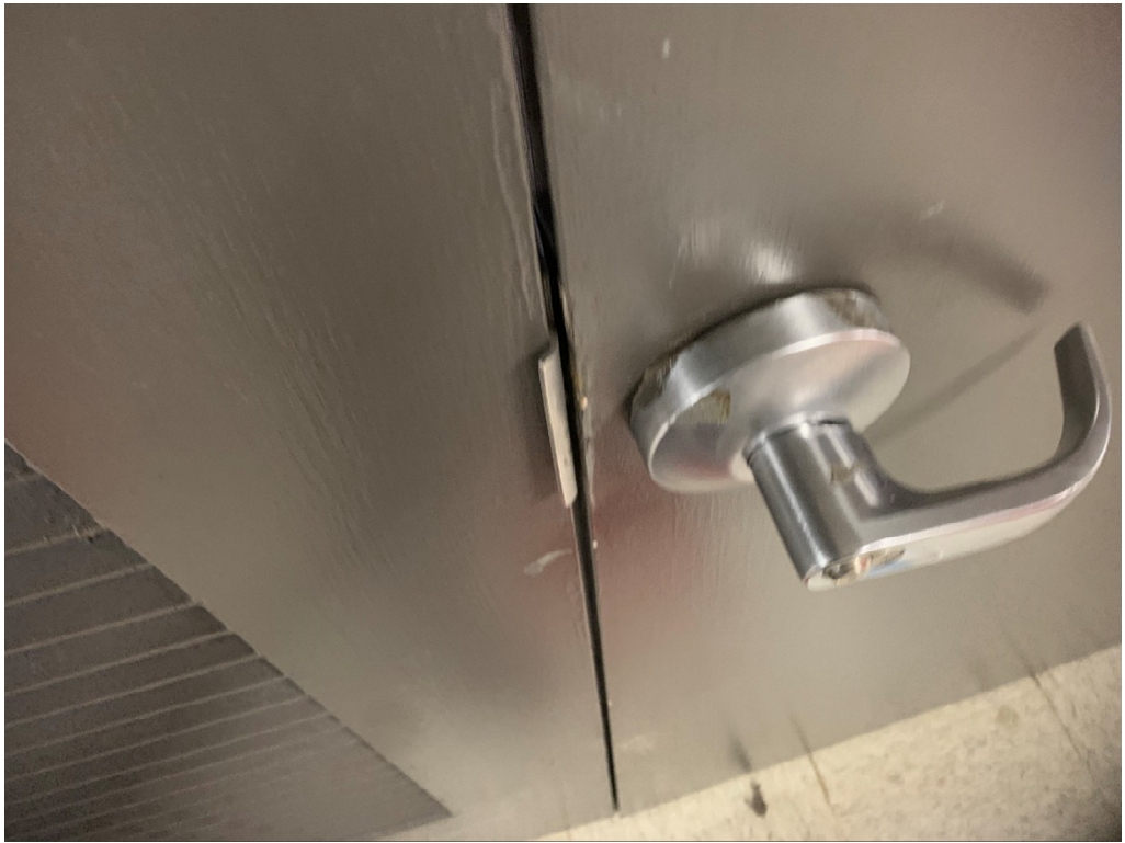
Figure 19 – Remove paint at hardware
