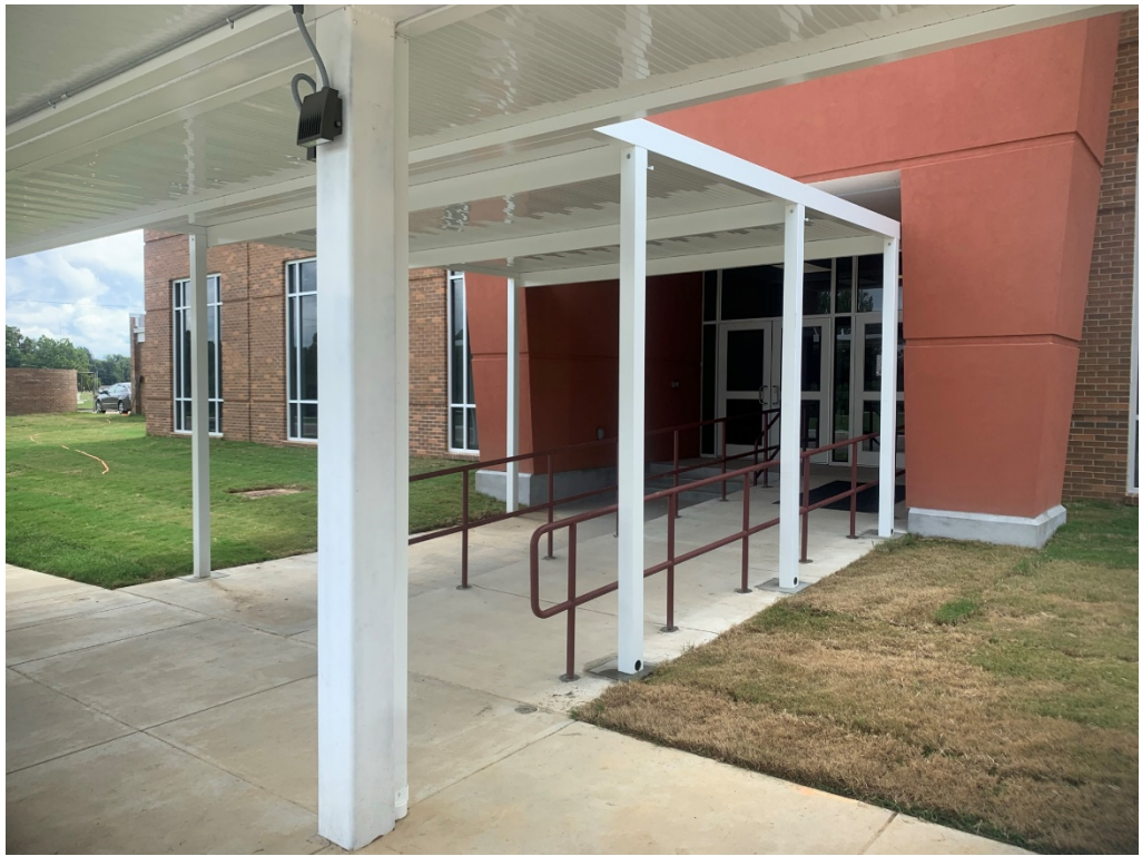
Figure 1 – Handrail Partially Installed
