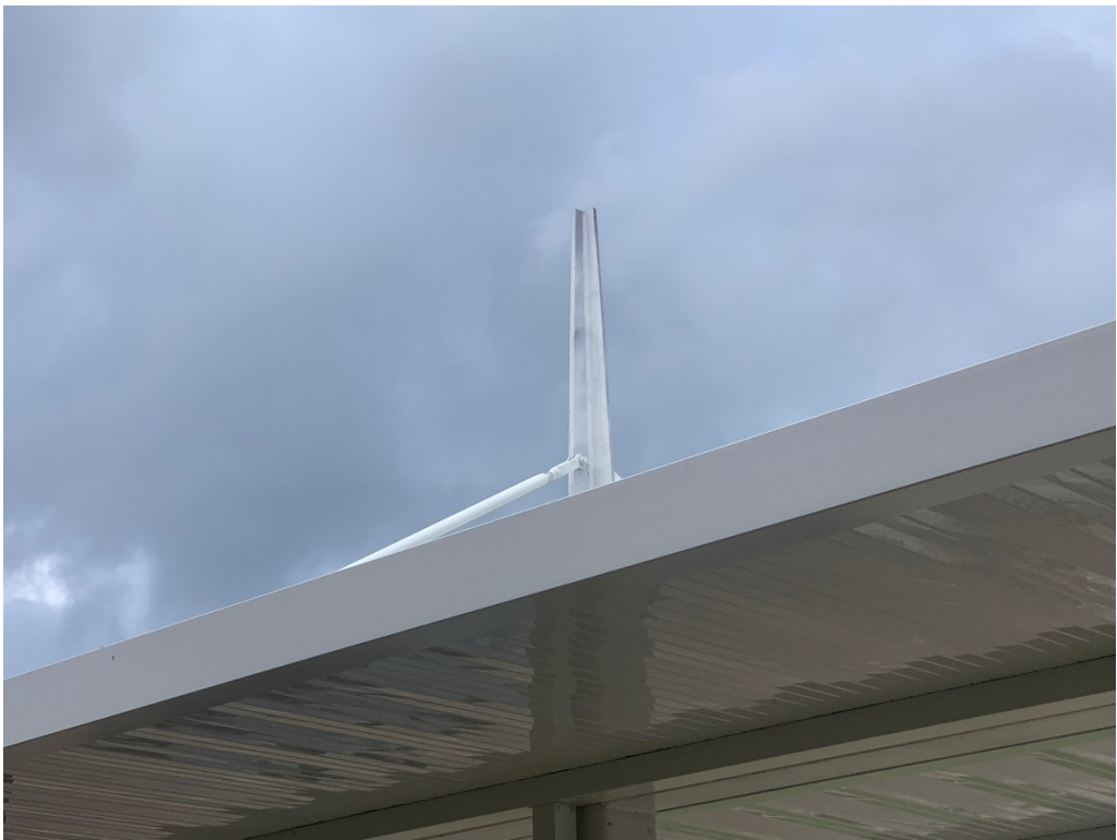
Figure 4 – Final coating needed at steel
