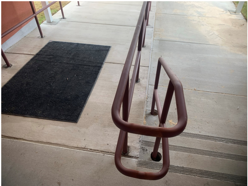
Figure 2 – Straighten handrail to lengths are parallel
