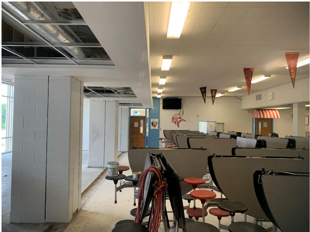
Figure 4 – Temporary Divider Removed at Cafeteria
