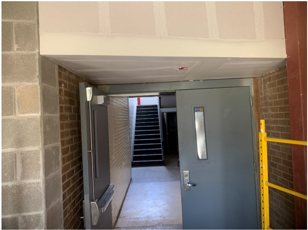
Figure 5 – Corridor Addition Opened Up
