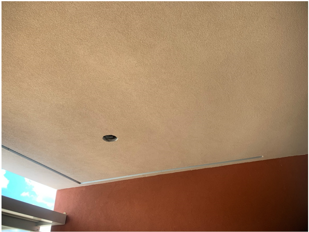
Figure 3 – Stucco Work at Entry Complete
