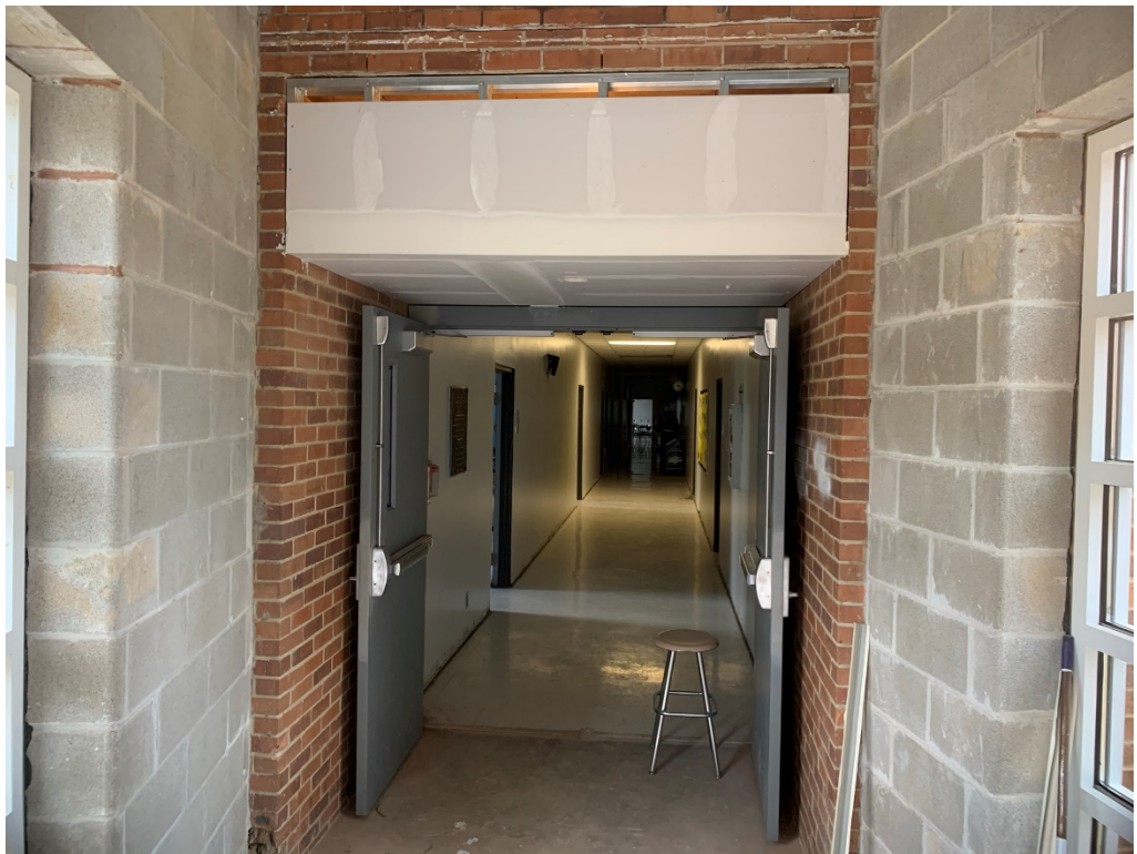
Figure 6 – Corridor Addition Opened Up
