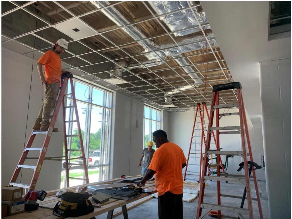
Figure 3 – Fire Alarm Installers at Work Throughout
