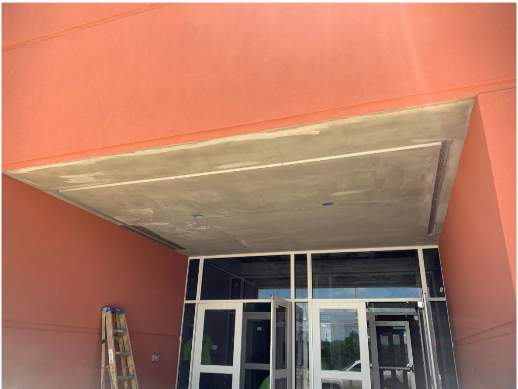
Figure 2 – Stucco in Progress at Ceiling
