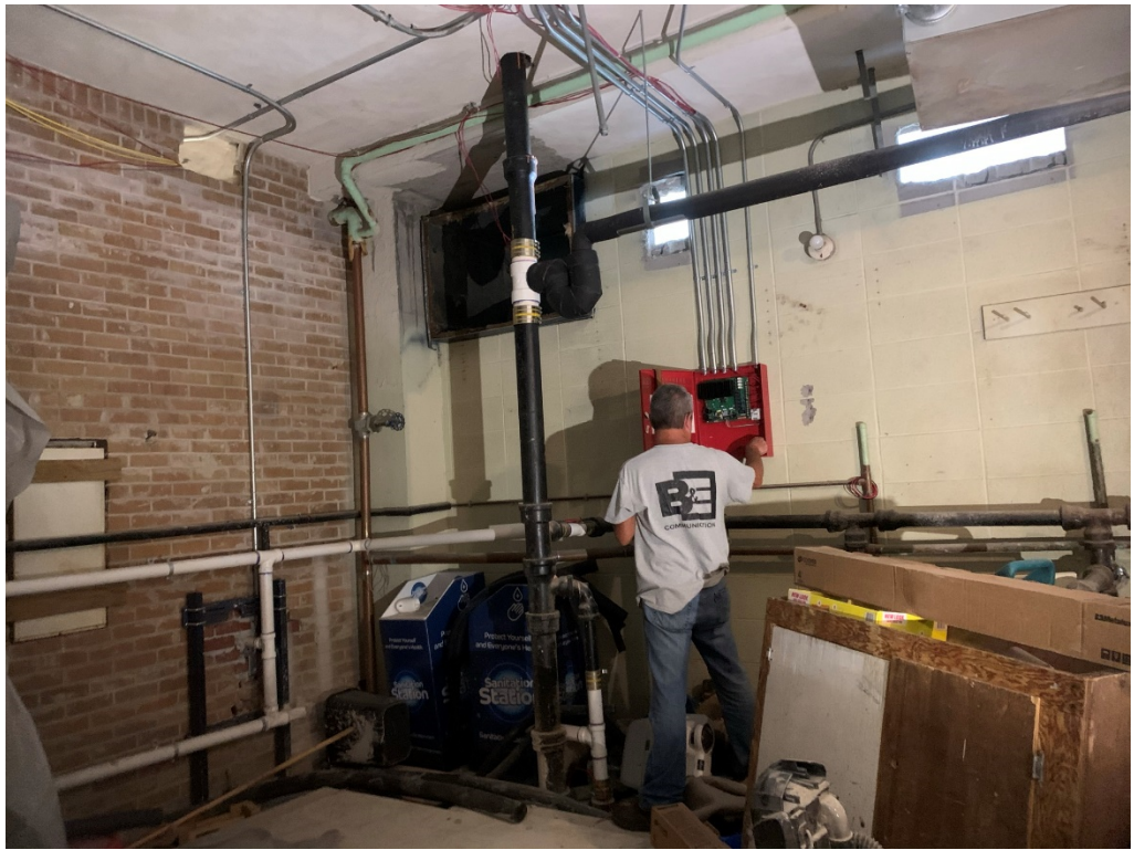
Figure 5 – Fire Alarm Installers at Work Throughout
