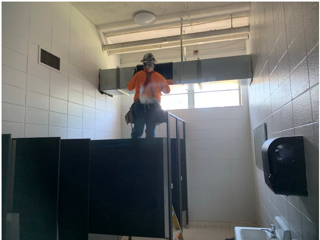
Figure 6 – Mechanical Workers at Lower Level
