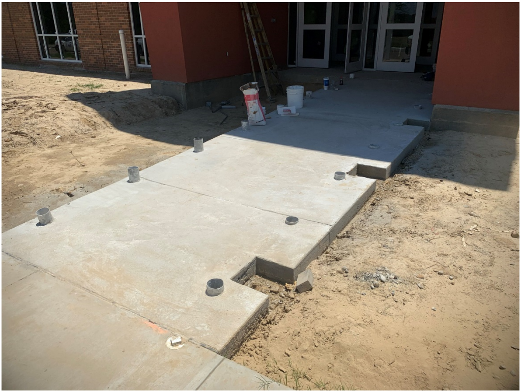
Figure 1 – Newly Install Concrete at Front Entry
