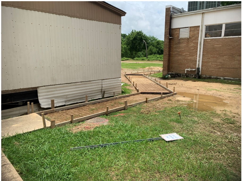
Figure 10 – Sidewalk Formed
