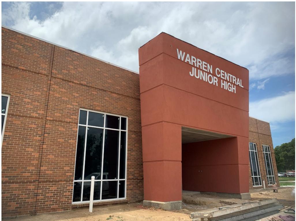
Figure 2 – Progress at Entry
