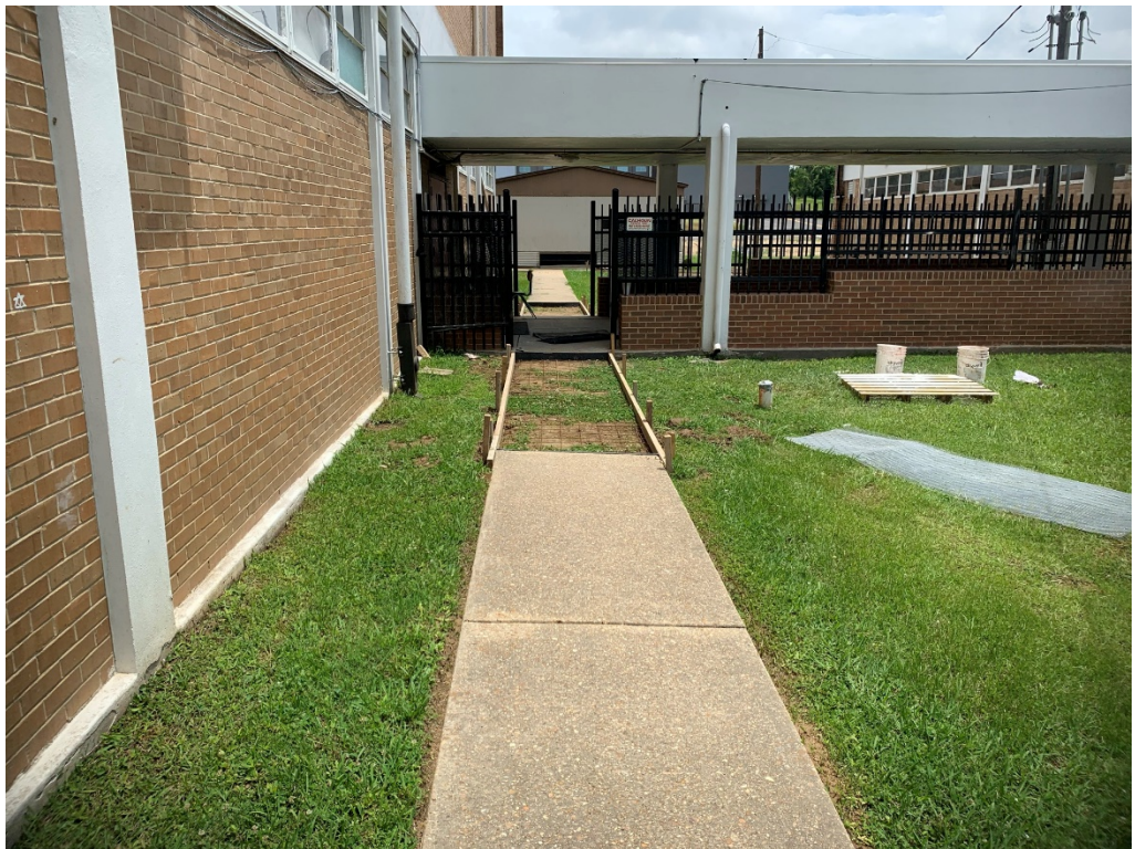
Figure 6 – Sidewalk Formed (vegetation should be removed before concrete installed)
