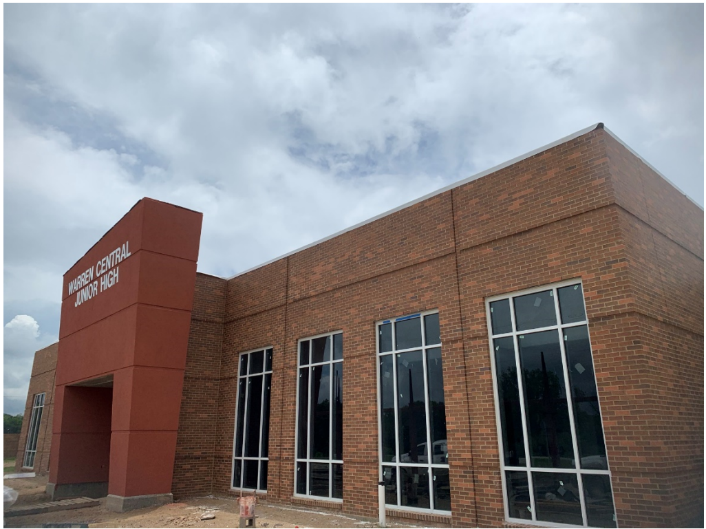
Figure 1 – Progress at Entry
