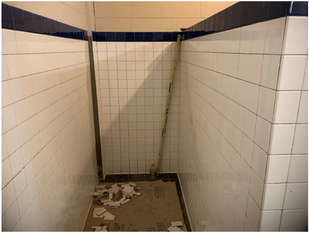
Figure 9 – Tile at Field House
