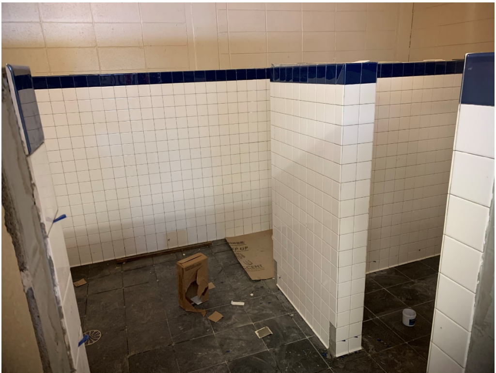
Figure 8 – Tile at Field House
