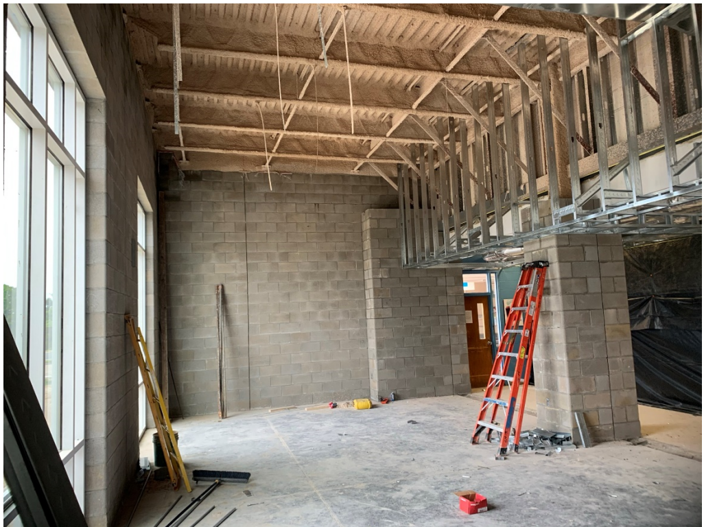
Figure 6 – Cafeteria Addition Space
