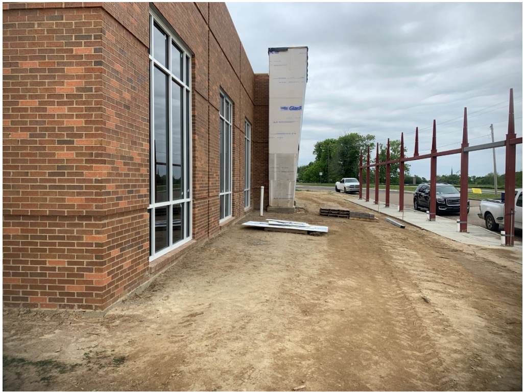
Figure 1 – Curtain Wall Installed at addition
