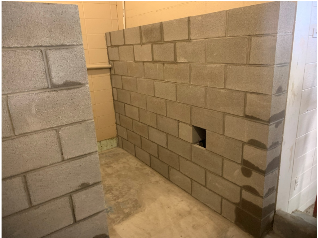
Figure 13 – Masonry Work at Field House Bathroom
