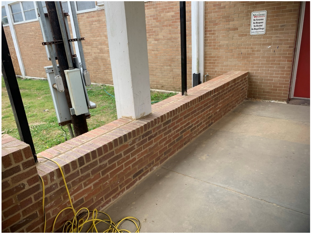
Figure 17 – Brick work at first floor connector
