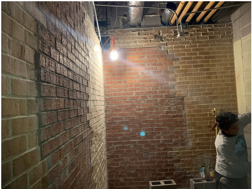
Figure 18 – Masonry Work in lowest floor bathroom
