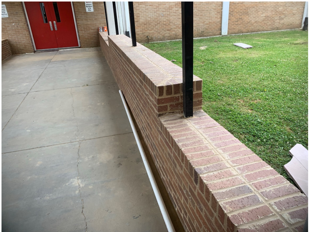
Figure 16 – Brick work at first floor connector
