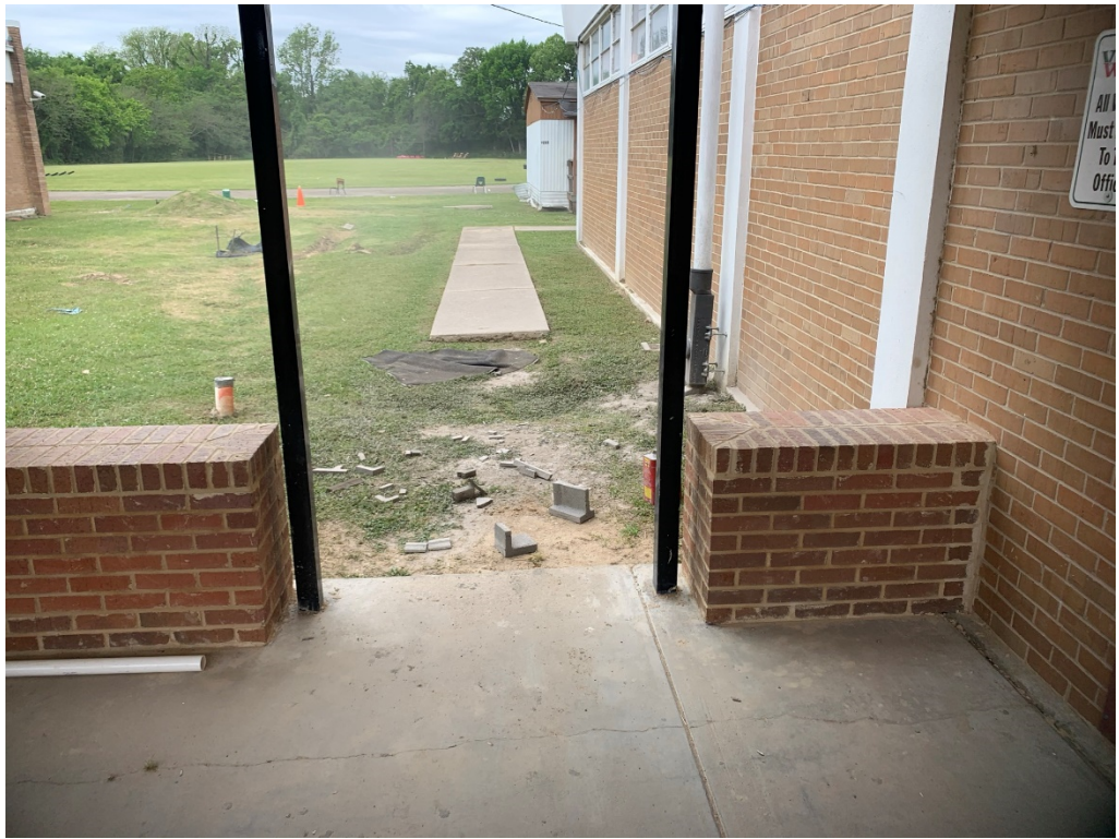
Figure 15 – Brick work at first floor connector
