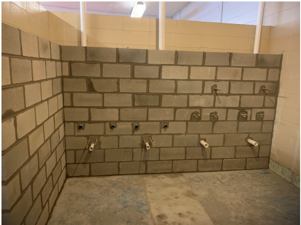
Figure 12 – Masonry Work at Field House Bathroom
