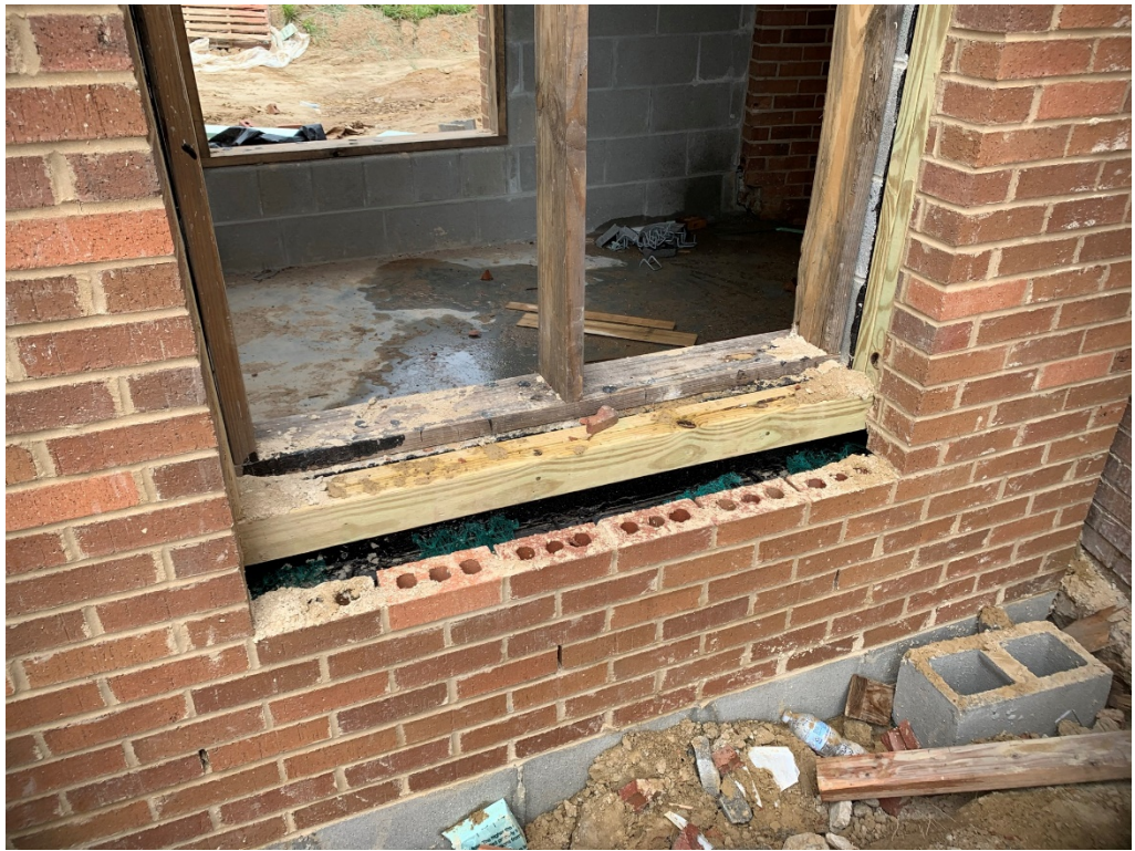
Figure 11 – Window Construction at 2 nd floor connector
