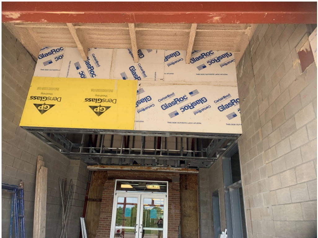
Figure 2 – Progress at main entry
