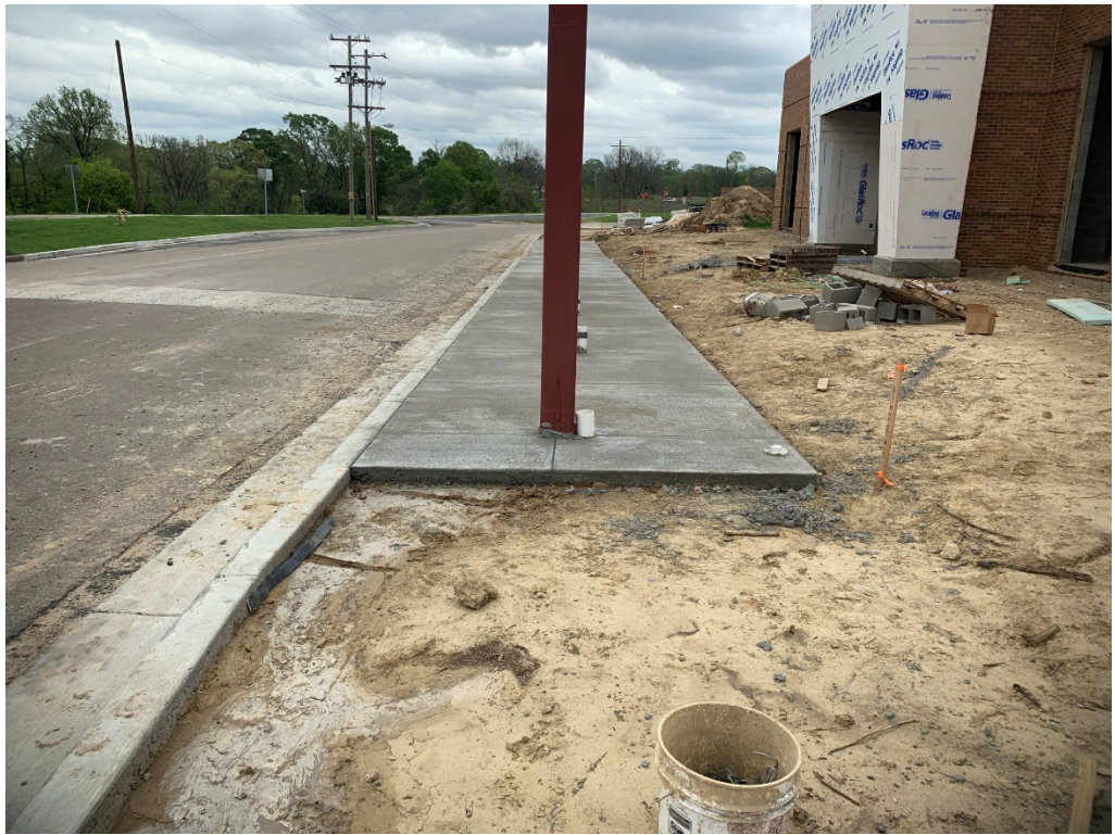
Figure 1 – New Sidewalk at Road
