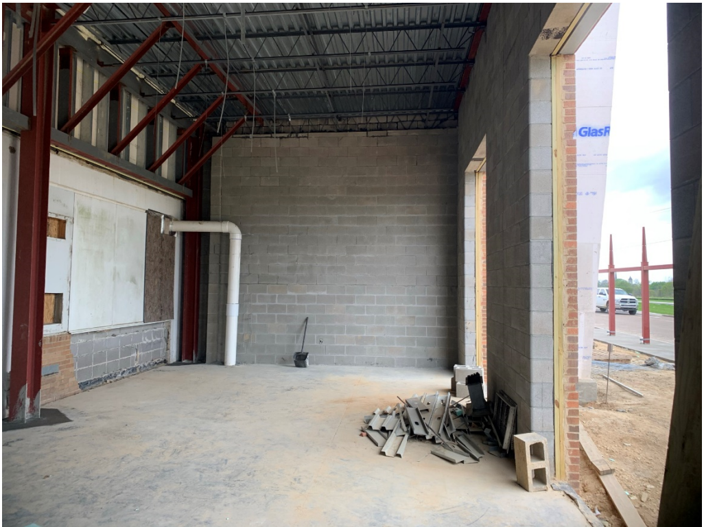
Figure 4 – New CMU Interior Wall
