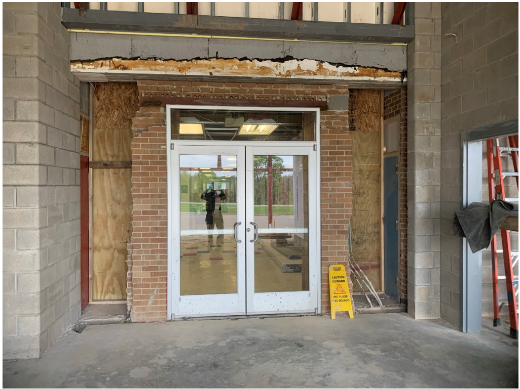
Figure 9 – Partially Demoed Entry
