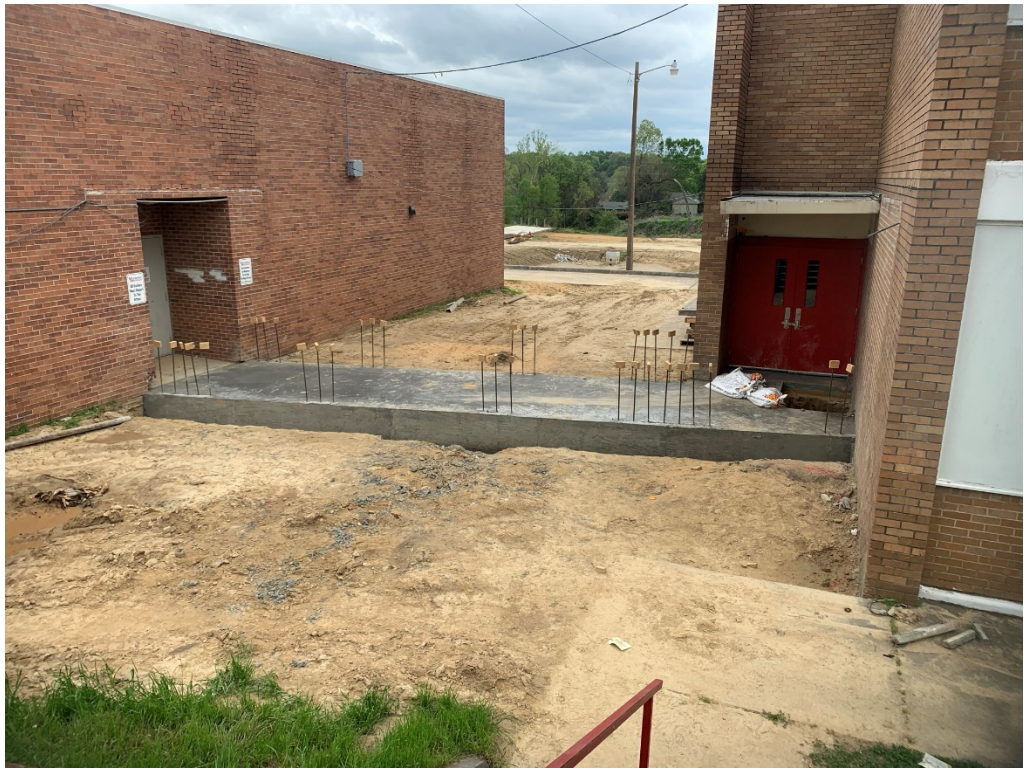
Figure 11 – New Slab @ Connector
