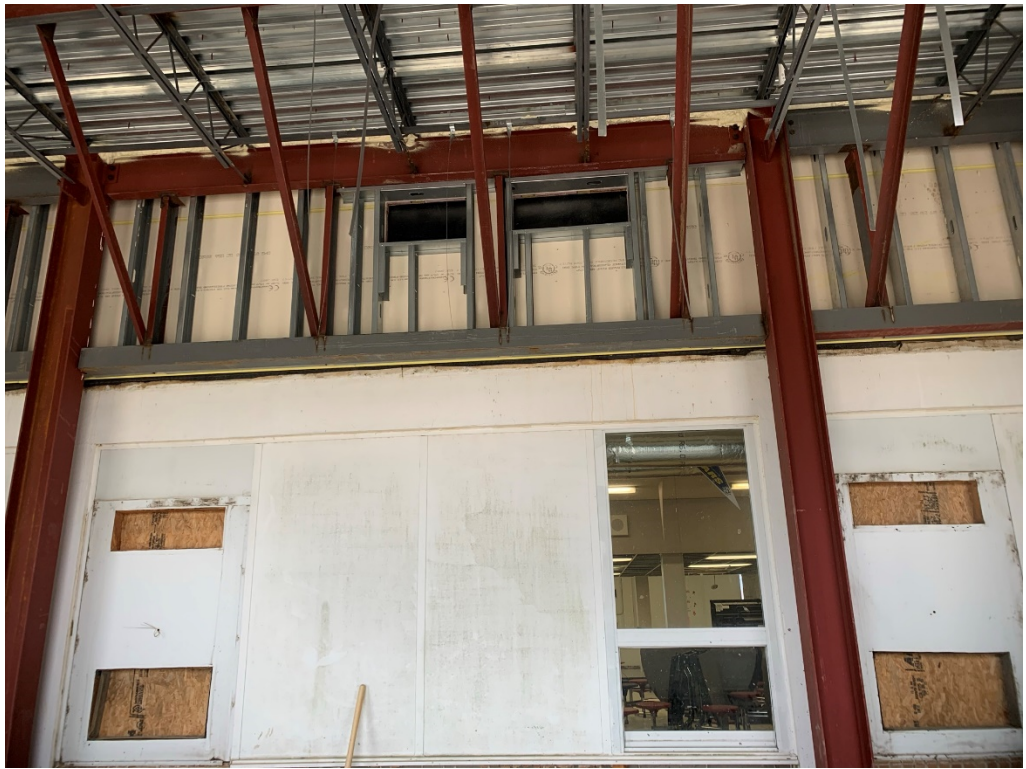
Figure 5 – Ducting Framed In
