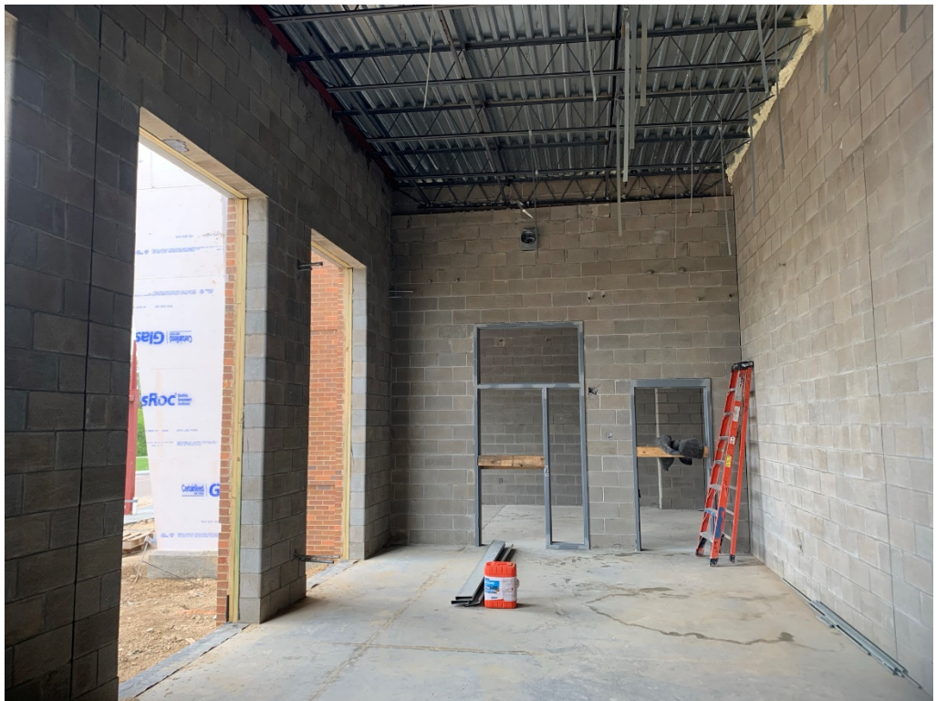
Figure 10 – New CMU Interior Wall with Frames
