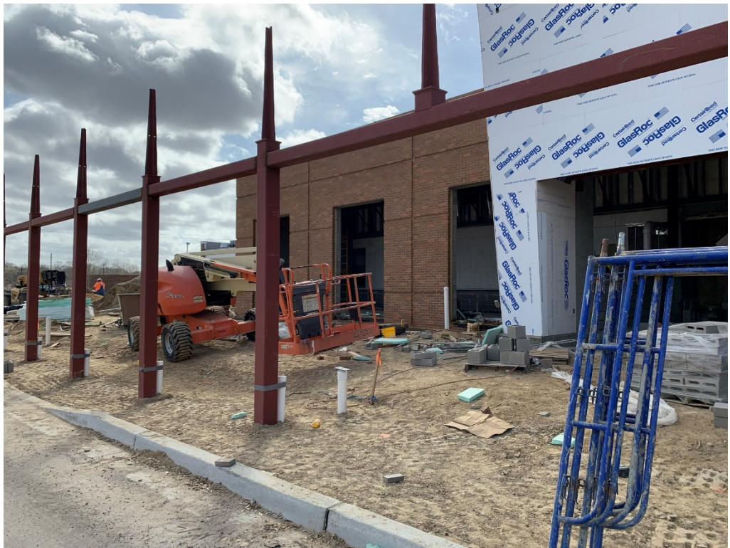
Figure 2 – North face of addition. When will spires be replaced with corrected spires?
