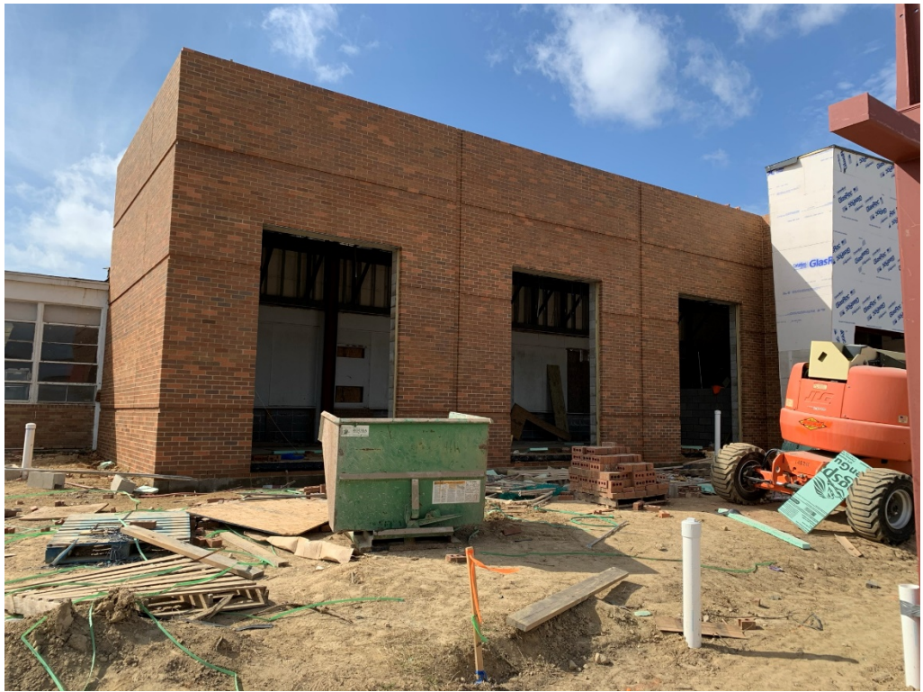
Figure 3 – Northeast corner of brick; brick reveals look good
