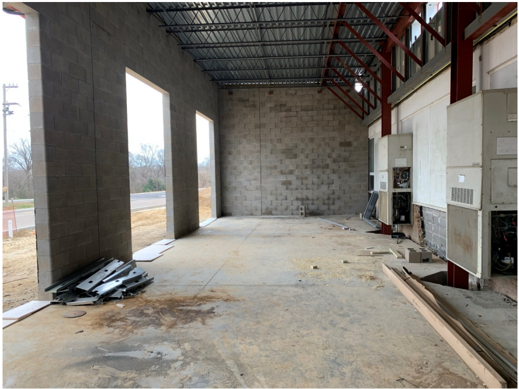
Figure 3 – Interior Addition Progress
