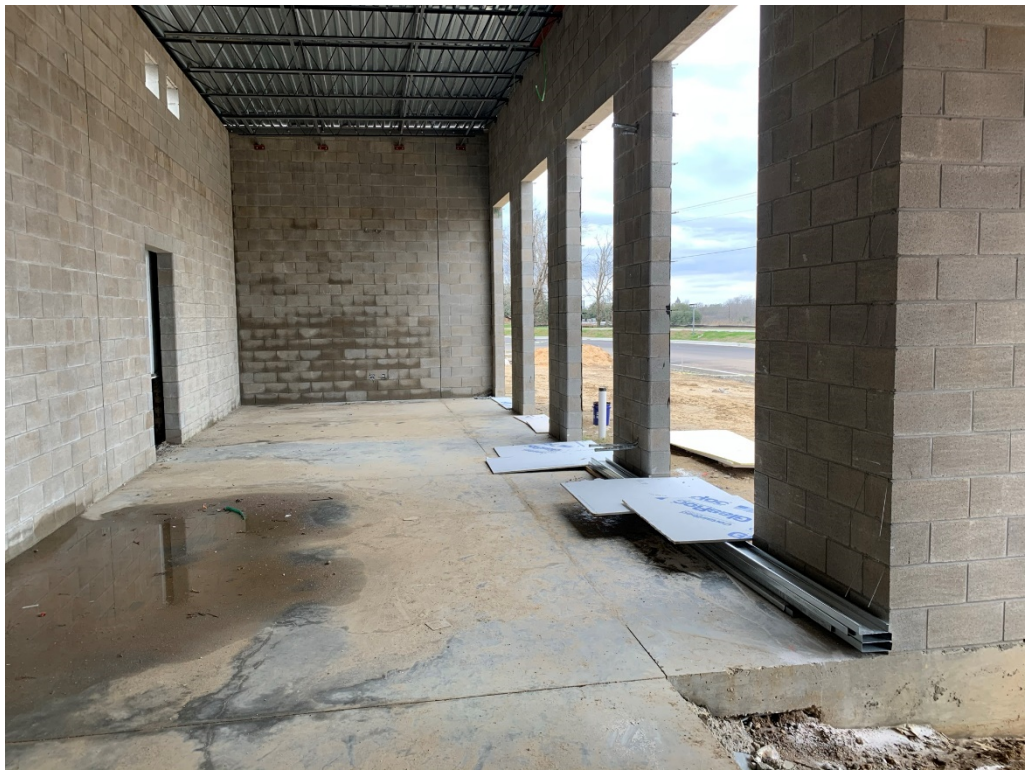
Figure 4 – Interior Addition Progress
