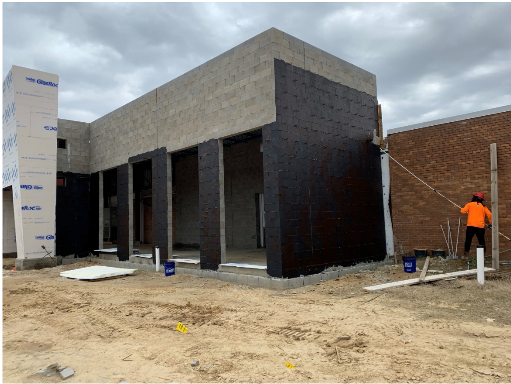
Figure 1 – Damp proofing at Exterior Masonry
