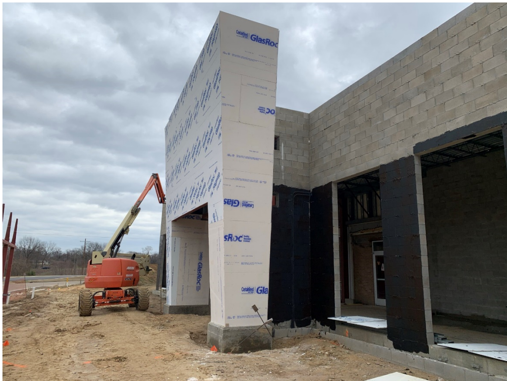
Figure 2 – Steel Entry Sheathing Wrapped
