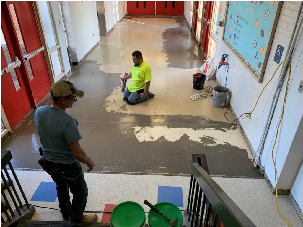
Figure 6 – Floor Work at Second Floor
