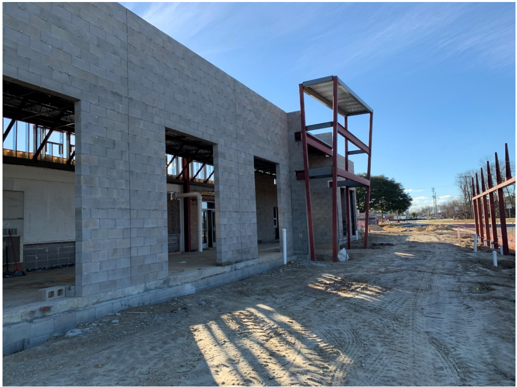
Figure 3 – Steel Entry Work
