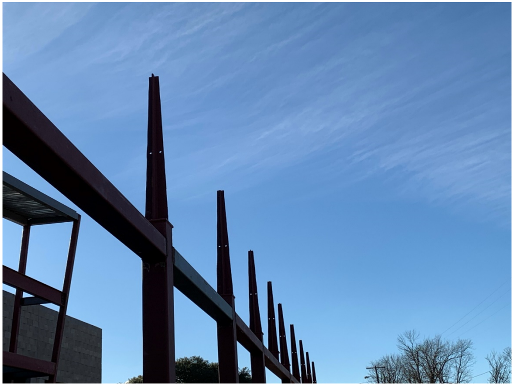
Figure 1 – Steel Spires need to Be Replaced with New spires that are cut Straight
