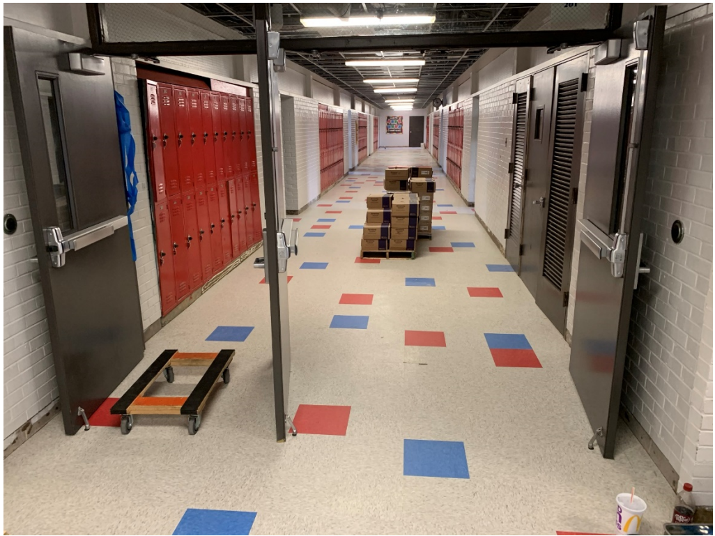
Figure 7 – Floor Work at Second Floor
