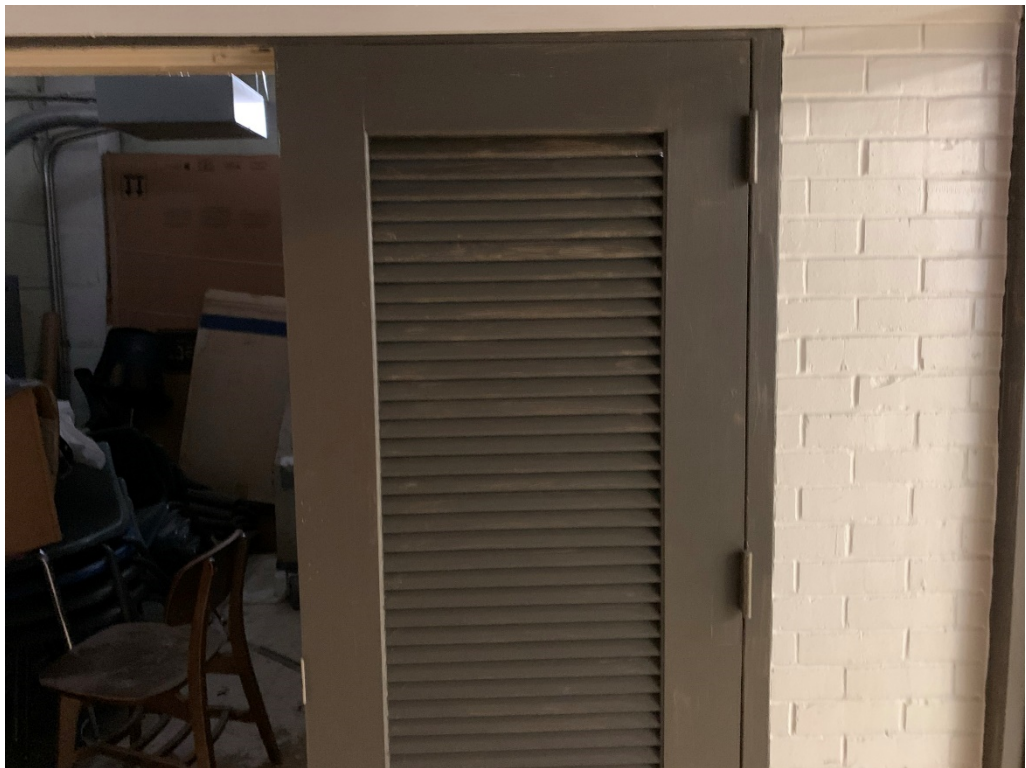
Figure 10 – Paint work is Ongoing
