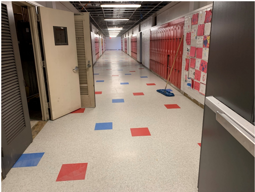
Figure 8 – Floor Work at Second Floor
