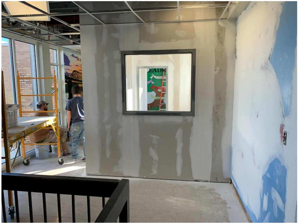
Figure 9 – Paint work is Ongoing
