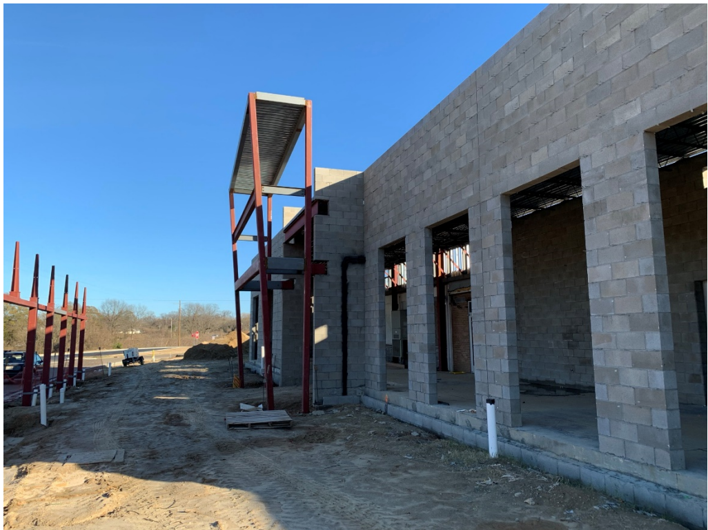
Figure 4 – Steel Entry Work
