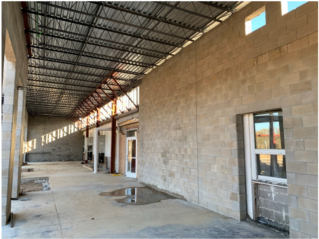
Figure 5 – Interior of New Addition
