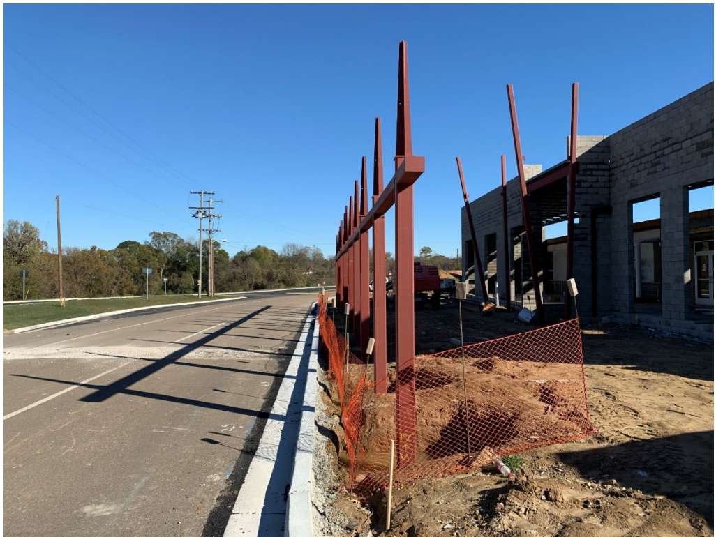
Figure 2 – Steel Work Partially Installed
