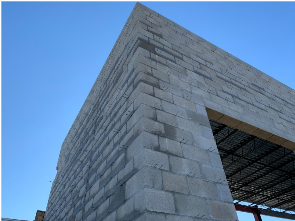
Figure 4 – Steel Work Partially Installed
