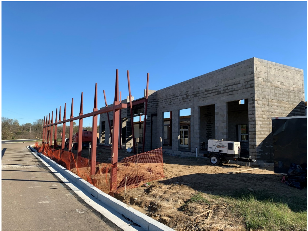
Figure 1 – CMU Blocked Installed
