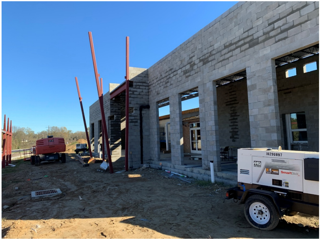
Figure 3 – Steel Work Partially Installed
