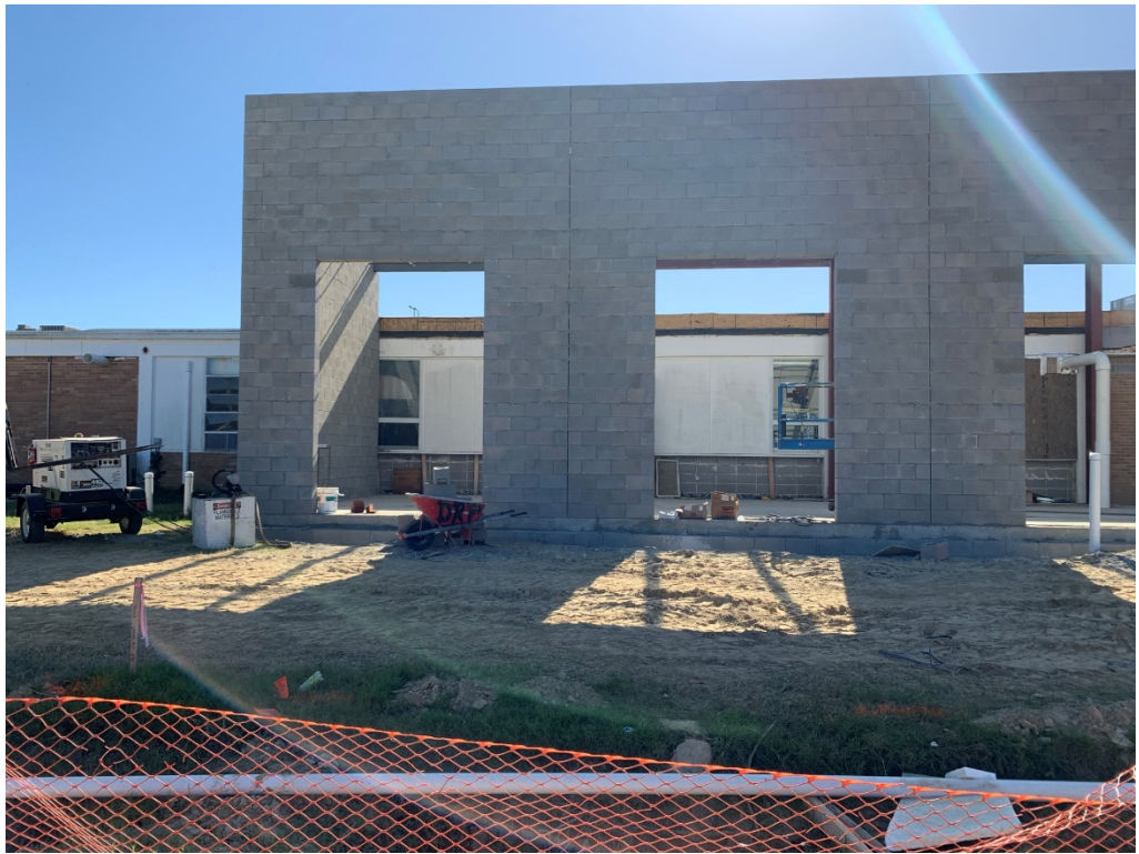
Figure 1 – CMU Blocked Installed
