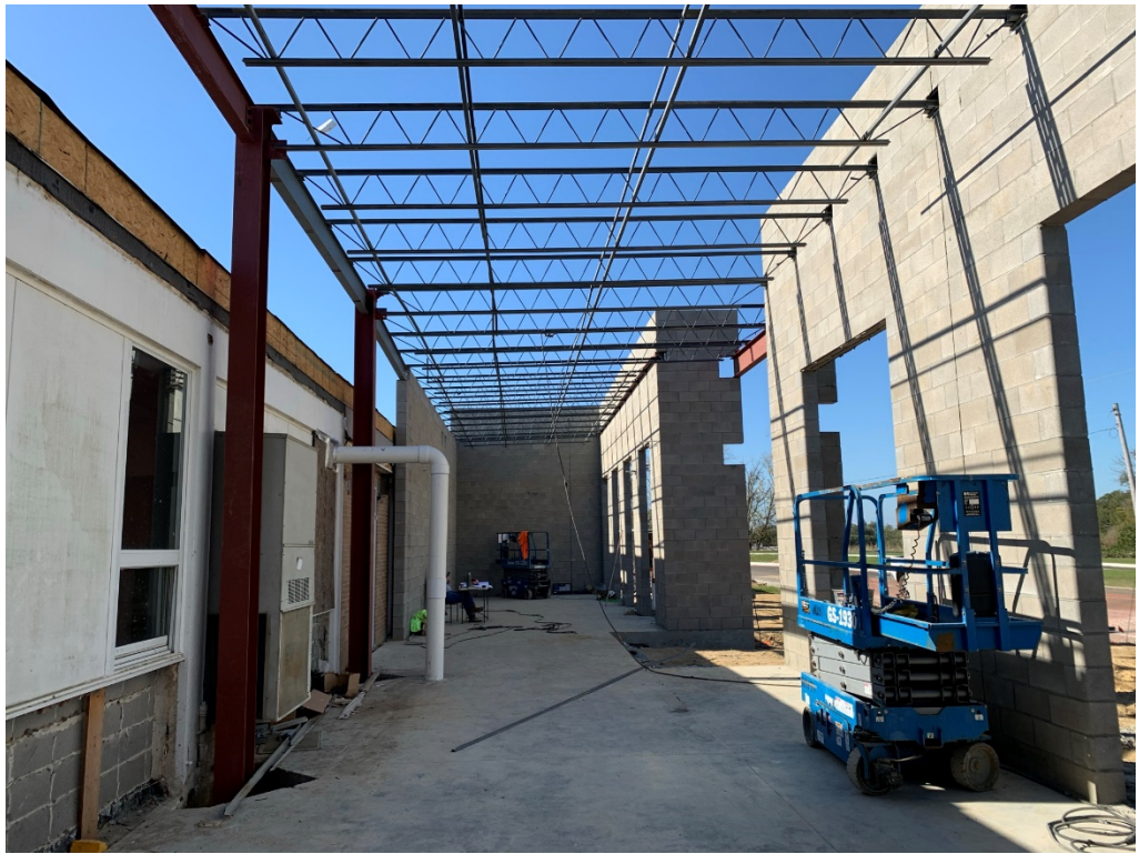
Figure 3 – Steel Work Partially Installed
