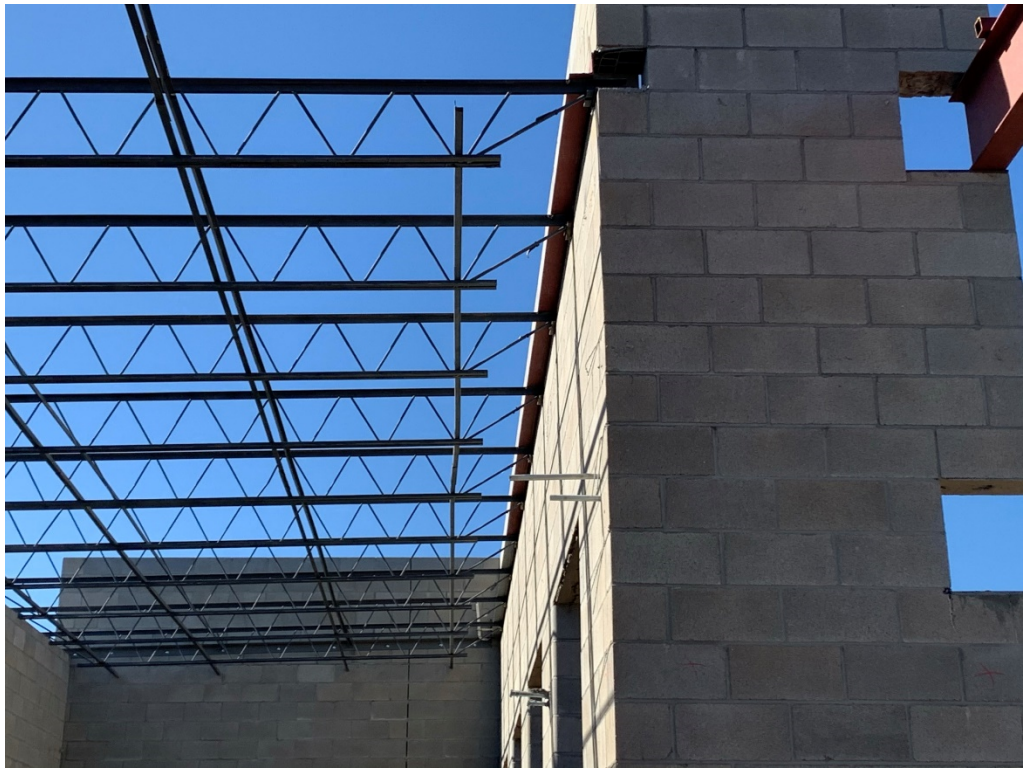
Figure 5 – Steel Work Partially Installed
