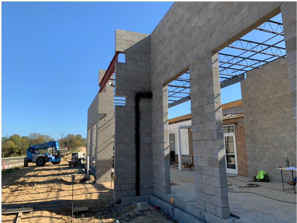
Figure 6 – Steel Work Partially Installed
