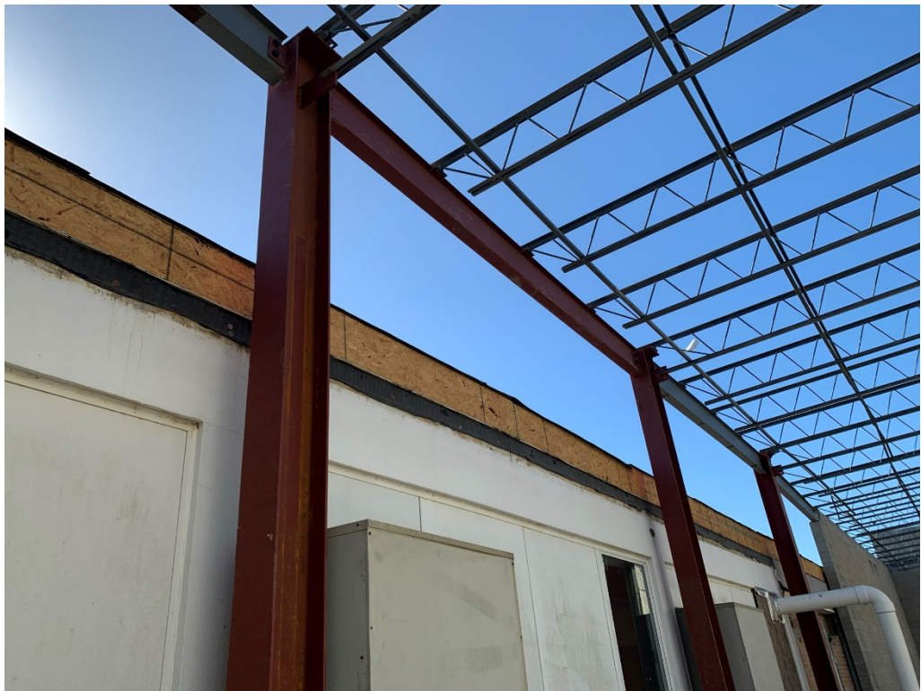
Figure 4 – Steel Work Partially Installed
