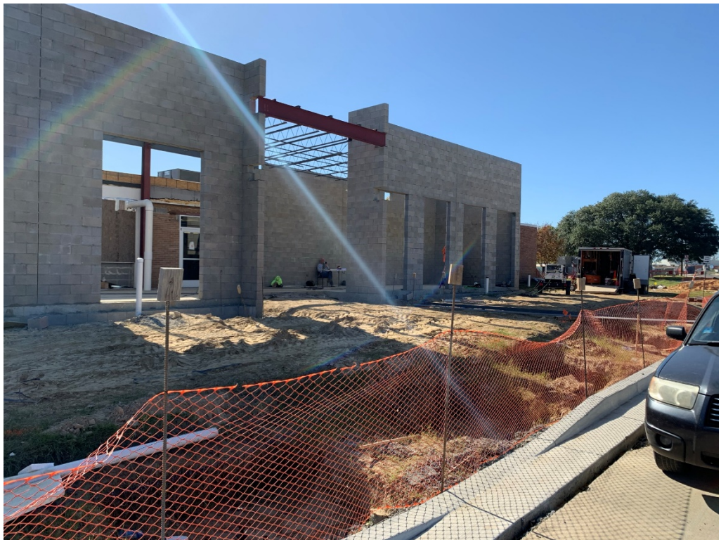
Figure 2 – Steel Work Partially Installed
