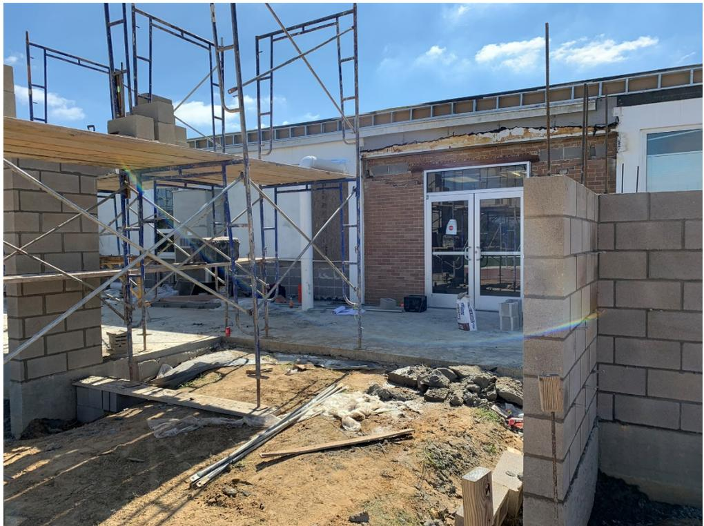
Figure 2 – CMU Blocked Install Ongoing
