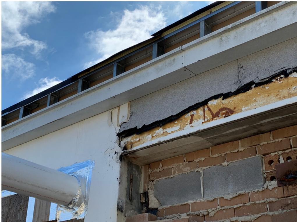
Figure 8 – Metal Stud Wall at Parapet
