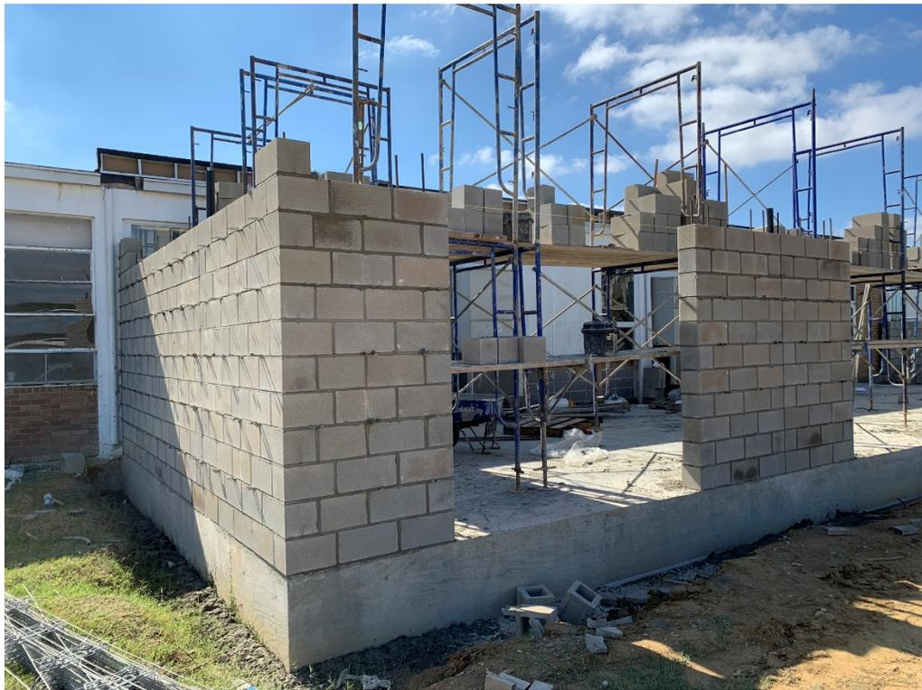
Figure 4 – CMU Blocked Install Ongoing
