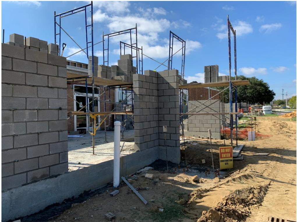
Figure 3 – CMU Blocked Install Ongoing
