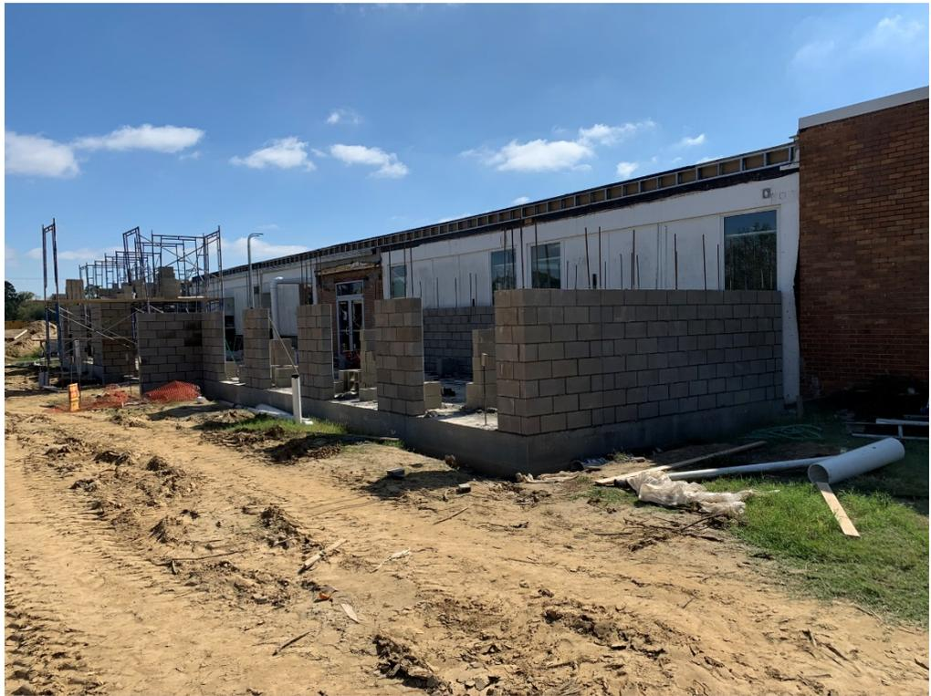
Figure 1 – CMU Blocked Install Ongoing
