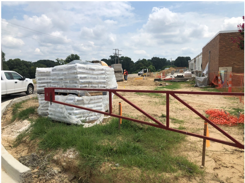
Figure 2 – Mortar Stored On Site
