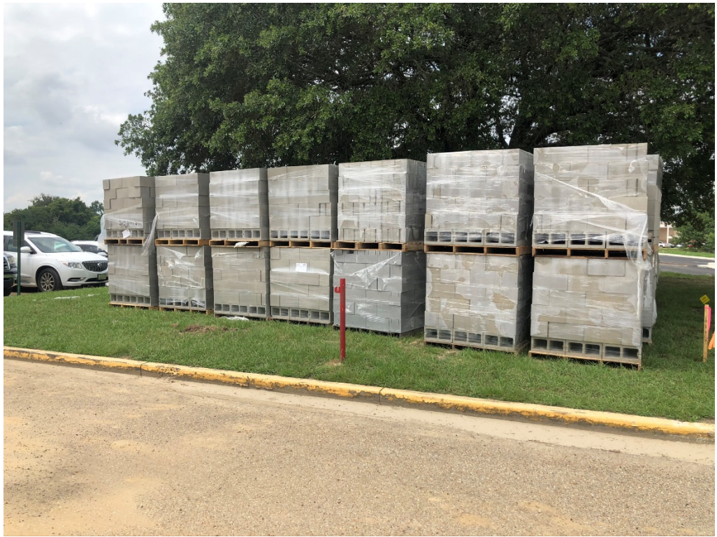
Figure 1 – CMU Stored On Site
