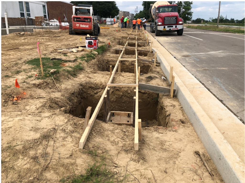
Figure 6 – Footings at Drop Off
