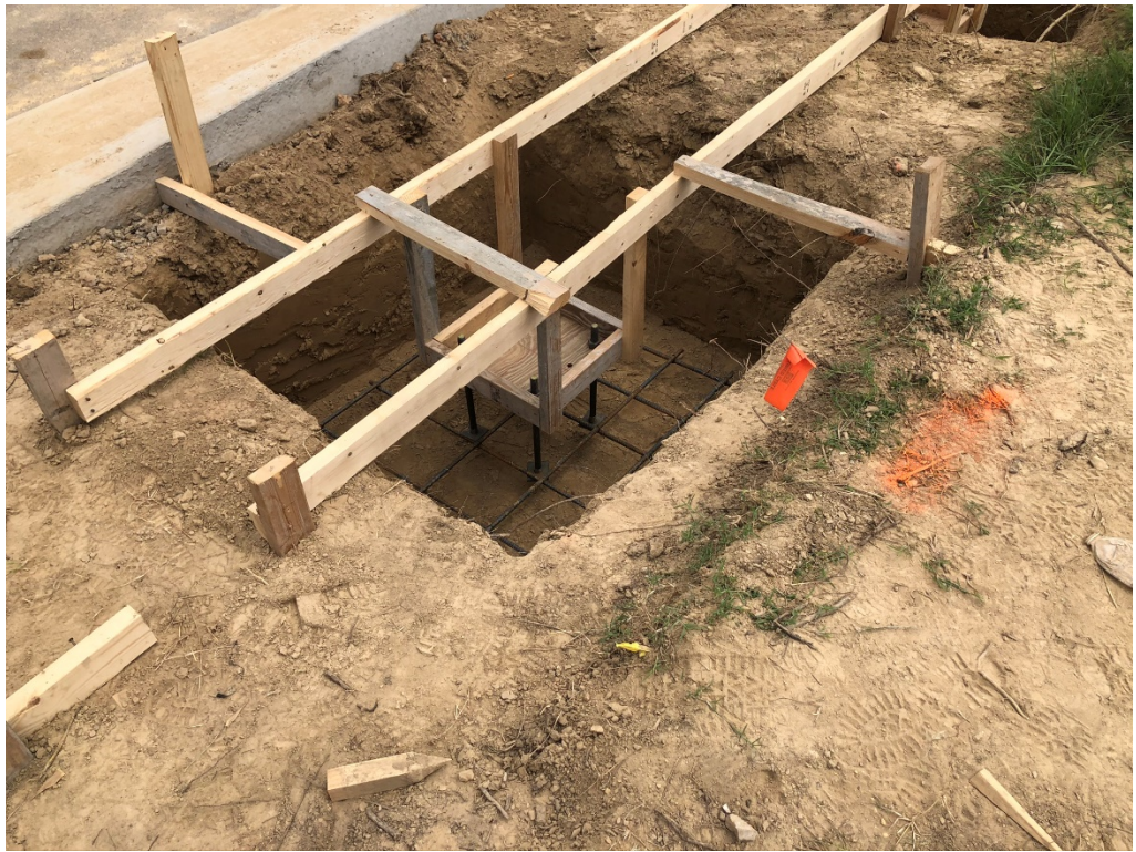
Figure 5 –Reinforcing @ Drop Off Footings
