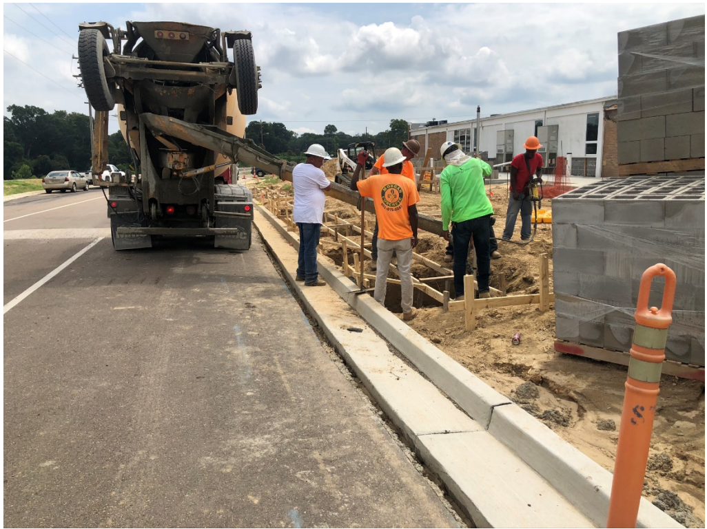
Figure 3 – Footing Pour at Drop Off Structure
