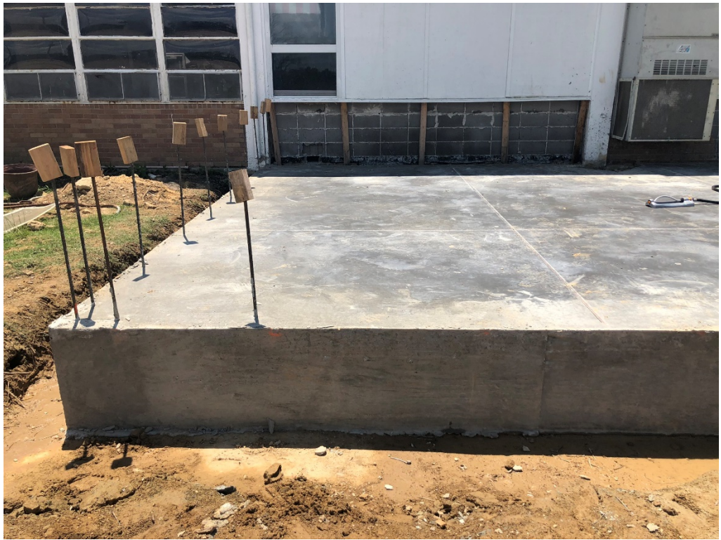
Figure 5 – Foundation Poured at Addition
