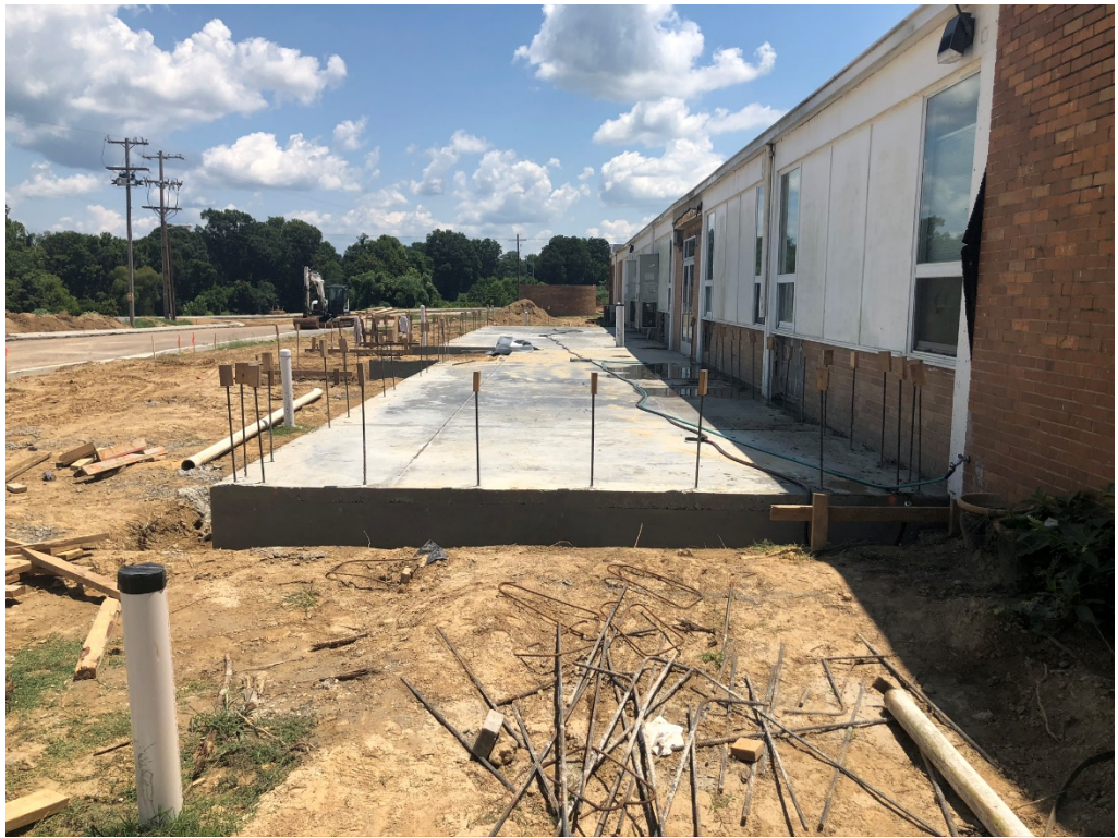
Figure 3 – Foundation Poured at Addition
