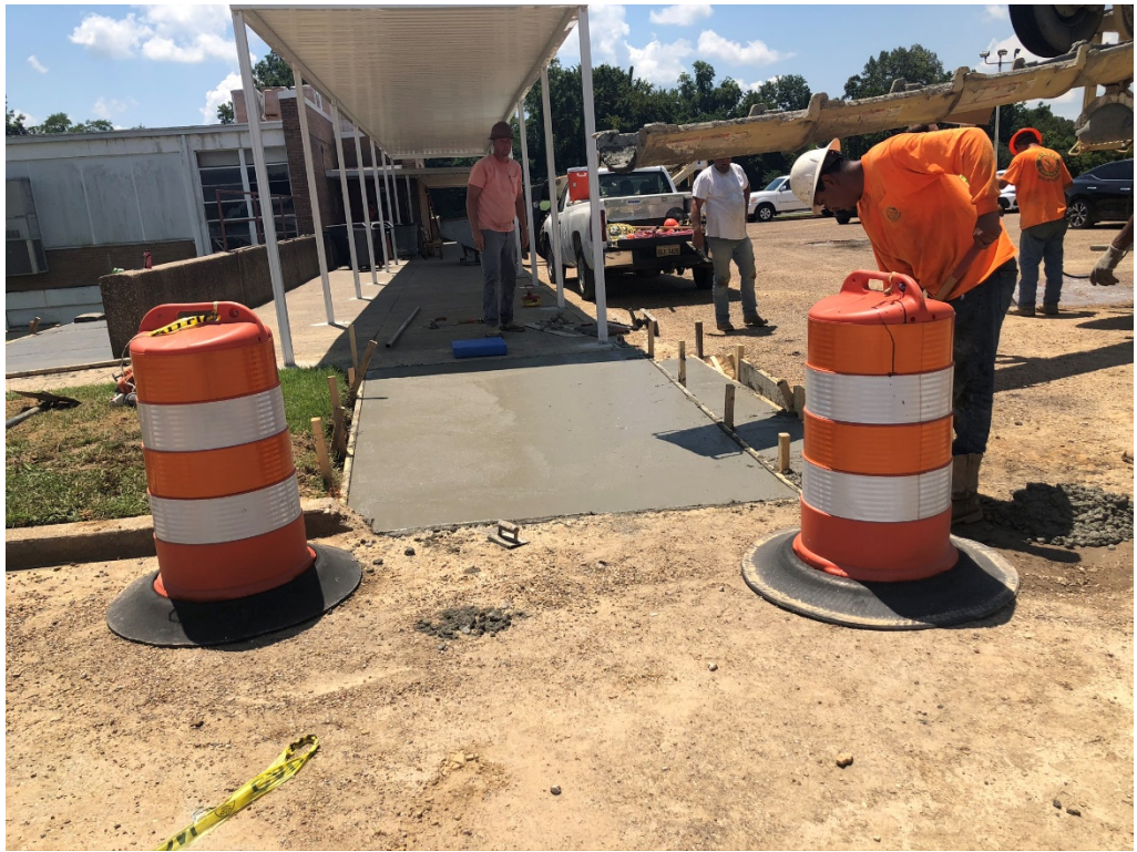
Figure 1 – Sidewalk Work at West Drop Off
