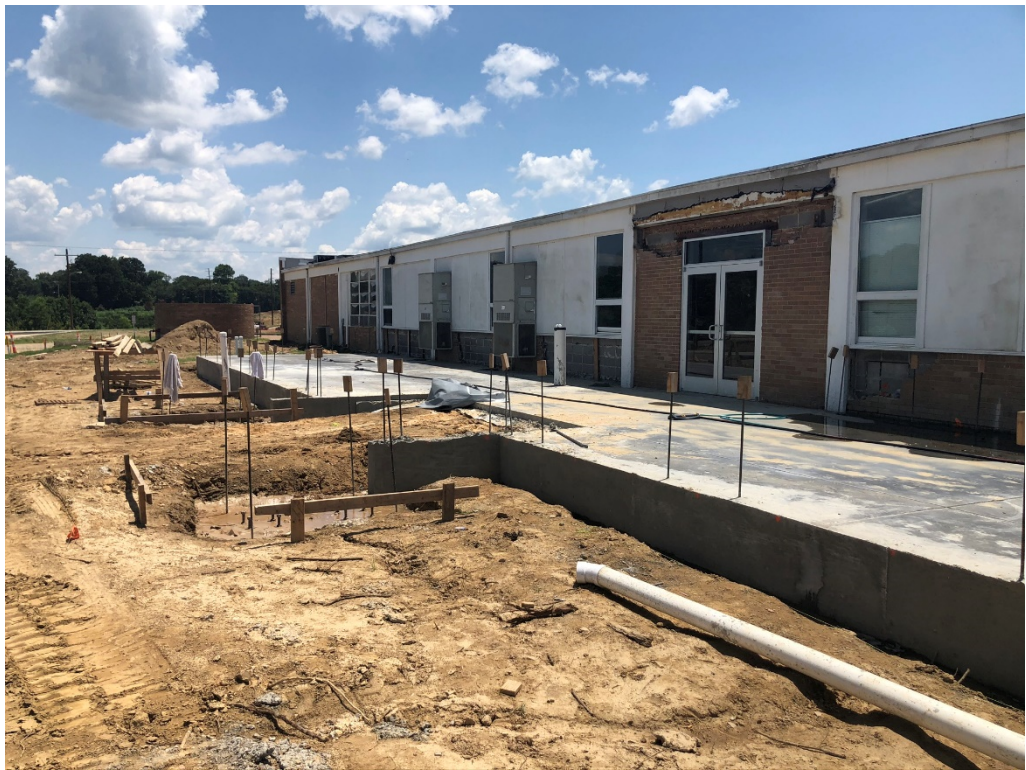
Figure 4 – Foundation Poured at Addition
