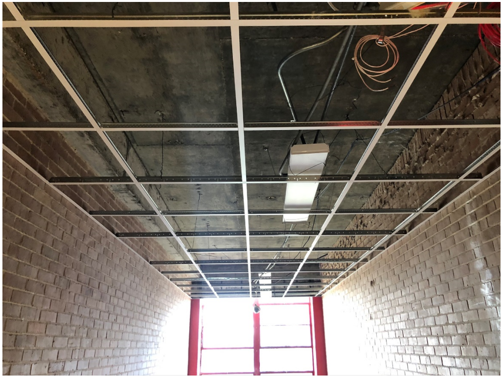
Figure 7 – Ceiling Grid at East hall 3 rd Floor
