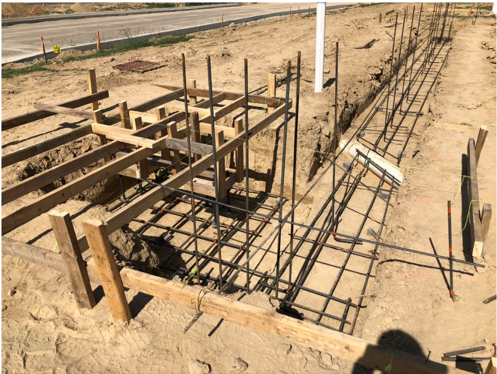
Figure 14 – Formed Grade Beam at Addition
