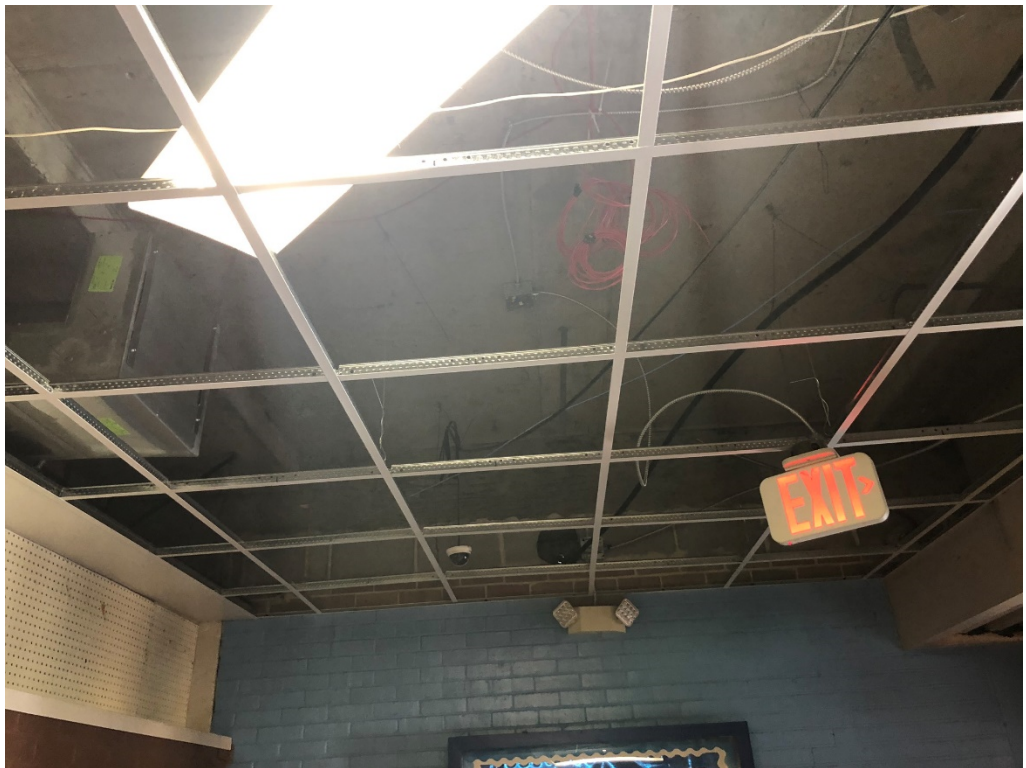
Figure 2 – Ceiling Grid at West hall 3 rd Floor
