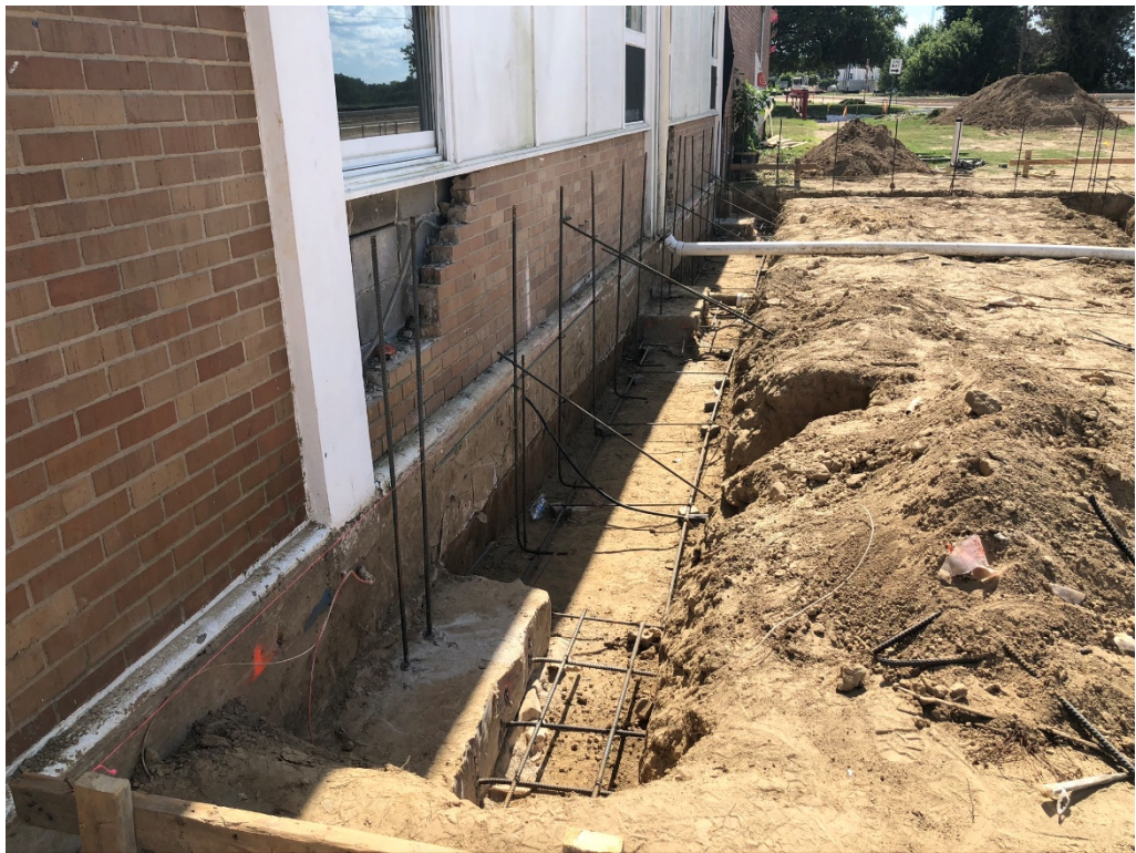
Figure 12 – Formed Grade Beam at Addition
