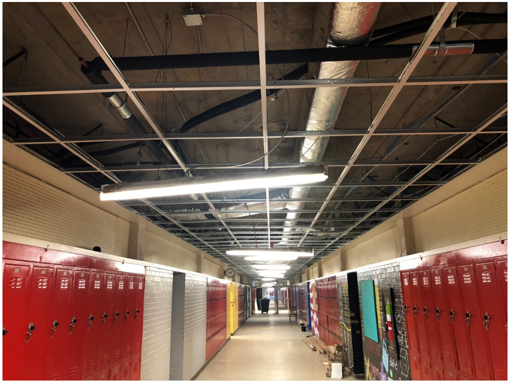
Figure 3 – Ceiling Grid at West hall 3 rd Floor
