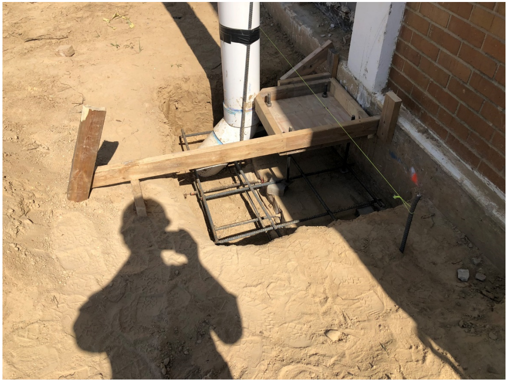
Figure 11 – Formed Spread Footing
