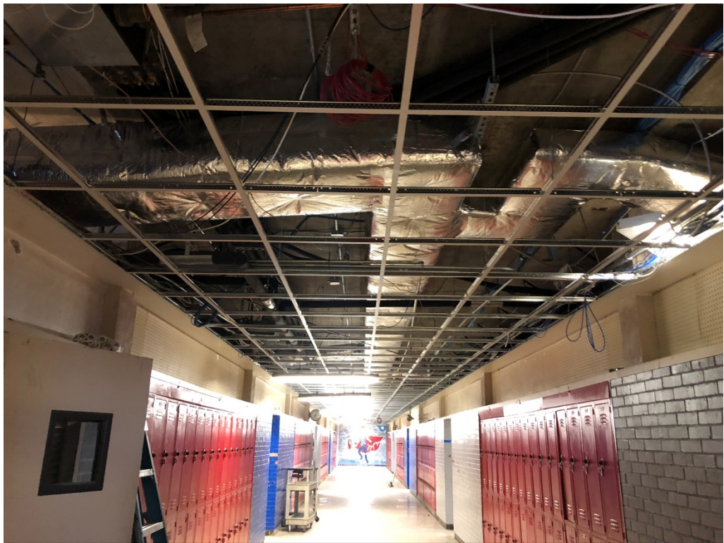
Figure 4 – Ceiling Grid at West hall 3 rd Floor
