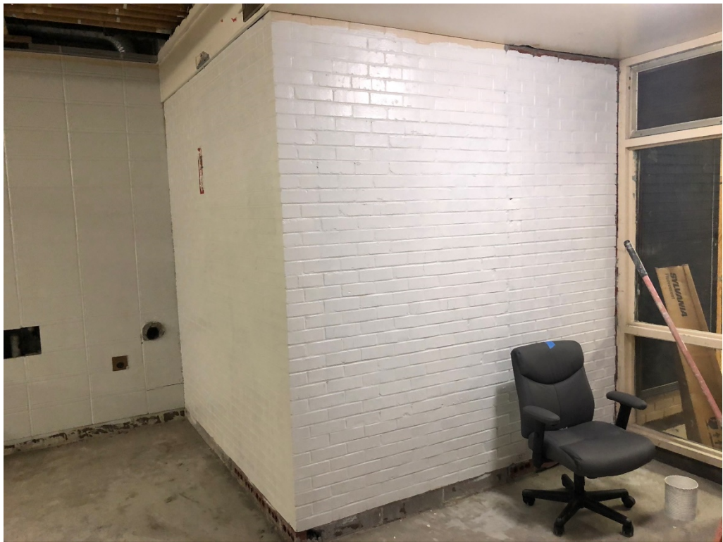
Figure 10 – 1 st Floor Bathroom and Painted Brick
