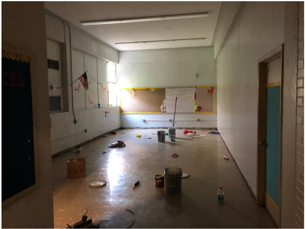
Figure 9 – 1 st Floor Paint Work Ongoing
