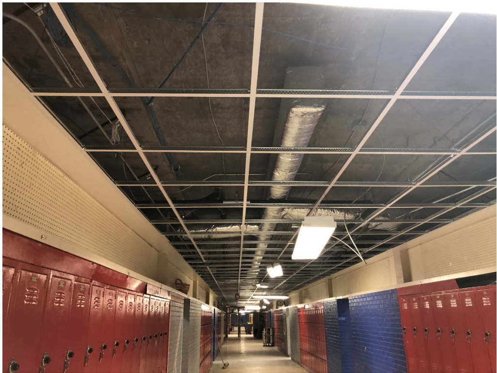
Figure 8 – Ceiling Grid at East hall 3 rd Floor
