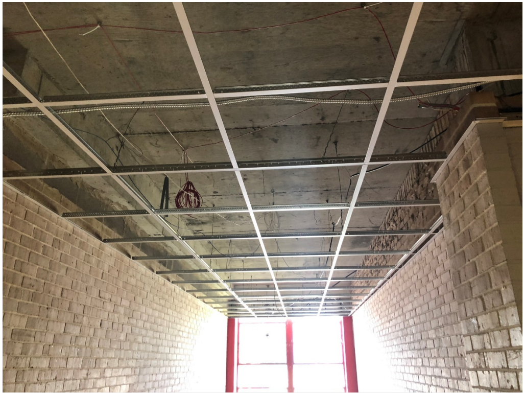
Figure 1 – Ceiling Grid at West hall 3 rd Floor
