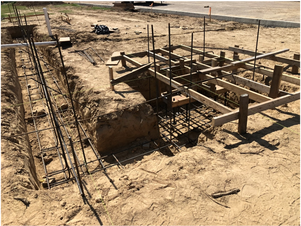
Figure 13 – Formed Grade Beam at Addition
