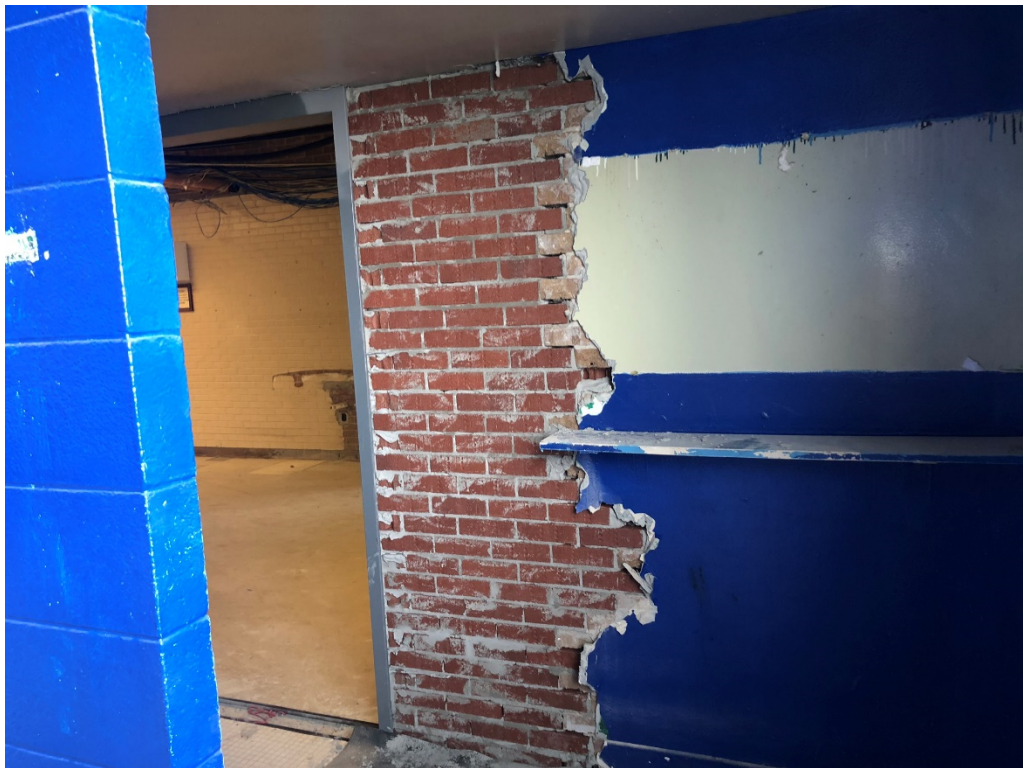
Figure 2 – Masonry Patch at Bathroom Interior 3 rd Floor
