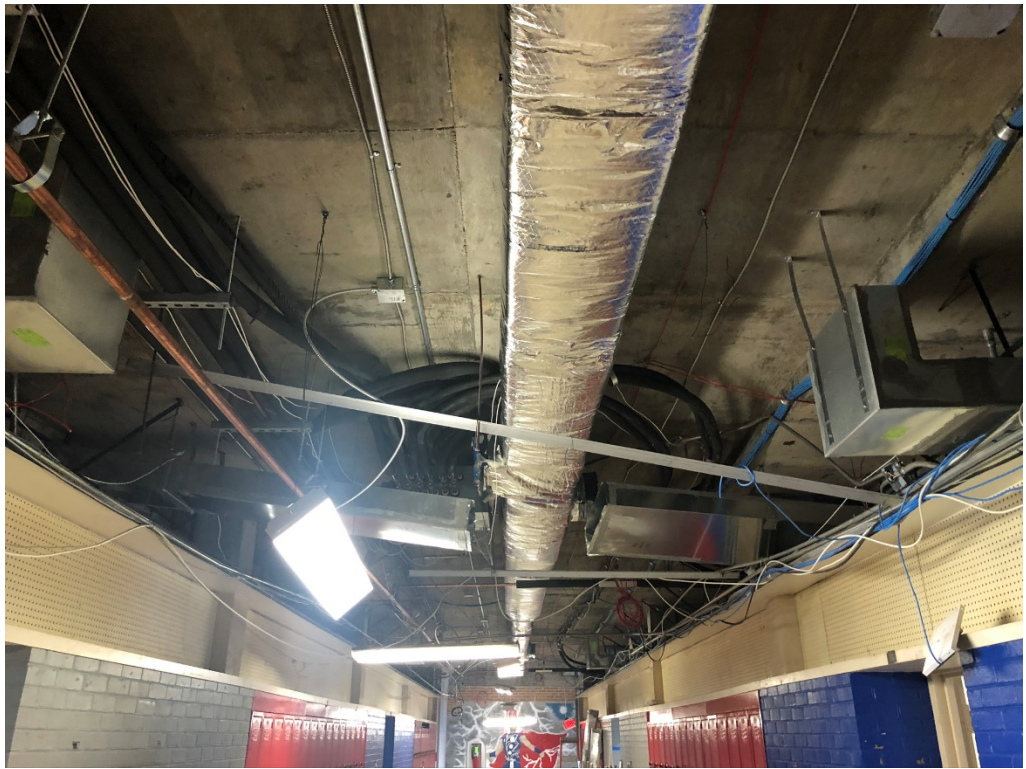
Figure 3 – Ductwork Insulated
