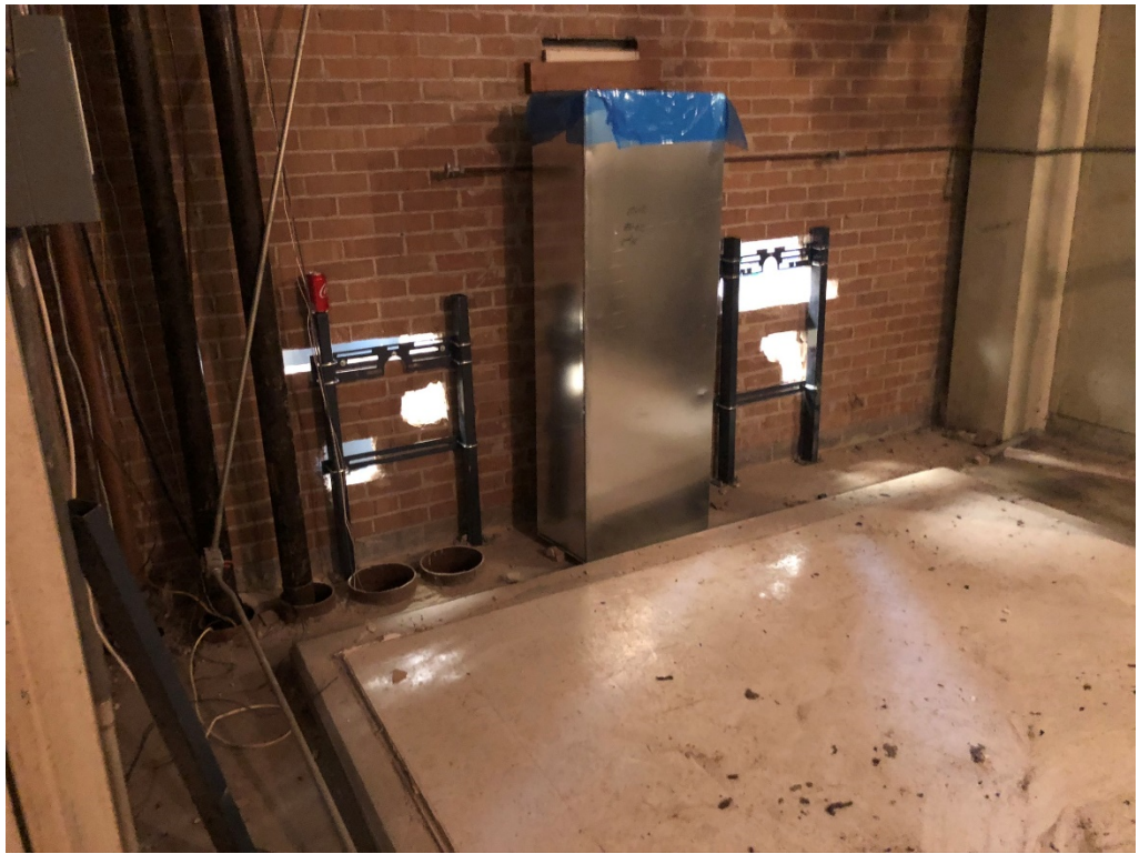
Figure 5 – EDF Carriers Installed
