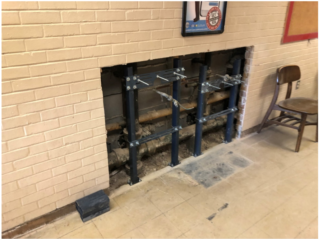
Figure 1 – EDF Carriers Installed
