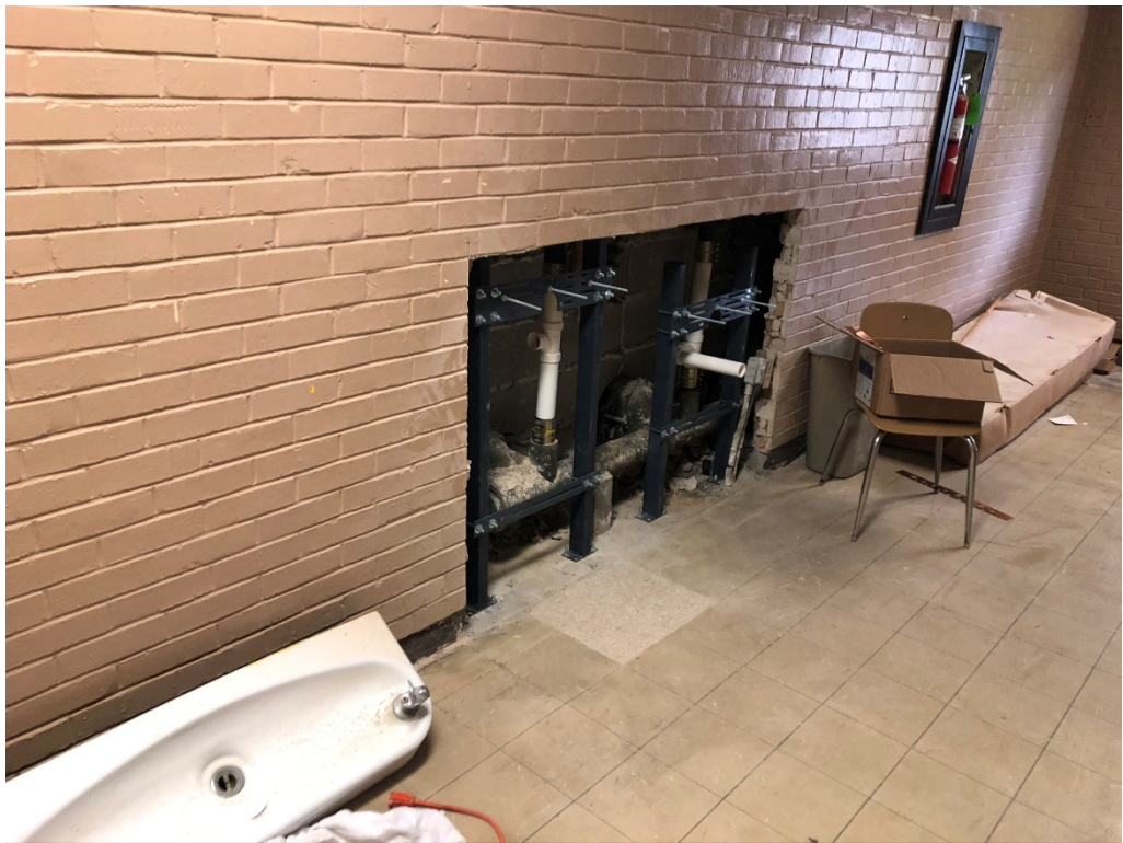
Figure 6 – EDF Carriers Installed
