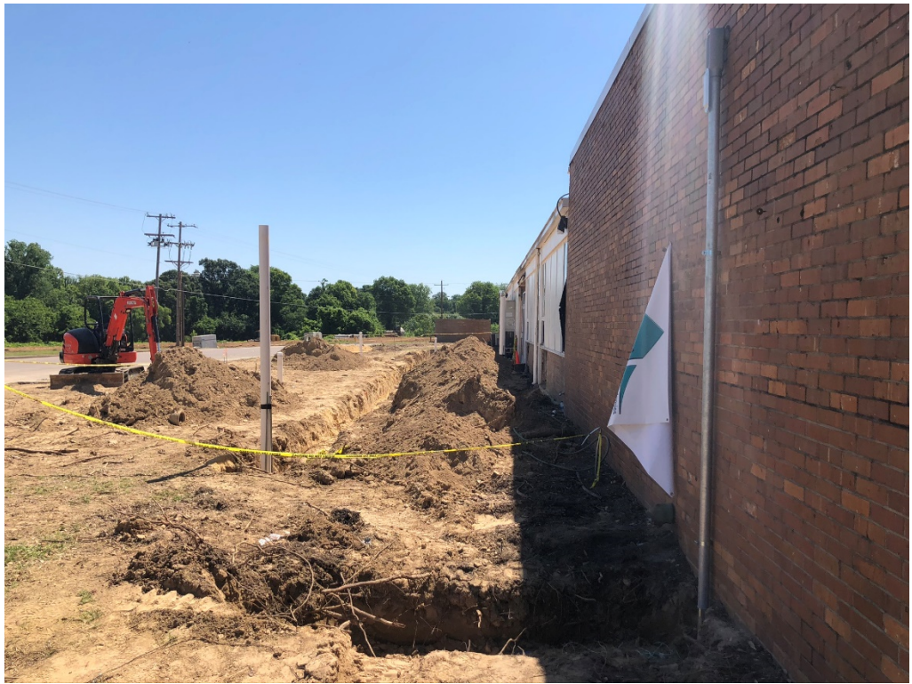
Figure 1 – Sewer work at Front Entry of Project in preparation for Addition
