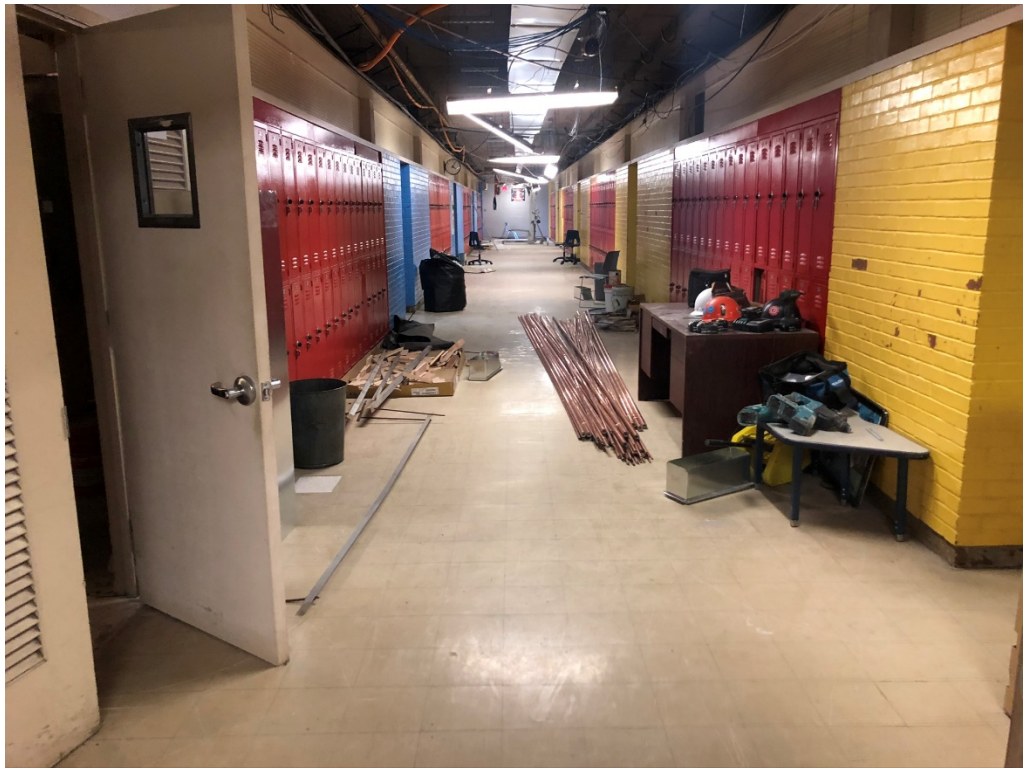
Figure 5 – Mechanical Rough In is Ongoing
