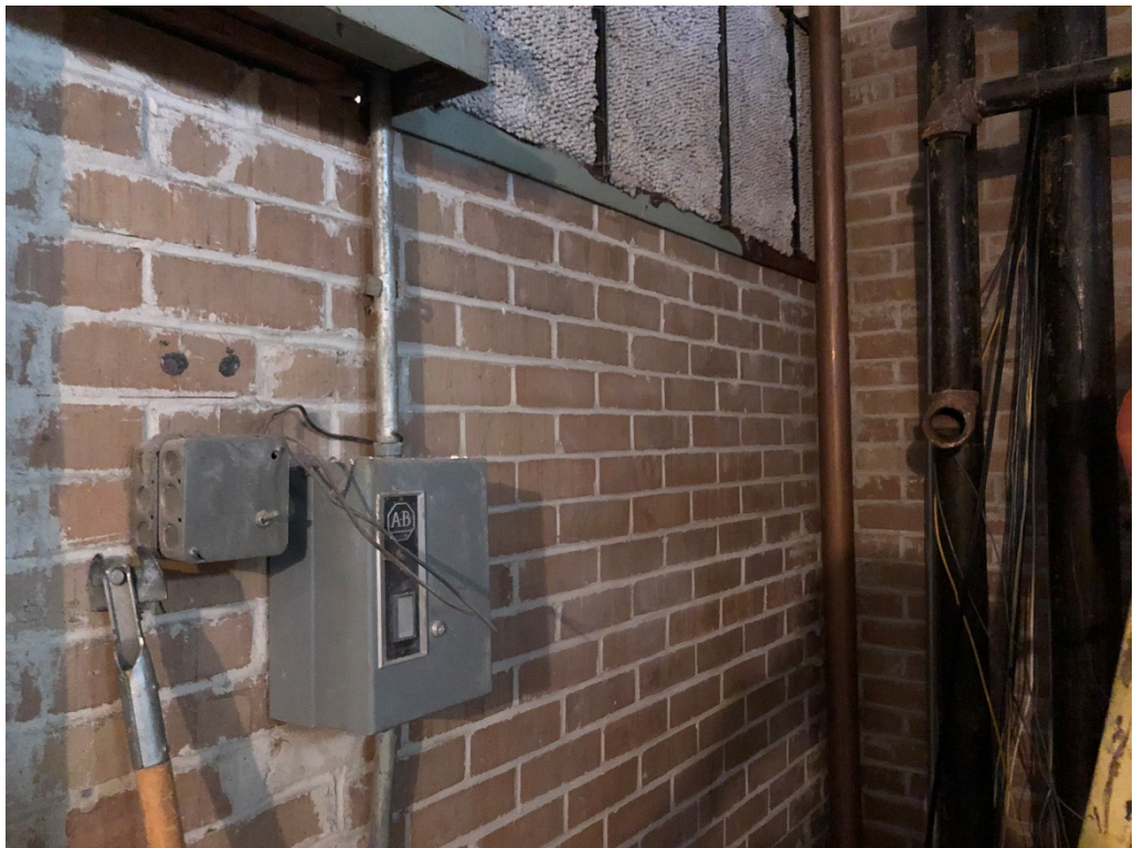
Figure 4 – Added Pipes has been demoed back @ Room E-323A
