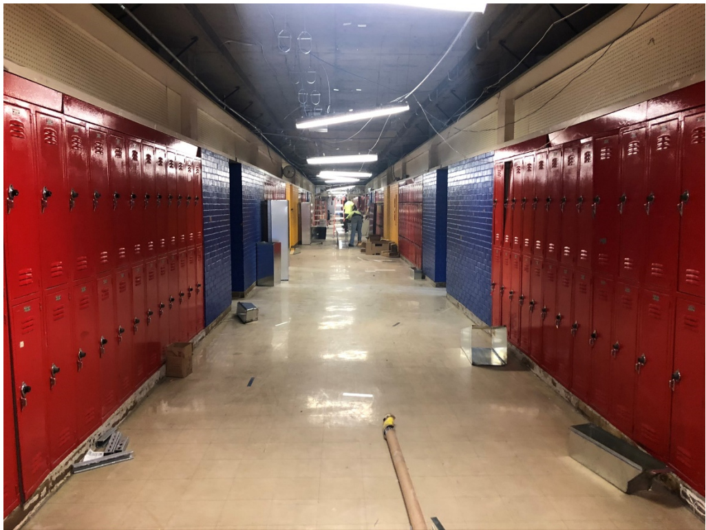
Figure 6 – Mechanical Rough In is Ongoing
