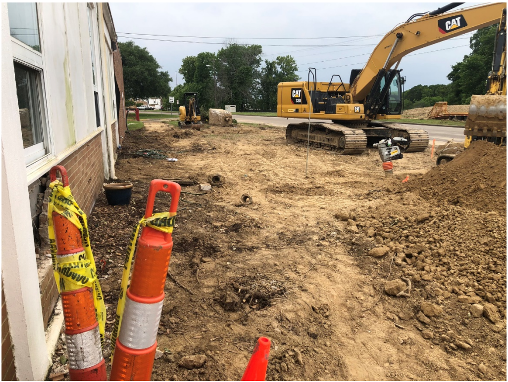
Figure 7 – Entry Addition Work Ongoing
