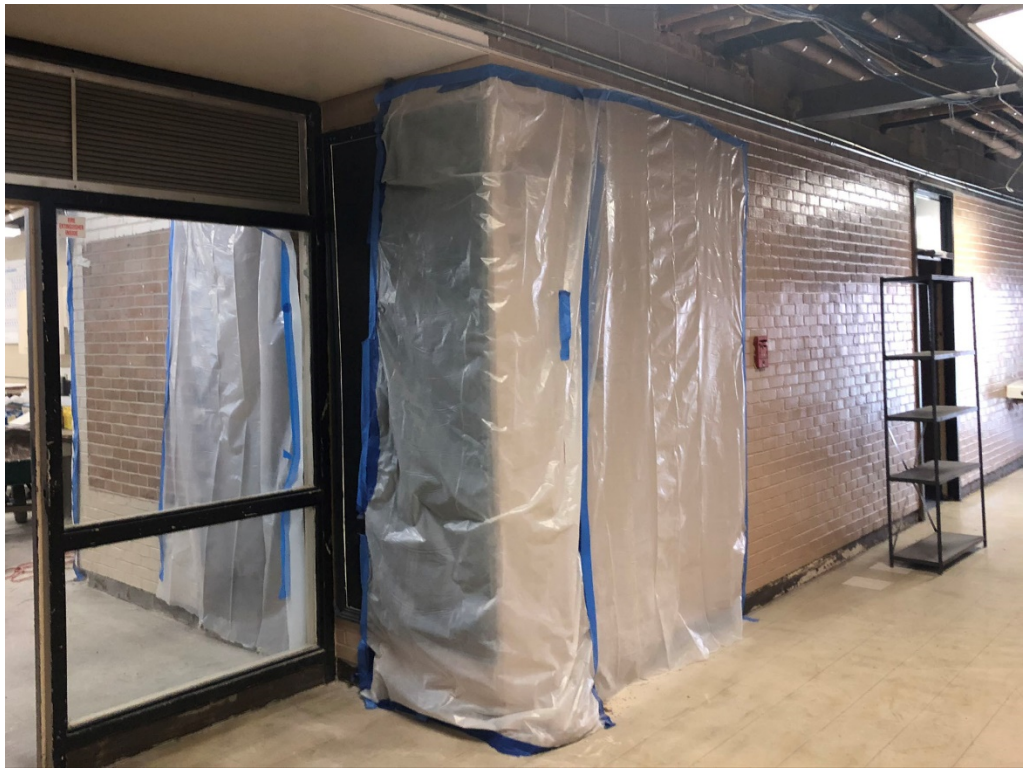
Figure 5 – Demo at lower floor Brick Wall Begun
