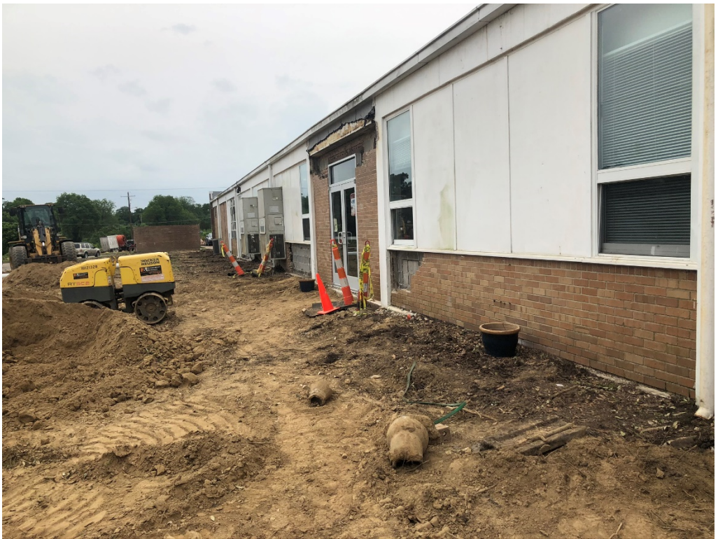
Figure 8 – Entry Addition Work Ongoing
