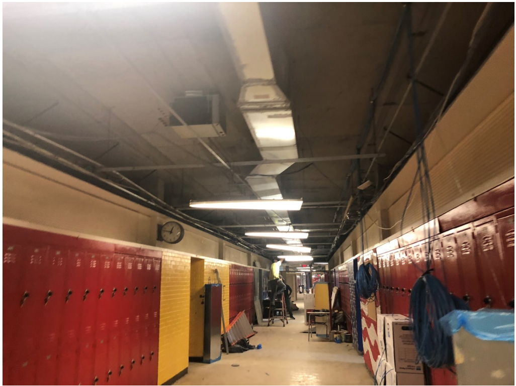
Figure 3 – Duct Runs installed at upper floor
