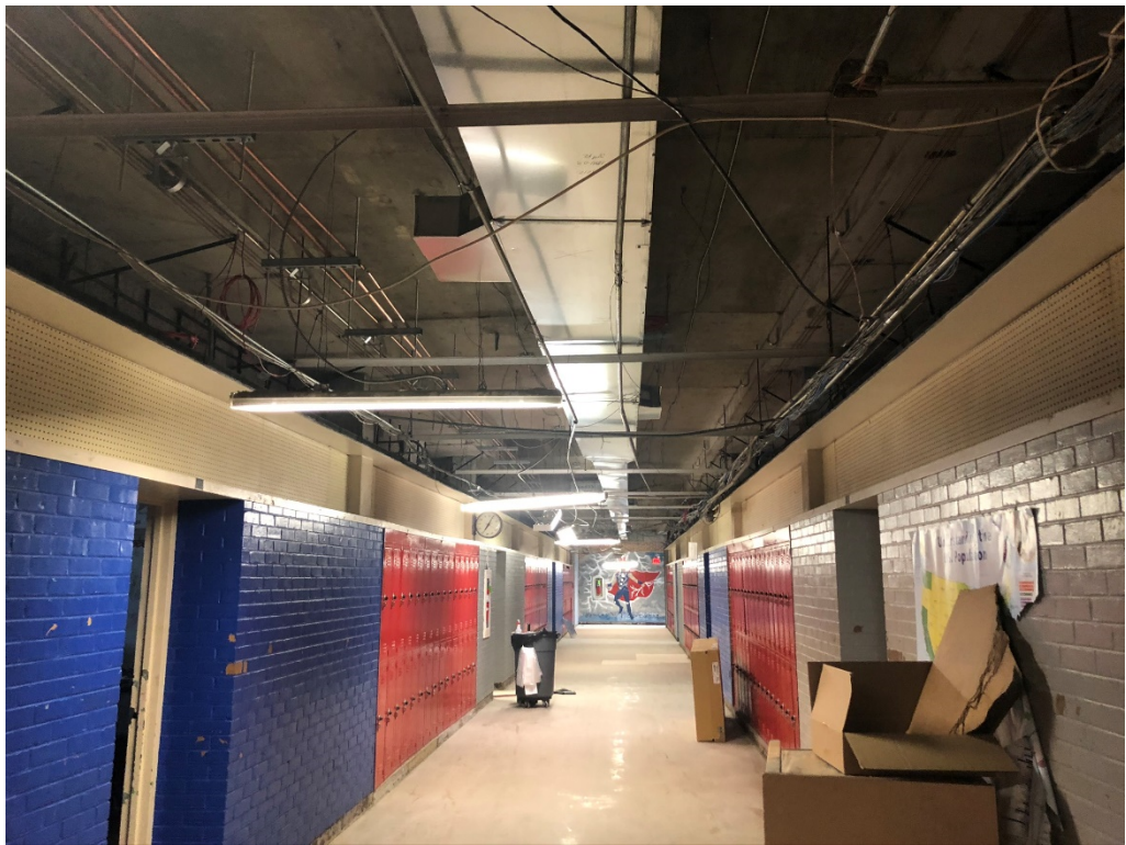
Figure 4 – Duct Runs installed at upper floor
