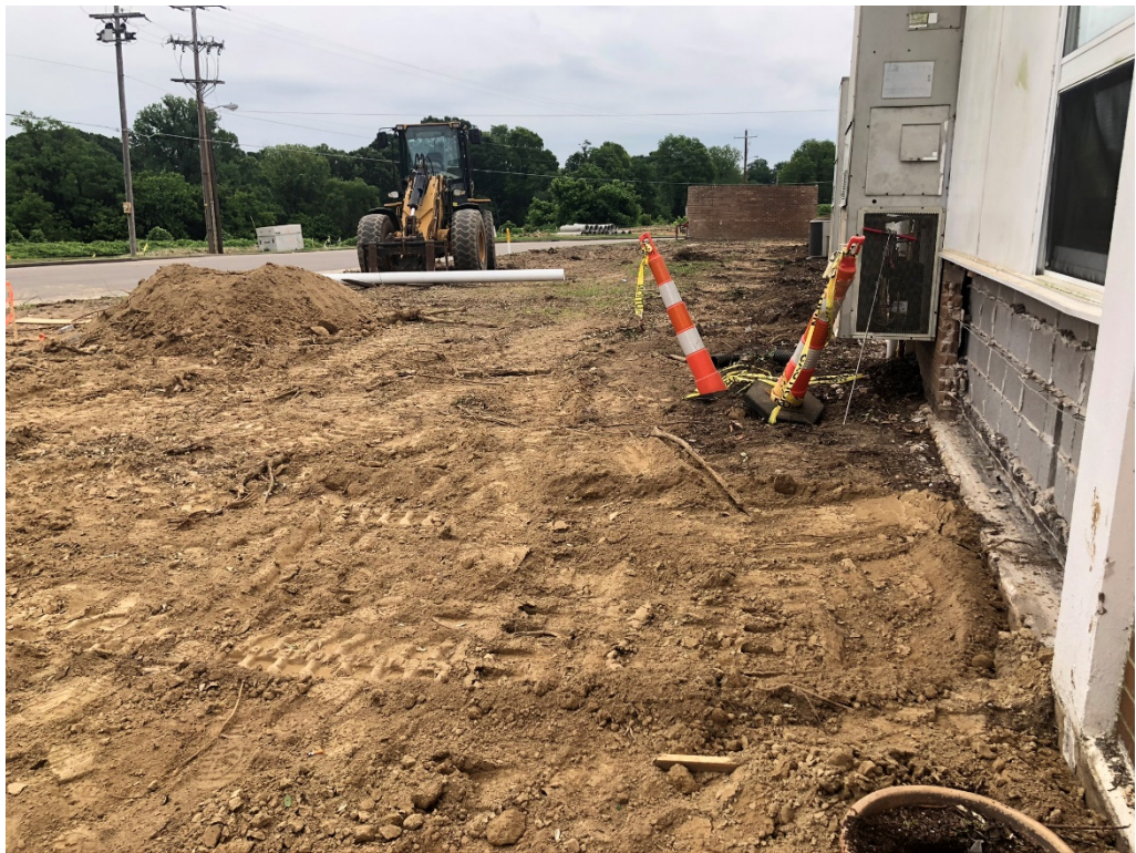
Figure 6 – Entry Addition Work Ongoing
