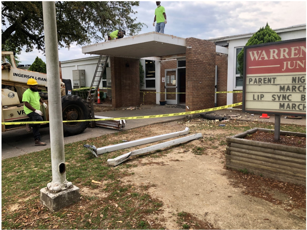
Figure 1 – School Entry Demo Begun
