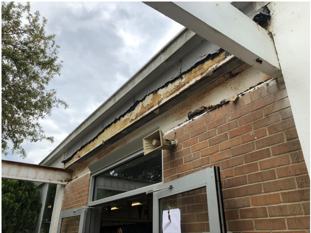
Figure 2 – Connection of Entry Awning to School
