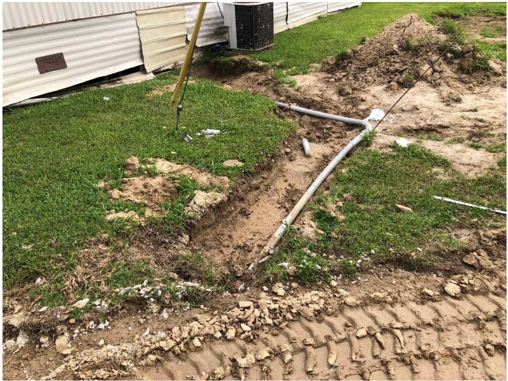
Figure 7 – Underground Electrical Exposed in Shallow Trench
