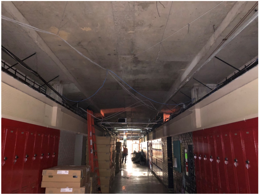
Figure 9 – Ceiling Demo and at East 3 rd Floor Hall
