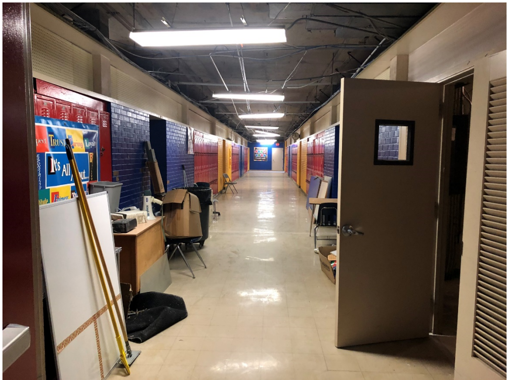
Figure 10 – Ceiling Demo and at West 3 rd Floor Hall
