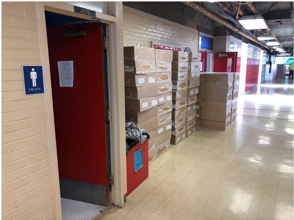
Figure 4 – Ceiling Tile Stored in Hall @ 3 rd Floor
