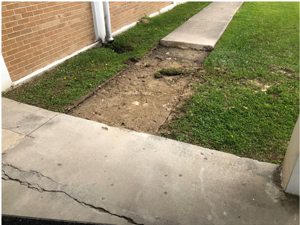
Figure 6 – Concrete cut and removed at 1 st floor breezeway
