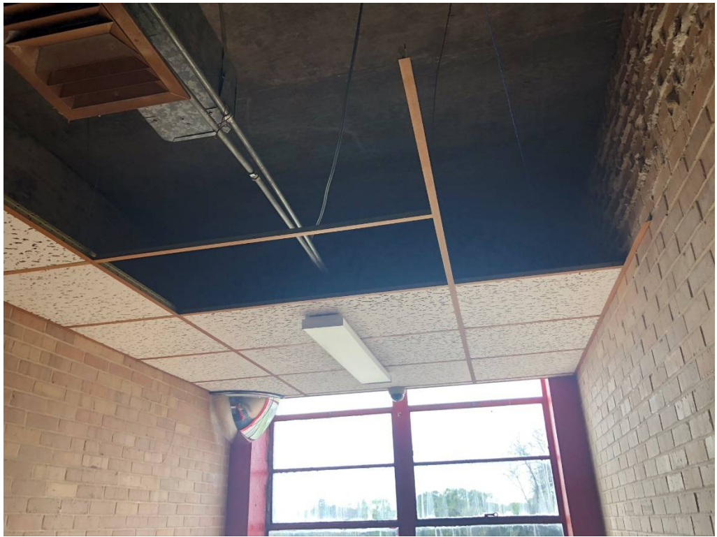
Figure 3 – West Wing 3 rd Floor Ceiling Demo Remaining
