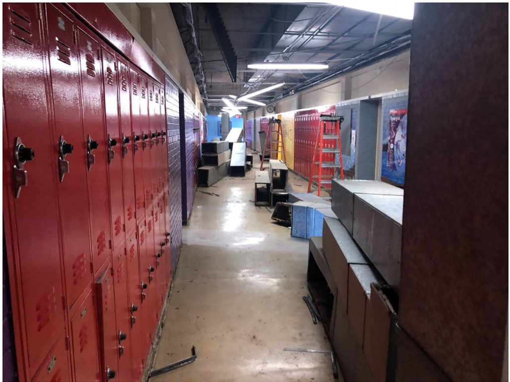
Figure 2 – West Wing 3 rd Floor HVAC Demo
