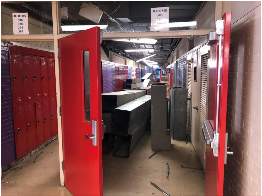
Figure 1 – West Wing 3 rd Floor HVAC Demo
