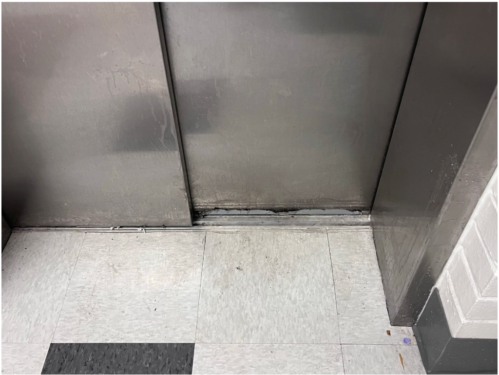
Figure 9 – Protective Film Never Removed
