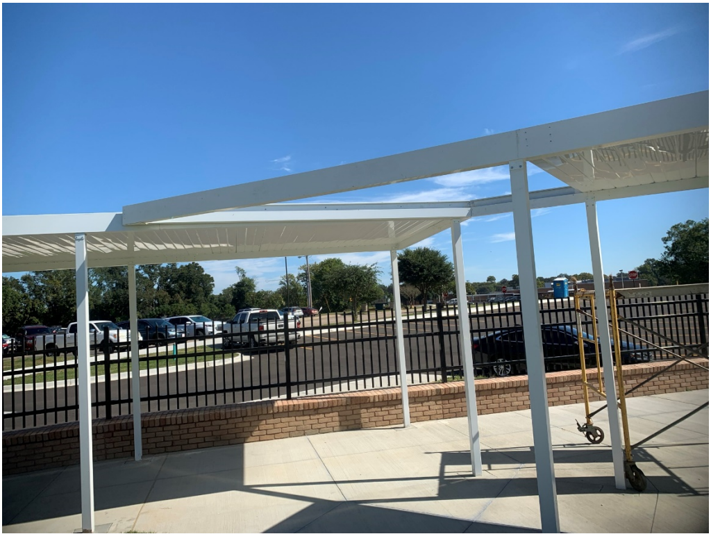
Figure 51 – Finish Awning Install
