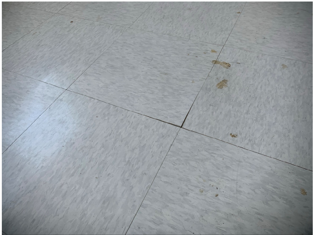
Figure 48 – Floor tile raised in admin area
