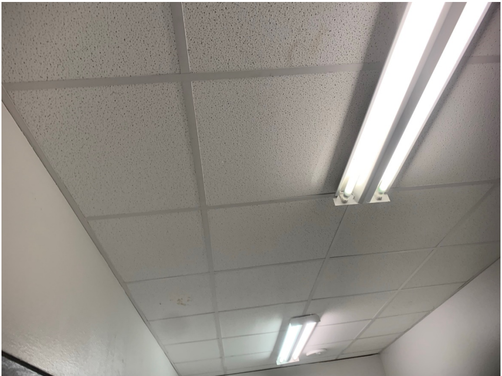
Figure 40 – Clean/replace ceiling tile @ E-111
