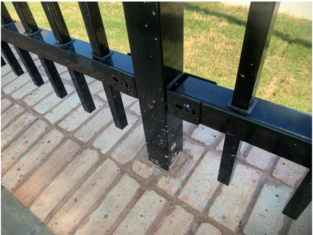
Figure 52 – Clean new fence and paint where scuffed
