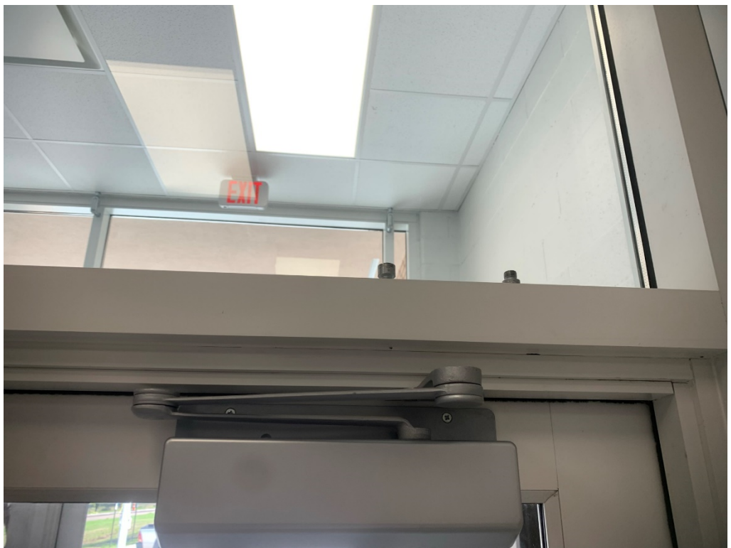
Figure 26 – Remove construction materials
