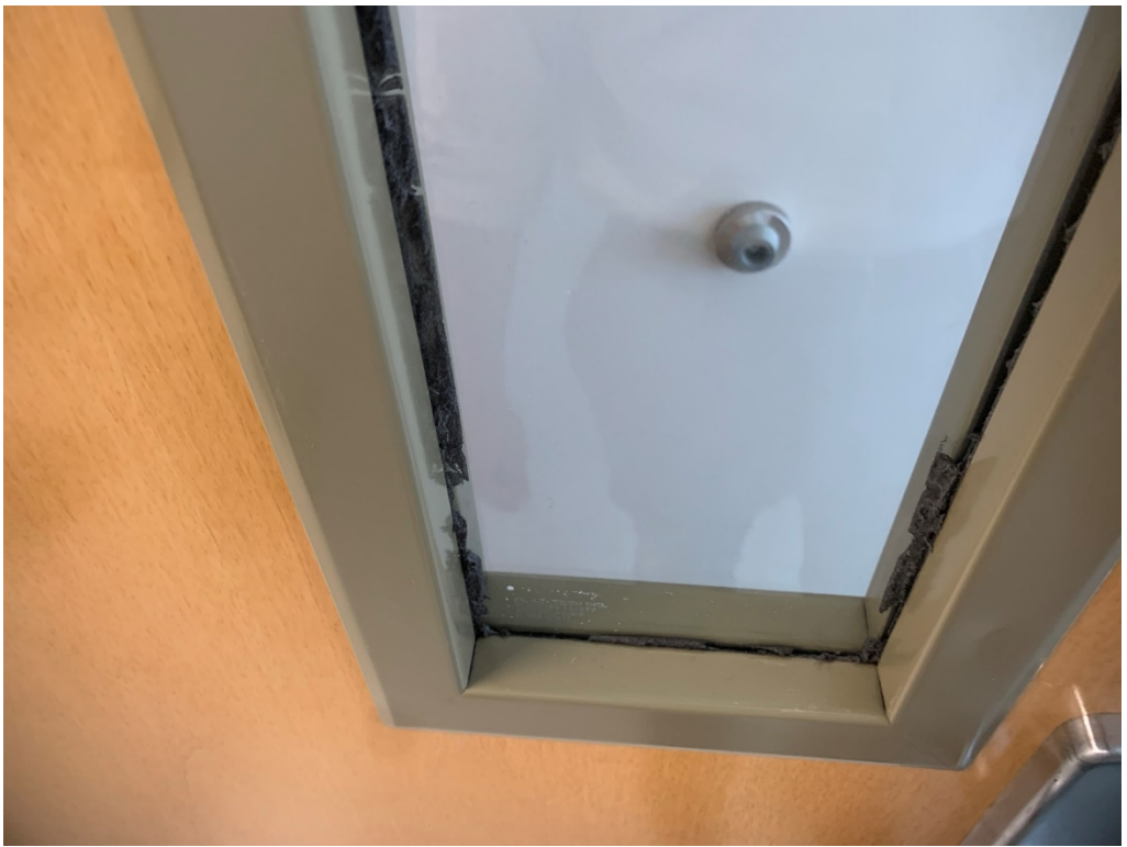
Figure 14 – Clean up edges where foam is tattered at glass installation
