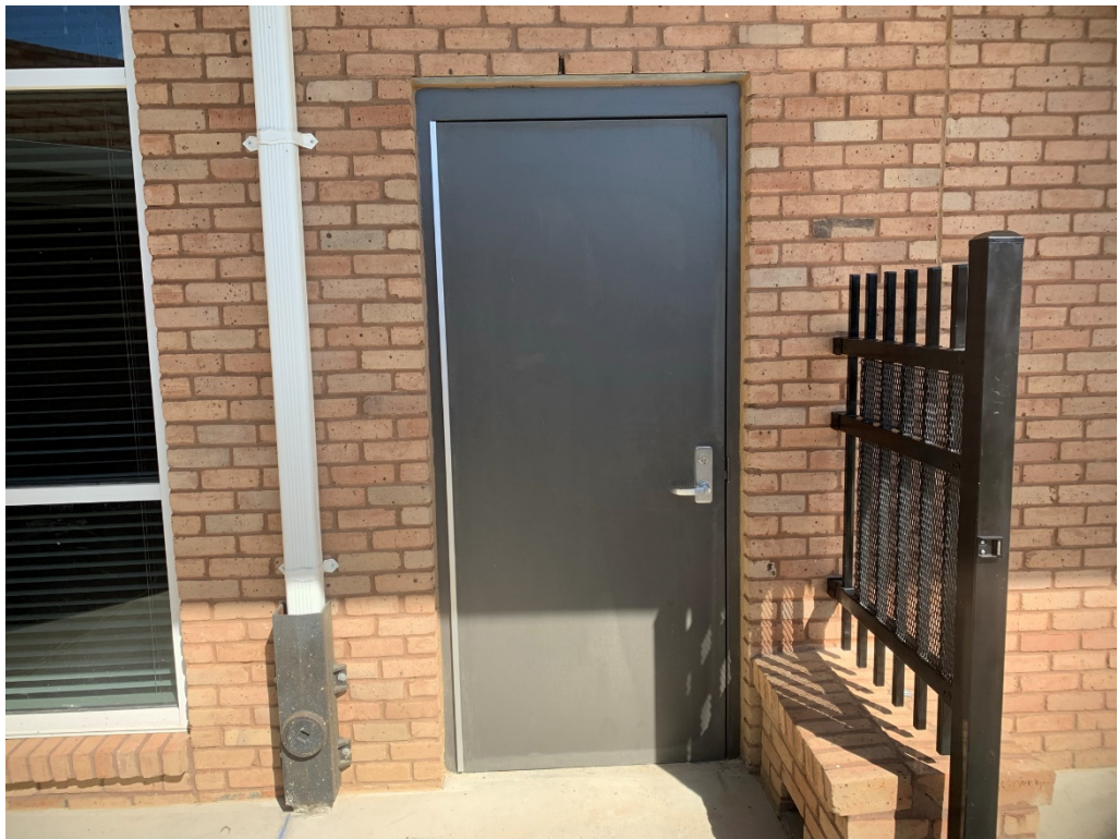
Figure 54 – Finish Painting Door Panel & Jamb
