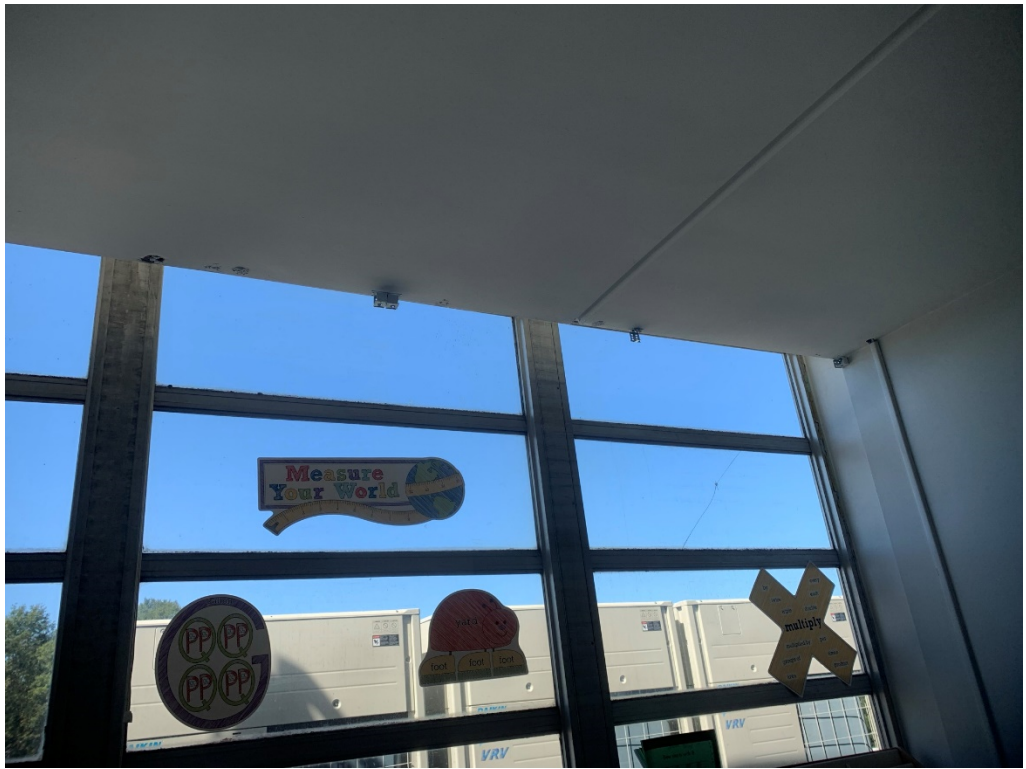
Figure 49 – Blinds still to be installed
