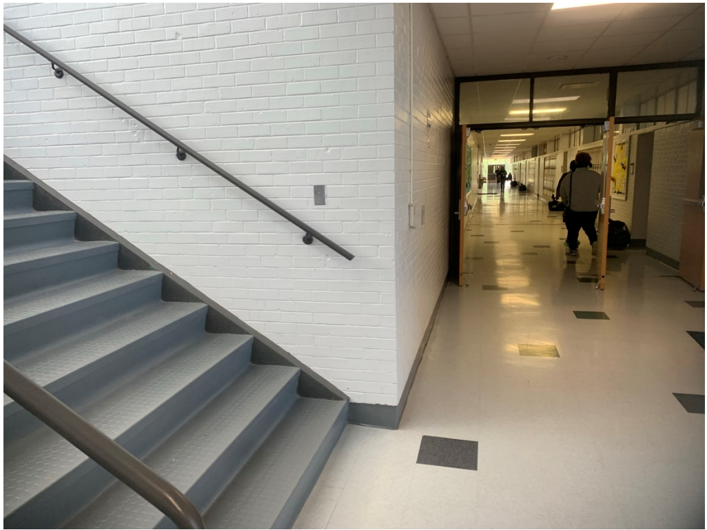
Figure 45 – Handrail does not extend 12" past last step
