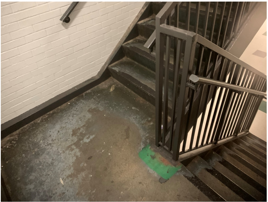
Figure 42 – Handrails do neither return to wall or are continuous per drawings
