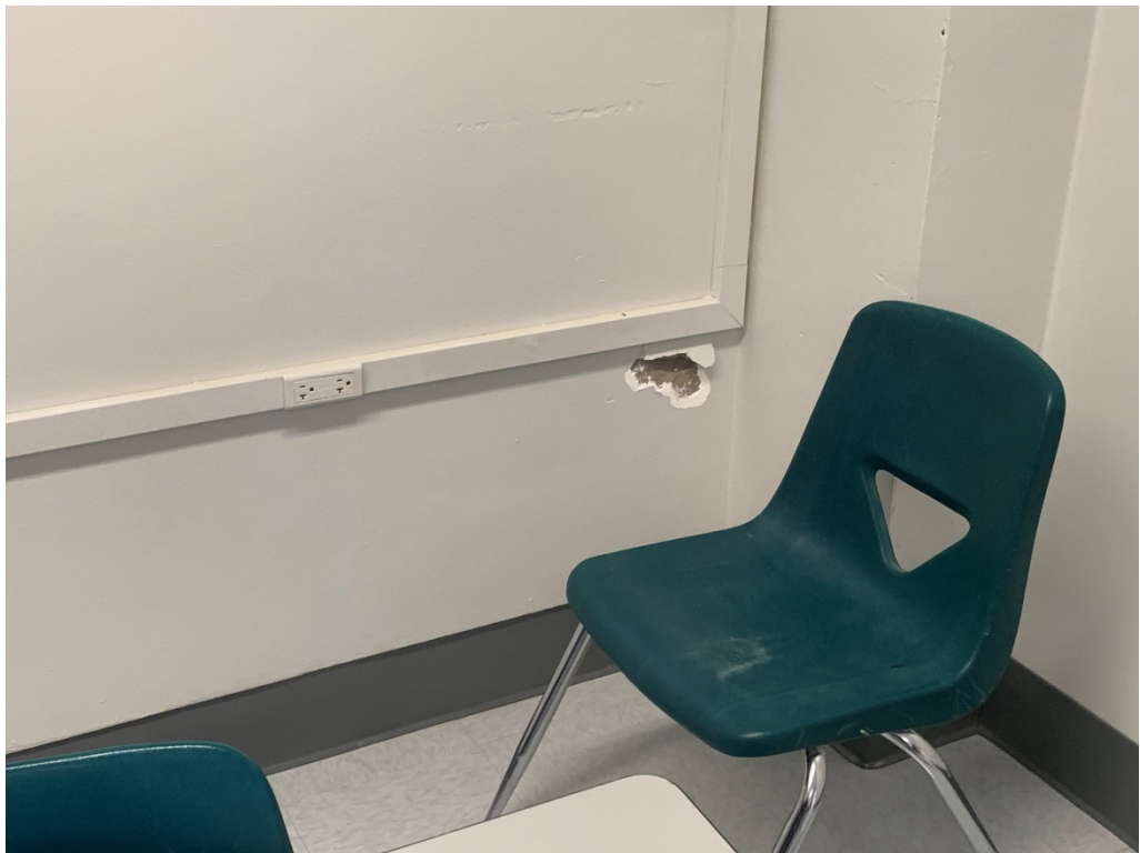
Figure 50 – Patch needed at E-308
