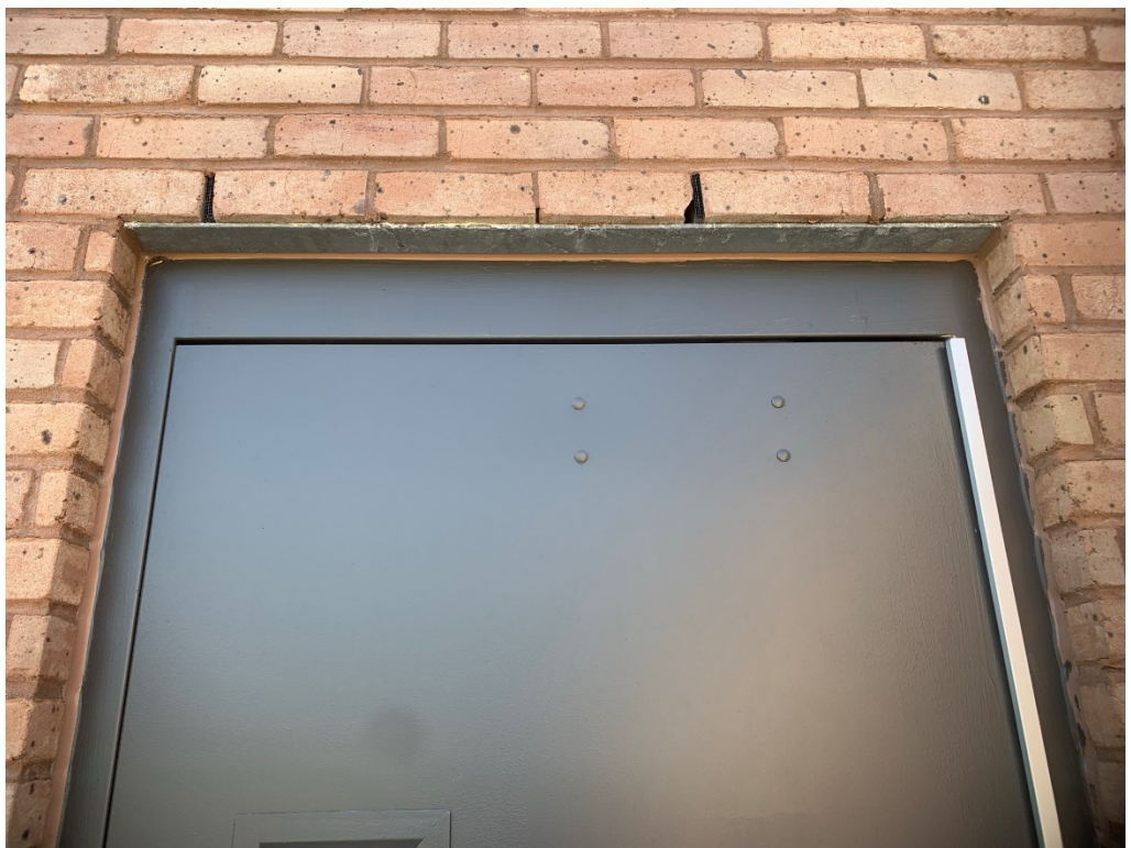
Figure 4 – Upper jamb still showing steaking
