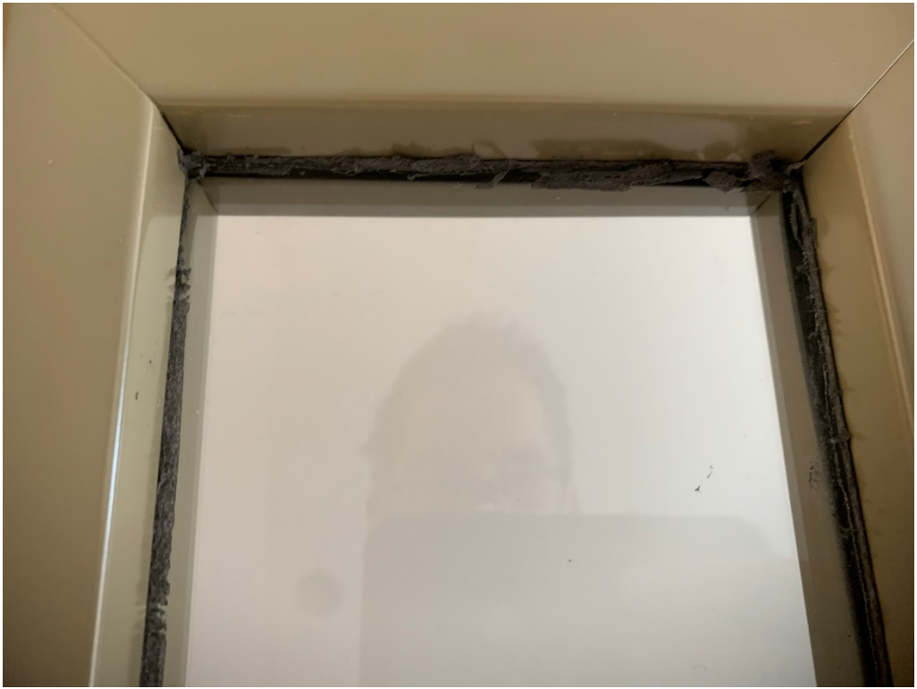
Figure 15 – Clean up edges where foam is tattered at glass installation
