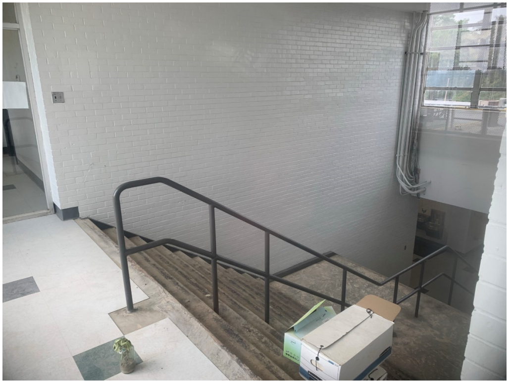
Figure 4 – Central handrail Installed
