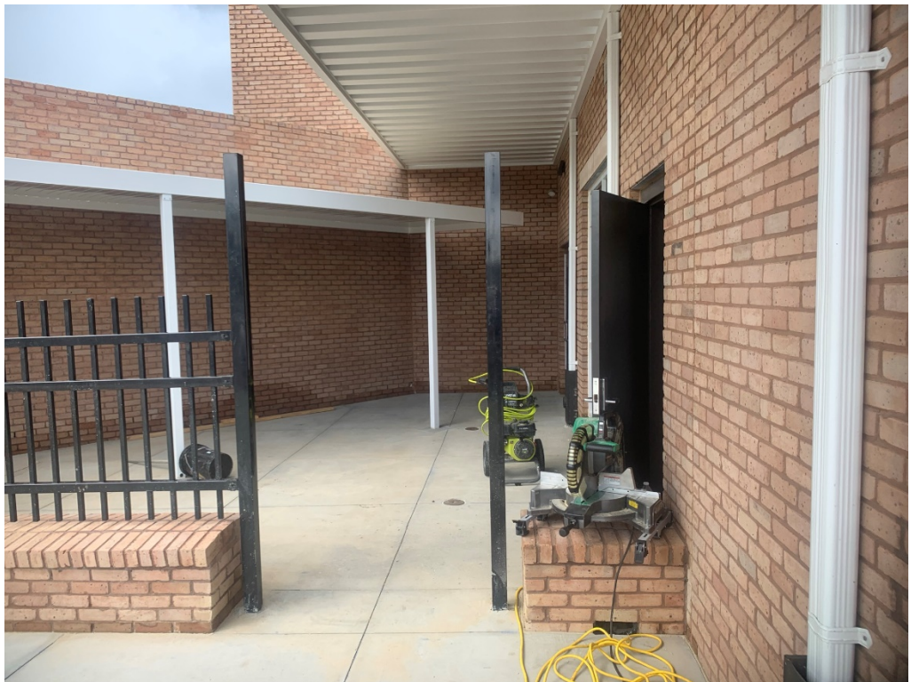
Figure 2 – Fence work is Ongoing
