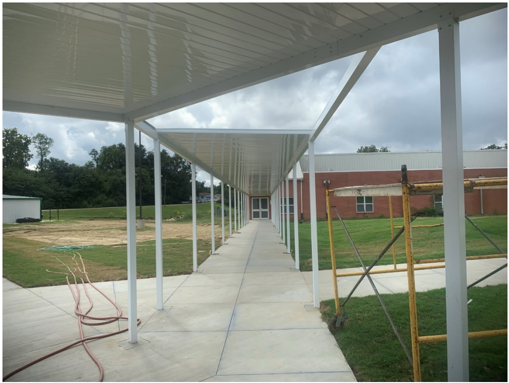
Figure 3 – Awning is Ongoing
