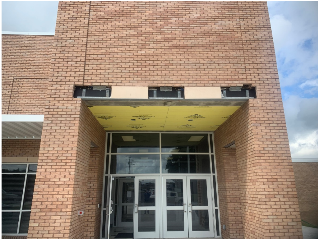
Figure 1 – Partial Lintel Removed for Correction
