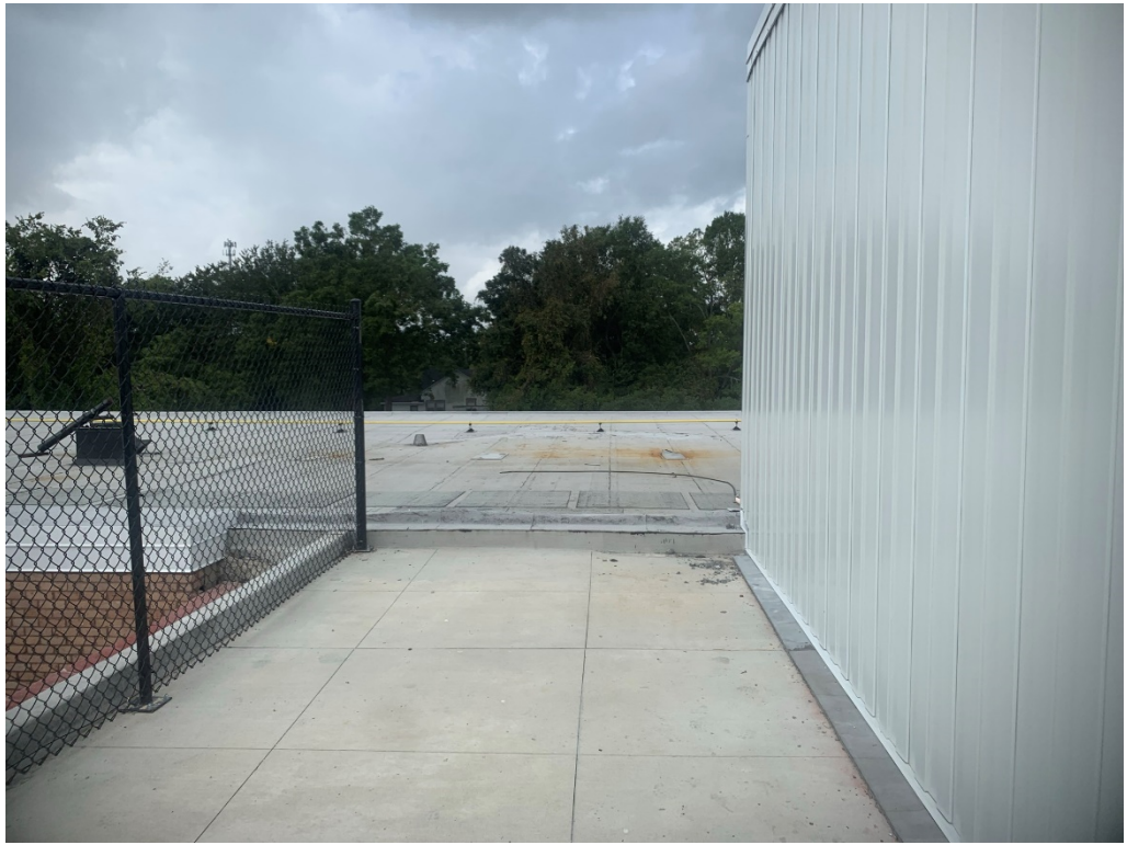
Figure 5 – Fence work is Ongoing
