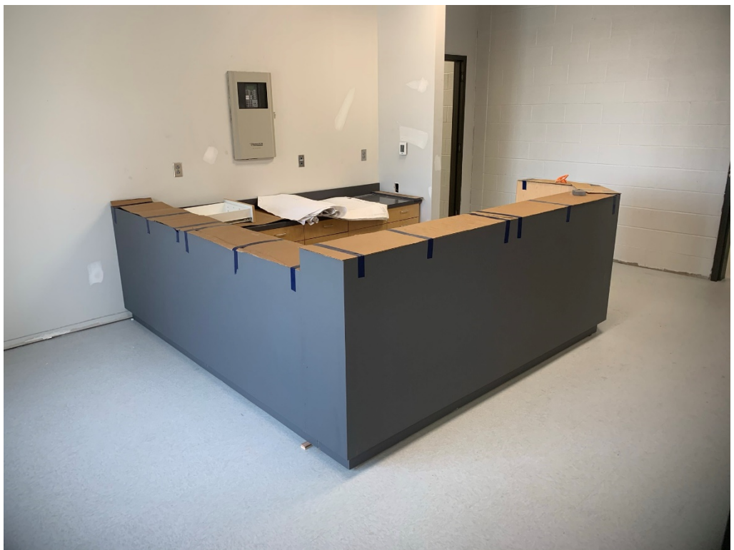
Figure 4 – New Millwork Installed
