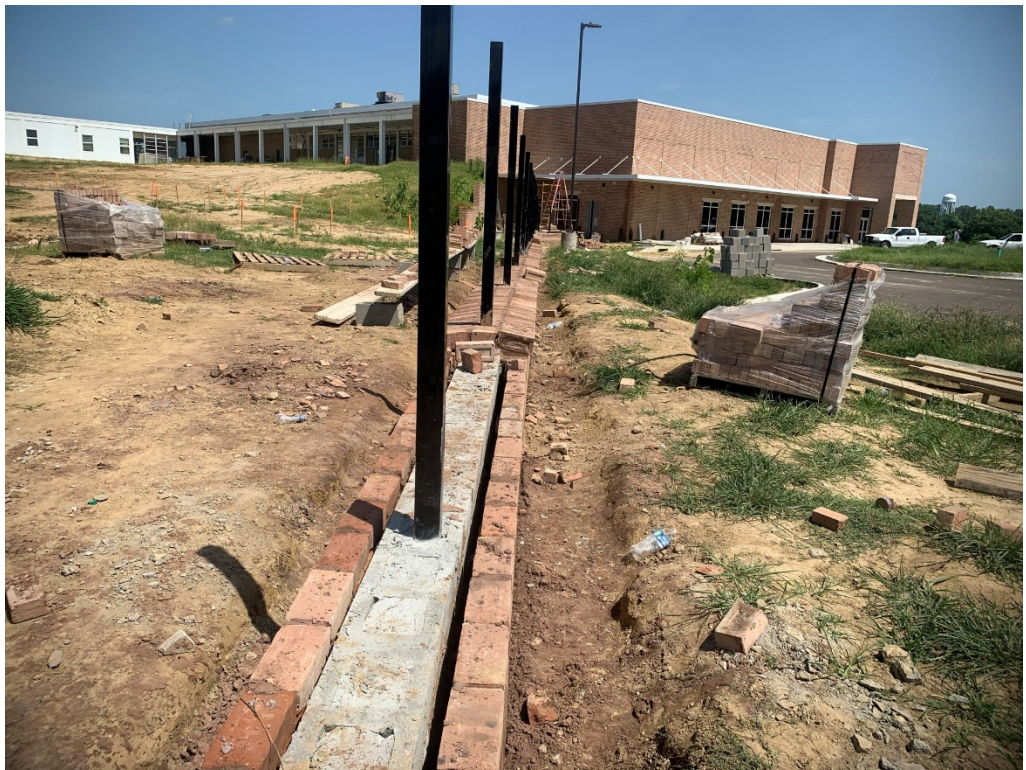
Figure 2 – Masonry is Ongoing
