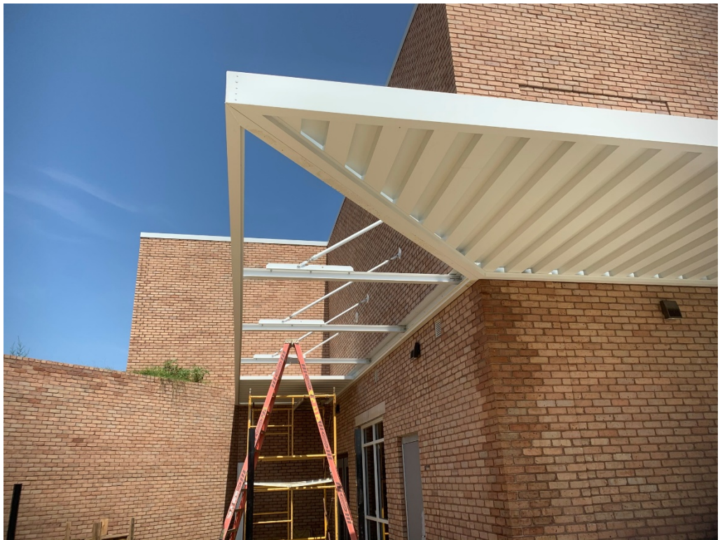
Figure 3 – Awning Installation is Ongoing
