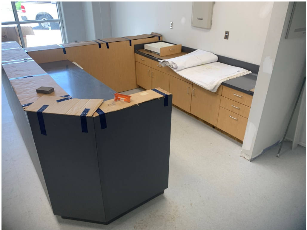
Figure 5 – New Millwork Installed
