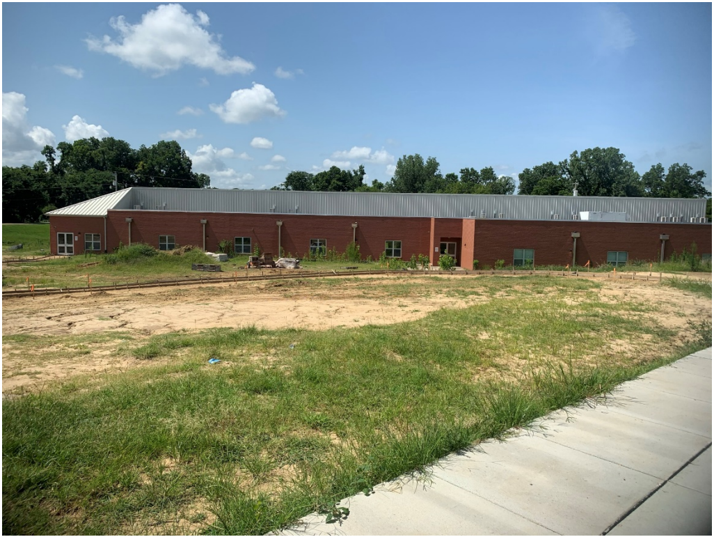
Figure 9 – Site Work is Ongoing
