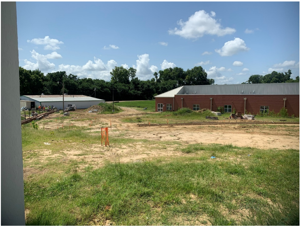
Figure 10 – Site Work is Ongoing
