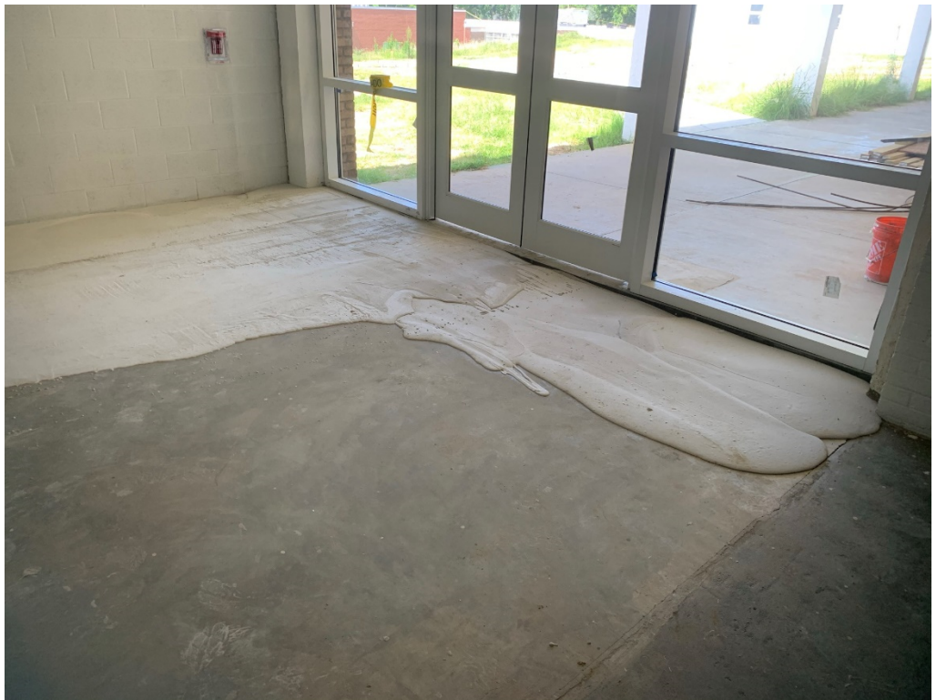
Figure 8 – Leveling at Up Floor in Ongoing for new Storefront Entrance
