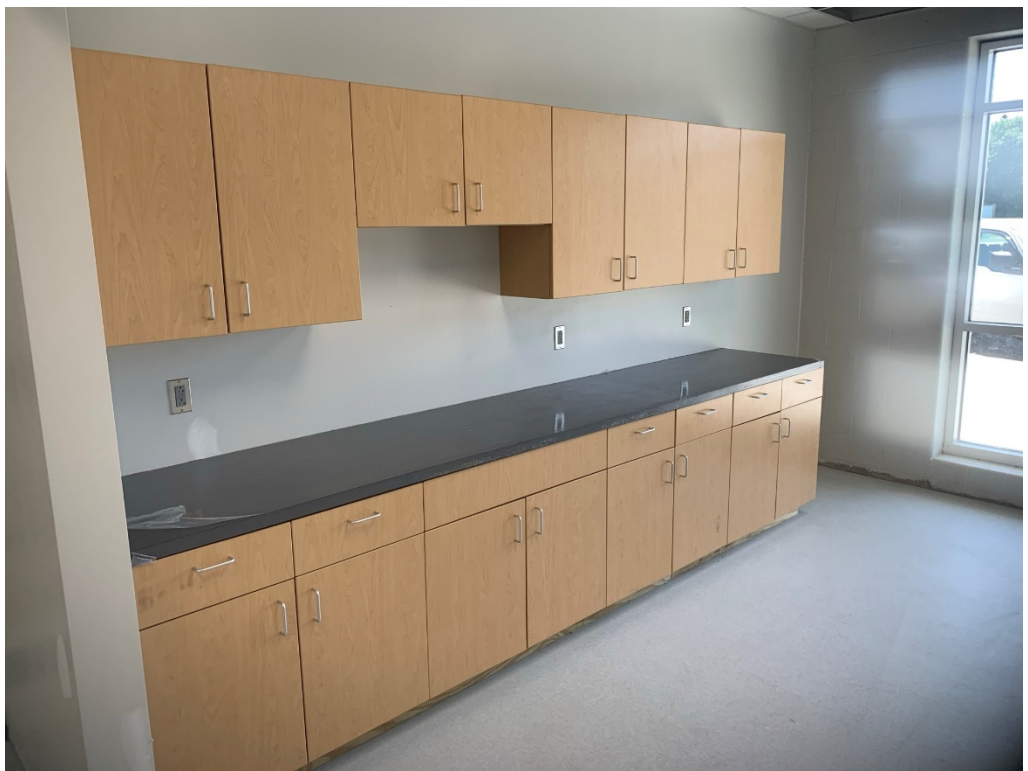
Figure 6 – New Millwork Installed
