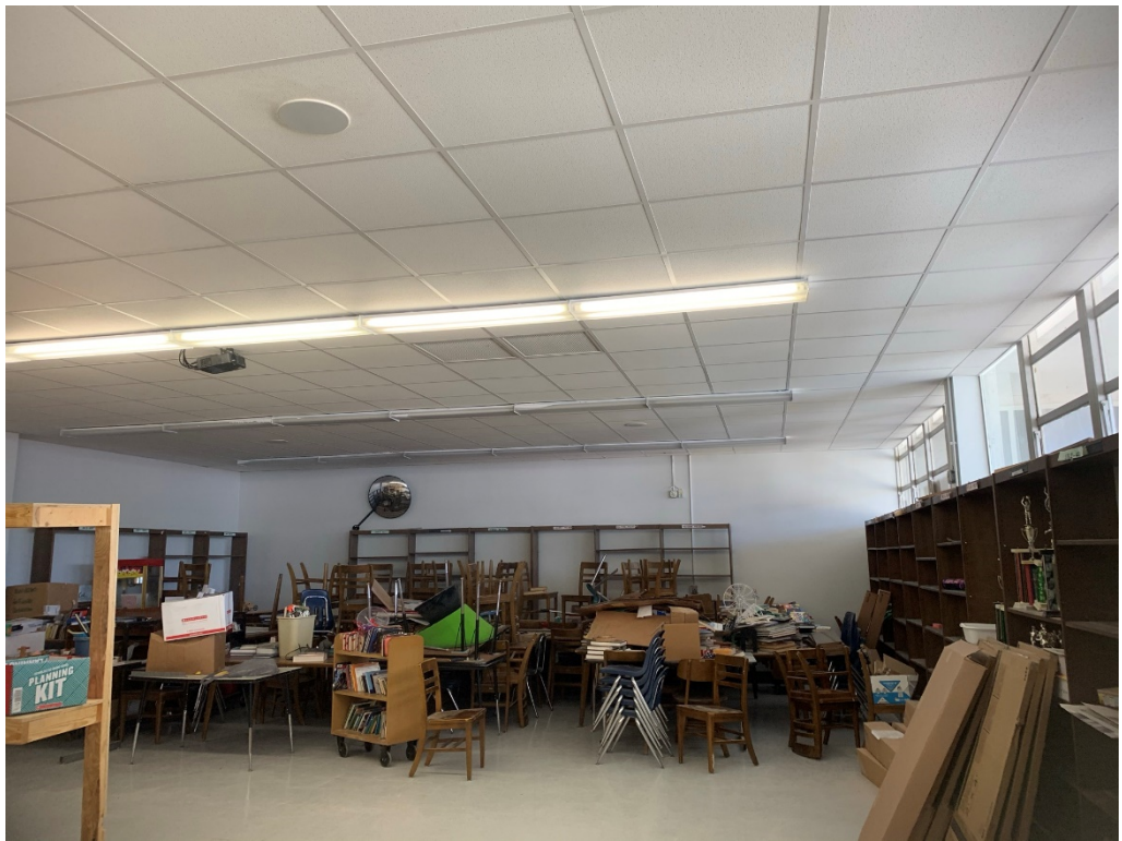
Figure 11 – New Ceiling in Library
