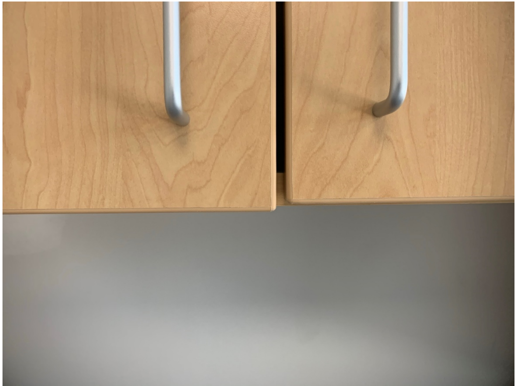
Figure 7 – Upper Millwork Doors Require Adjustment
