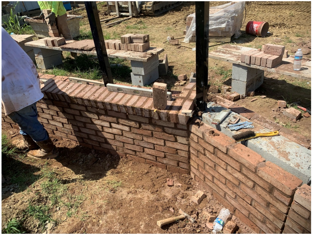
Figure 1 – Masonry is Ongoing
