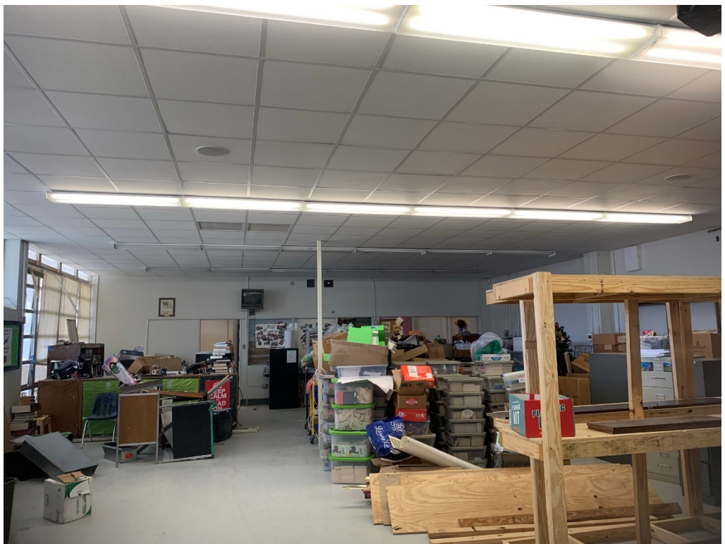
Figure 12 – New Ceiling in Library
