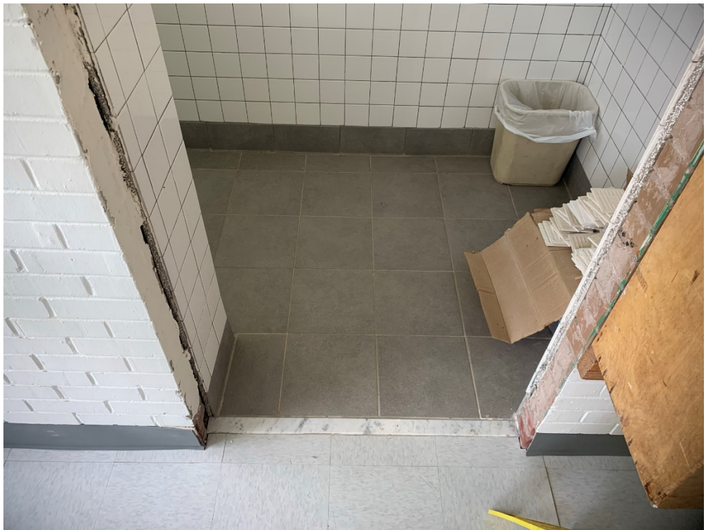
Figure 13 – Jambs Still to be Finished at Bathrooms
