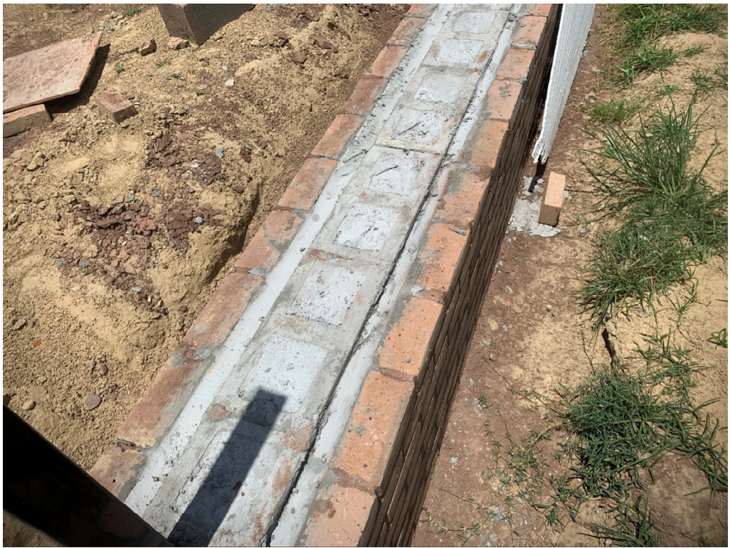
Figure 16 – Filled Block Wall
