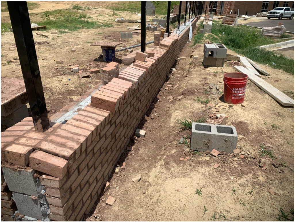
Figure 15 – Masonry Work at Low Fence
