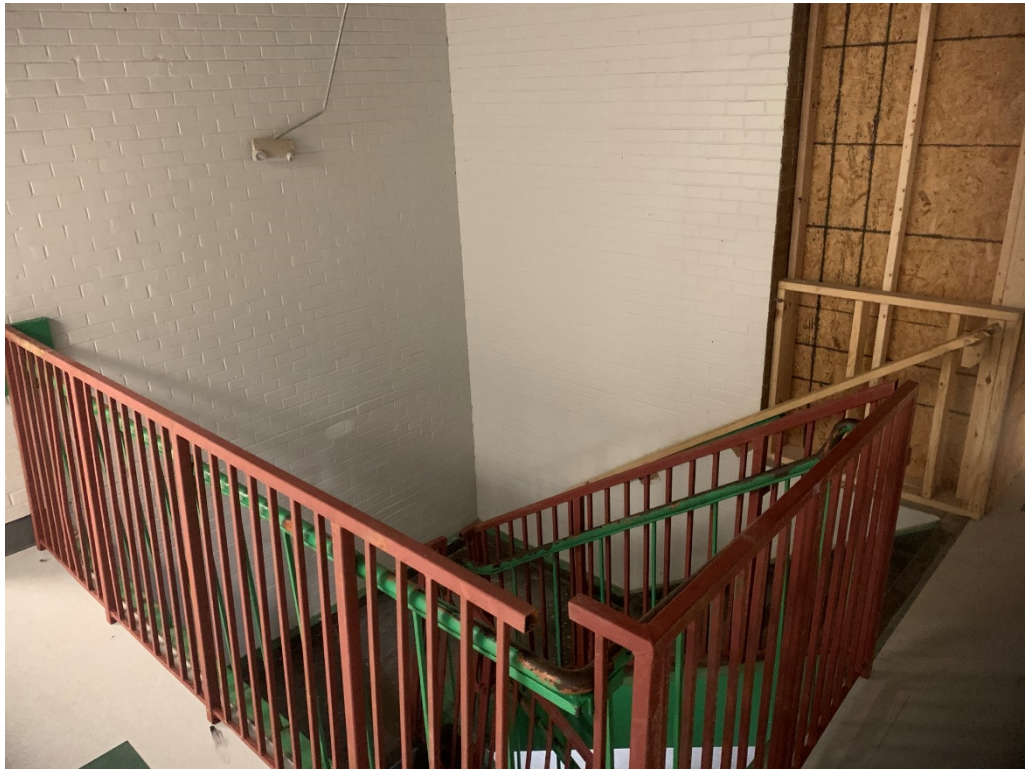
Figure 11 – Metal Railing being fitted
