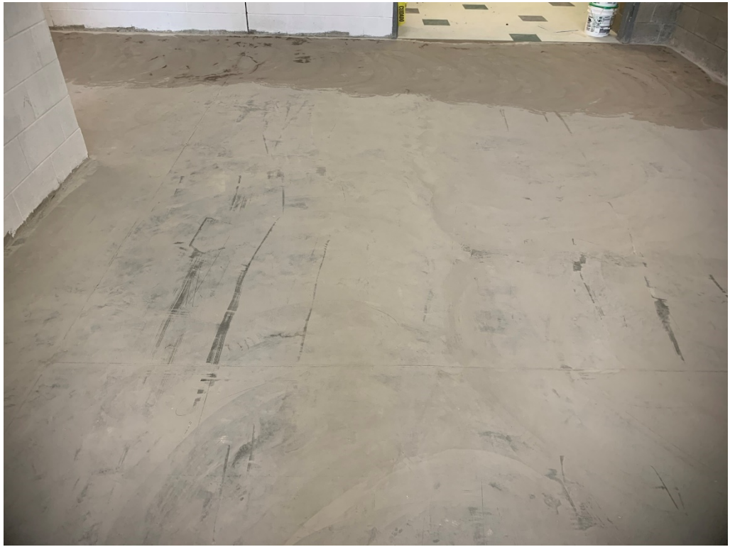
Figure 5 – Floor Prep at Addition
