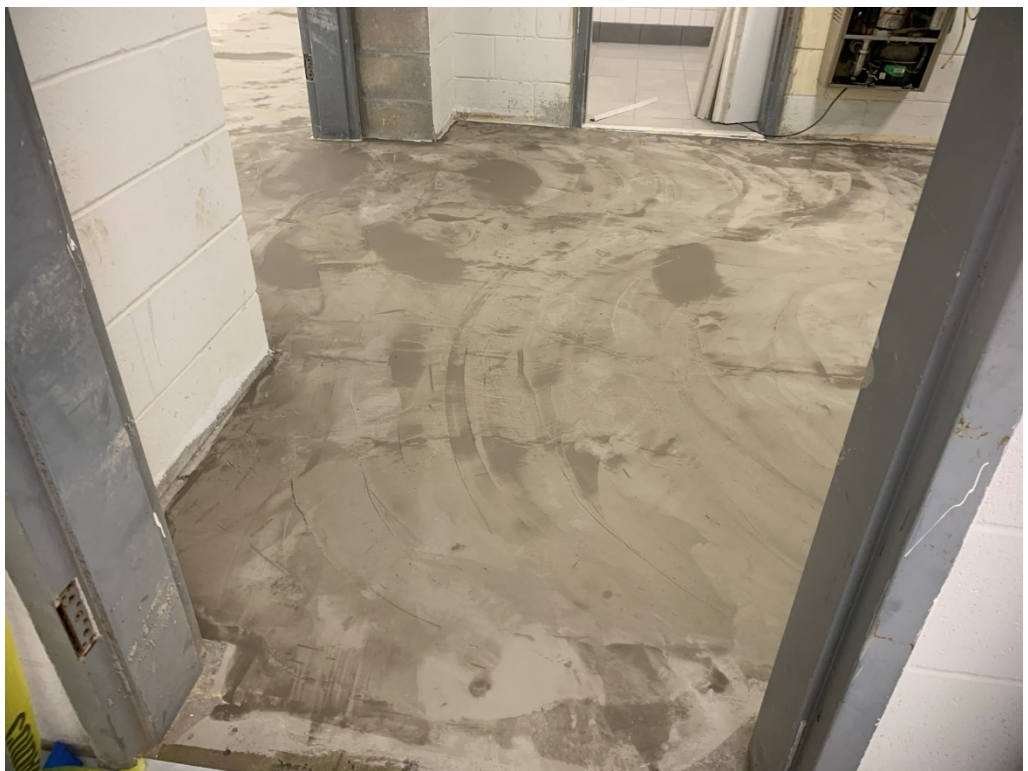
Figure 8 – Flooring Levelled Up and Ready for VCT
