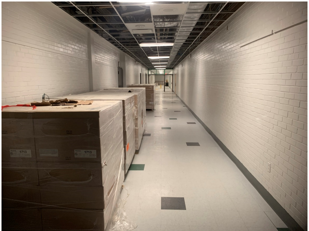
Figure 10 – Ceiling Tile awaiting Installation
