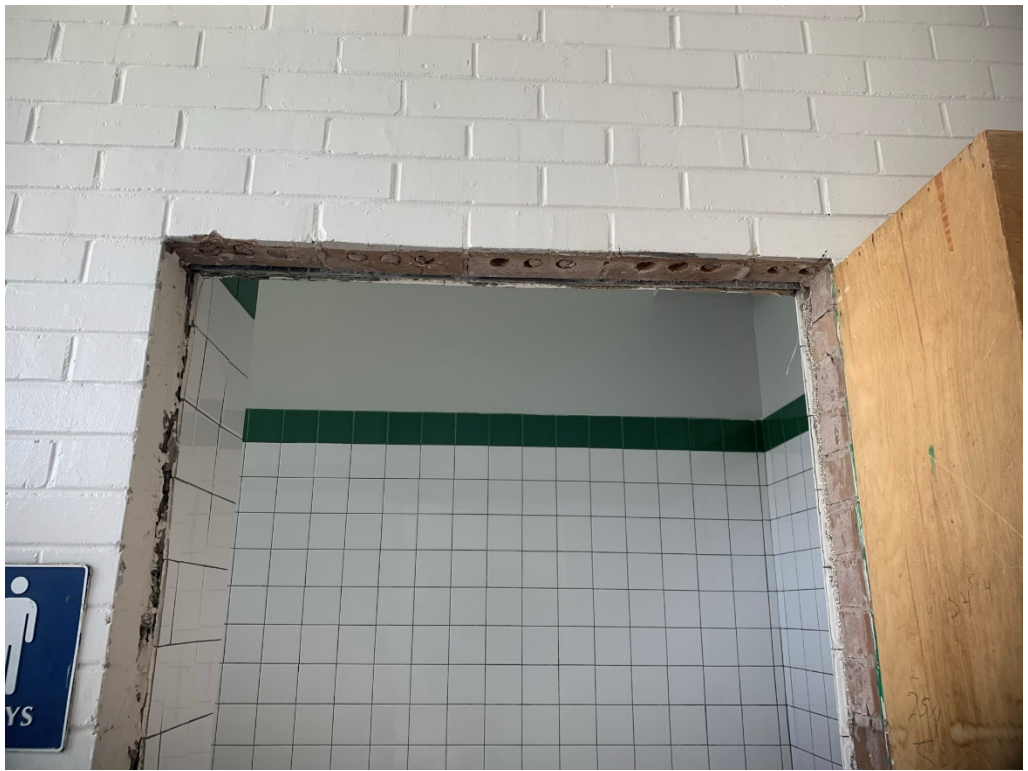
Figure 12 – Jambs Still to be Finished at Bathrooms
