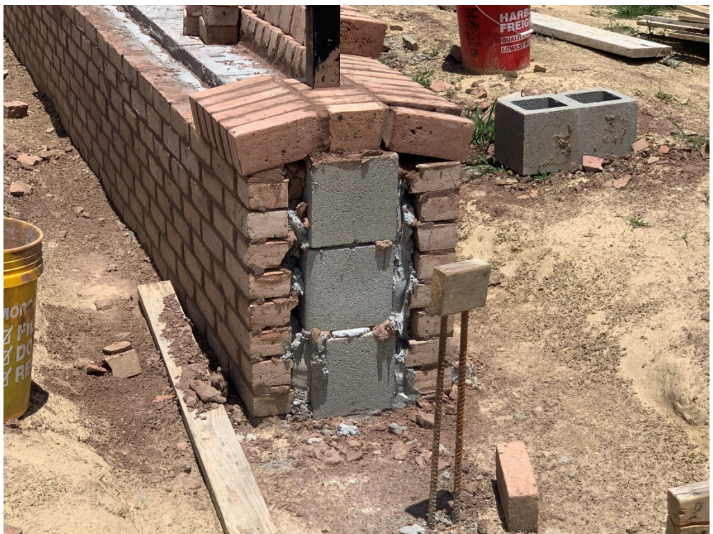
Figure 14 – Masonry Work at Low Fence
