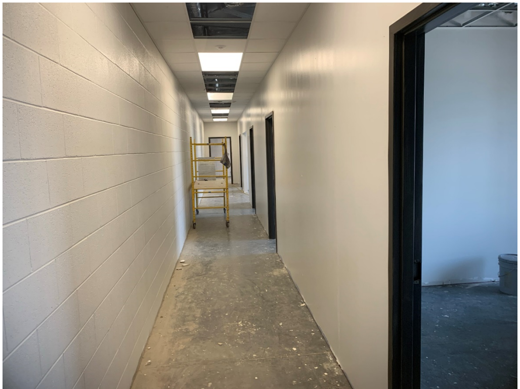
Figure 4 – Paint at office Nearing Completion
