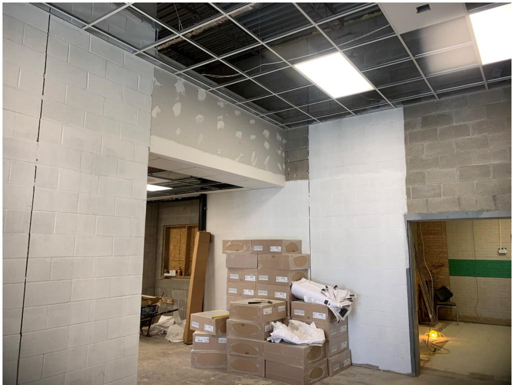
Figure 2 – Bulk Head Finishing Work
