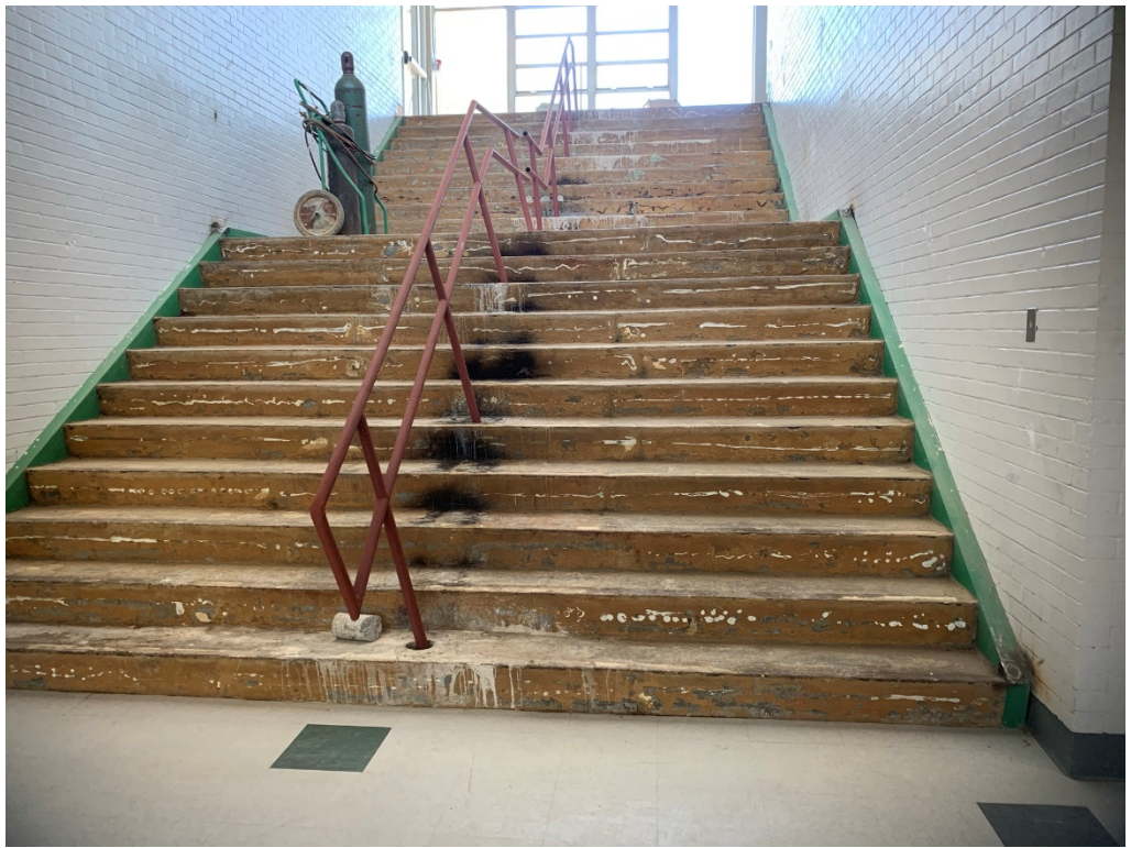
Figure 6 – Rail Installation is Ongoing
