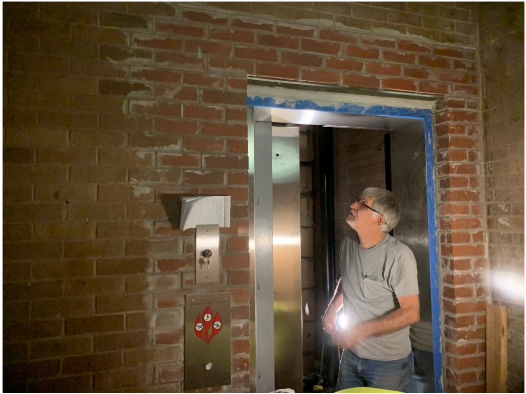
Figure 5 – Elevator Trim Install is Ongoing
