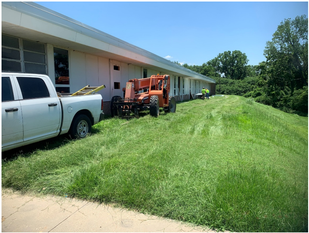
Figure 9 – Workers Installing panels
