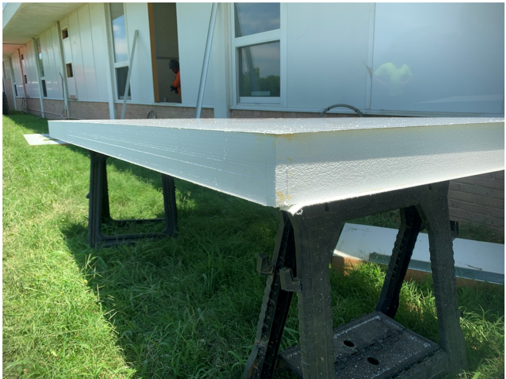
Figure 11 – Foam Panel (cut on site to fit)
