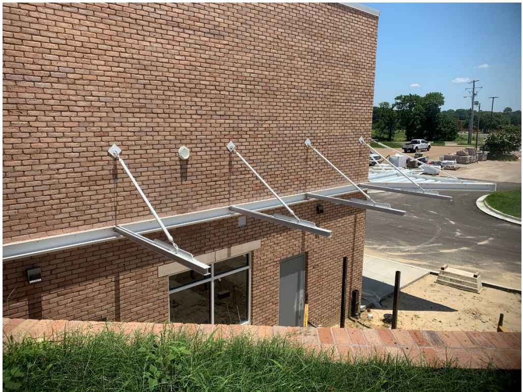
Figure 5 – Awning Install is Ongoing
