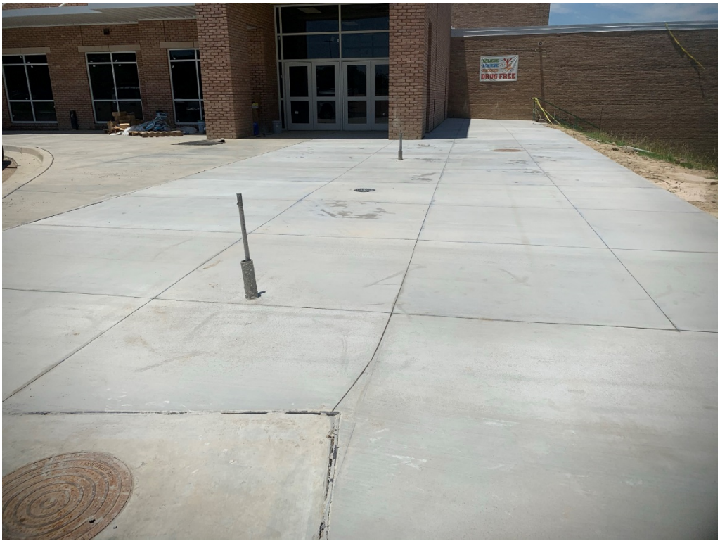
Figure 1 – New Concrete at Entry
