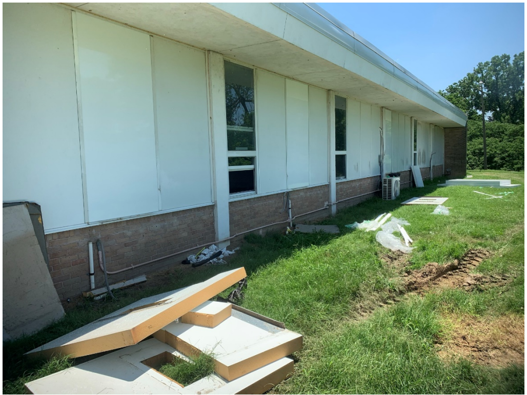
Figure 10 – New Panel Installations
