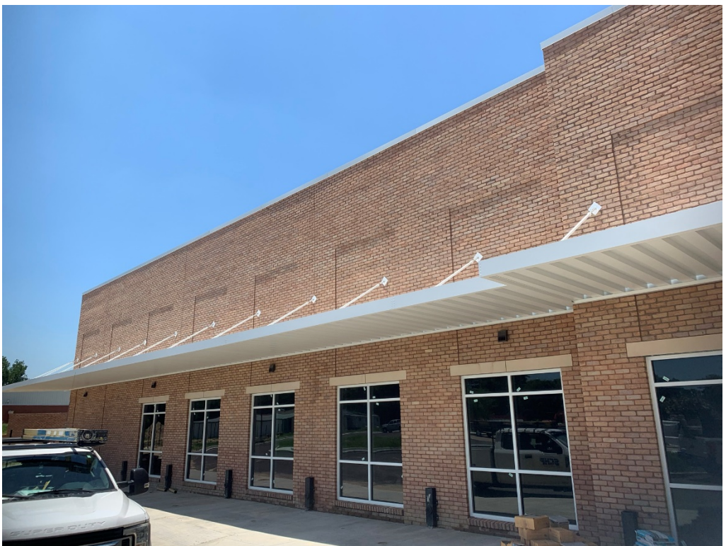
Figure 4 – Majority of Awning has been installed
