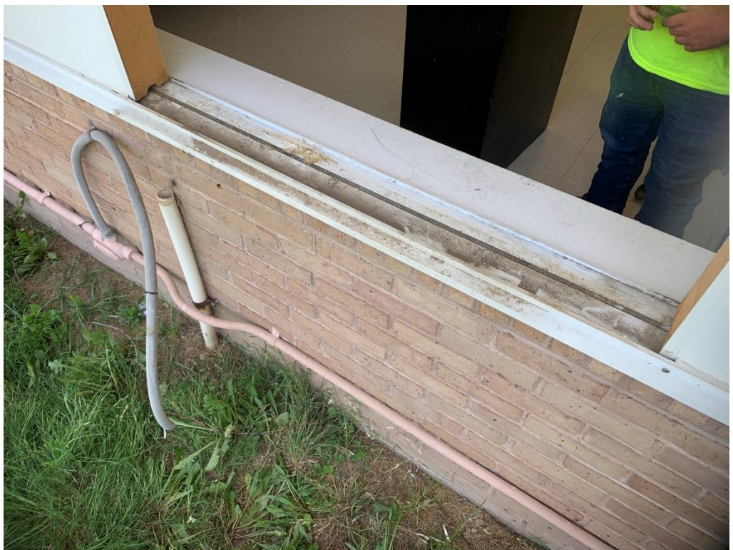
Figure 12 – Bottom of Opening Before Panel Install
