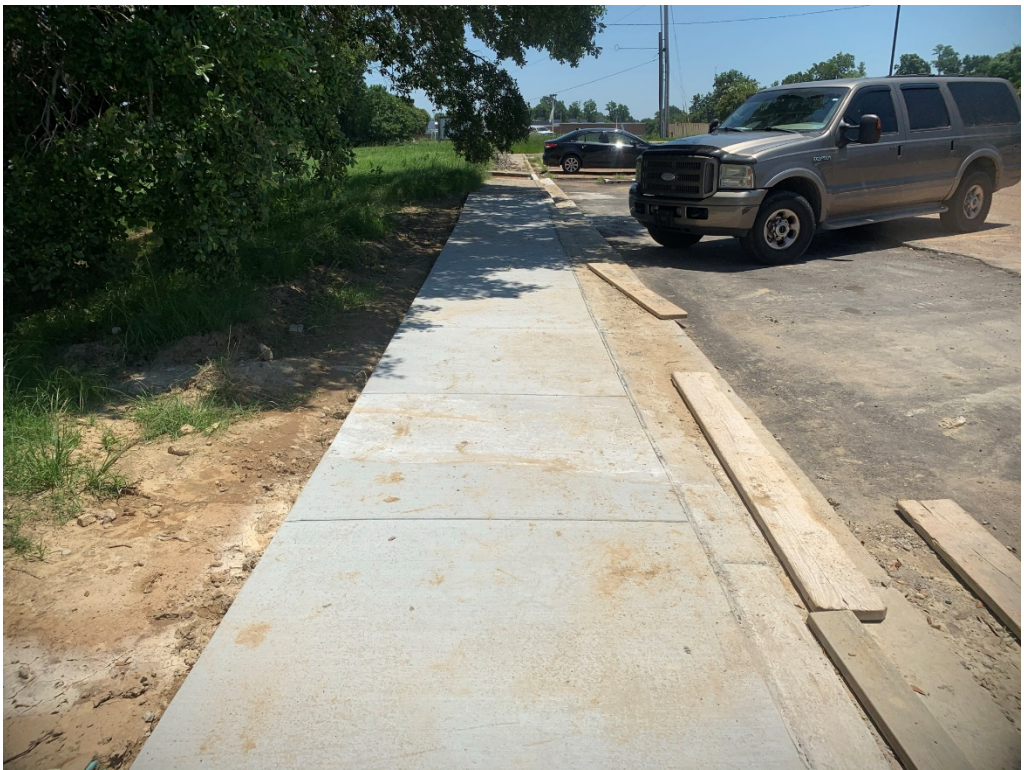
Figure 2 – New Concrete at Sidewalk
