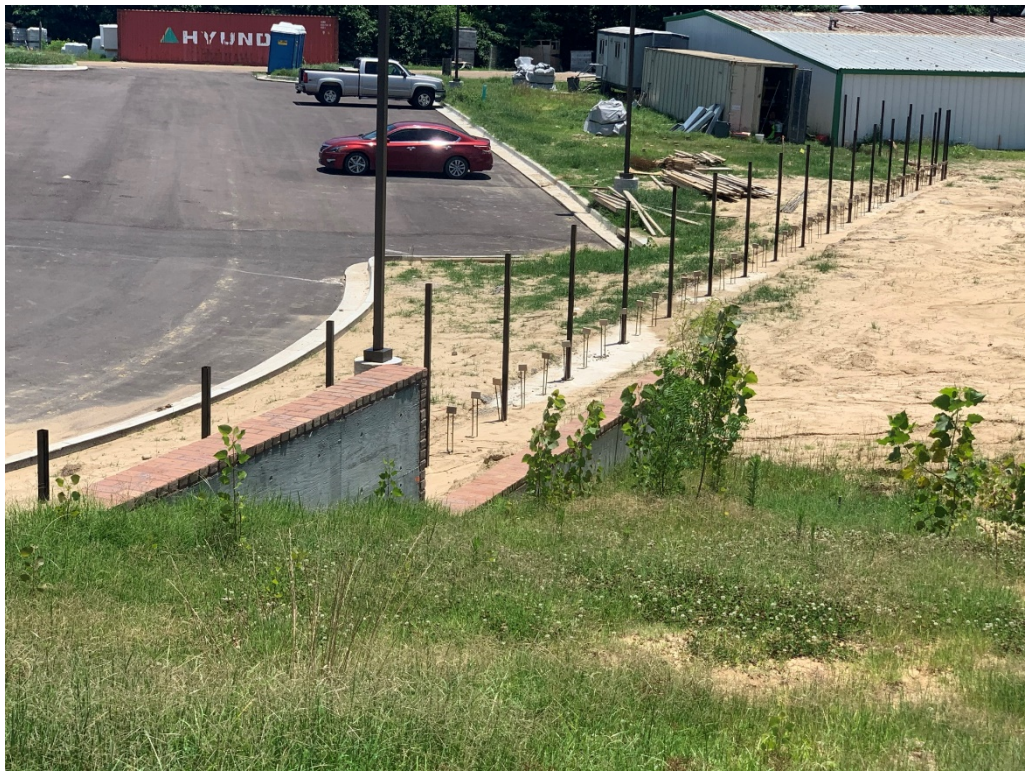
Figure 7 – Fence Posts Installed
