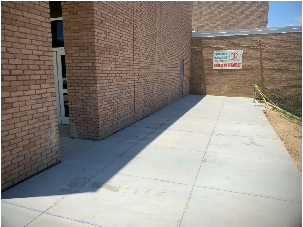
Figure 3 – New Concrete at Entry
