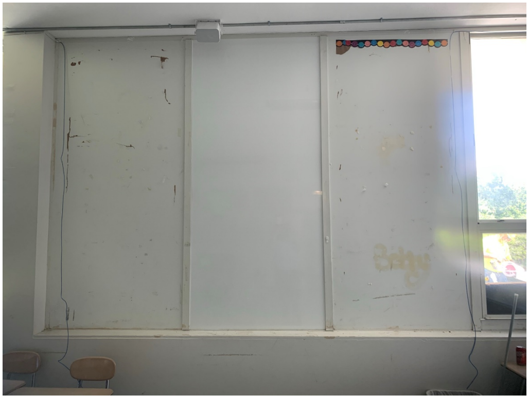
Figure 14 – Typical Installation of New Panels
