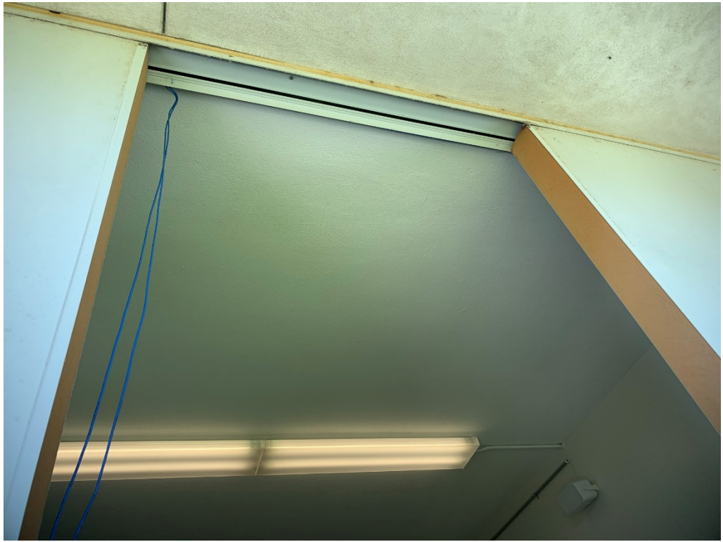
Figure 13 – Top of Opening Before Panel Install
