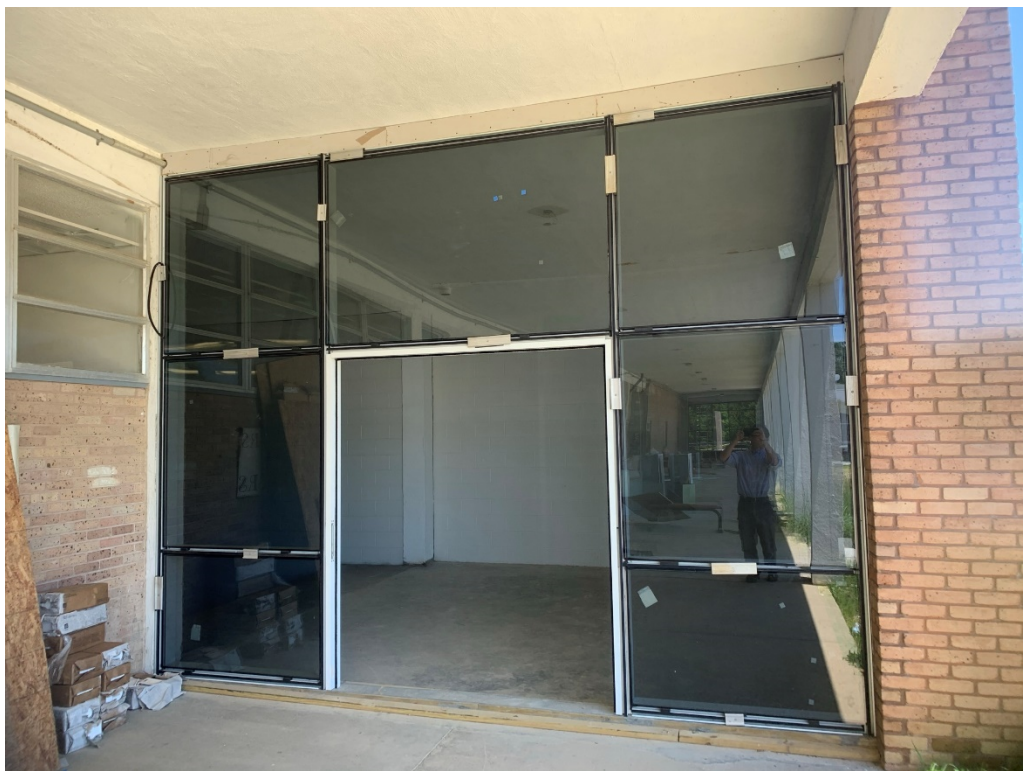
Figure 6 – Curtain Wall Progress at Upper Floor Entry
