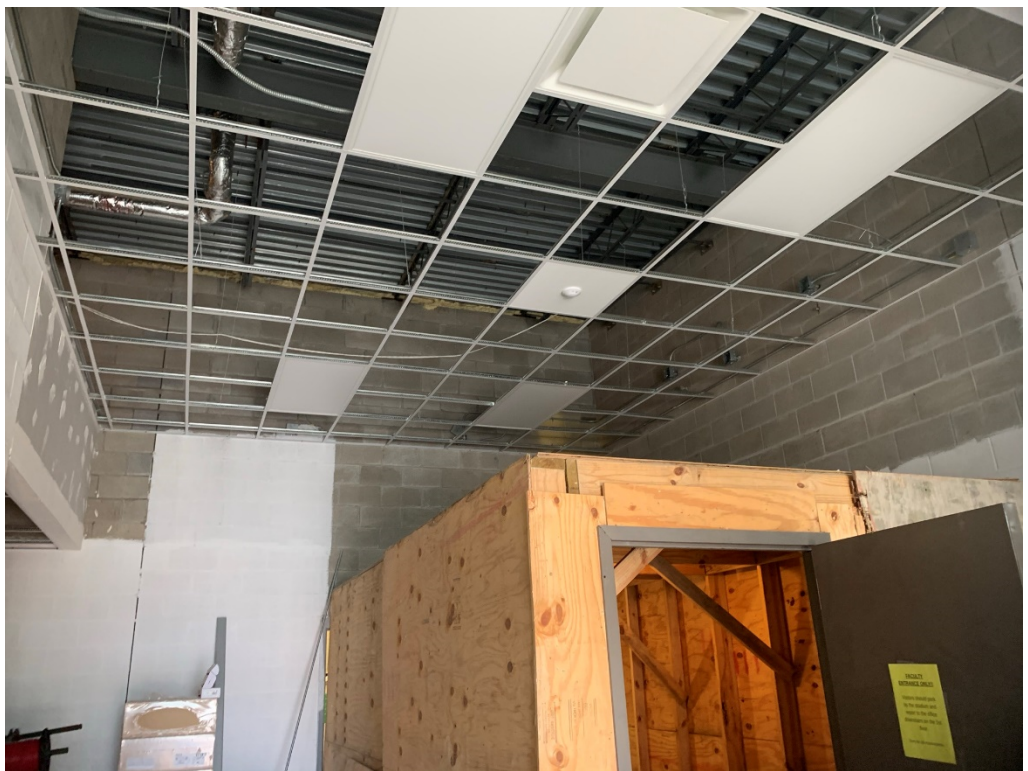
Figure 6 – Ceiling Grid Install at Entry
