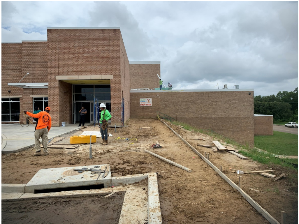
Figure 1 – Roof Work is nearing completion
