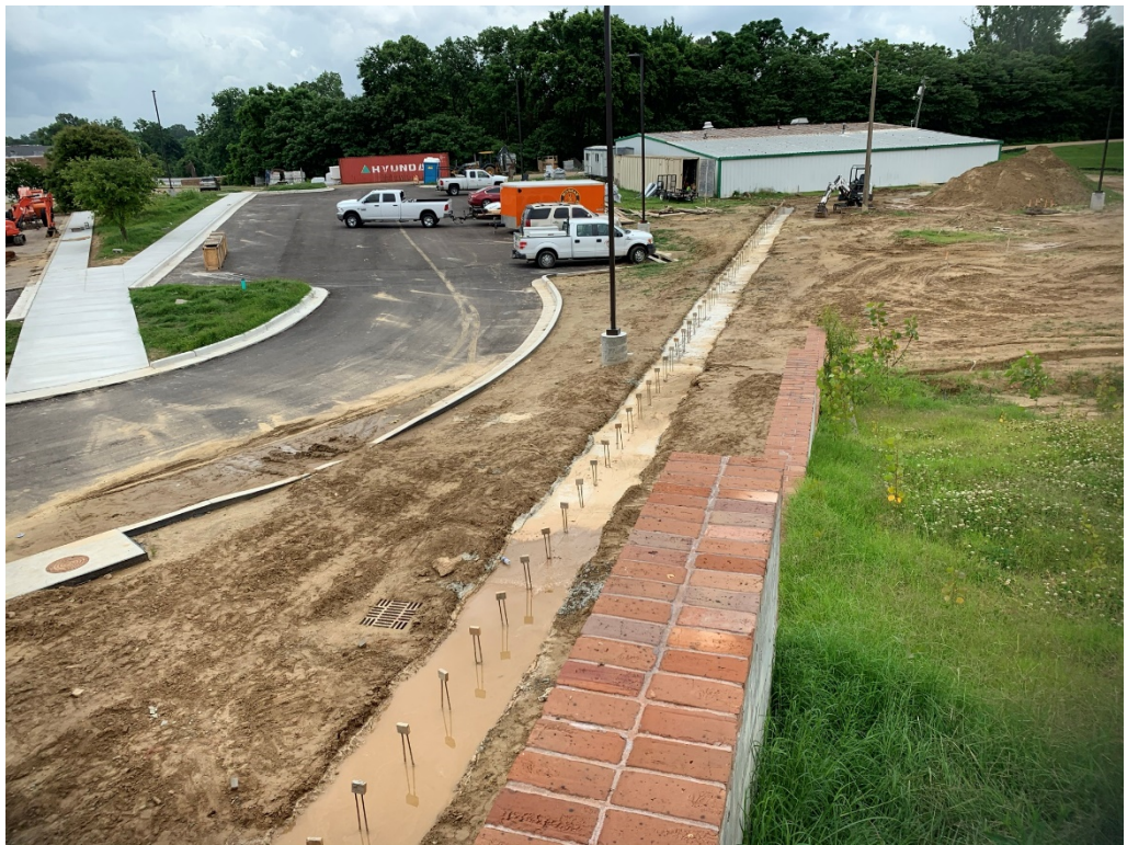
Figure 13 – New Sidewalk Base
