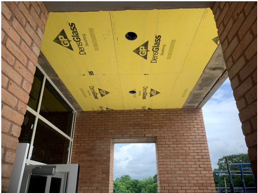
Figure 5 – Gypsum Ceiling Installed
