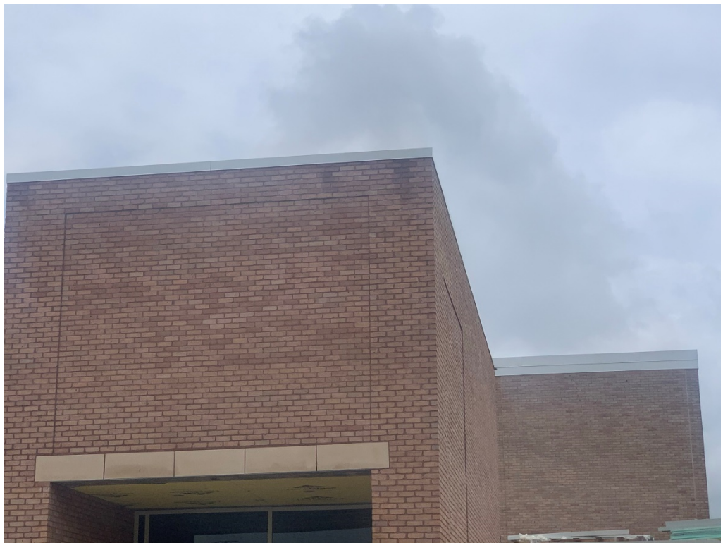
Figure 2 – Roof Trim Installed at parapet
