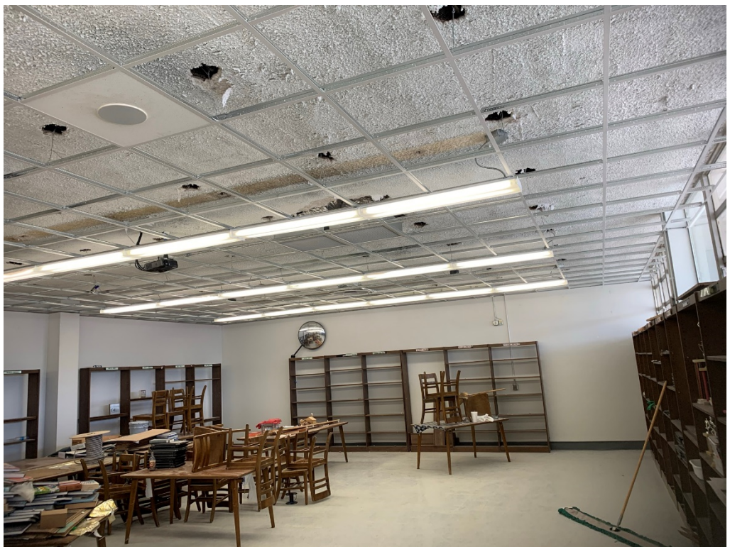
Figure 12 – New Ceiling in Library
