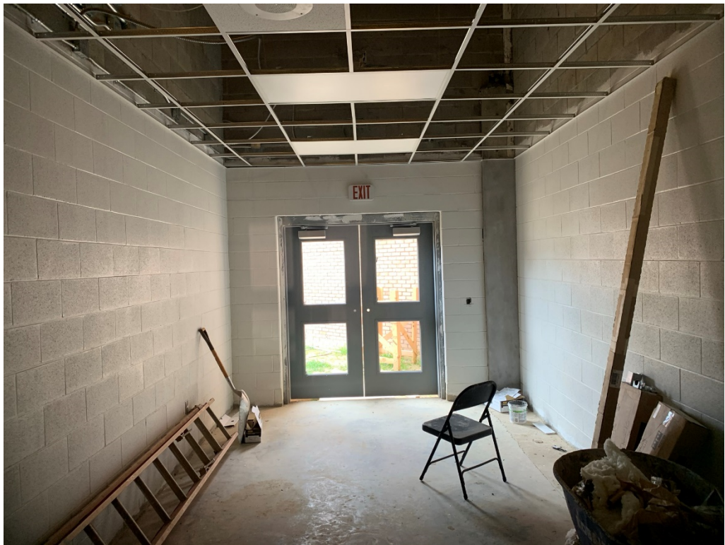
Figure 9 – Exit Doors Installed
