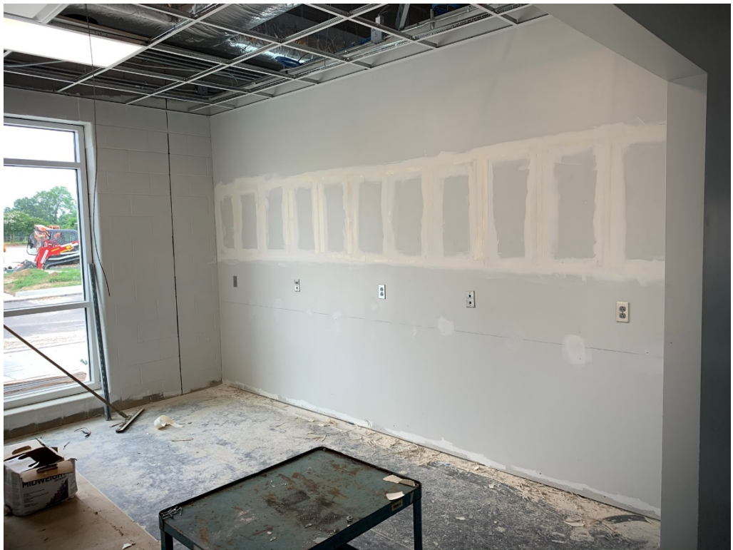
Figure 7 – Drywall Repair at Work Room
