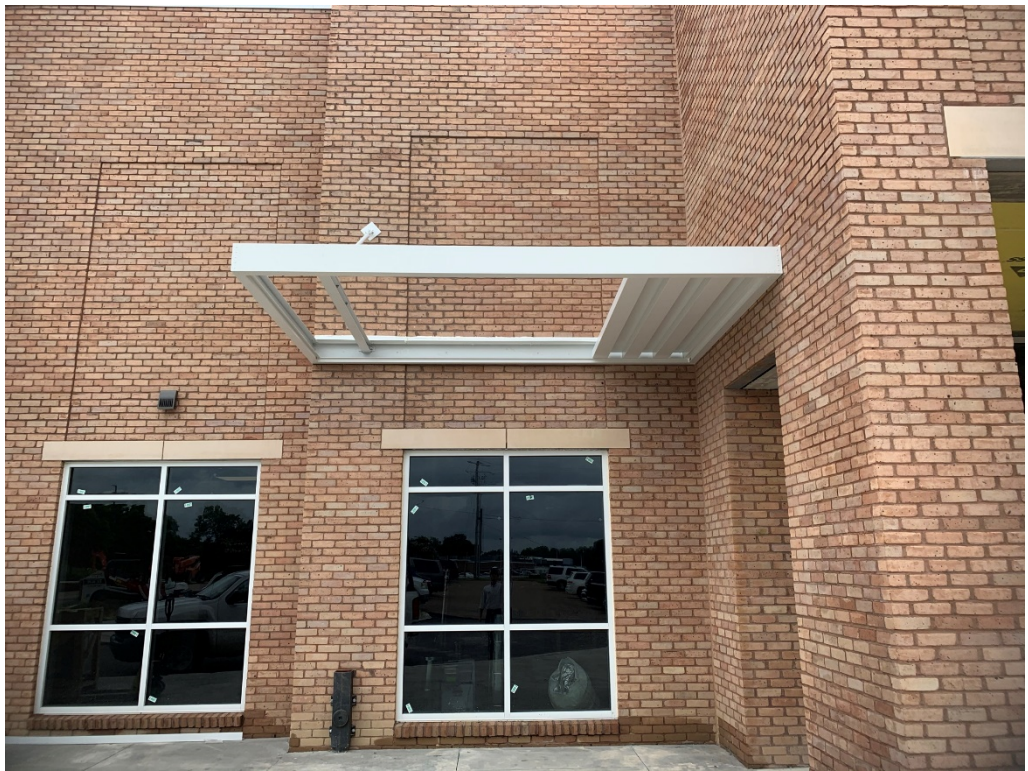
Figure 3 – Metal Awning Install has begun
