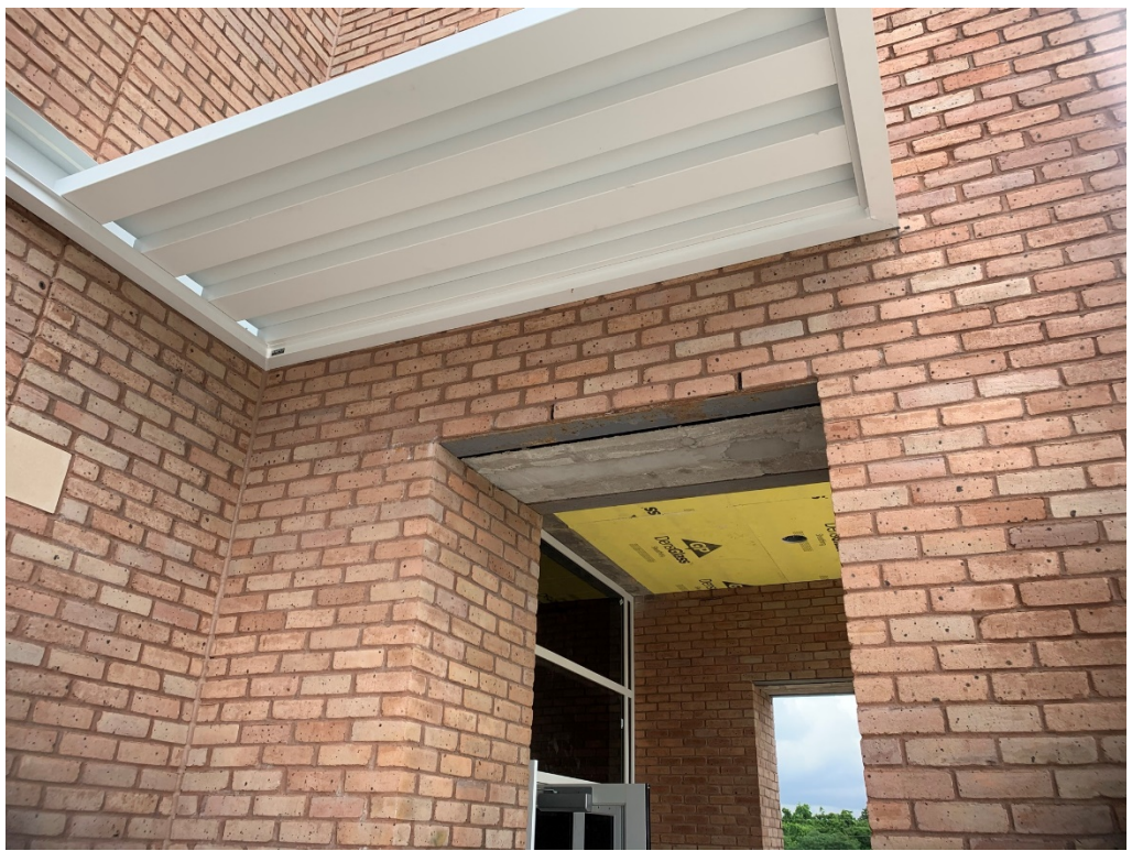
Figure 4 – Metal Awning Install has begun
