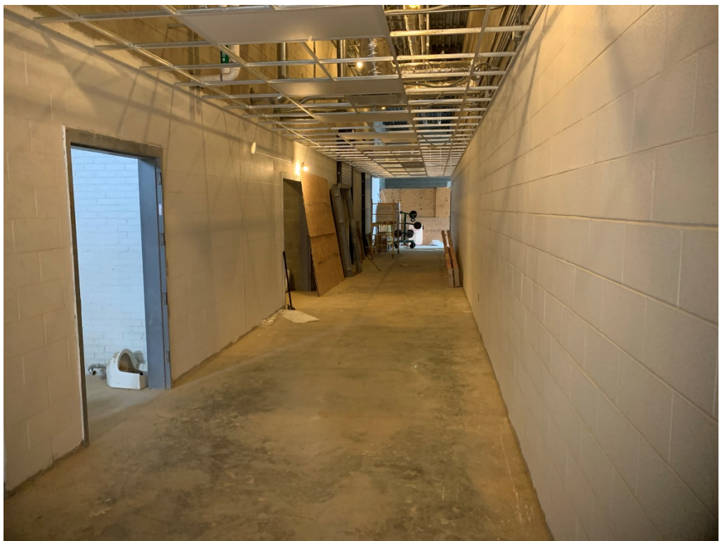
Figure 8 – Ceiling Grid installed at Hall
